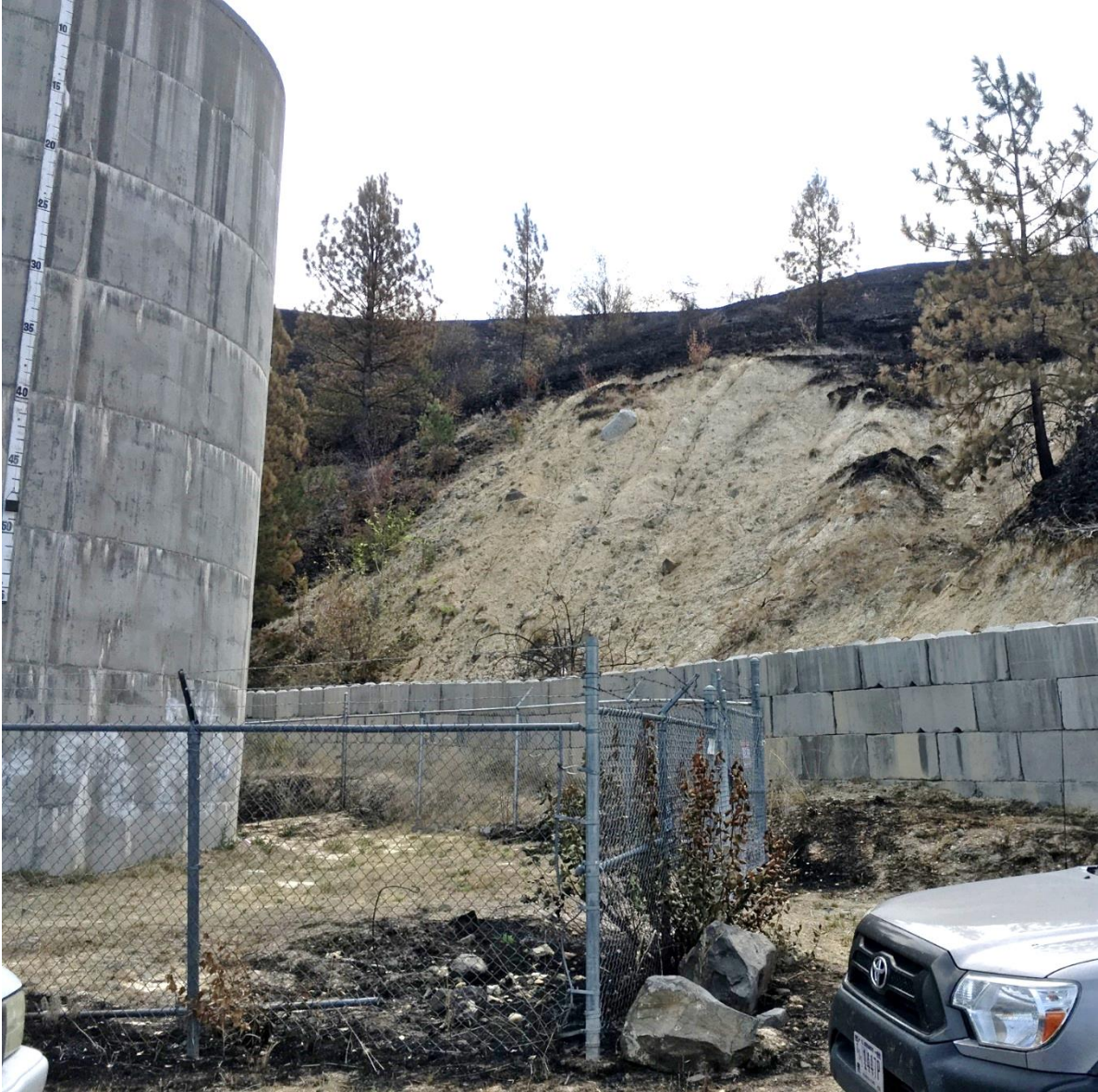
Figure 3. Landslide with glacial diamict exposed behind wall and light-colored sediment deposited within security fence.
