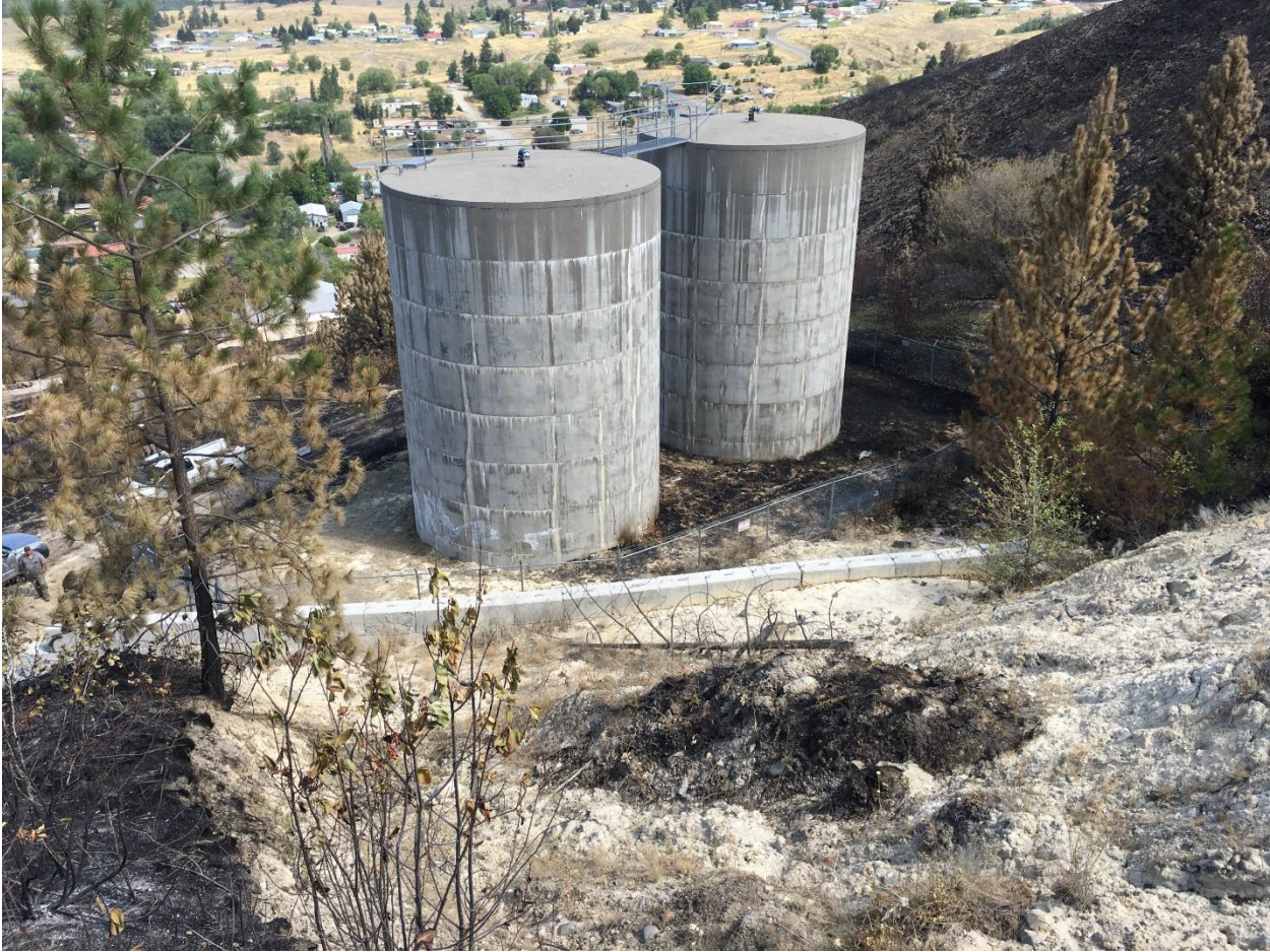
Figure 2. Retaining wall made of ecology blocks behind water tanks, approximately 15 feet from the western tank. Photo shows recent sediment deposited against the wall.
