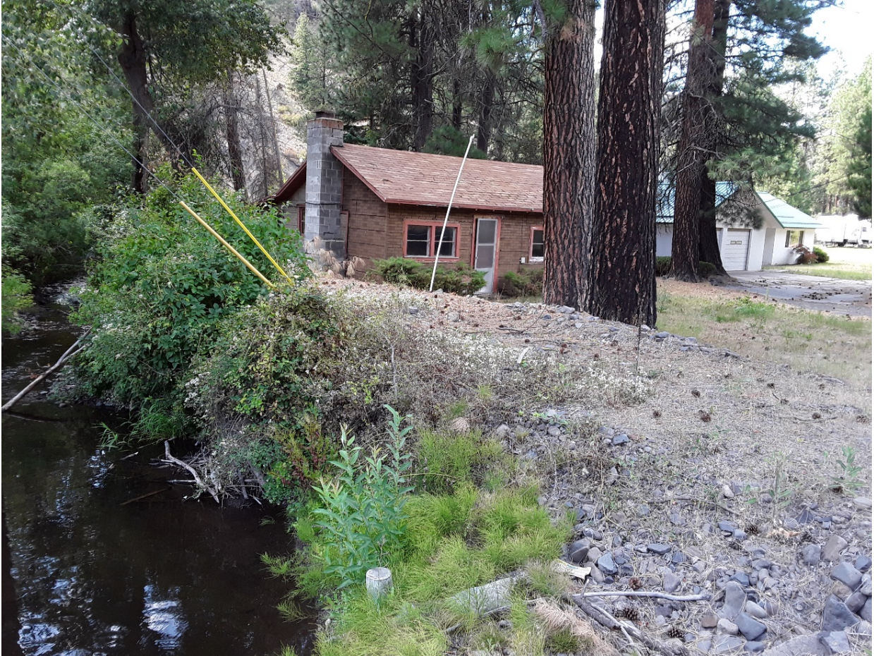
Figure 5. Home at 14710 WA-410 downstream of box culvert under SR410 along Rock Creek. Note berm built to protect house. Site 1 on Figure 2.
