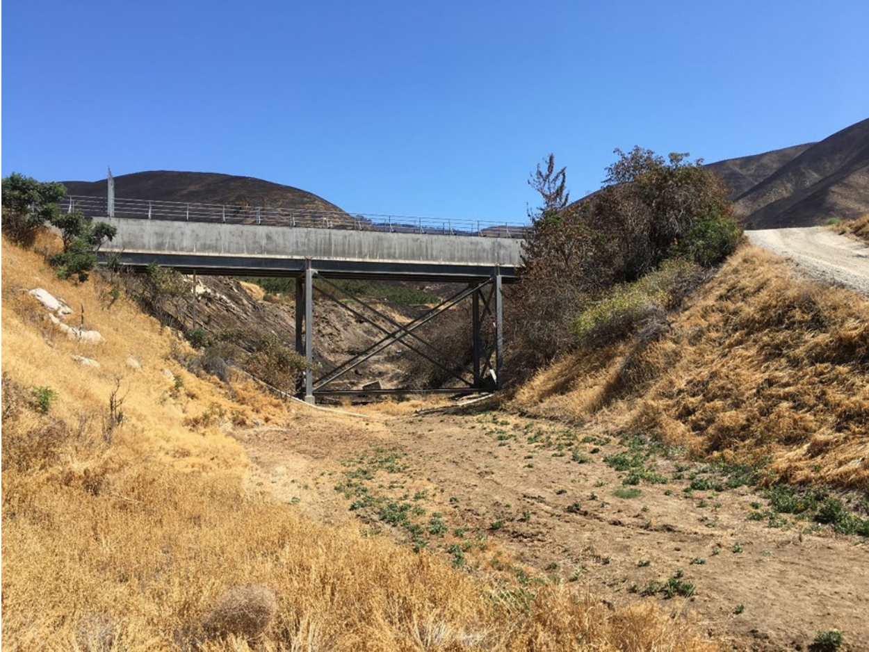
Figure 1. Photo taken where irrigation canal crosses unnamed drainage in a flume with high combined hazard for debris flows. This location is above the intersection of Kenoyer and Red Apple Roads (Location 4 on Plate 1).
