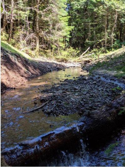
Figure 2. Bear Creek culvert after removal.
