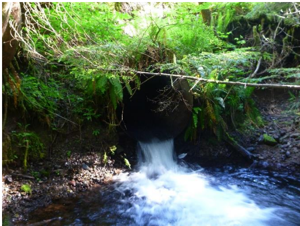
Figure 1. Bear Creek culvert prior to removal.
