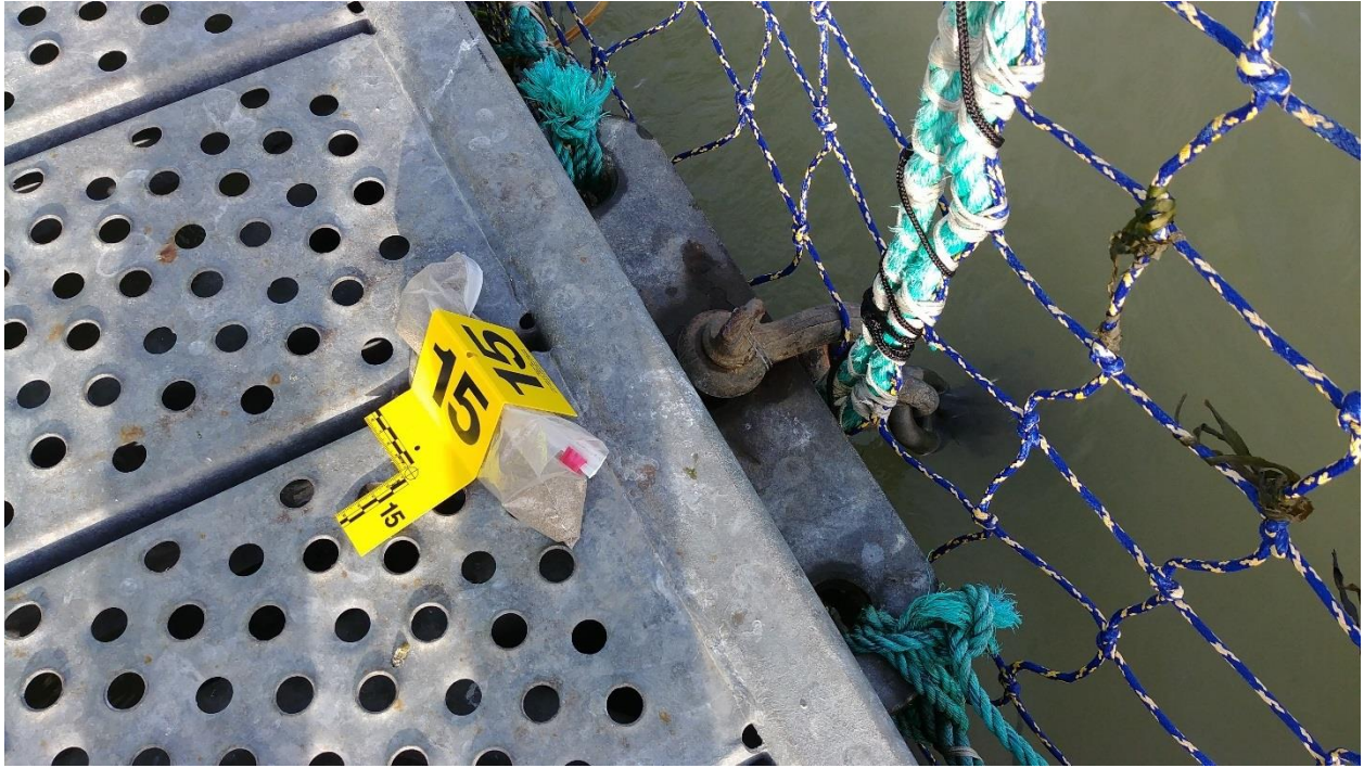
Figure C-48: Anchor #15, East Side of the Net Pens
