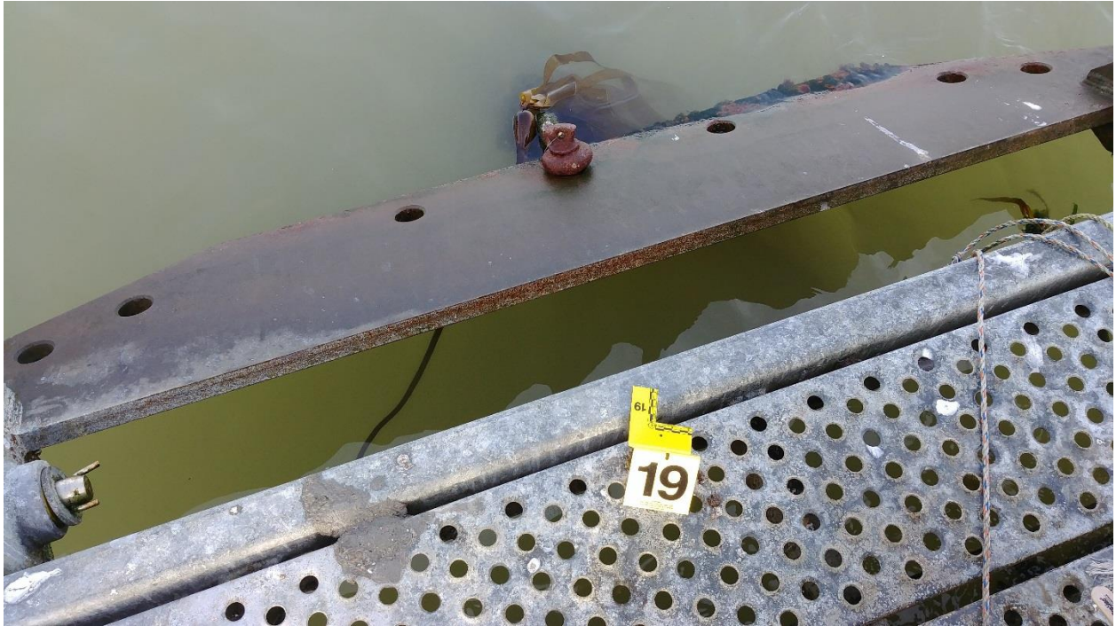
Figure C-56: Anchor #19, NE Corner of the Net Pens
