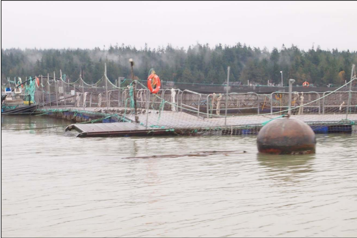
Photograph 11: View of the Depressed Pen Support Float at the Northwest Corner, Looking Southeast.
