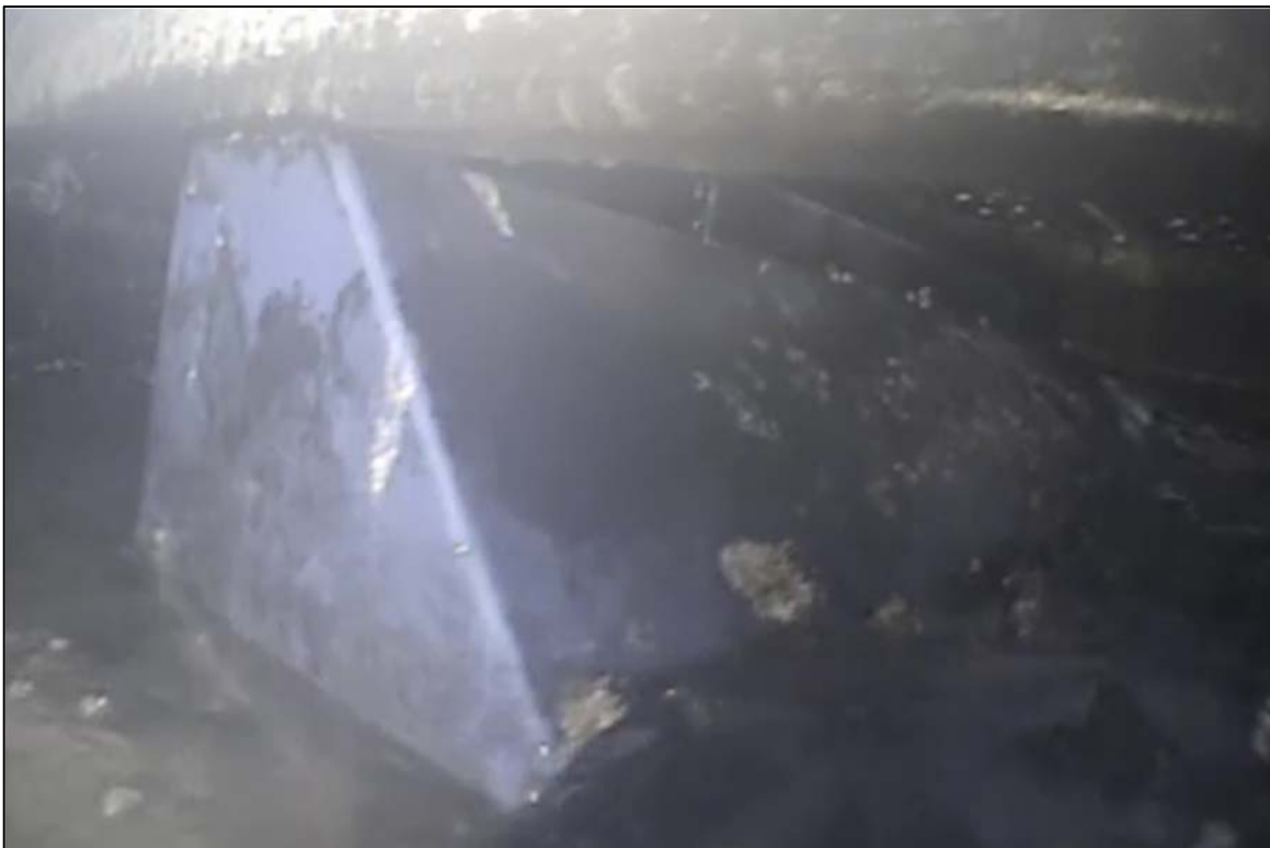
Photograph 12: View of the Northwest Corner Pen Support Float, Looking Southeast.
