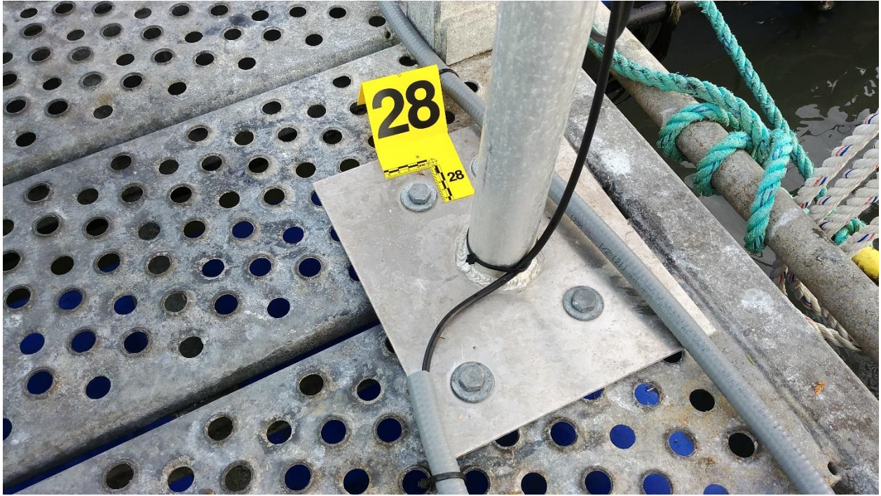
Figure C-72: Dissimilar Metals
