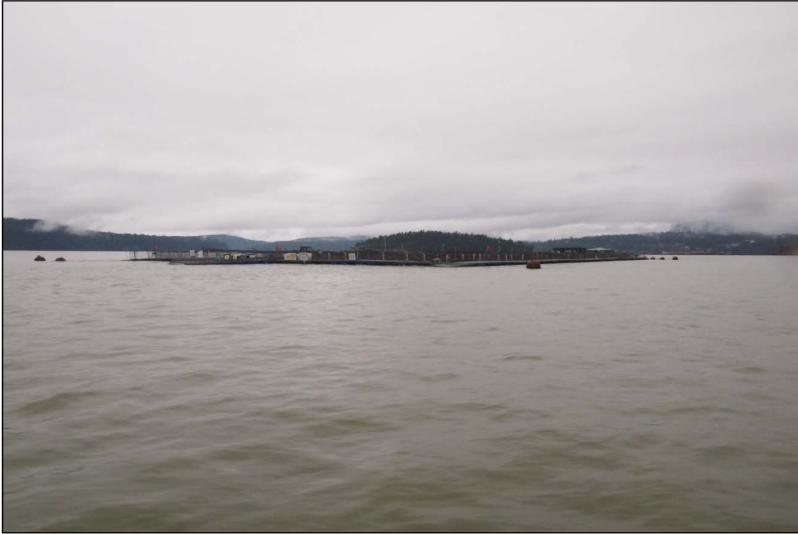
Photograph 5: Overall View of the Fish Net Pen System, Looking Northwest.
