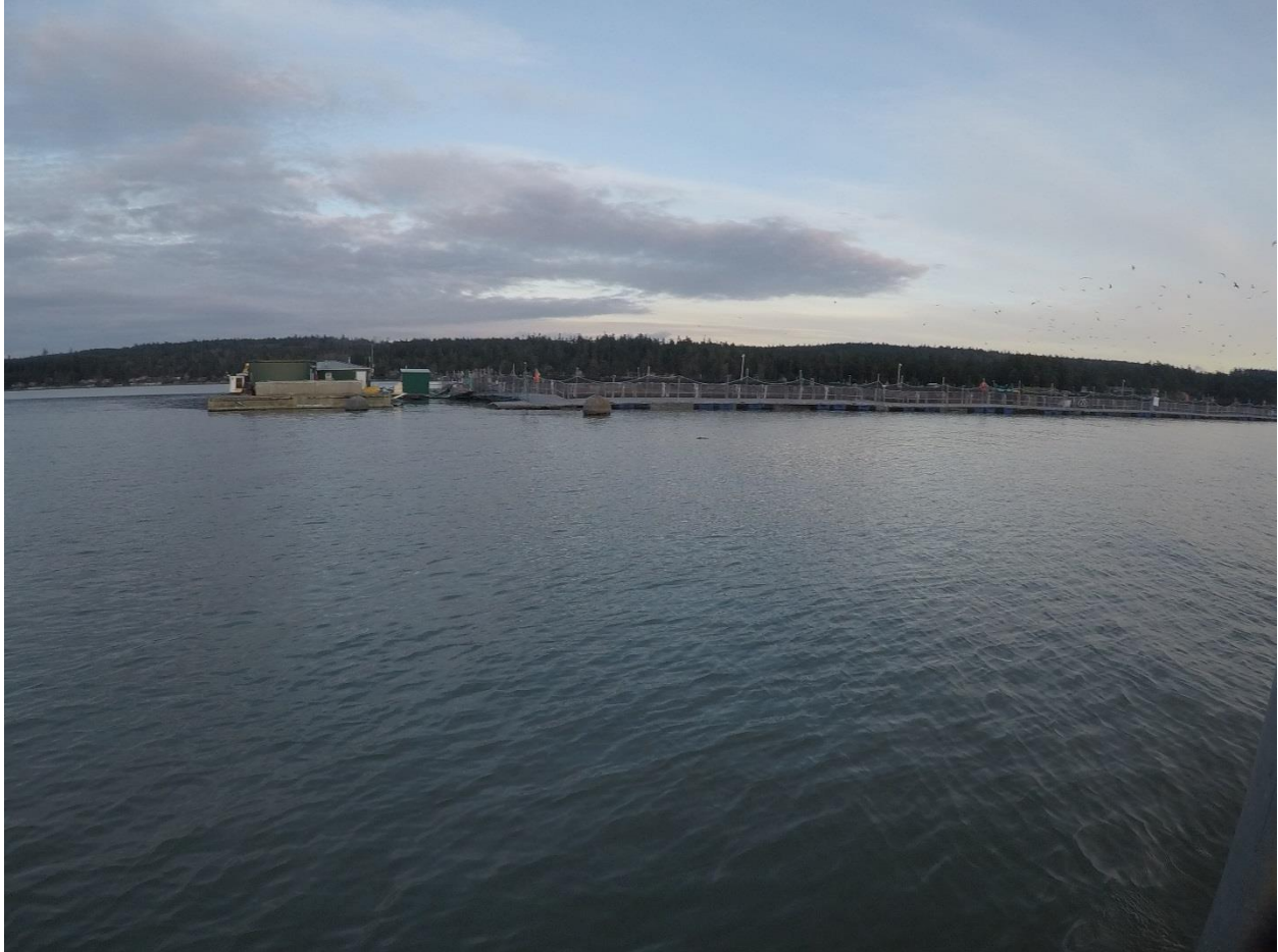
Figure C-2: Hope Island Net Pens - Overview from NW
