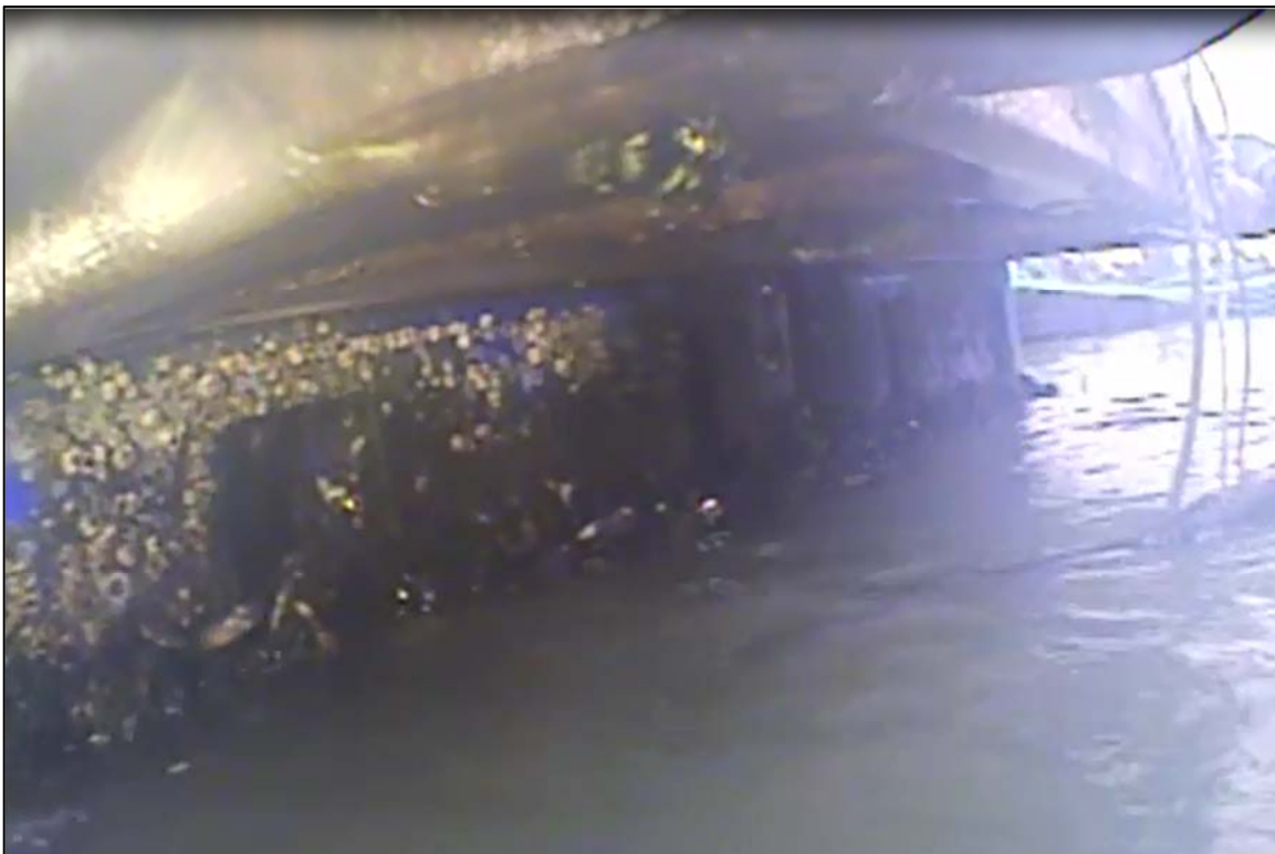
Photograph 14: View of the Northeast Corner Pen Support Float, Looking Southwest.
