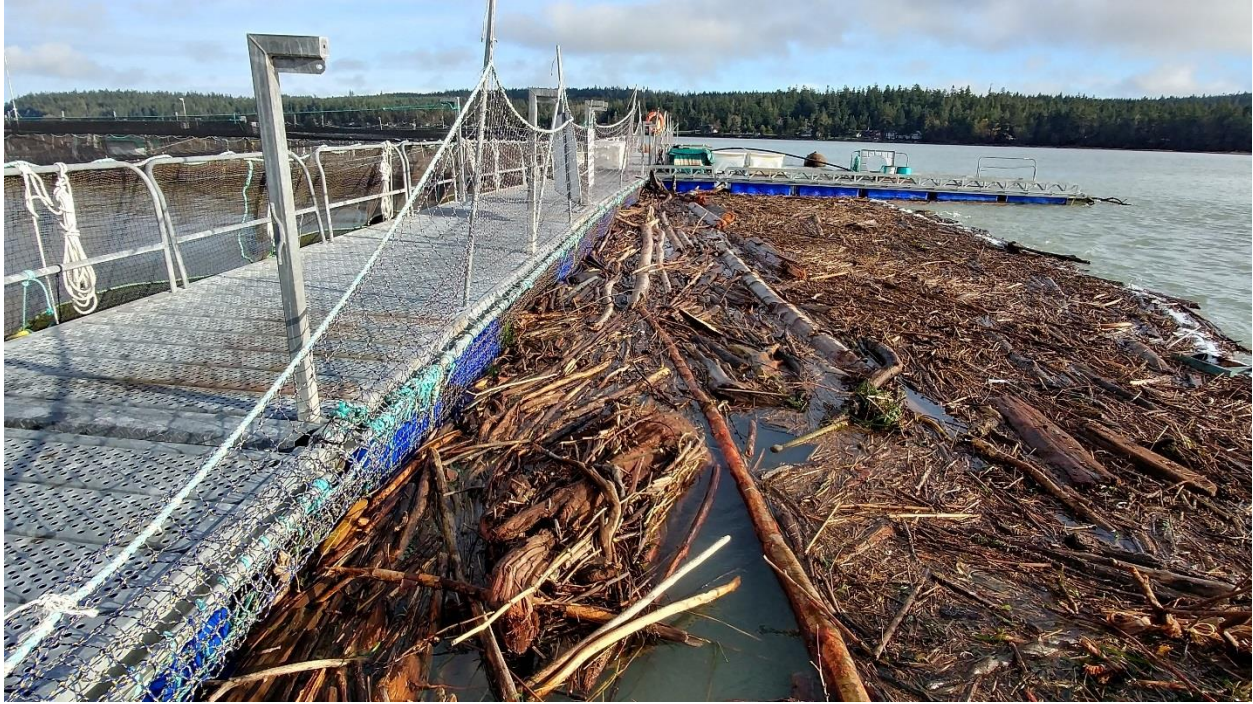
Figure C-14: Hope Island Net Pens - Debris Buildup on South End, Looking East
