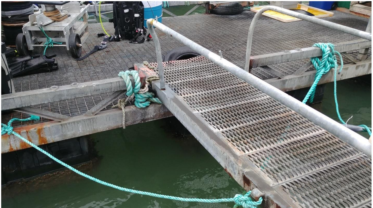
Figure C-85: Gangway Connecting Dive Float to Main Barge. Note No attachment, only Bearing.
