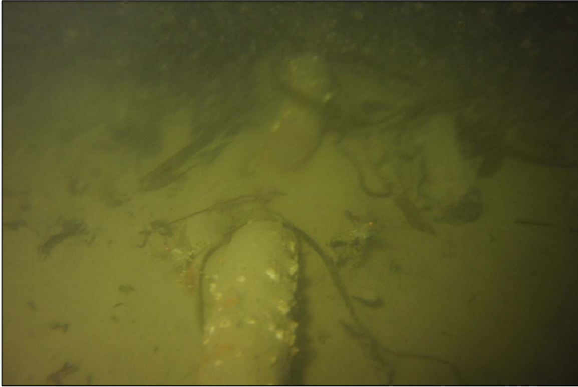
Photograph 37: View of Lower Anchor Chain on Channel Bottom at Anchor 15, Looking East.
