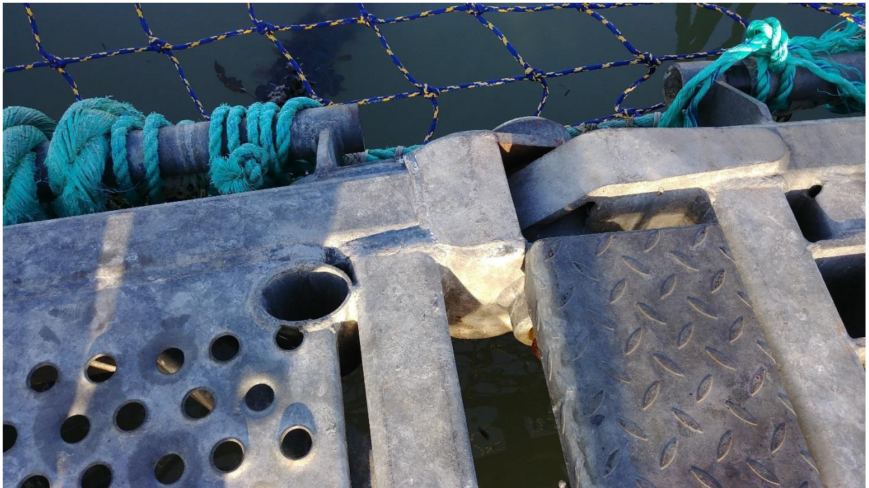
Figure C-95: Hinge between Segments of Main Walkways
