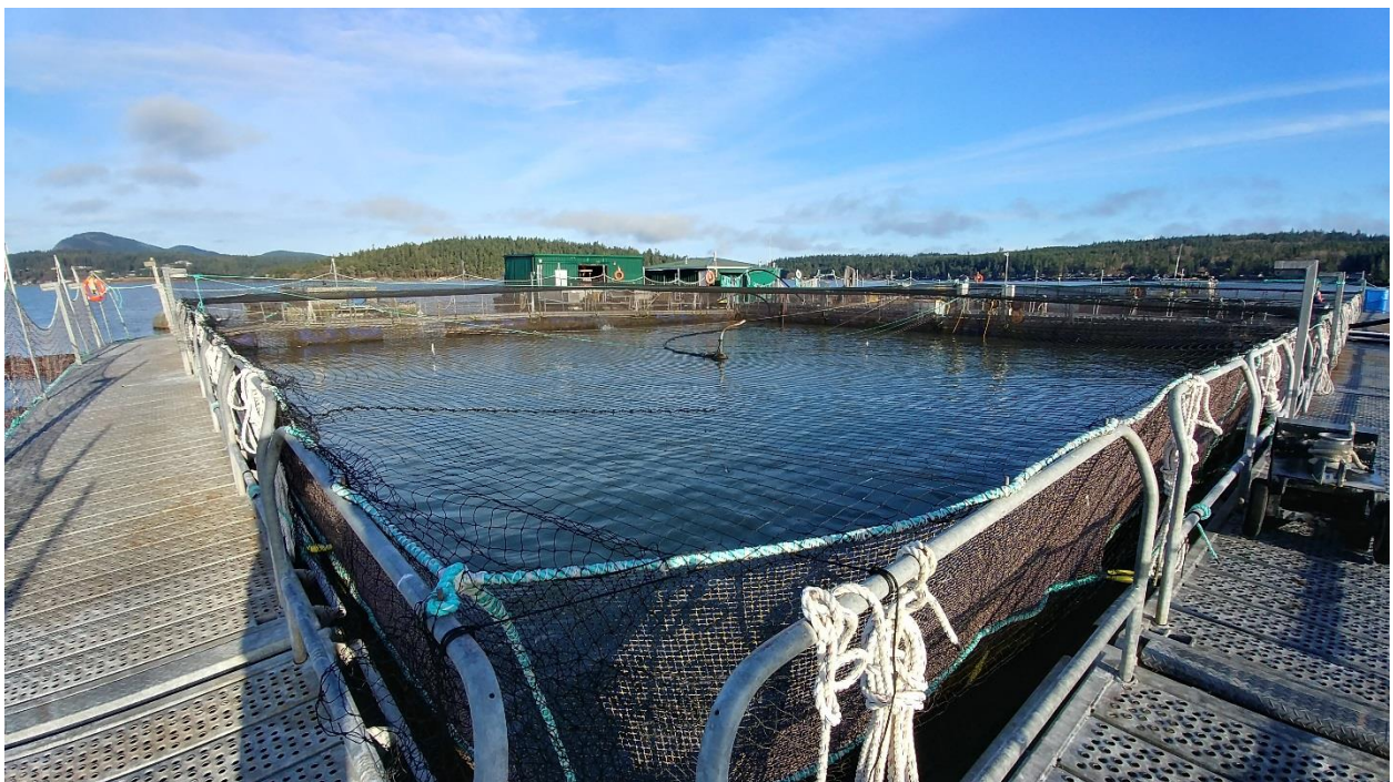
Figure C-7: Hope Island Net Pens - NW Corner of Pens, Looking North
