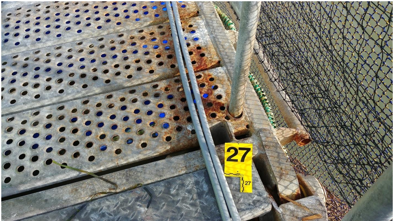
Figure C-71: Minor Corrosion
