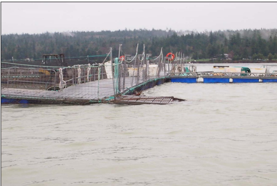
Photograph 18: View of the Depressed Pen Support Float (During High Ebb Tidal Flow) at the Southwest Corner, Looking Northeast.
