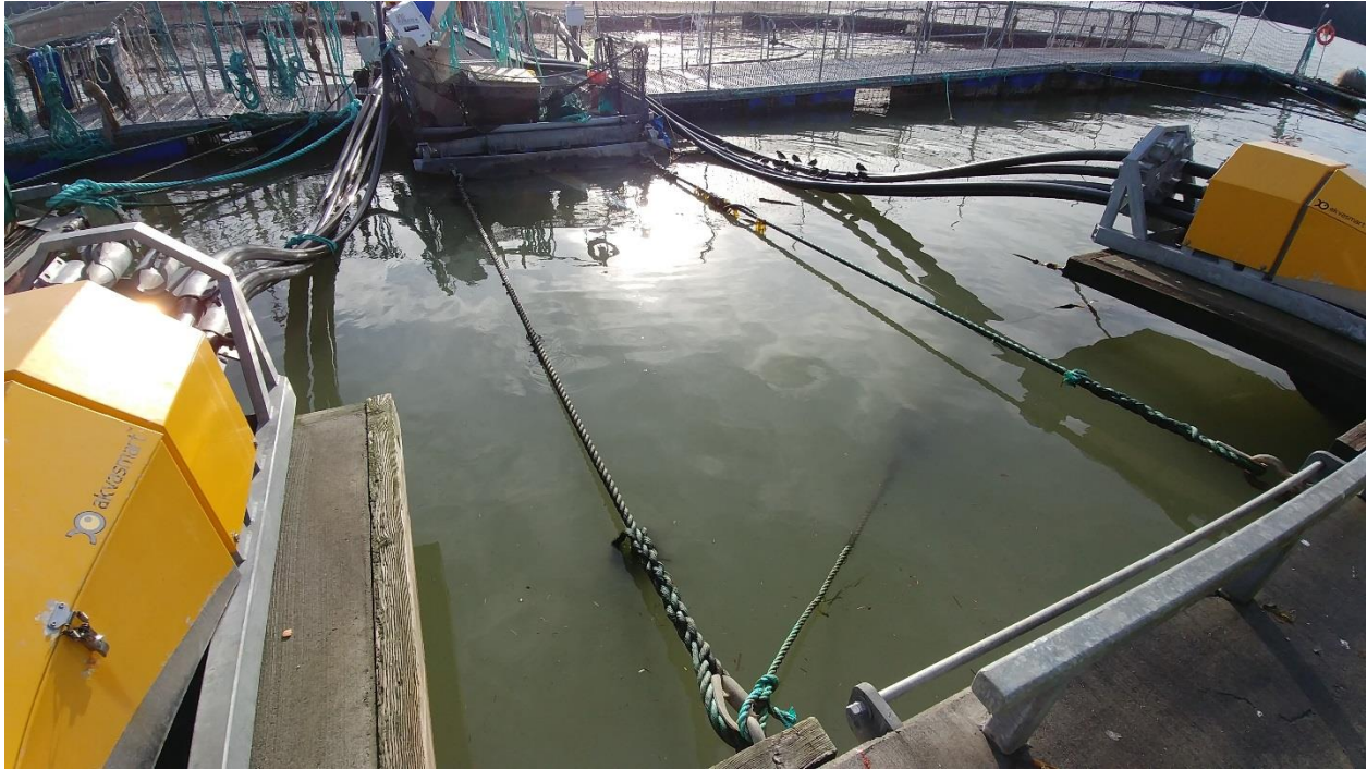
Figure C-90: No Walkway Connection Between Feed Barge and Net Pens.
