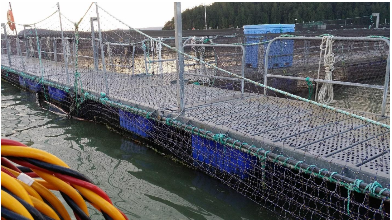
Figure C-9: Hope Island Net Pens - NW Corner of Pens, Looking North
