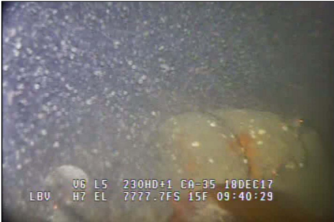
Photograph 42: View of the Exposed Anchor Stem at Anchor 3, Looking Southwest. Photo taken from an ROV.
