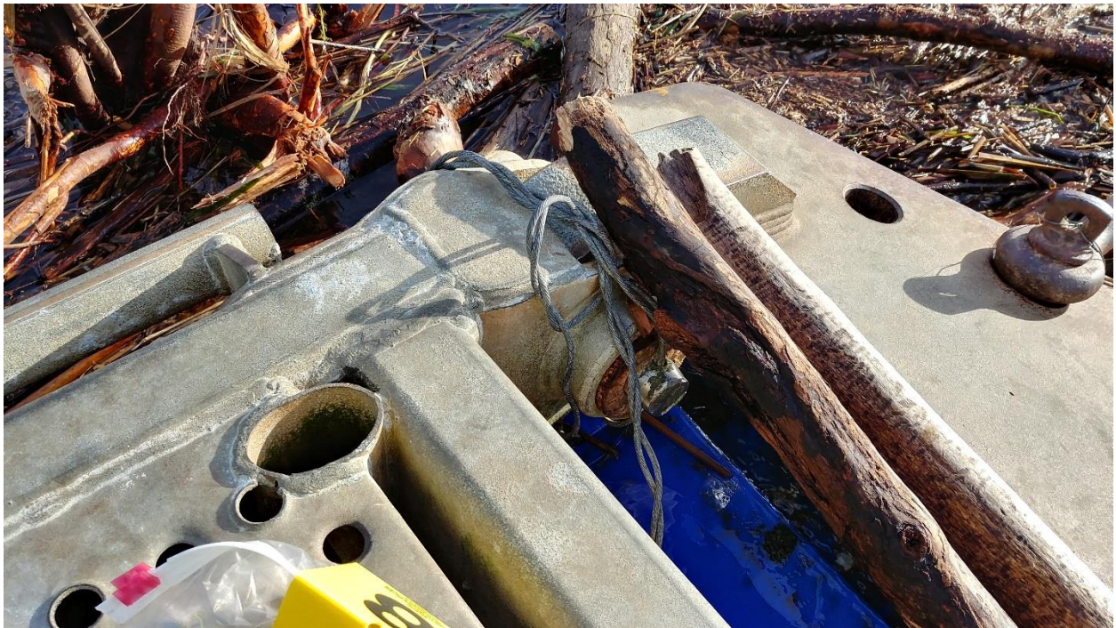
Figure C-35: Anchor #8, SW Corner of the Net Pens
