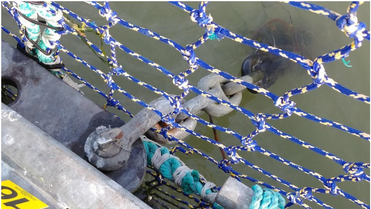
Figure C-51: Anchor #16, East Side of the Net Pens
