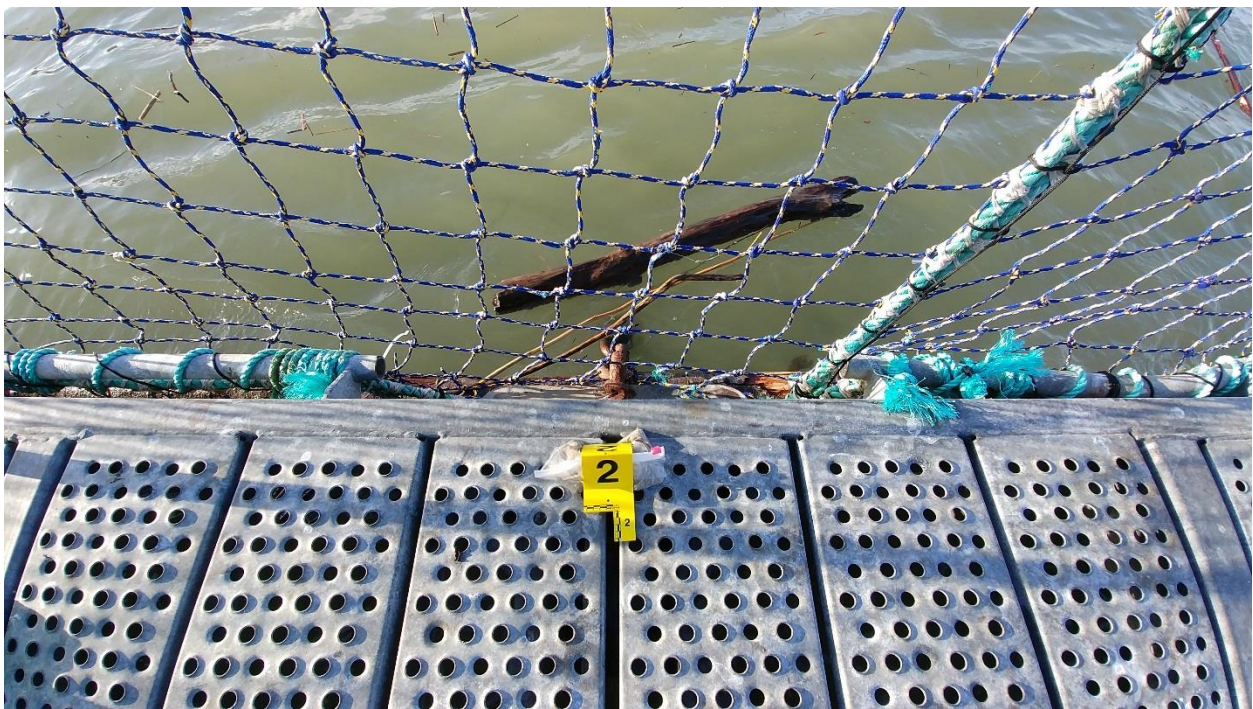
Figure C-23: Anchor #2, West Side of the Net Pens
