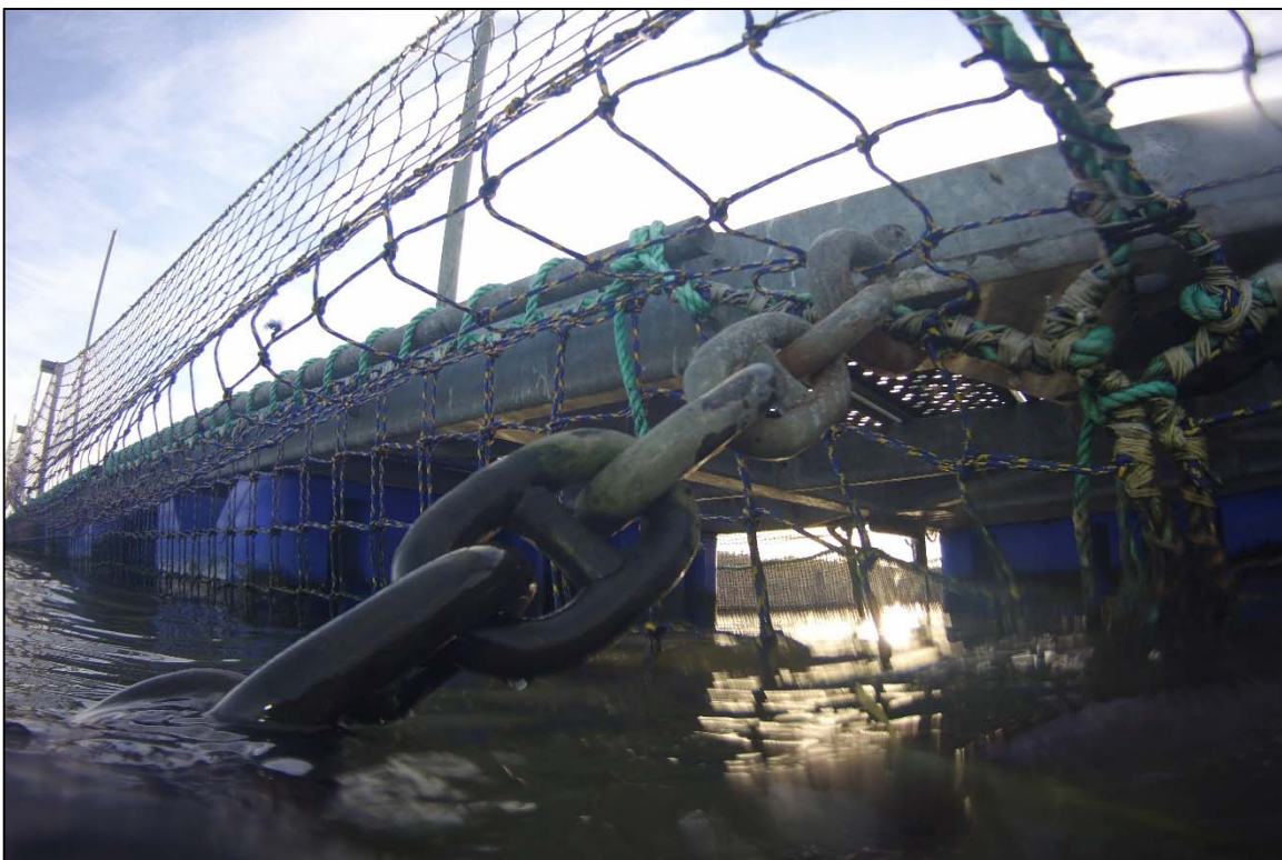
Photograph 24: View of Upper Anchor Chain at Anchor 16 (Typical), Looking Southwest.
