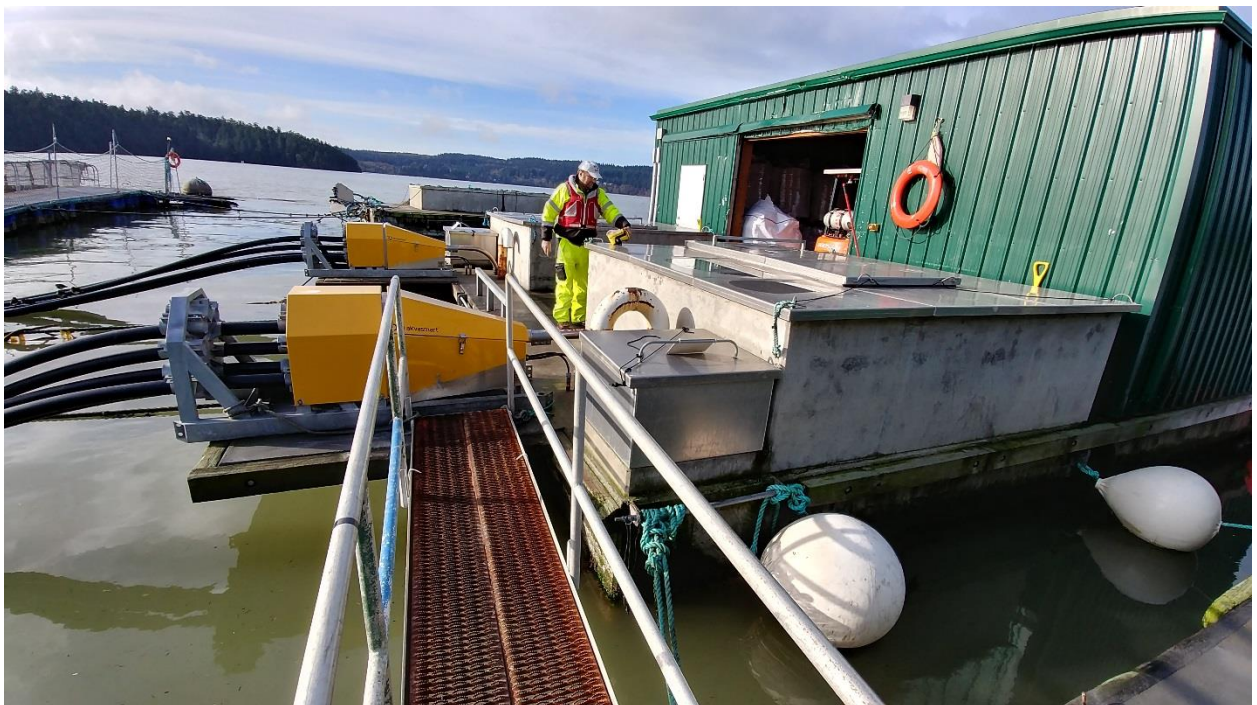
Figure C-87: View Looking NW at the Feed Barge
