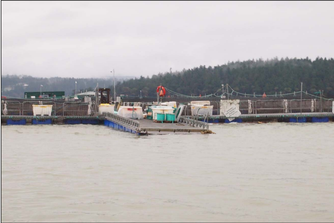
Photograph 17: View of the Depressed Pen Support Float (During High Ebb Tidal Flow) at the Center of the South End, Looking Northeast.
