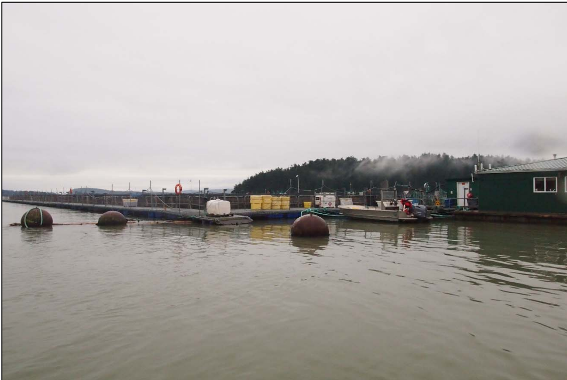
Photograph 4: Overall View of the Fish Net Pen System, Looking Southwest.
