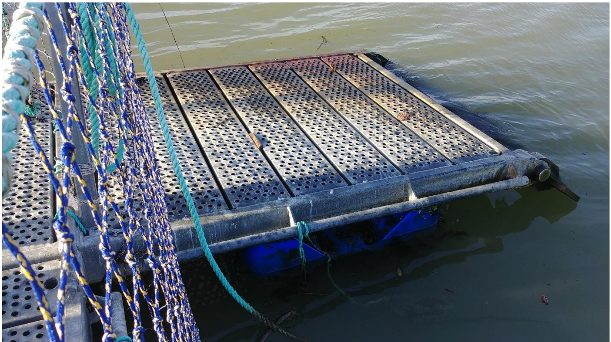
Figure C-11: Hope Island Net Pens - NW Corner, Sinking Platform
