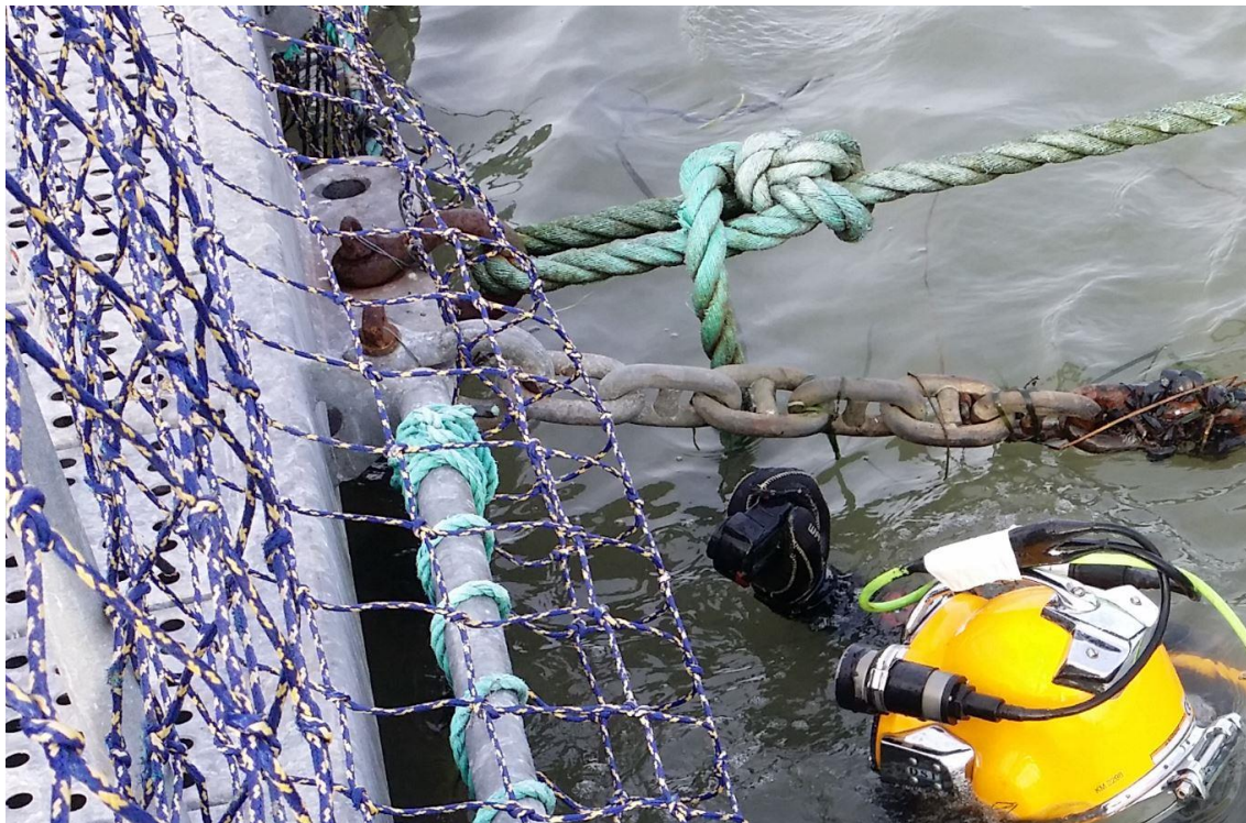
Figure 8: Mooring Bracket at Hope Island Net Pens
