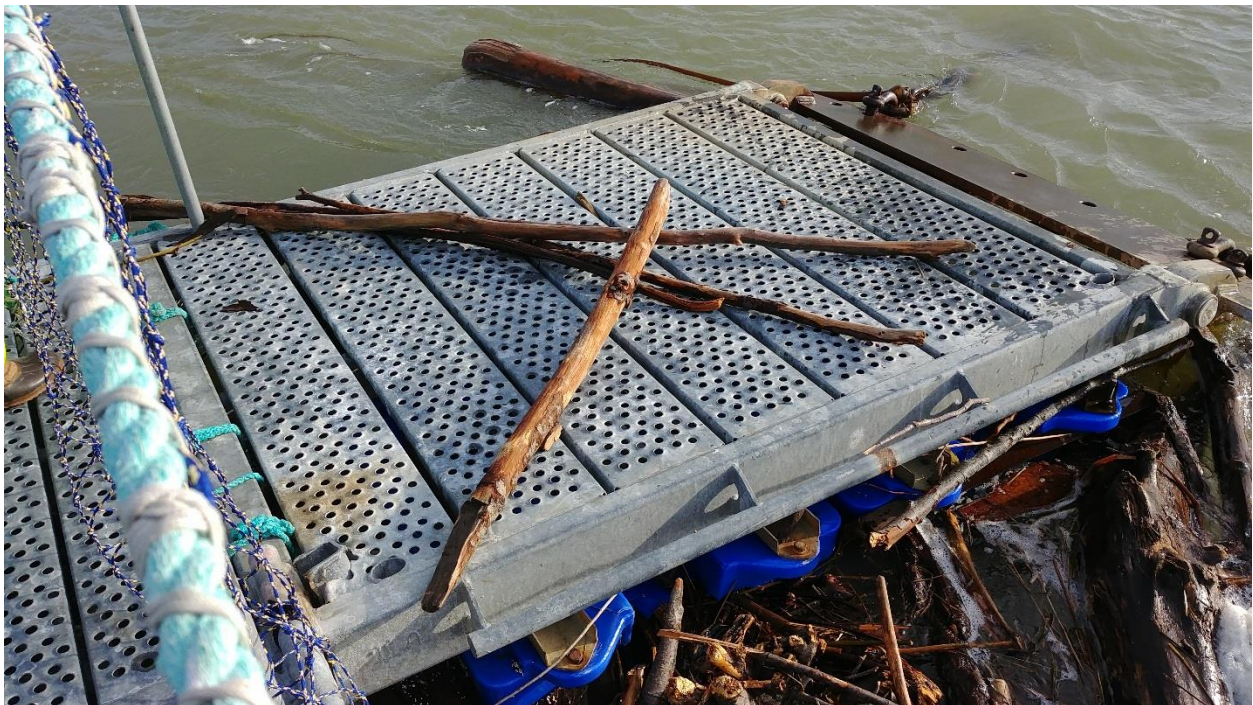
Figure C-13: Hope Island Net Pens - SE Corner, Sinking Platform
