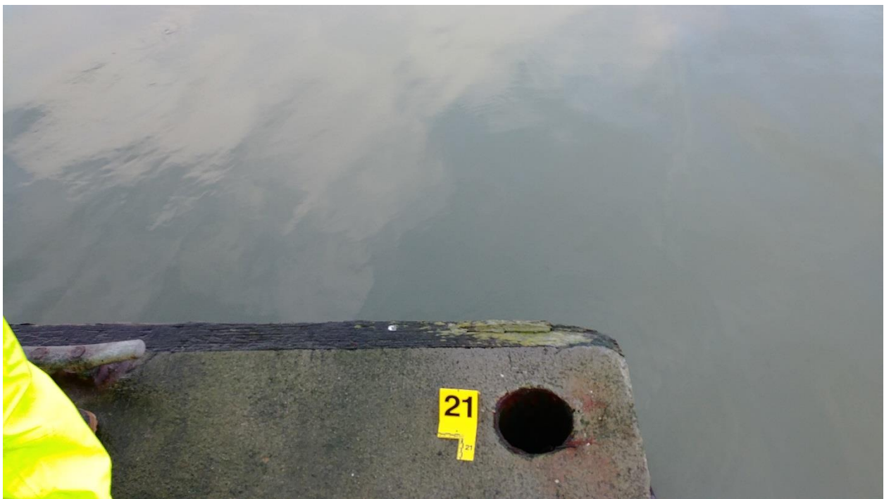
Figure C-61: Anchor #21, NE Corner of the Main Barge. Connection Point Shared with Anchor #21..
