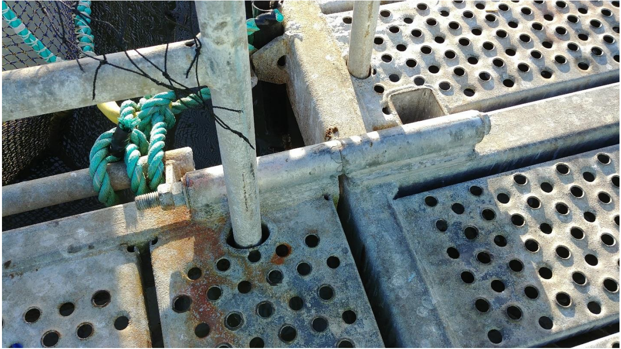
Figure C-94: Barrel Hinge Connection Between Main Walkways and
