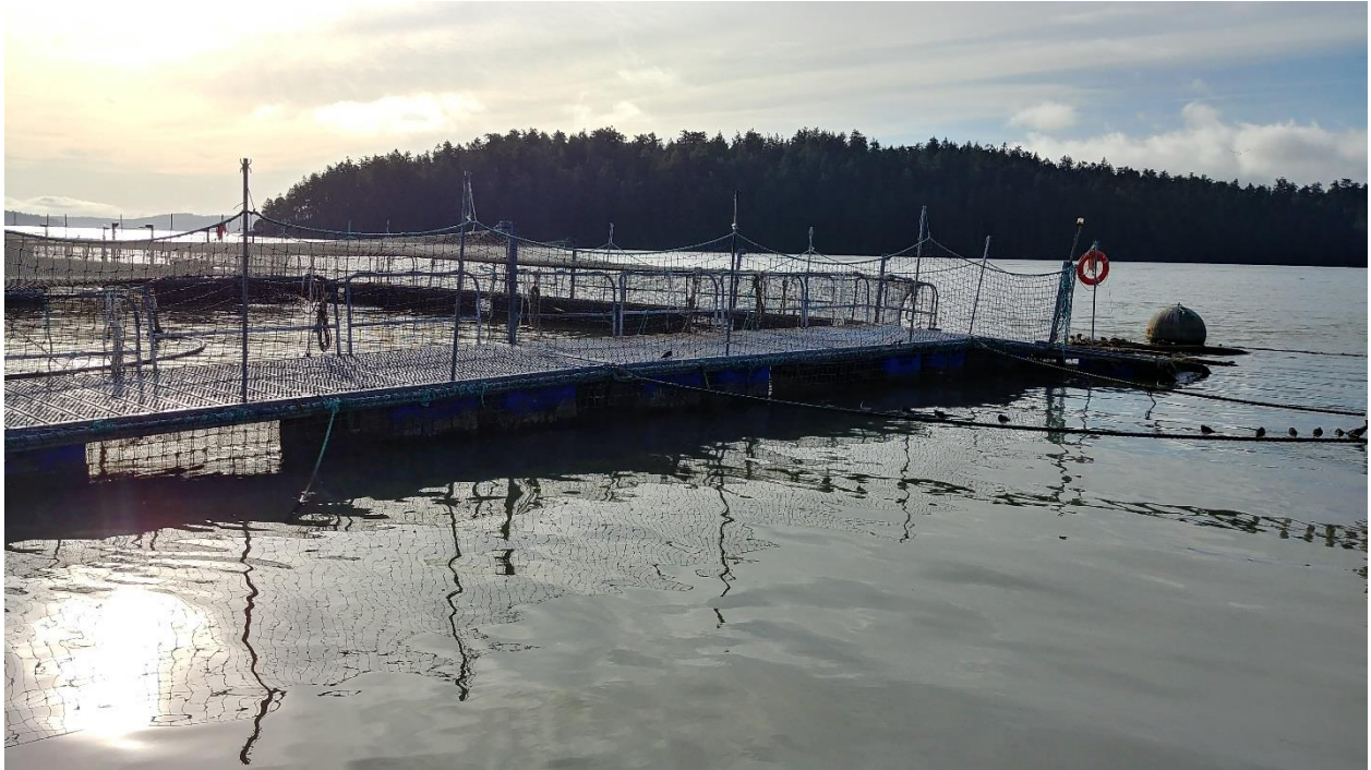
Figure C-8: Hope Island Net Pens - NW Corner of Pens, Looking North
