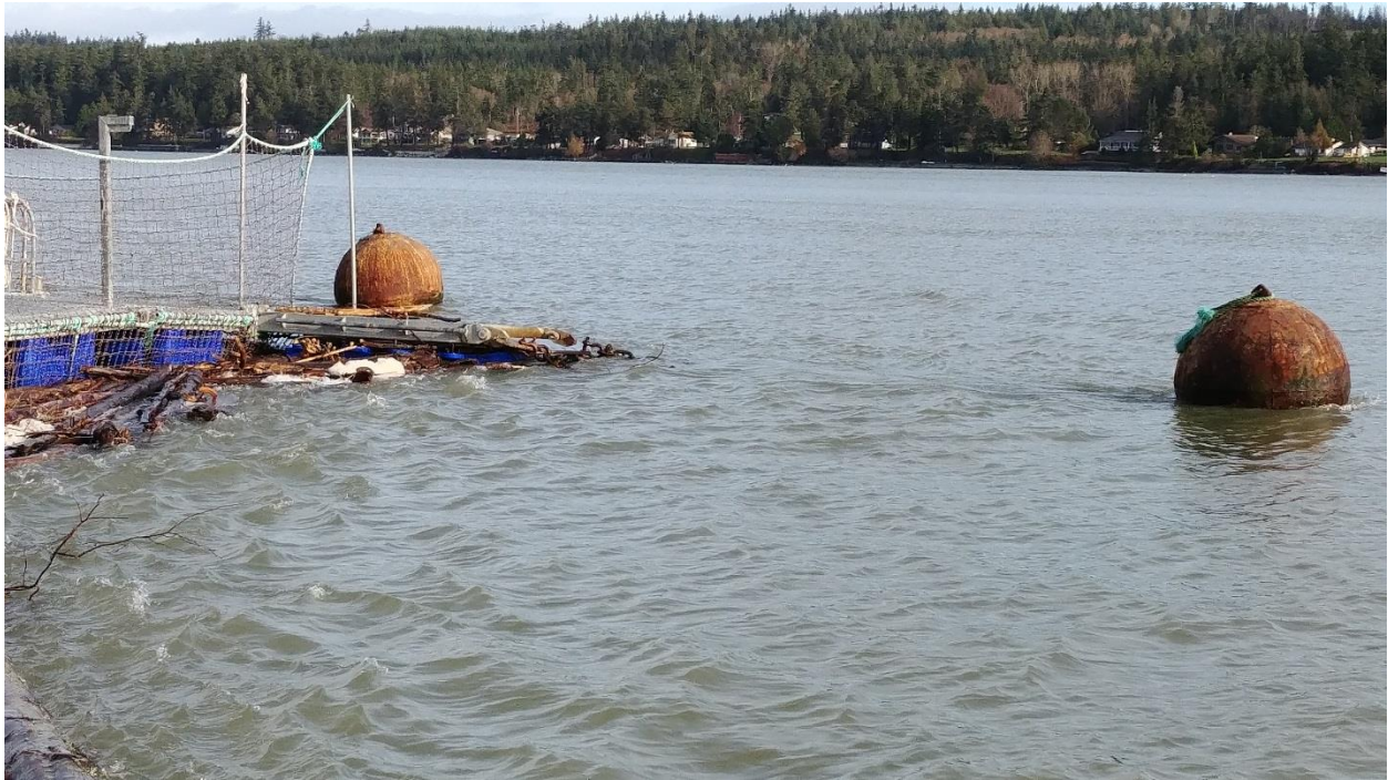
Figure C-16: Current from the South Traps Debris Against the Net Pen
