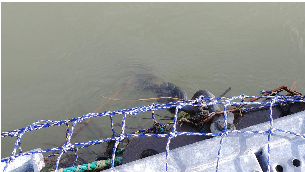
Figure C-45: Anchor #13, East Side of the Net Pens
