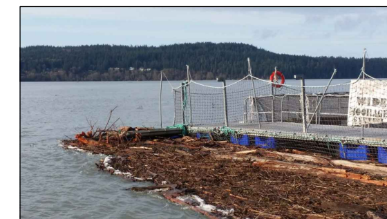
PHOTO 5 DEBRIS BUILDUP ON SOUTH END OF FACILITY
