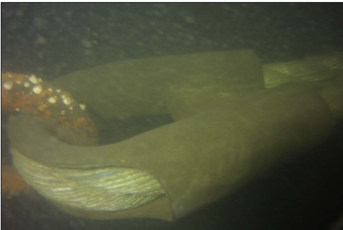
Photograph 28: View of Upper Thimble at Anchor 18 (Typical), Looking North.
