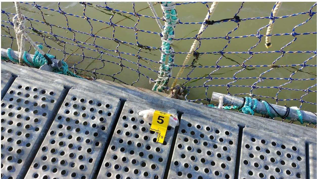
Figure C-29: Anchor #5, West Side of the Net Pens
