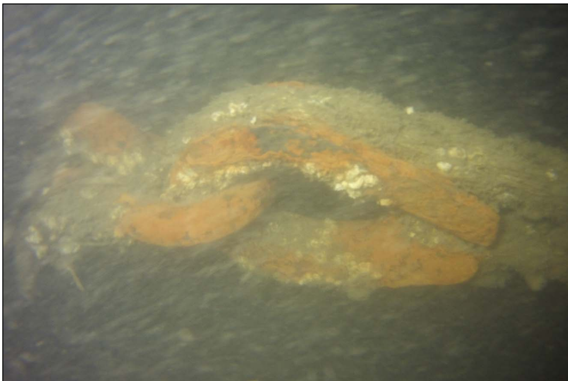
Photograph 32: View of Lower Anchor Chain to Rope Connection (Thimble and Shackle) at Anchor 21 (Typical), Looking East.
