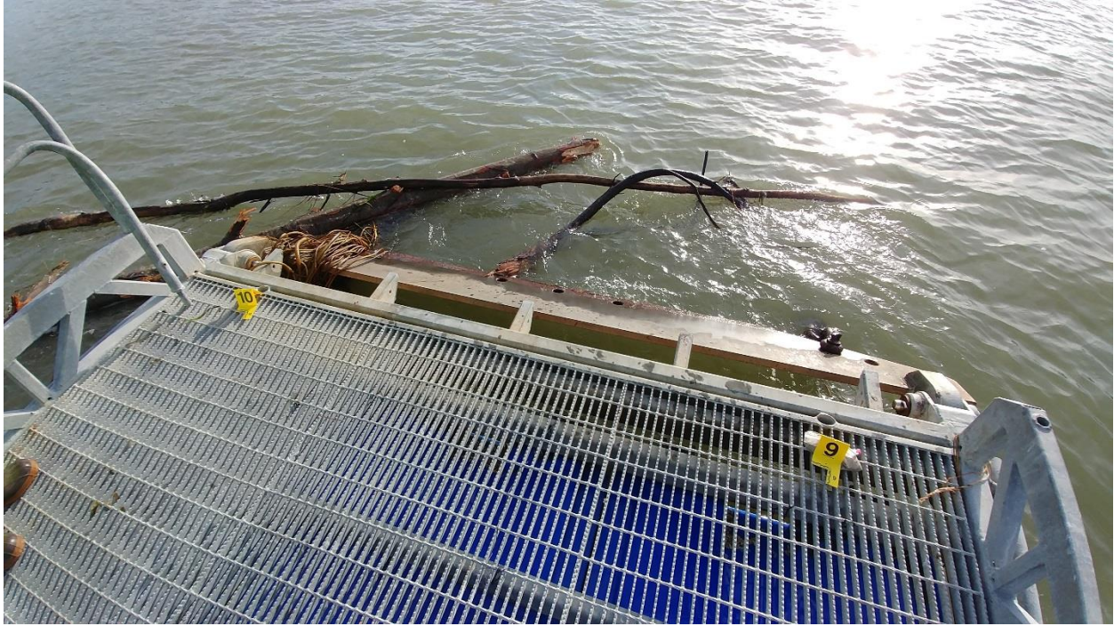
Figure C-38: Anchors #9 and #10, South Side of the Net Pens
