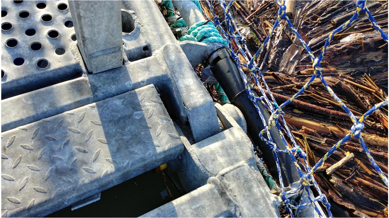
Figure C-96: Hinge between Segments of Main Walkways with UHMW Covering Side Pipe
