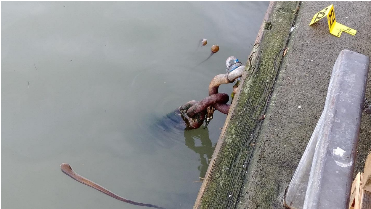
Figure C-65: Anchor #22, North Side of the Feed Barge, East of Centerline.
