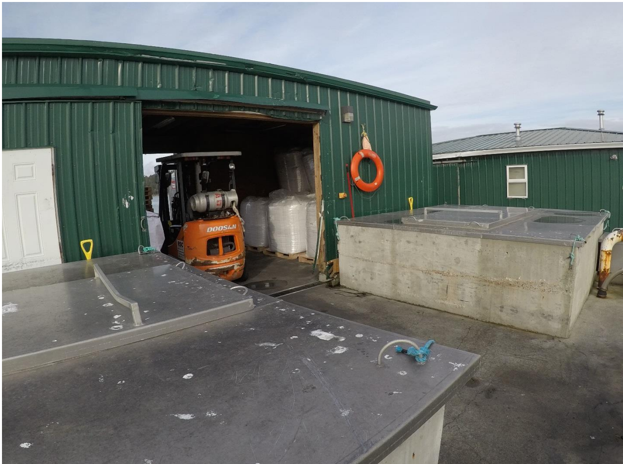
Figure C-89: Feed Barge, Containing Feed Silos and Storage. Forklift does not leave Feed Barge.
