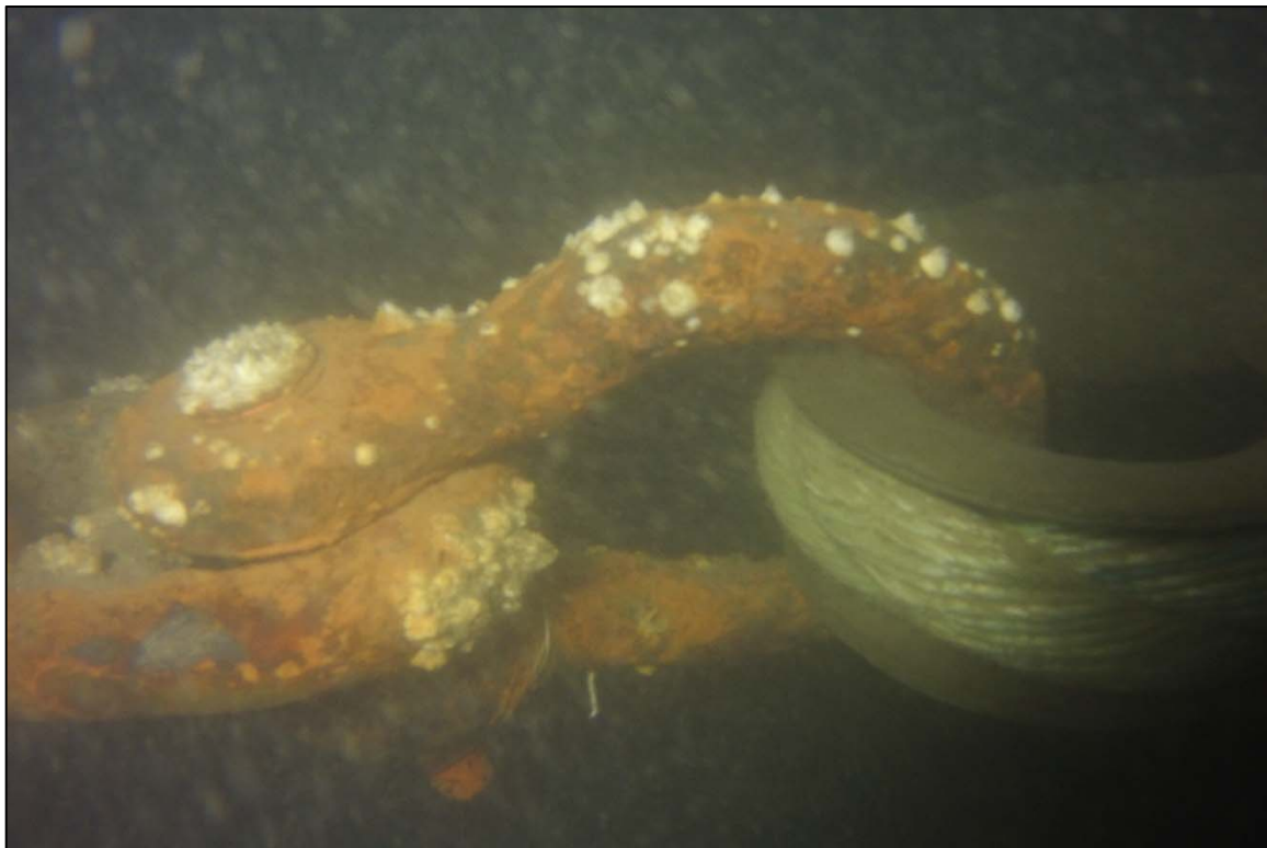
Photograph 26: View of Upper Anchor Chain to Rope Connection (Thimble and Shackle) at Anchor 18 (Typical), Looking North.
