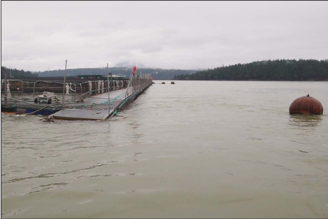
Photograph 15: View of the Depressed Pen Support Float (During High Ebb Tidal Flow) at the Southeast Corner, Looking North.
