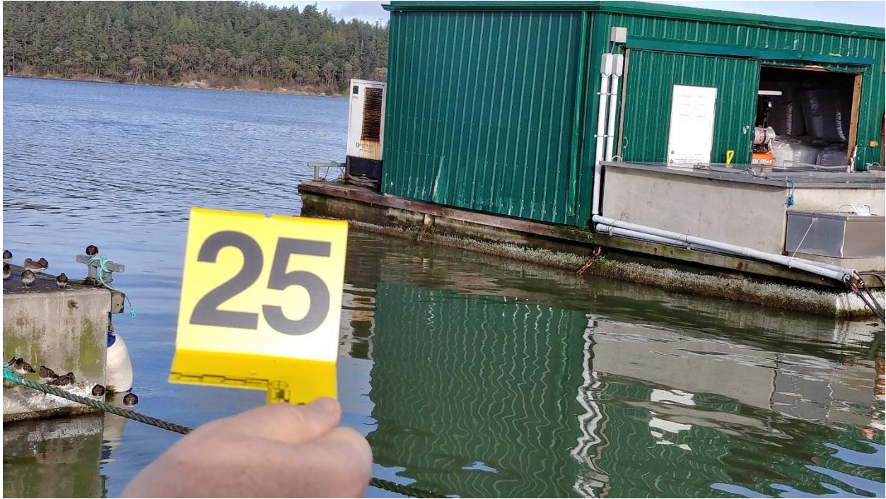
Figure C-68: Anchor #25, West Side of Feed Barge. Anchor Bridle System.
