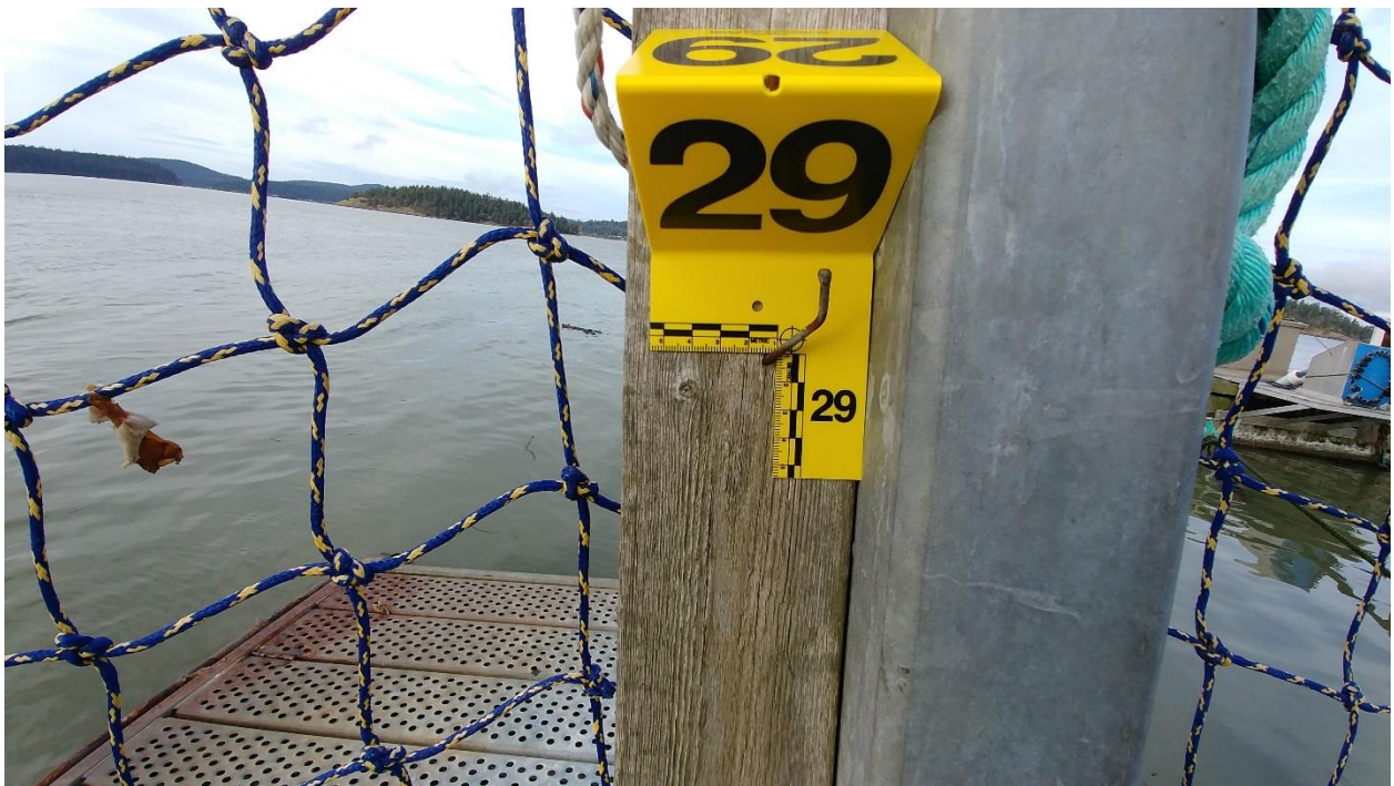
Figure C-73: Exposed Nail
