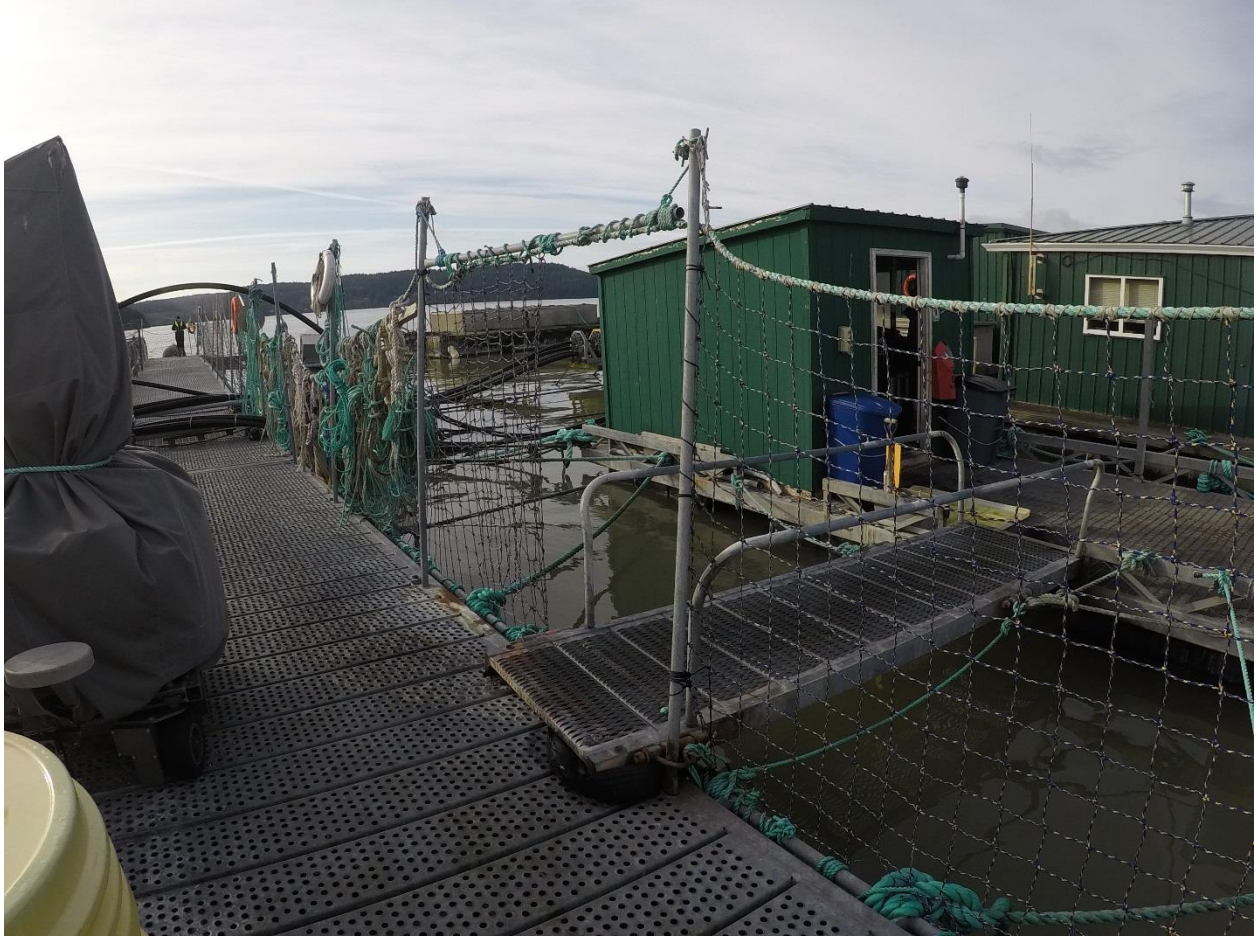
Figure C-84: Gangway Connecting Net Pens to Dive Float. Note Low Overhead Clearance.
