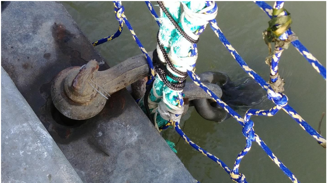
Figure C-49: Anchor #15, East Side of the Net Pens
