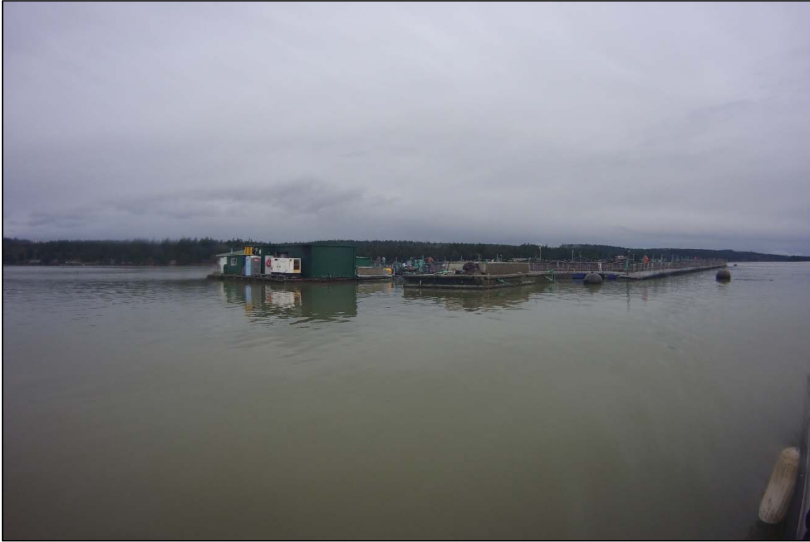
Photograph 3: Overall View of the Fish Net Pen System, Looking Southeast.
