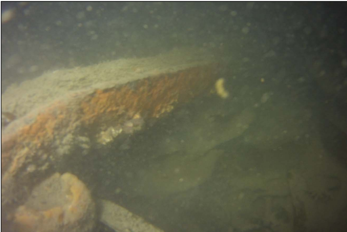
Photograph 38: View of Lower Thimble on Channel Bottom at Anchor 19, Looking Southeast.
