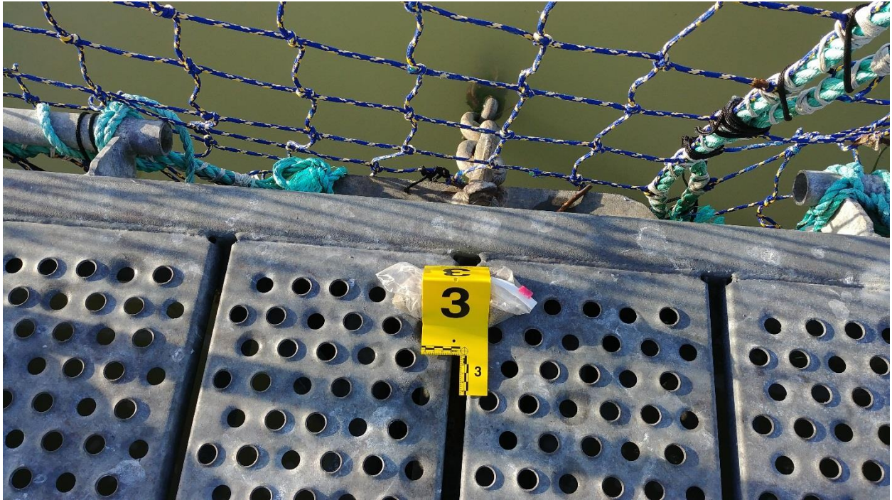
Figure C-24: Anchor #3, West Side of the Net Pens
