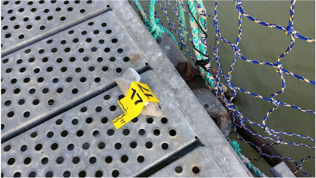
Figure C-52: Anchor #17, East Side of the Net Pens
