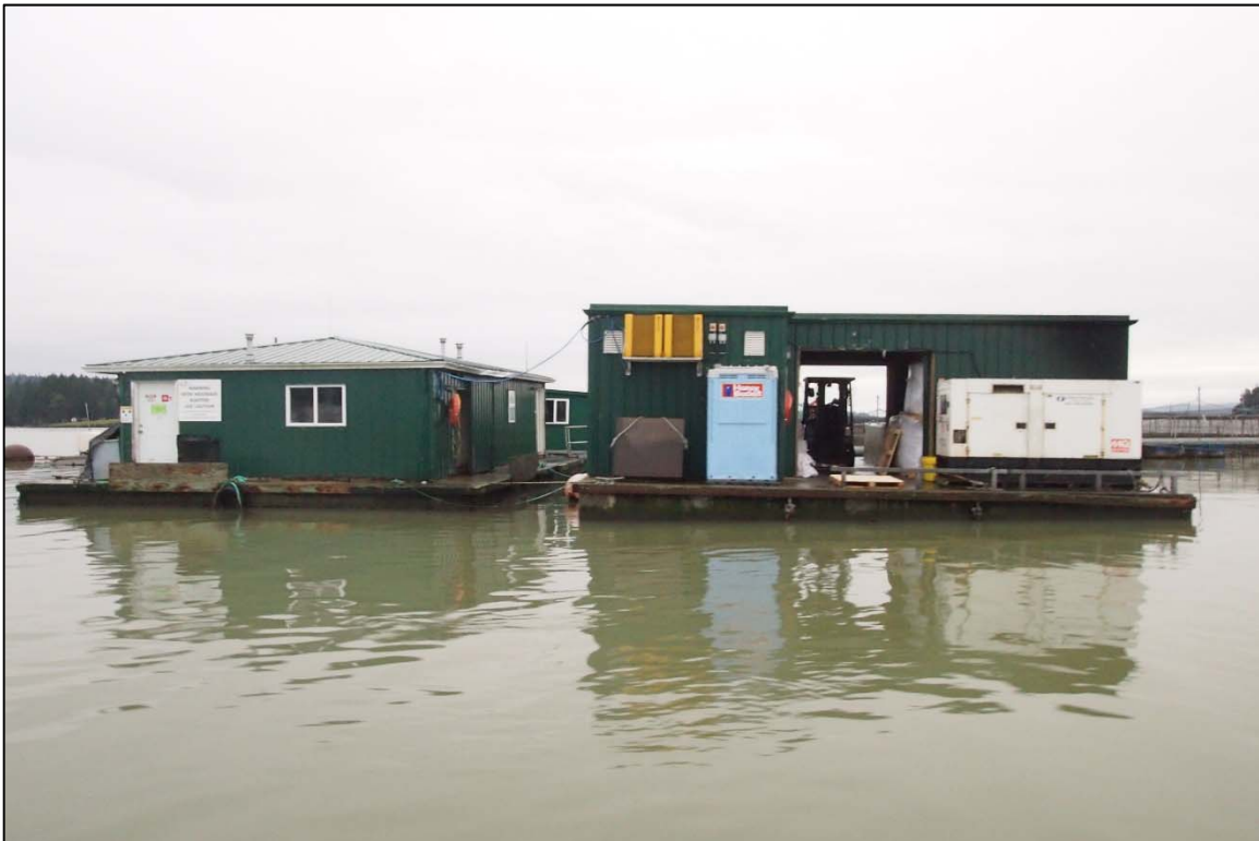
Photograph 20: View of the Storage Buildings Located on the North End, Looking South.
