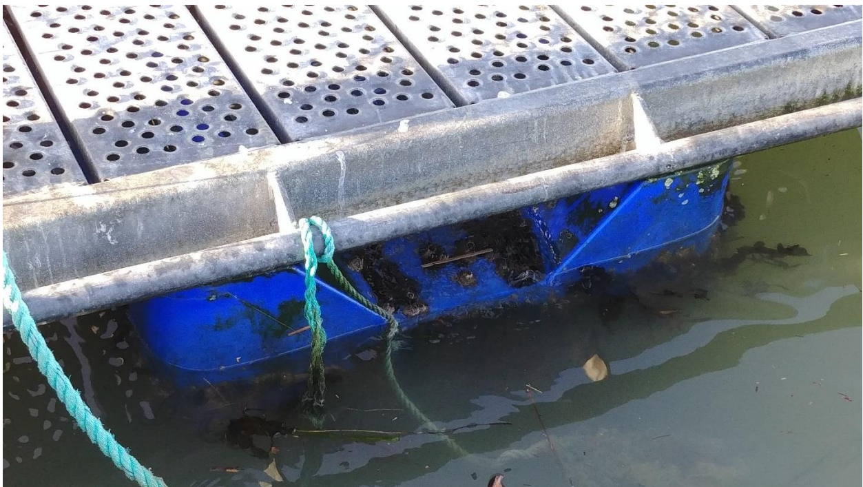
Figure C-101: Float Tub Example – Plastic Tub with Foam Inside
