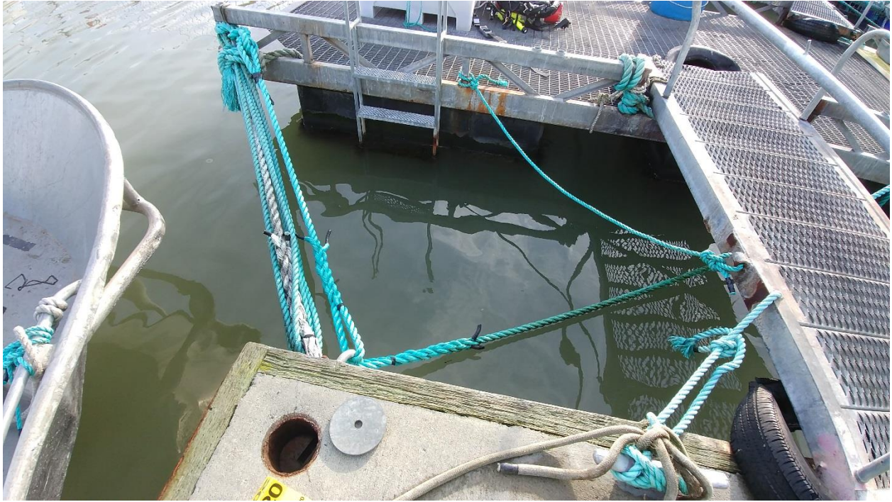
Figure C-58: Anchor #20, SE Corner of the Main Barge. Part of an Anchor Bridle System.
