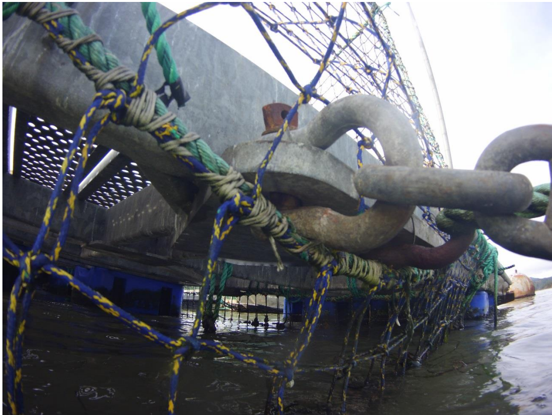
Figure 10: Typical Mooring Bracket at Hope Island
