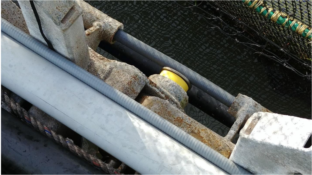
Figure C-100: Walkway Hinge Bushing, Containment Net Railing Being Used as a Conduit
