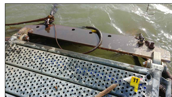
PHOTO 7 HINGED MOORING BRACKET AND ANCHOR CHAINS
