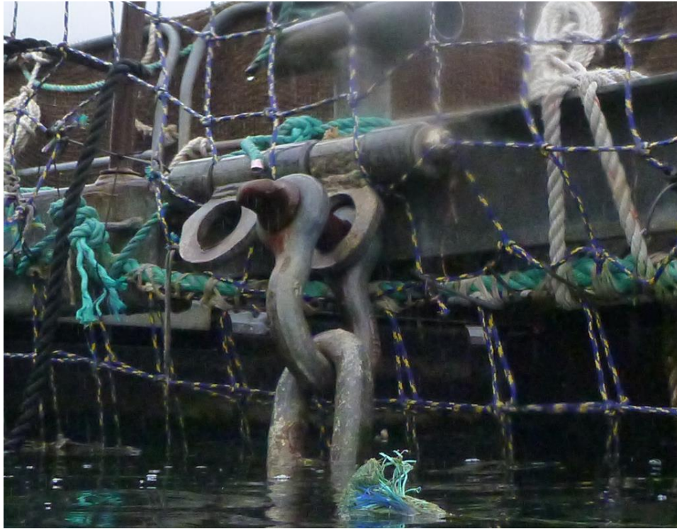
Figure 6: Cypress Island Site 1 - Mooring Bracket at Line 20
