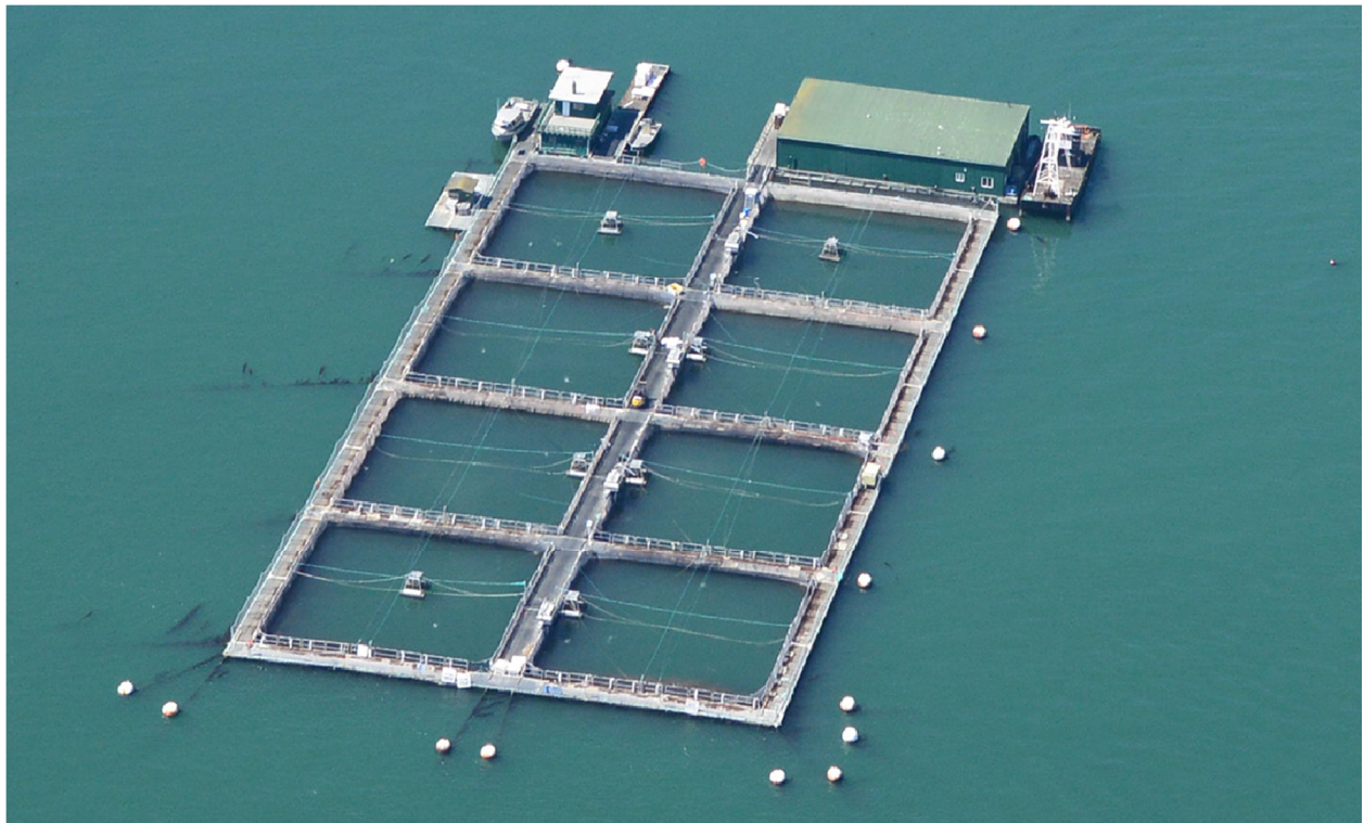
Figure C-1: Cypress Island Net Pen Site 1 – Oblique Aerial from NorthEast
