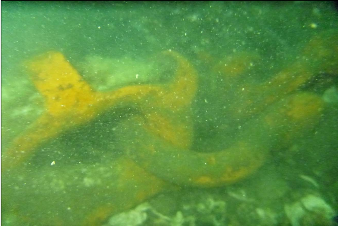
Photograph 73: View of the Rope to Lower Anchor Chain Connection (Thimble and Shackle) at Site 1 Anchor Line 21, Looking East.
