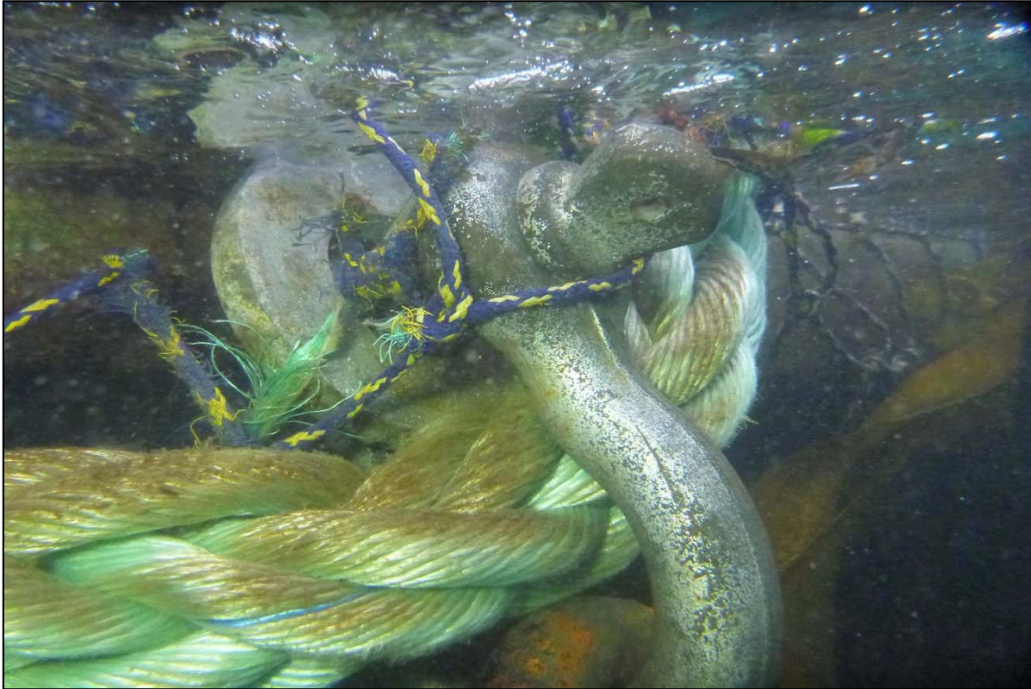
Photograph 49: View of the Float to Upper Anchor Chain Connection at Site 1 Anchor Chain 13, Looking Northwest.
