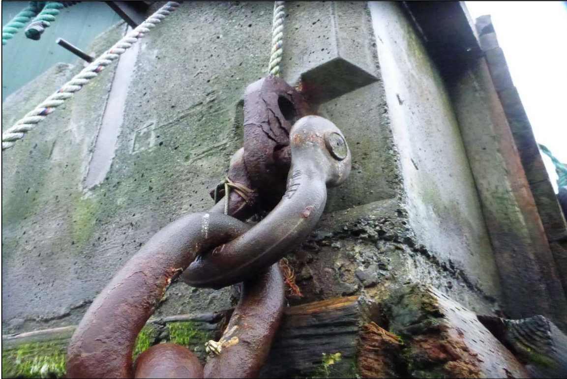
Photograph 19: View of the Feed Barge to Upper Anchor Chain Connection at Site 1 Anchor Line 3, Looking East.
