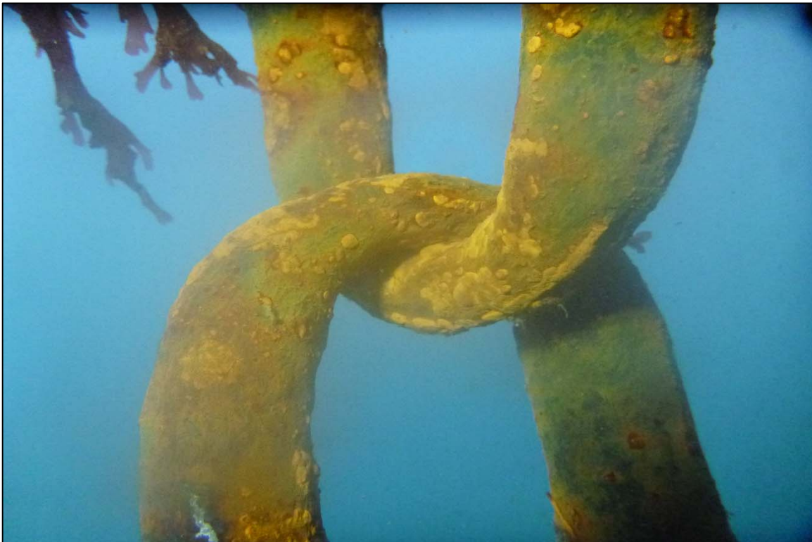
Photograph 38: View of the Severe Corrosion and up to 75% Section Loss on the Buoy Chain at Site 1 Anchor Line 9, Looking East.
