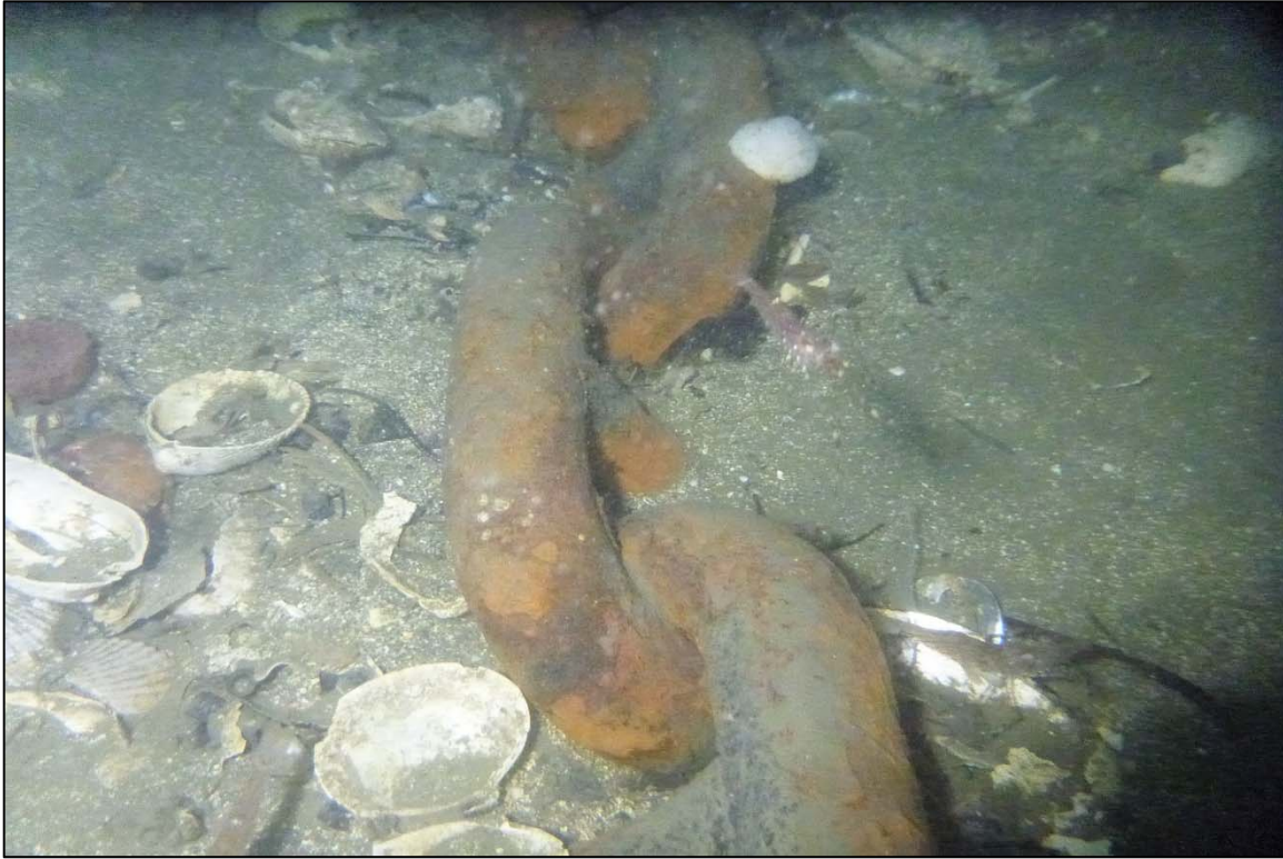
Photograph 33: View of the Lower Anchor Chain Embedment in the Channel Bottom at Site 1 Anchor Chain 7, Looking North.
