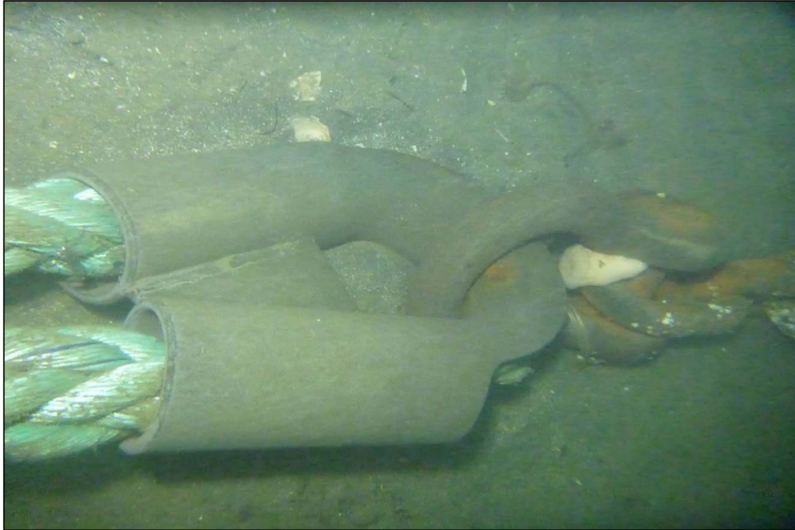
Photograph 81: View of the Rope to Lower Anchor Chain Connection (Thimble and Shackle) at Site 1 Anchor Line 24, Looking West.
