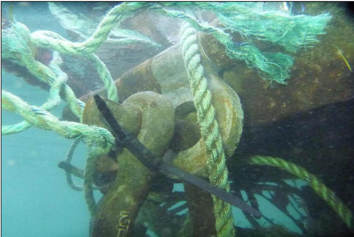
Photograph 78: View of the Float to Upper Anchor Chain Connection at Site 1 Anchor Line 23, Looking Southeast.
