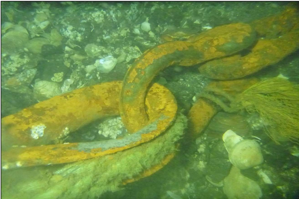
Photograph 62: View of the Rope to Lower Anchor Chain Connection (Thimble and Shackle) at Site 1 Anchor Line 18, Looking Northeast.
