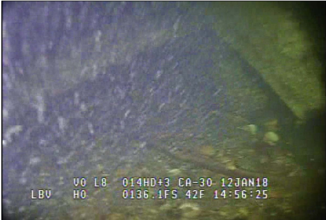
Photograph 51: View of the Exposed Anchor Resting on the Channel Bottom at Site 1 Anchor Line 13, Looking North.
