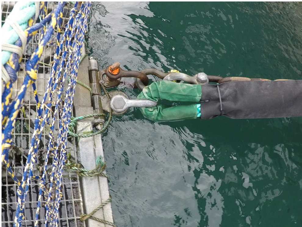
Figure C-8: Cypress Island Net Pen Site 1 – Connection between Concrete Barge and Net Pen
