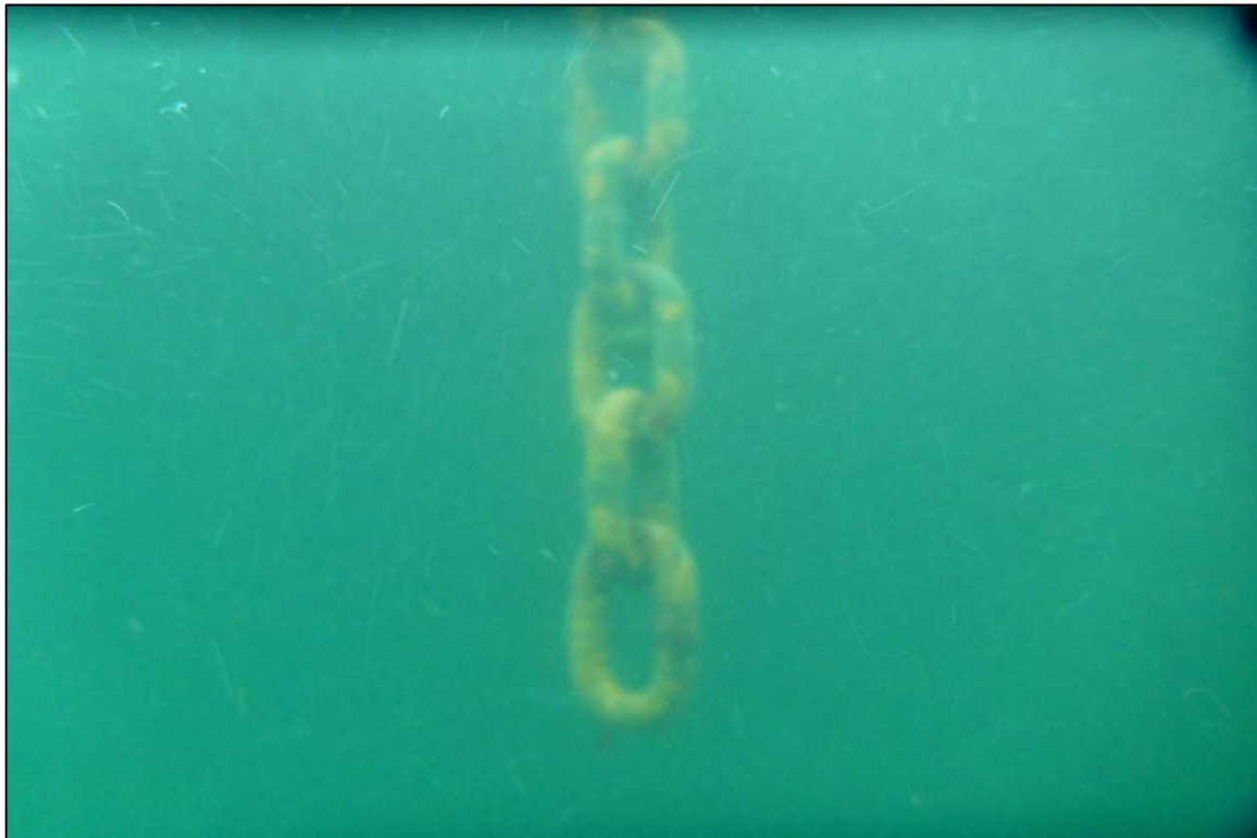
Photograph 12: View of the Termination of the Upper Anchor Chain at Site 1 Feed Barge South Anchor Line, Looking North.
