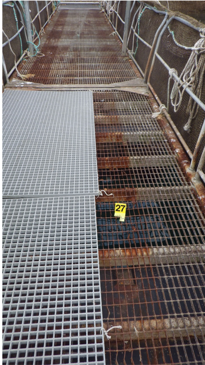
Figure C-25: Cypress Island Net Pen Site 1 – Fiberglass grating overlaid on walkway
