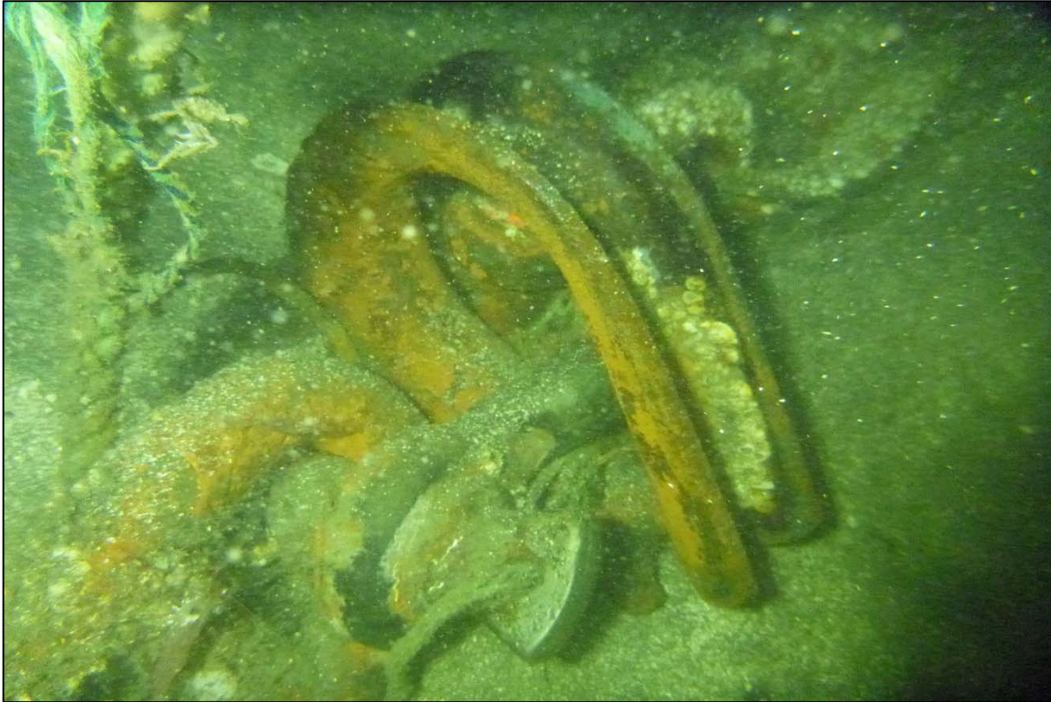
Photograph 45: View of the Loose Thimble at the Rope to Lower Anchor Chain Connection at Site 1 Anchor Chain 11, Looking Northwest.
