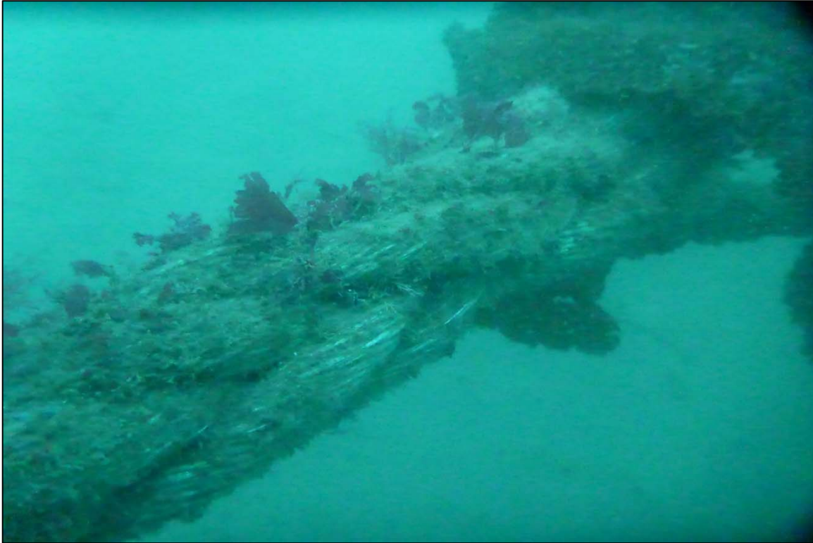
Photograph 29: View of Light Marine Growth on the Rope (Typical) at Site 1 Anchor Line 6, Looking North.
