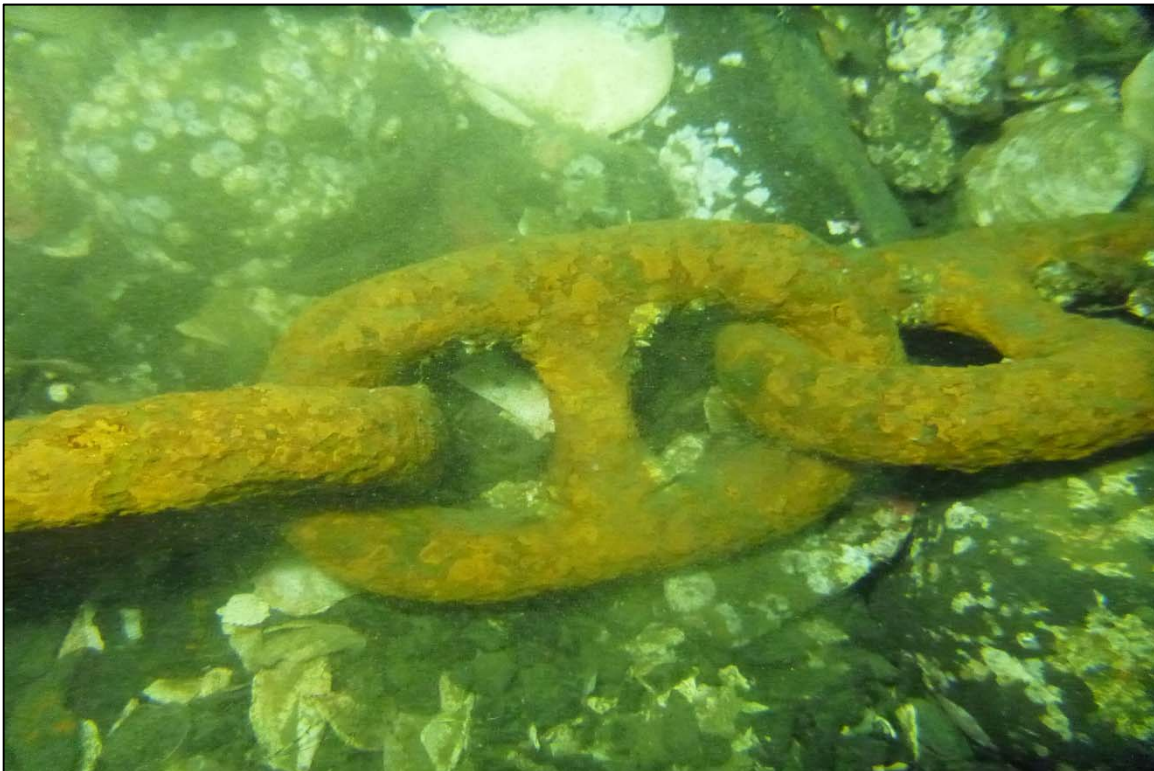
Photograph 74: View of Section Loss in the Lower Anchor Chain at Site 1 Anchor Chain 21, Looking East.
