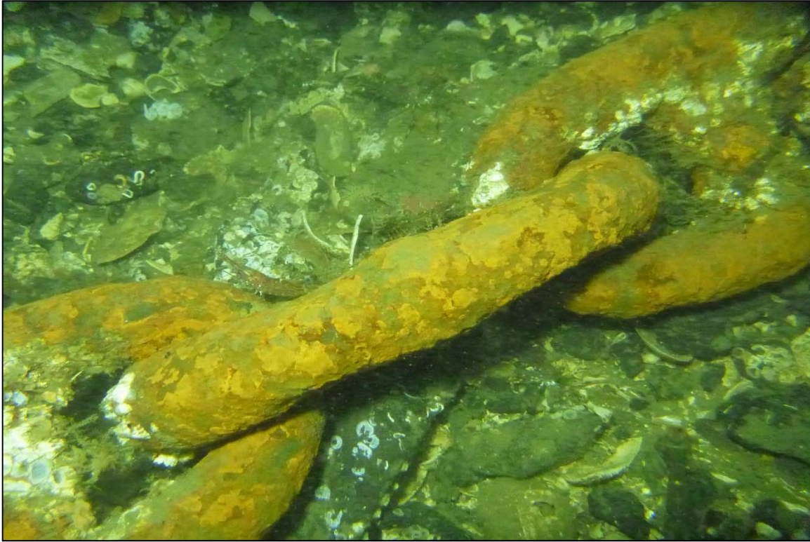
Photograph 63: View of Severe Corrosion on the Lower Anchor Chain at Site 1 Anchor Line 18, Looking Northeast.
