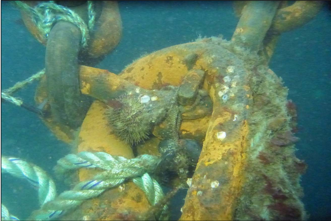
Photograph 65: View of the Upper Anchor Chain to Rope Connection (Thimble and Shackle) at Site 1 Anchor Line 19, Looking North.
