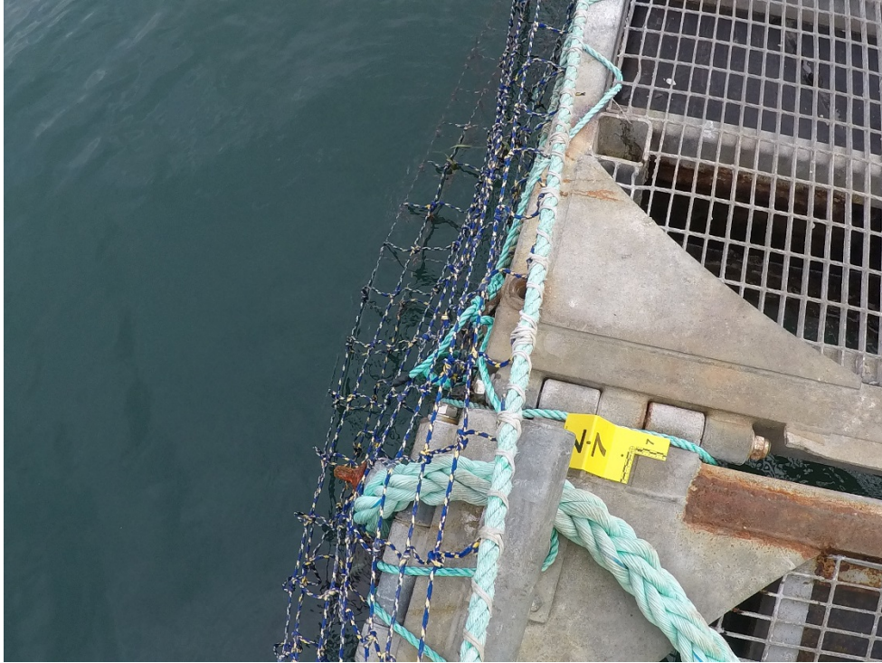
Figure C-9: Cypress Island Net Pen Site 1 – Connection at Anchor Line 7 and typical float-to-float hinge connection
