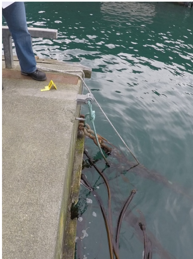
Figure C-6: Cypress Island Net Pen Site 1 – Anchor Line 3 at Concrete Barge
