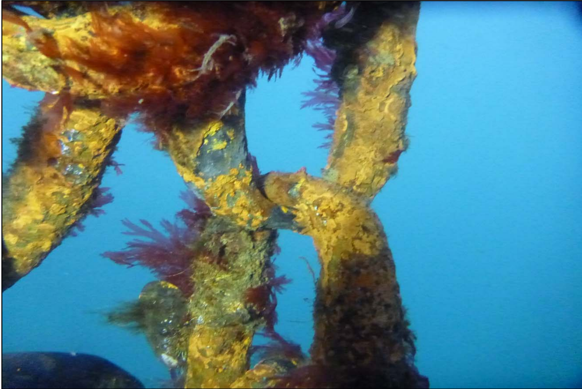
Photograph 57: View of the Severe Corrosion and Section Loss on the Buoy Chain at Site 1 Anchor Line 17, Looking North.
