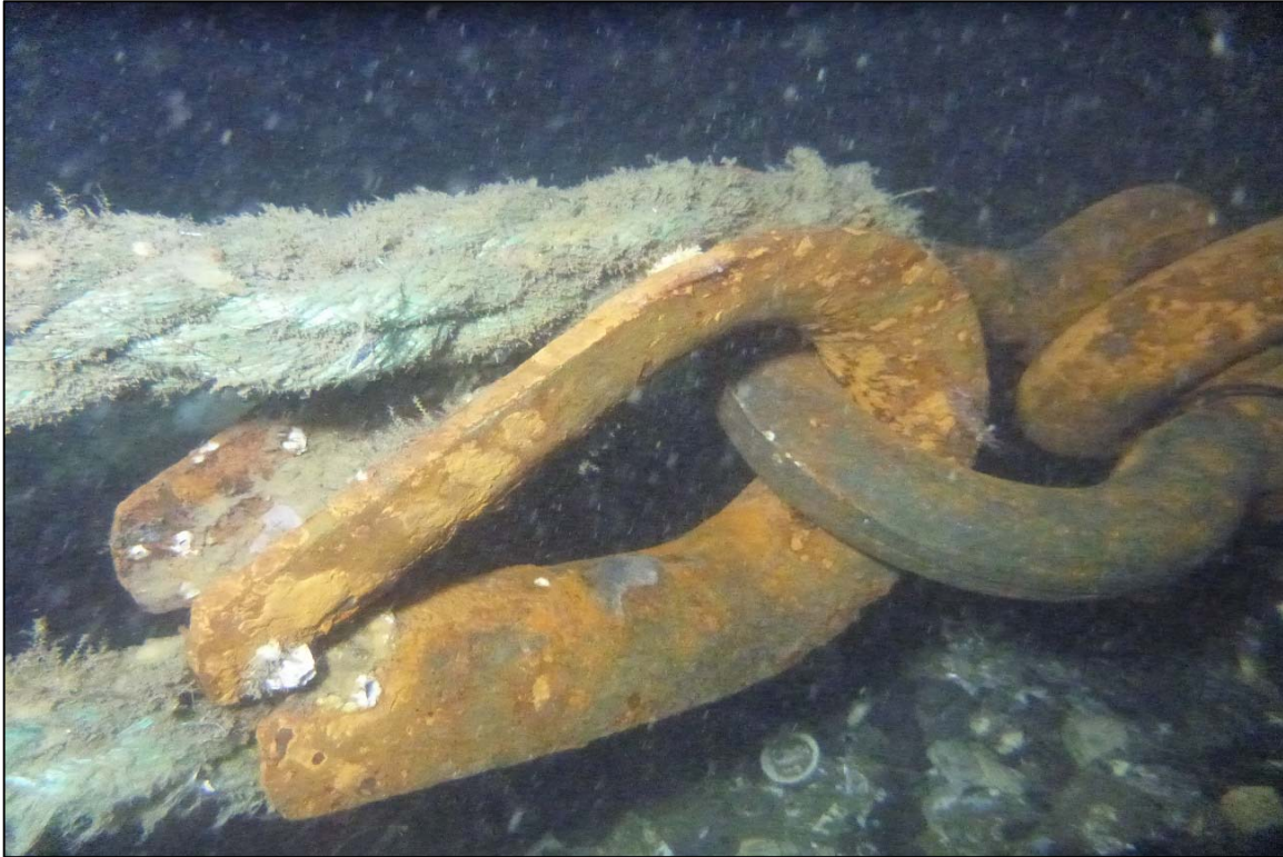
Photograph 59: View of the Rope to Lower Anchor Chain Connection (Thimble and Shackle) at Site 1 Anchor Line 17, Looking Northeast.
