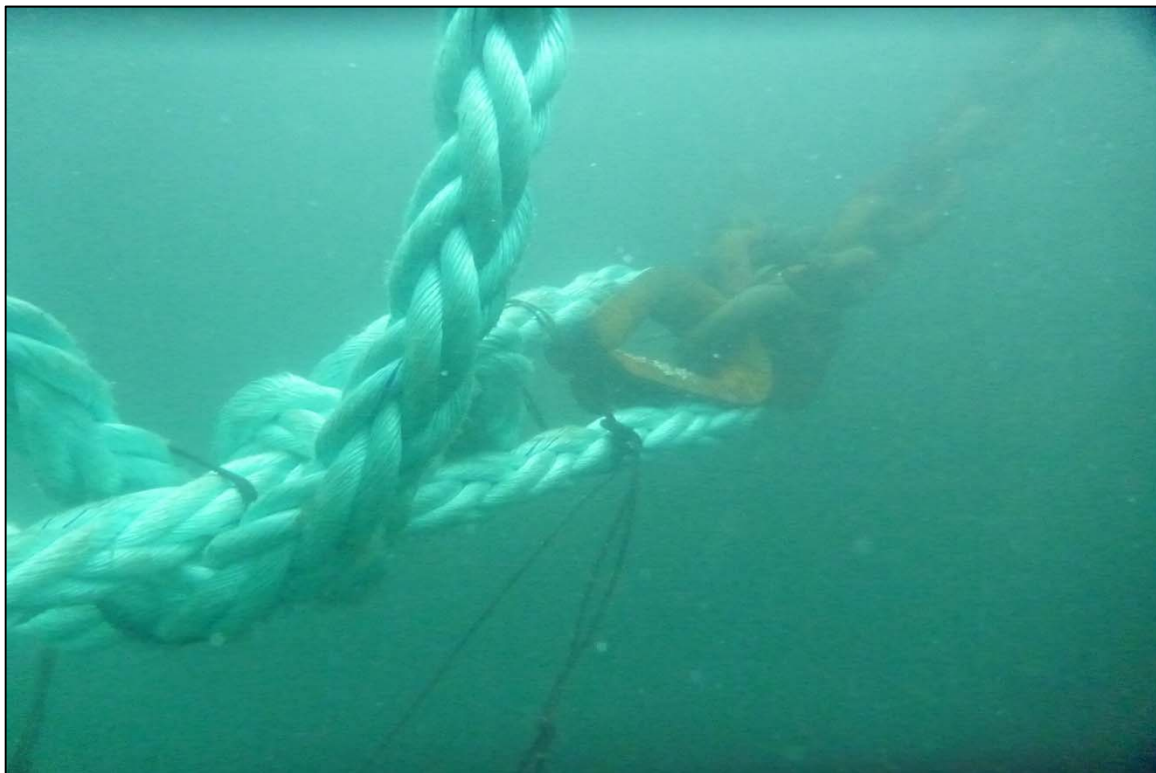
Photograph 68: View of the Upper Anchor Chain to Rope Connection (Thimble and Shackle) with a Bowline Knot at Site 1 Anchor Chain 20, Looking Northwest.
