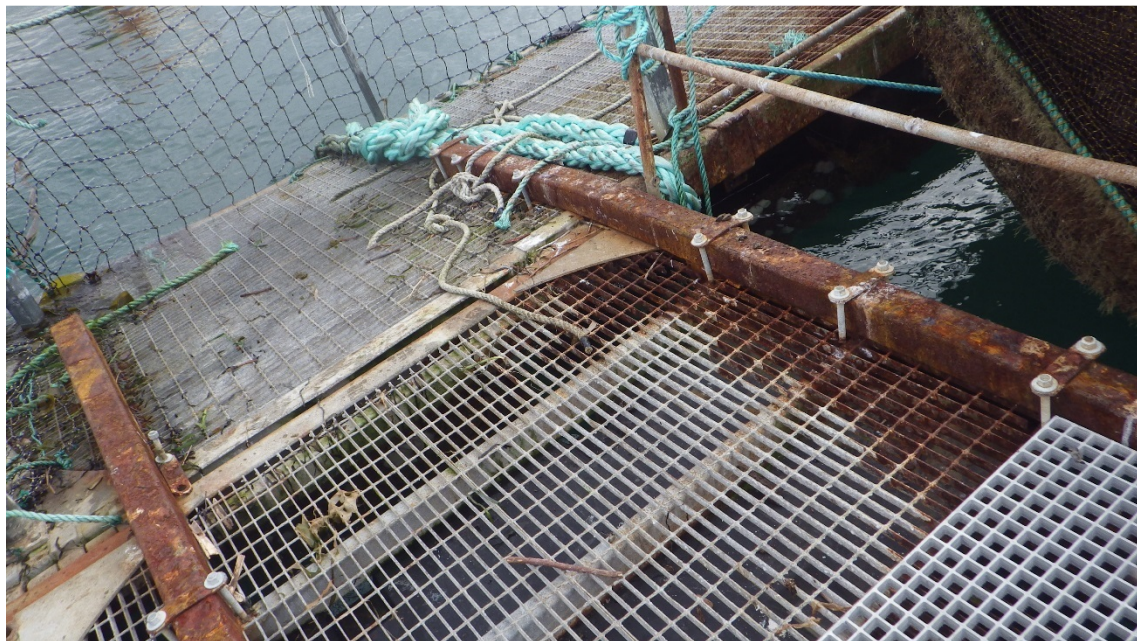
Figure C-21: Cypress Island Net Pen Site 1 – Repair with HSS on northeast corner
