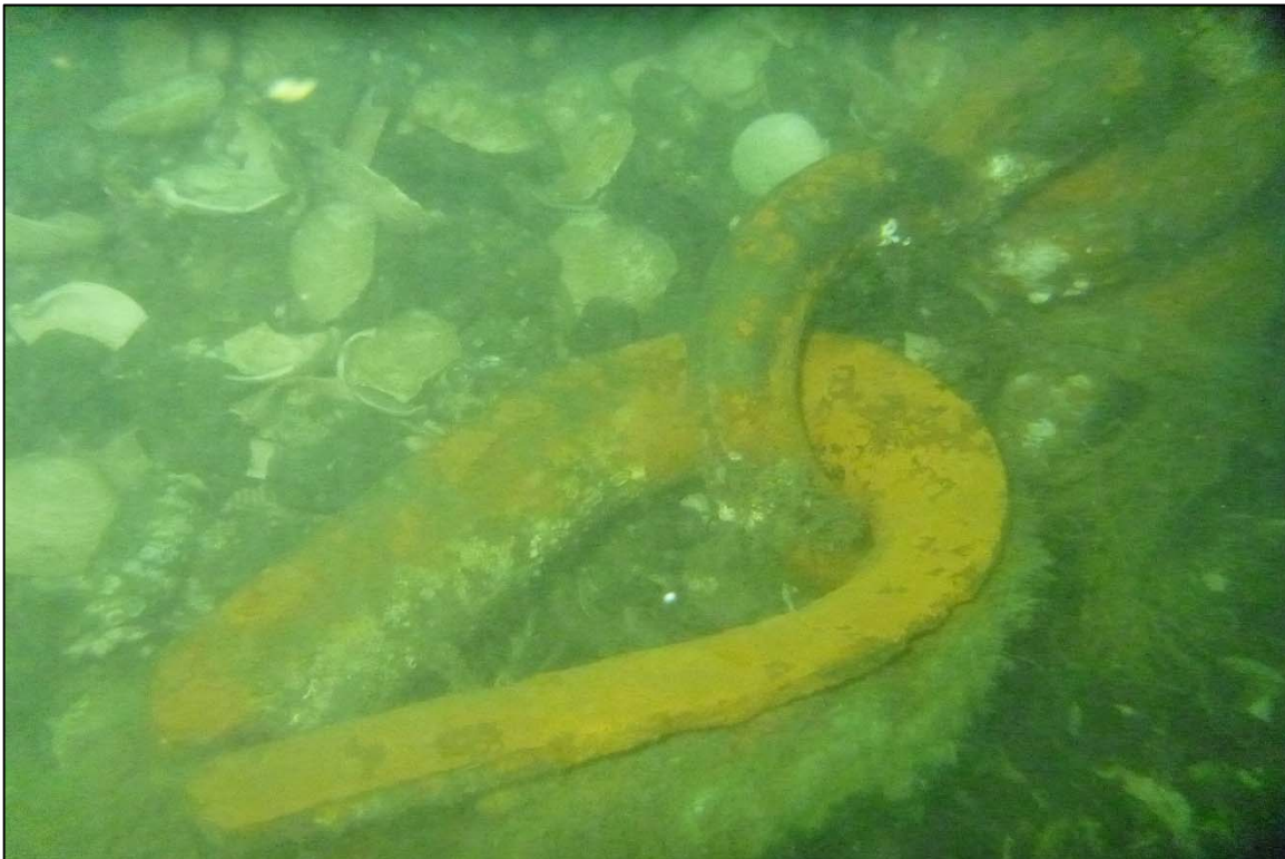
Photograph 76: View of the Rope to Lower Anchor Chain Connection (Thimble and Shackle) at Site 1 Anchor Line 22, Looking East.
