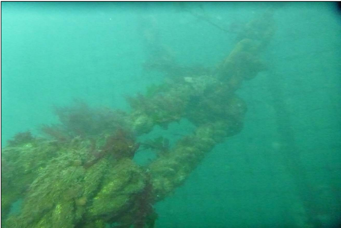
Photograph 72: View of the Upper Anchor Chain to Rope Connection (Shackle) with a Bowline Knot at Site 1 Anchor Chain 21, Looking Northwest.
