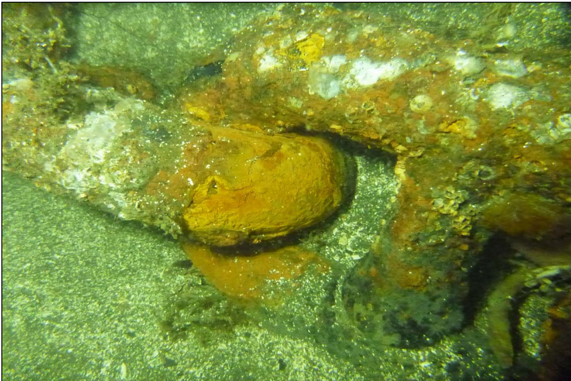
Photograph 46: View of Moderate Corrosion on the Lower Anchor Chain at Site 1 Anchor Line 11, Looking West.
