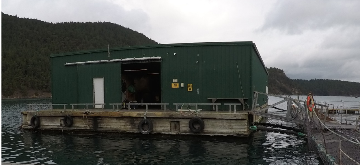
Figure C-3: Cypress Island Net Pen Site 1 – Storage Shed on Concrete Float
