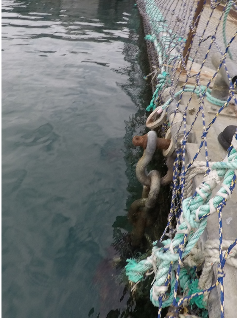
Figure C-17: Cypress Island Net Pen Site 1 – Connection at Anchor Line 20
