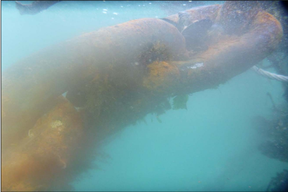
Photograph 55: View of the Upper Anchor Chain at Site 1 Anchor Line 16, Looking Southwest.
