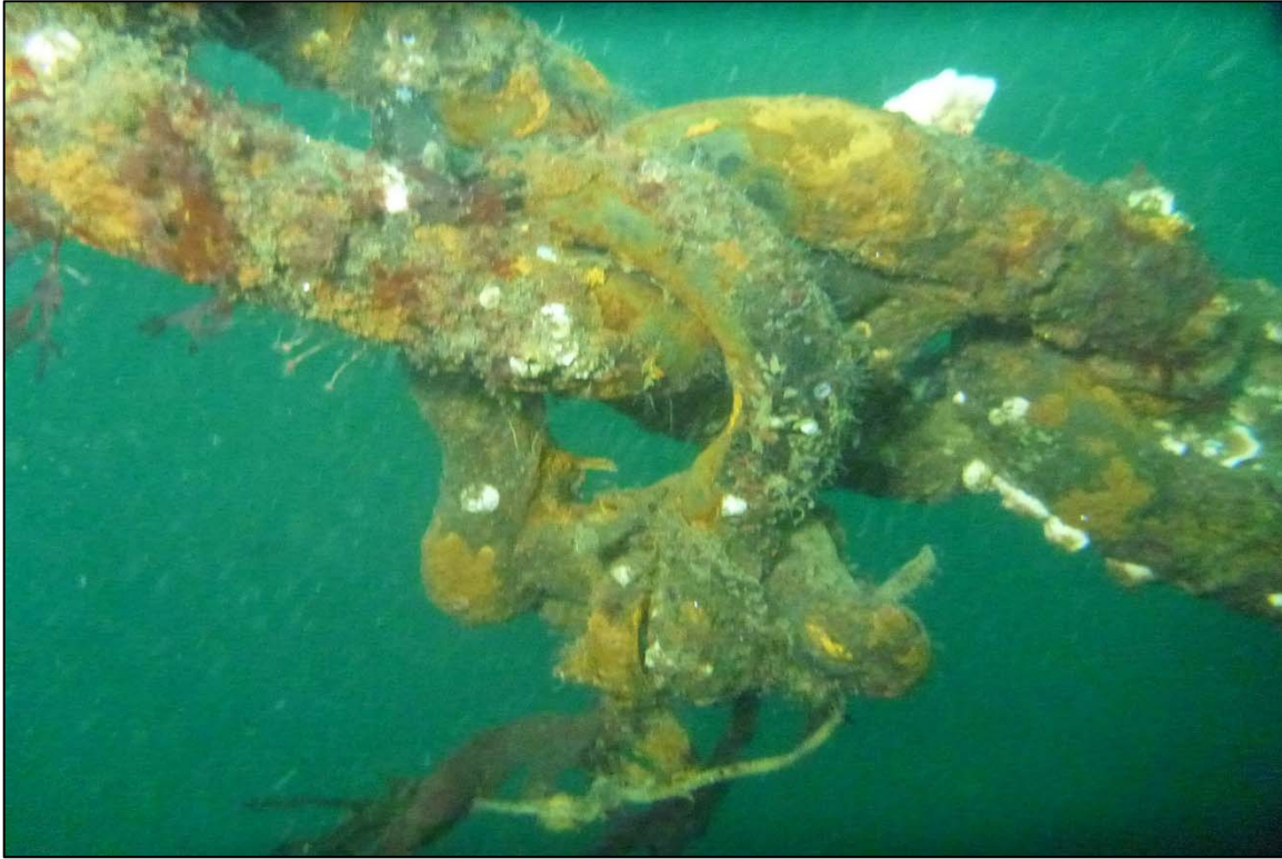
Photograph 47: View of Moderate Corrosion on the Upper Anchor Chain at Site 1 Anchor Chain 12, Looking North.
