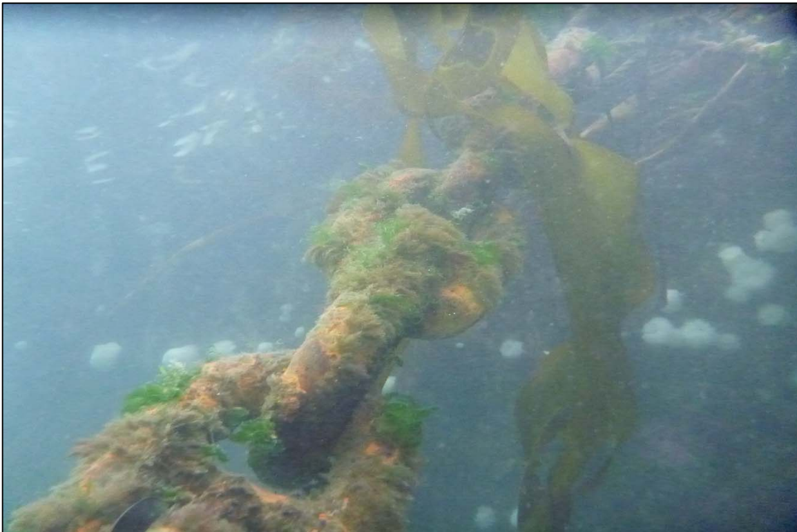
Photograph 22: View of Marine Growth and Light Corrosion on the Upper Anchor Chain at Site 1 Anchor Line 4, Looking Northeast.
