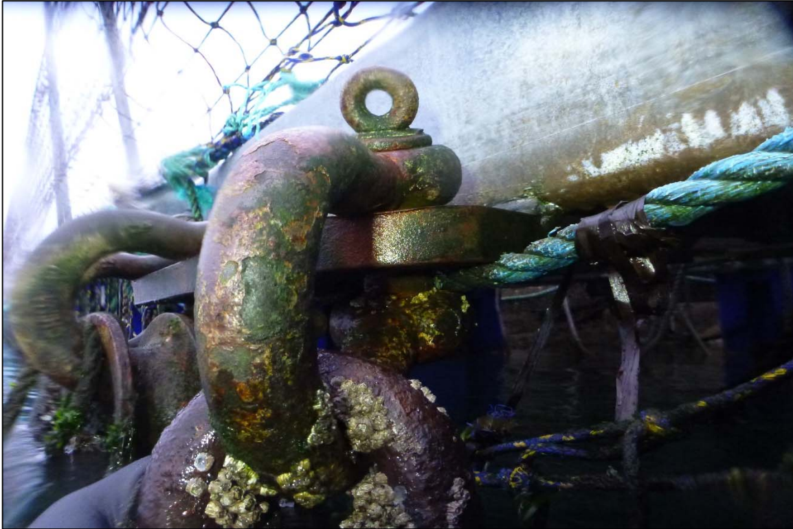
Photograph 29: View of Upper Chain to Float Connection (Shackle) at Site 3 Anchor Line 6A, Looking West.
