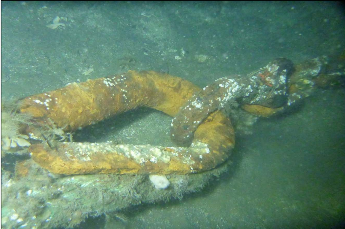
Photograph 39: View of Lower Anchor Chain to Rope Connection (Shackle and Thimble) at Site 3 Anchor Line 8, Looking North.
