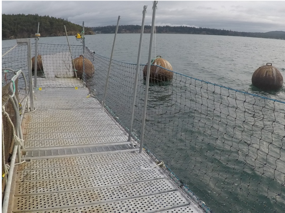
Figure C-5: Cypress Island Net Pen Site 3 – Anchor Lines 5, 6, 6A, and 7 on northeast corner
