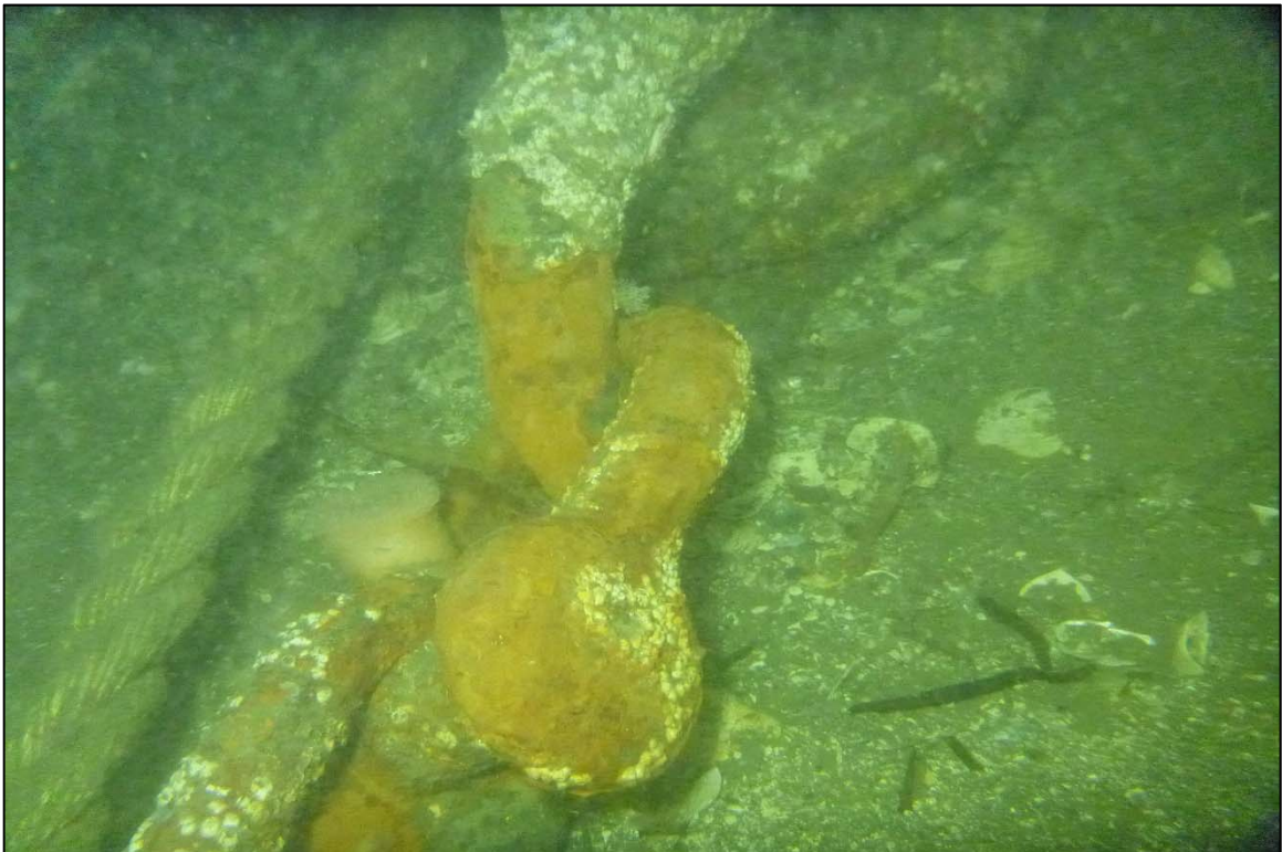
Photograph 32: View of Lower Anchor Chain to Anchor (Shackle and Stem) on the Channel Bottom at Site 3 Anchor Line 6A, Looking East.
