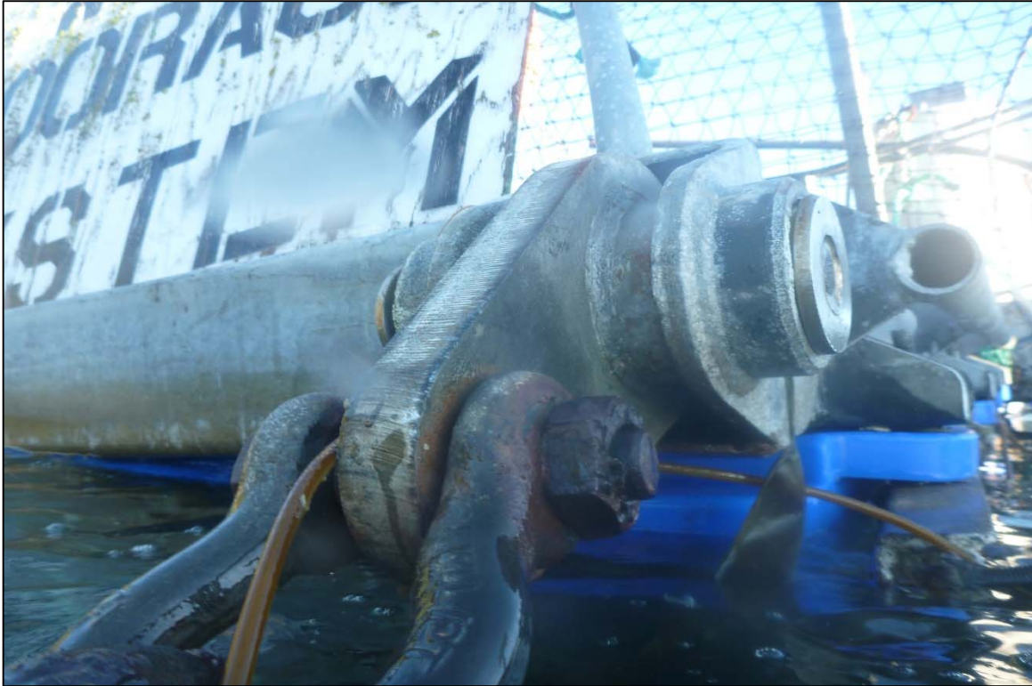
Photograph 63: View of Upper Anchor Chain to Float Connection (Shackle) at Site 3 Anchor Line 18, Looking North.
