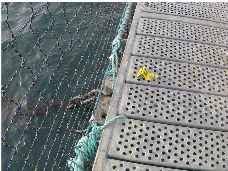
Figure C-10: Cypress Island Net Pen Site 3 – Connection at Anchor Line 12
