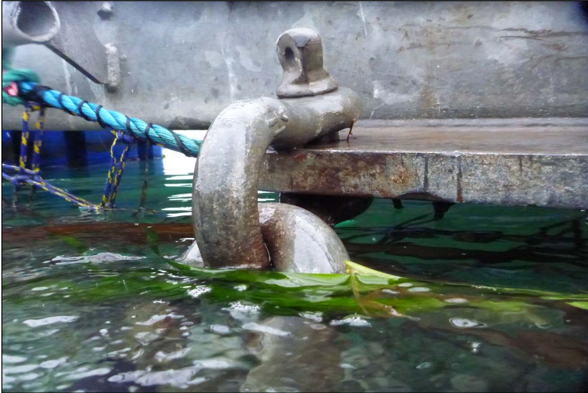
Photograph 11: View of Upper Anchor Chain to Float Connection at Site 3 Anchor Line 21, Looking Southwest.
