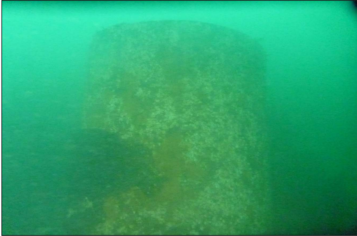
Photograph 73: View of Pile Anchor at Site 3 Anchor Line 21, Looking Northwest.
