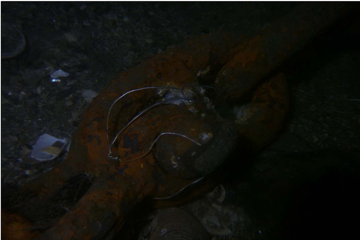
Photograph 66: View of Lower Anchor Chain Condition (Shackle) with Loose Safety Wire and Corrosion at Site 3 Anchor Line 19, Looking West.
