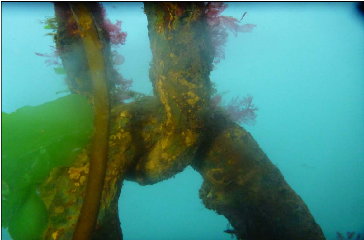
Photograph 76: View of Section Loss on the Buoy Chain due to Abrasion between the Links at Site 3 Anchor Line 23, Looking North.
