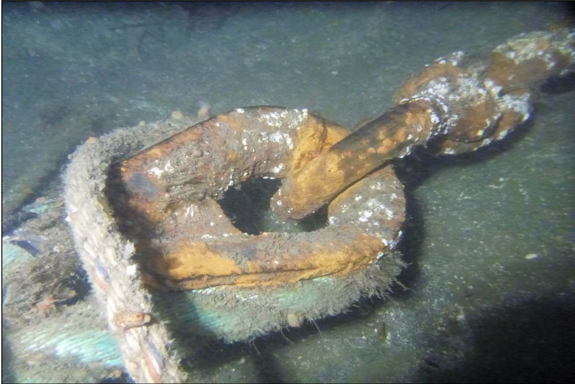
Photograph 43: View of Lower Anchor Chain to Anchor Rope Connection (Shackle and Thimble) at Site 3 Anchor Line 9, Looking East.
