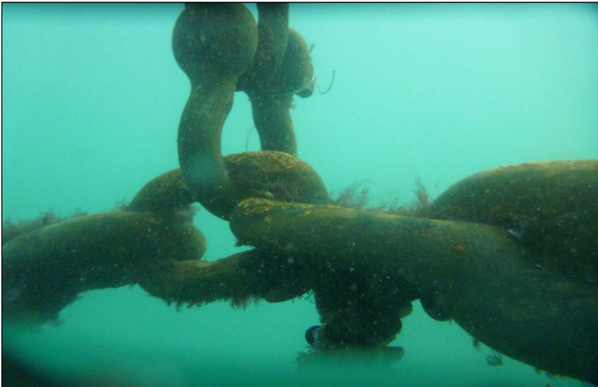
Photograph 86: View of Upper Anchor Chain to Buoy Chain (Shackle) at Site 3 Anchor Line 28, Looking East.
