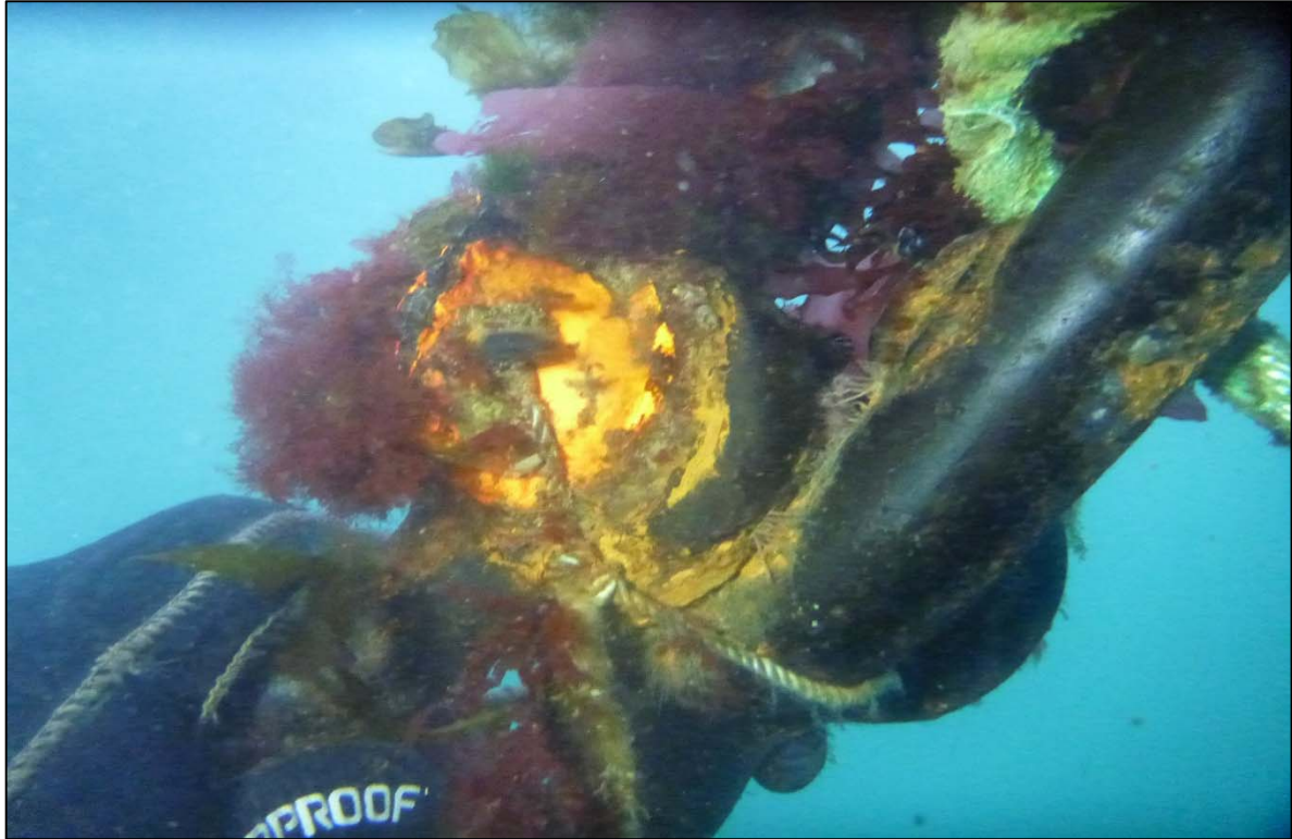
Photograph 35: View of Upper Anchor Chain to Anchor Rope Connection (Shackle and Safety Rope) at Site 3 Anchor Line 7, Looking Southeast.
