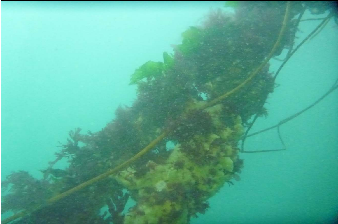
Photograph 25: View of Upper Anchor Chain Condition at Site 3 Anchor Line 5, Looking Northwest.
