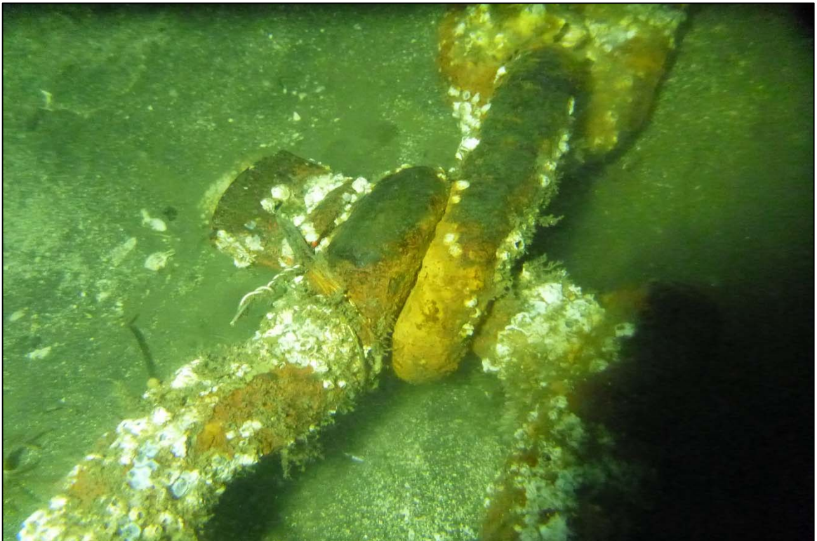
Photograph 40: View of Lower Anchor Chain to Anchor Connection (Shackle and Stem) at Site 3 Anchor Line 8, Looking North.
