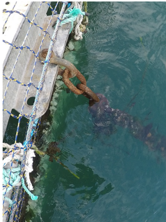
Figure C-24: Cypress Island Net Pen Site 3 – Connection at Anchor Line 26
