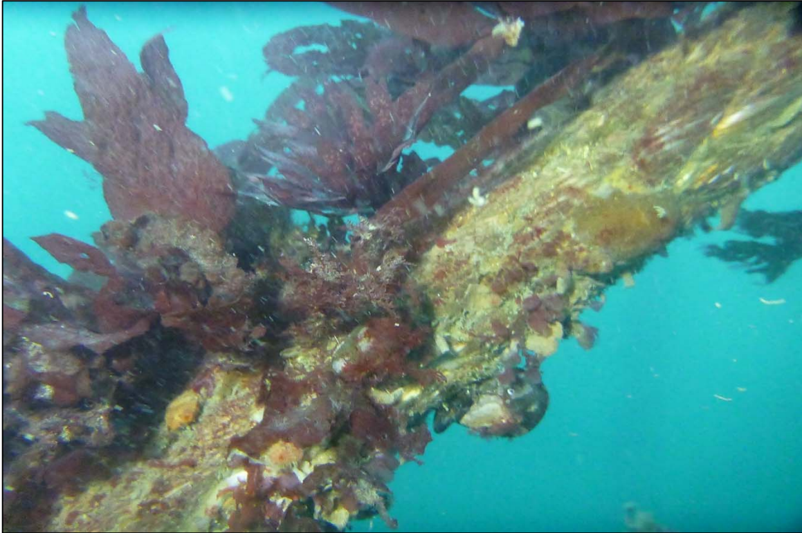
Photograph 19: View of Heavy Marine Growth on the Anchor Rope at Site 3 Anchor Line 3, Looking North.
