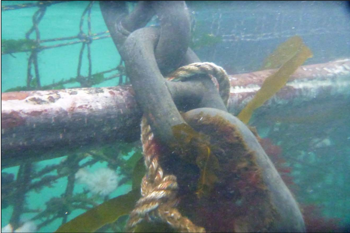
Photograph 41: View of Upper Chain with Trapped Timber Debris between Predator Net and Anchor Chain at Site 3 Anchor Line 9, Looking Northwest.
