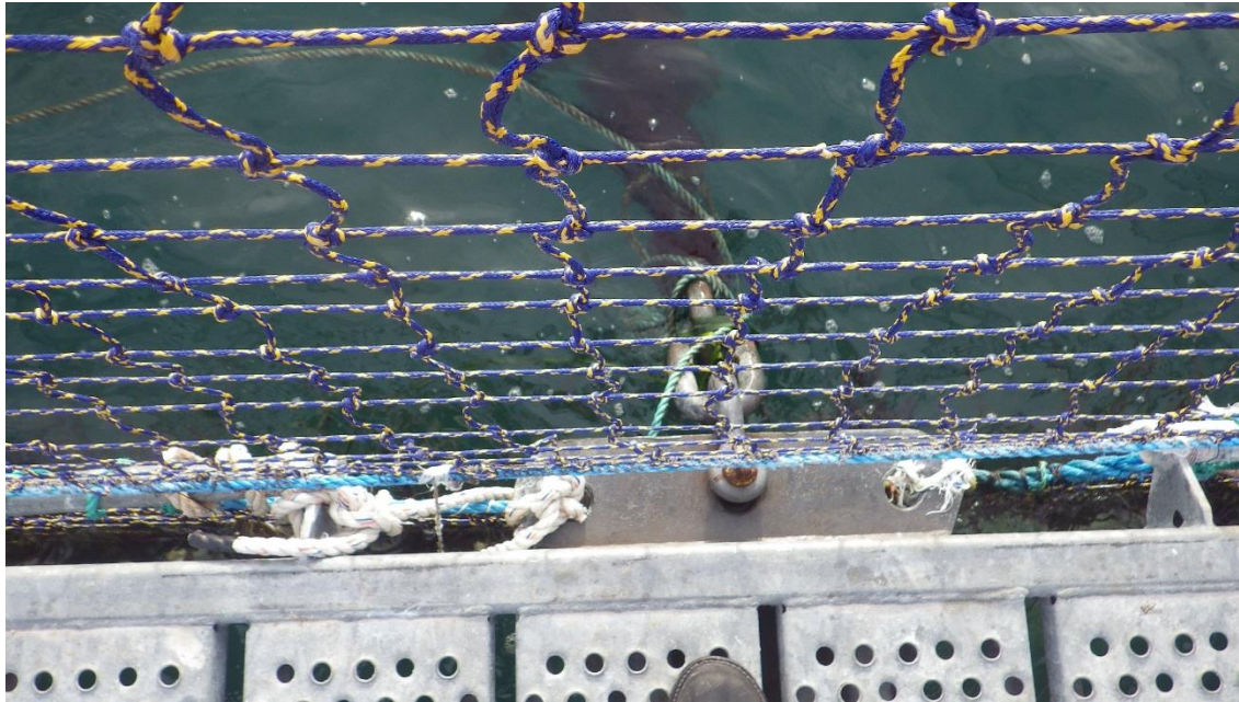
Figure 6: Cypress Island Site 3 Typical Mooring Bracket
