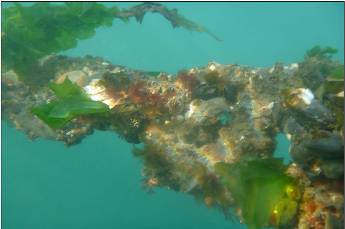
Photograph 58: View of Upper Anchor Chain to Anchor Rope Connection with Heavy Marine Growth at Site 3 Anchor Line 15, Looking Southwest.
