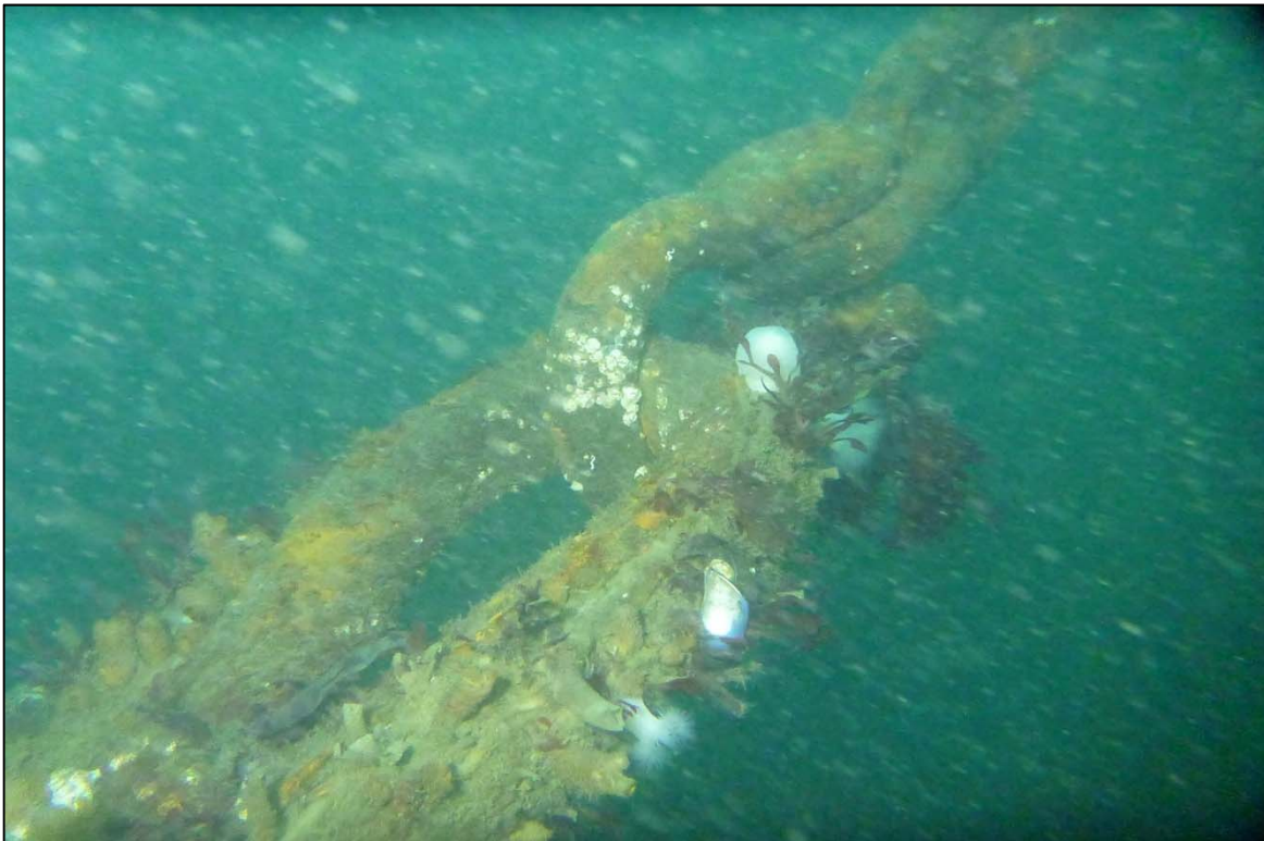
Photograph 16: View of Rope to Lower Anchor Chain Connection (Shackle and Thimble) at Site 3 Anchor Line 2, Looking North.
