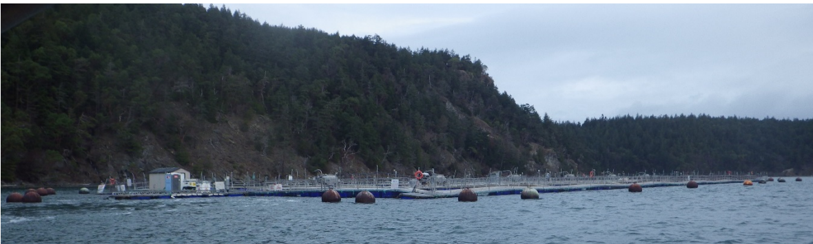
Figure C-2: Cypress Island Net Pen Site 3 – Overview from southeast
