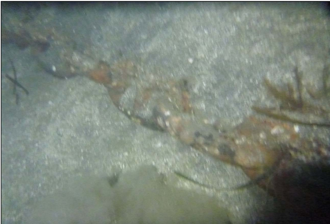
Photograph 44: View of Lower Anchor Chain Mostly Buried at the Channel Bottom Anchor Line 9, Looking North.
