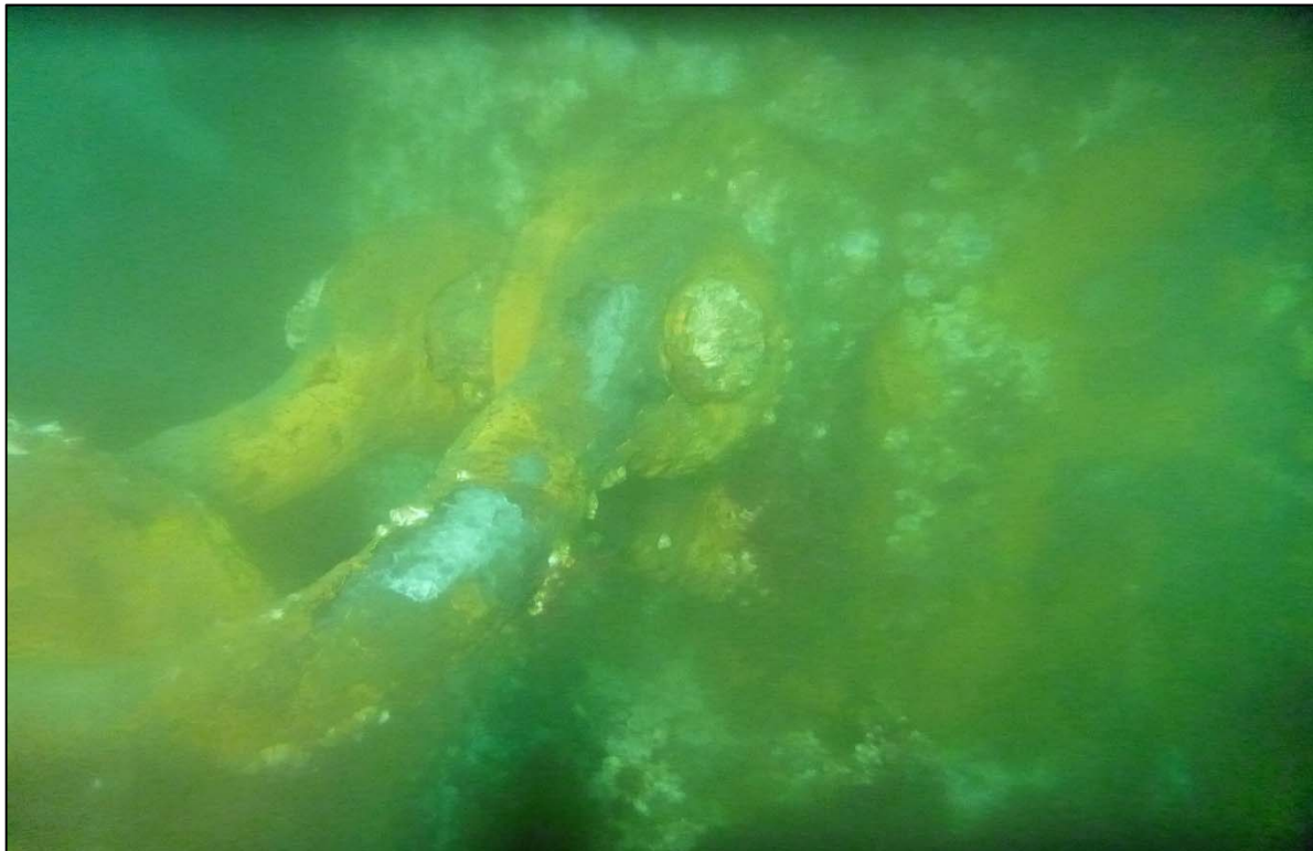
Photograph 84: View of Lower Anchor Chain to Anchor Connection with (Shackle) at Site 3 Anchor Line 27, Looking North.
