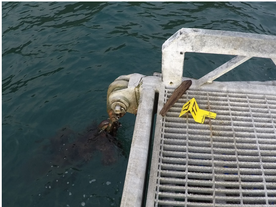
Figure C-14: Cypress Island Net Pen Site 3 – Connection at Anchor Line 17
