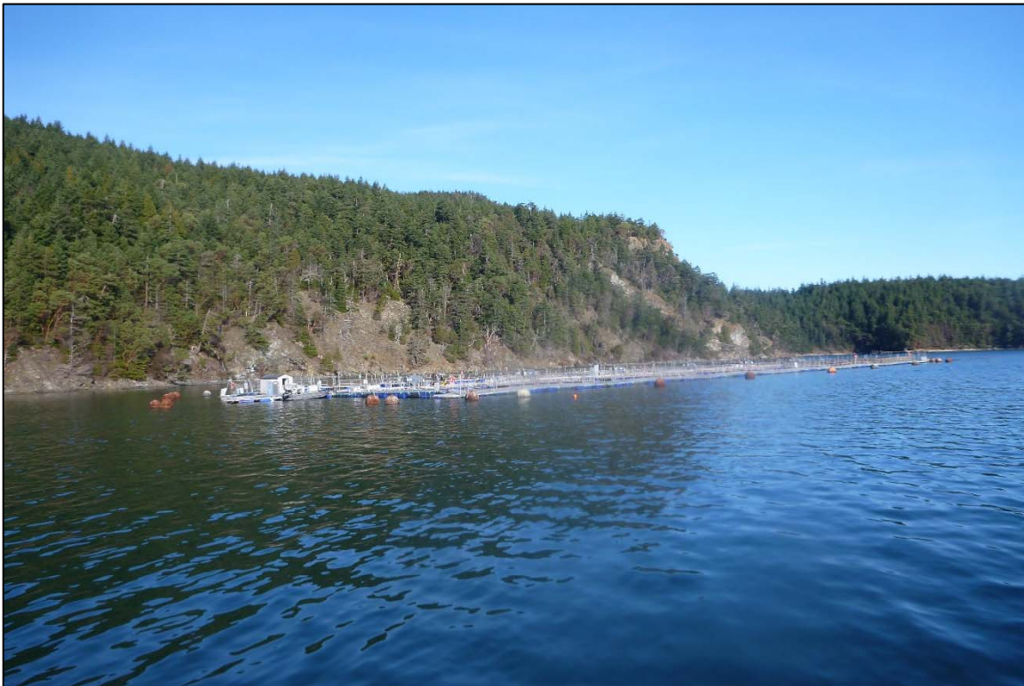
Photograph 2: Overall View of the Site 3 Fish Net Pens System, Looking North.
