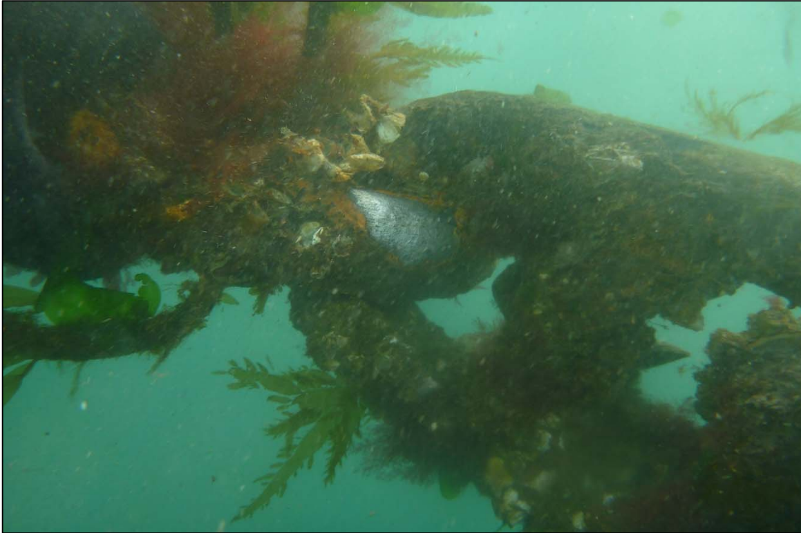
Photograph 59: View of Upper Anchor Chain Condition with Corrosion at Site 3 Anchor Line 16, Looking North.
