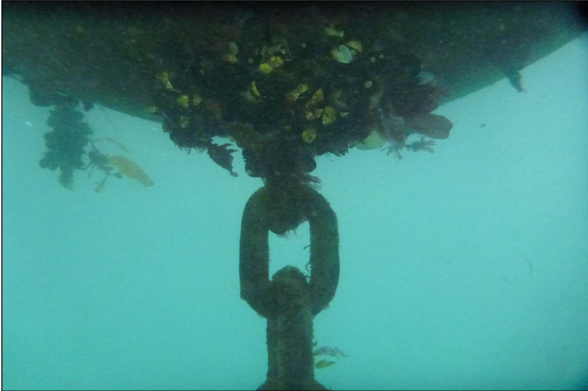
Photograph 71: View of Buoy Connection at Site 3 Anchor Line 21, Looking Northeast.
