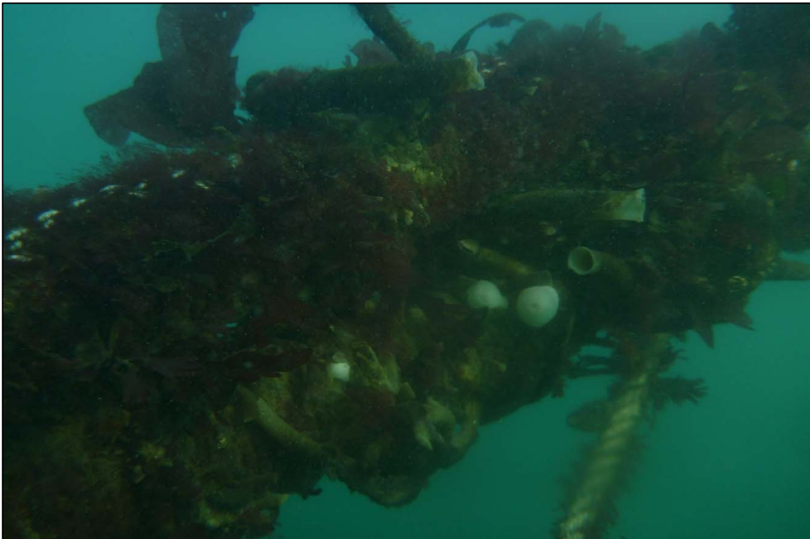
Photograph 64: View of Anchor Rope with Heavy Marine Growth at Site 3 Anchor Line 18, Looking West.
