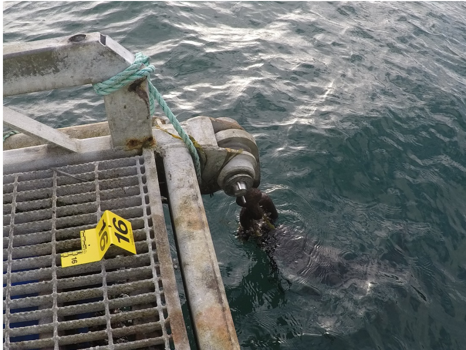
Figure C-13: Cypress Island Net Pen Site 3 – Connection at Anchor Line 16
