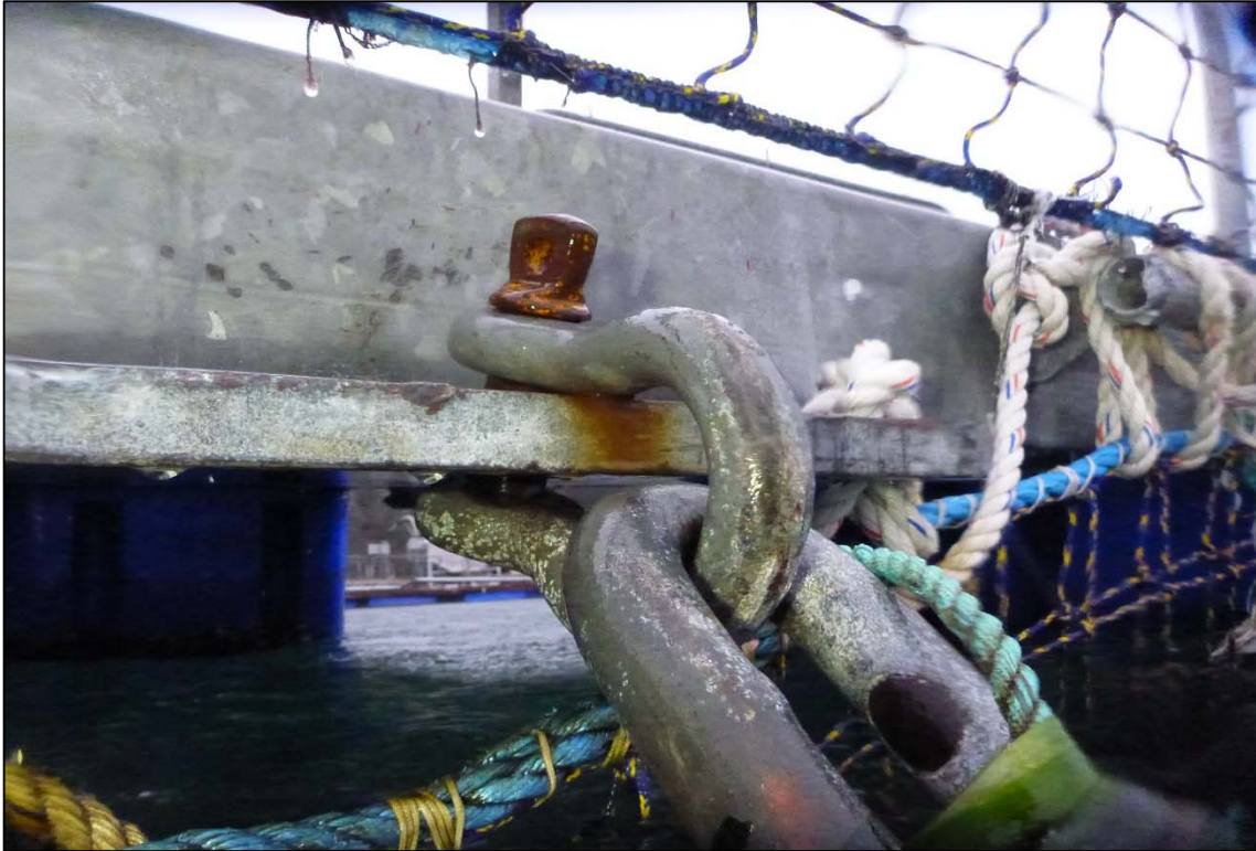
Photograph 45: View of Upper Anchor Chain to Float Connection (Shackle) at Site 3 Anchor Line 10, Looking North.
