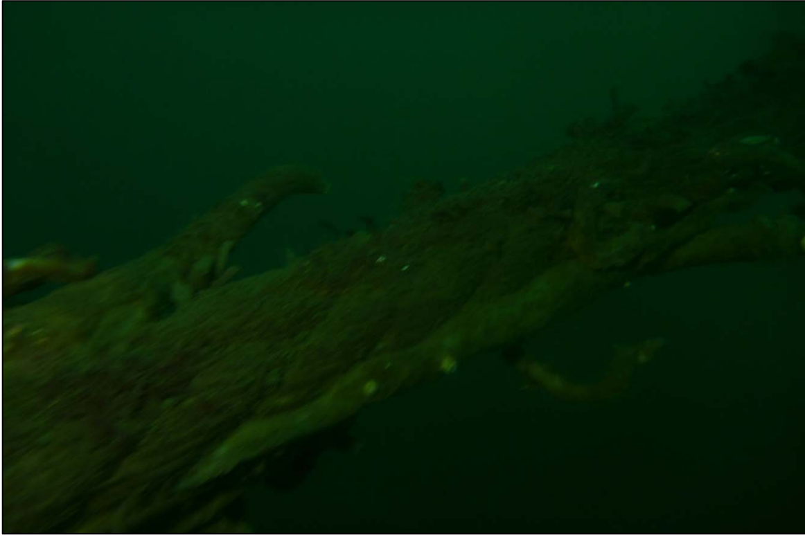
Photograph 57: View of Lower Anchor Rope Condition at Site 3 Anchor Line 14, Looking West.
