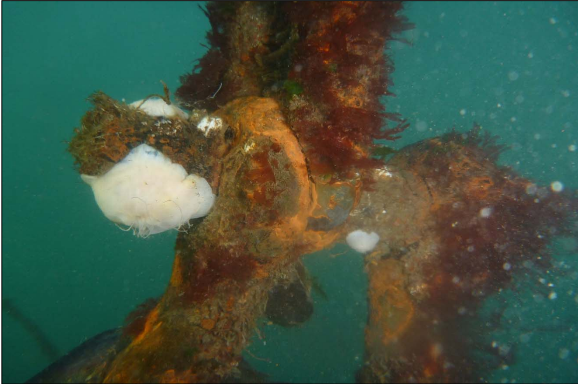
Photograph 65: View of Anchor Chain to Buoy Chain Connection (Shackle) with Corrosion and Pitting at Site 3 Anchor Line 19, Looking Northwest.
