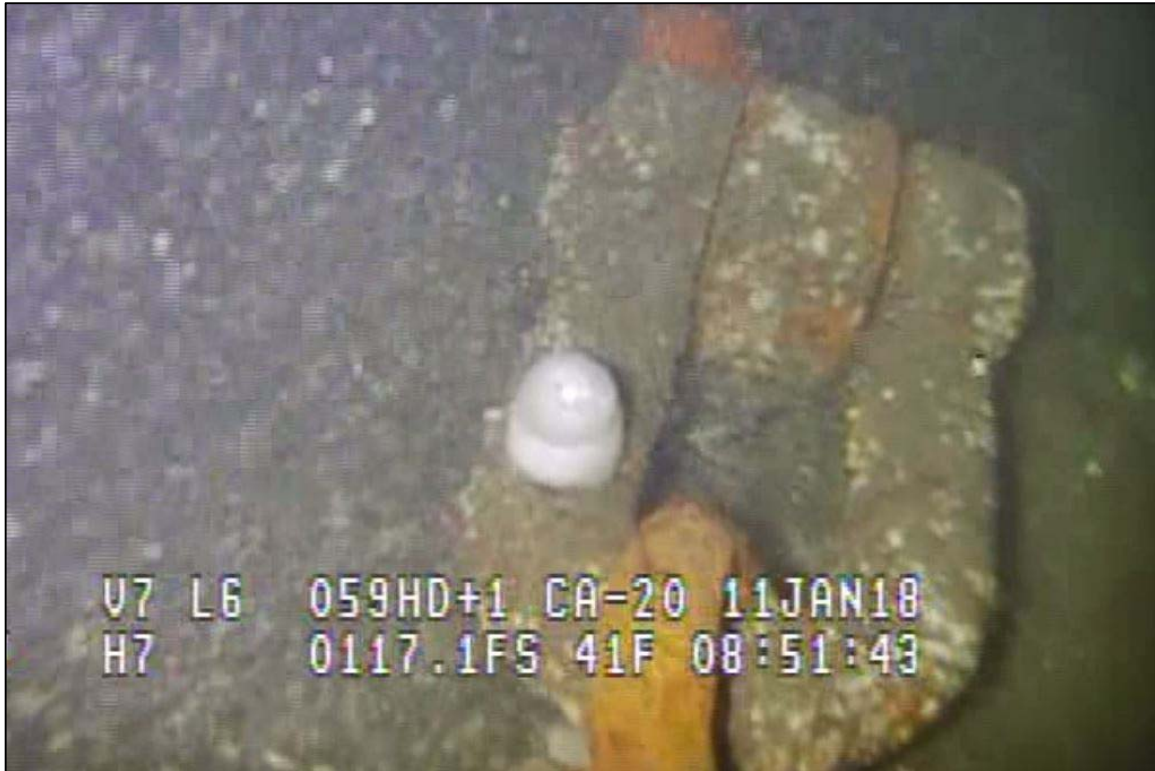
Photograph 17: View of Lower Anchor Chain to Anchor Stem Connection (Shackle) at Site 3 Anchor Line 2, Looking North.
