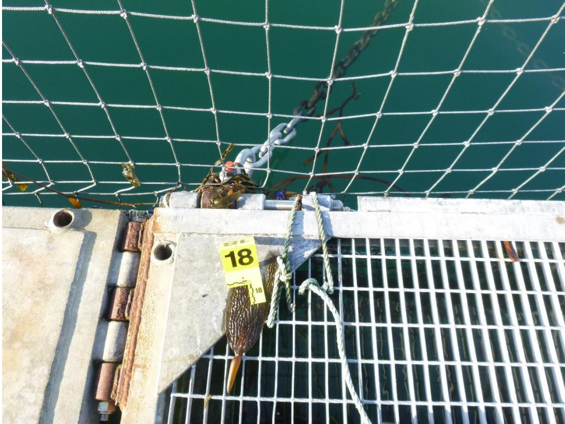
Figure C-60: Anchor 18 Left Padeye, Shackle and Chain
