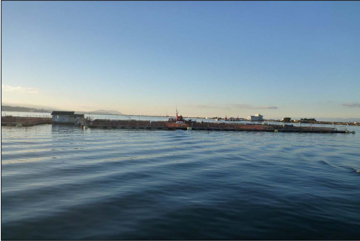
Photograph 3: Overall View of the Primary Fish Net Pens System, Looking West.
