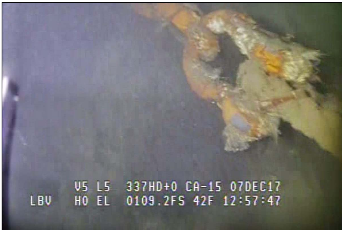
Photograph 63: View of Lower Anchor Chain to Rope Connection (Rope and Shackle) at Primary System Anchor Line 19, Looking Northwest.
