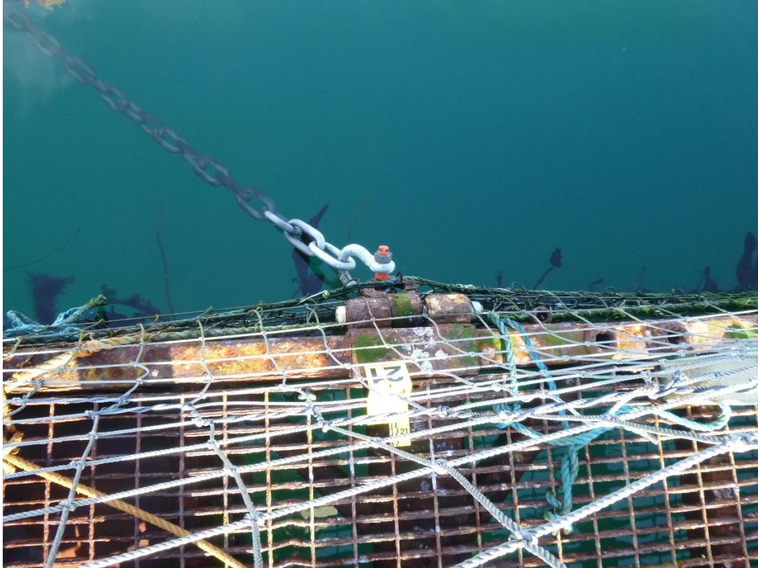
Figure C-70: Anchor 21 Right Padeye, Shackle and Chain (Single Hinge Setup)
