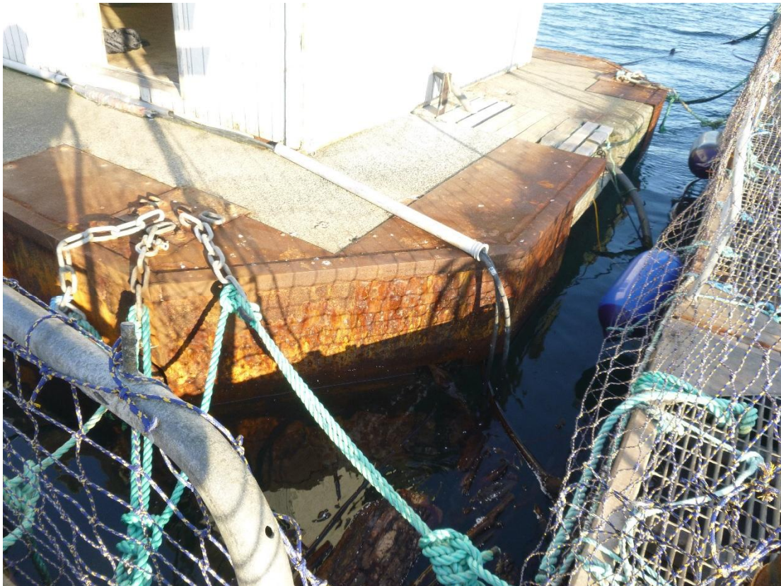
Figure C-91: Southwest Corner of Office and Gen-set Barge – Looking East
