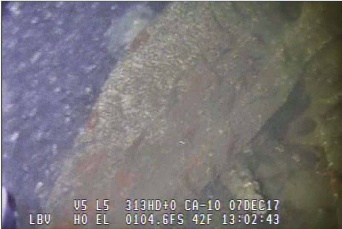
Photograph 68: View of Anchor South Fluke Exposure in the Channel Bottom at Primary System Anchor Line 19, Looking West.
