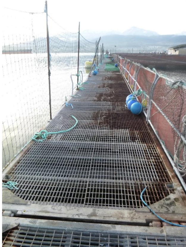
Figure C-8: Floating Docks Between Anchor 2 and 3 (Looking South)
