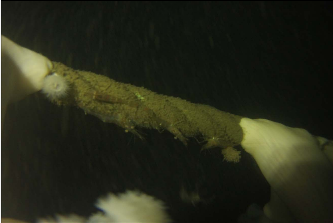
Photograph 33: View of Rope with Minor Marine Growth at Anchor 10 (Typical), Looking South.
