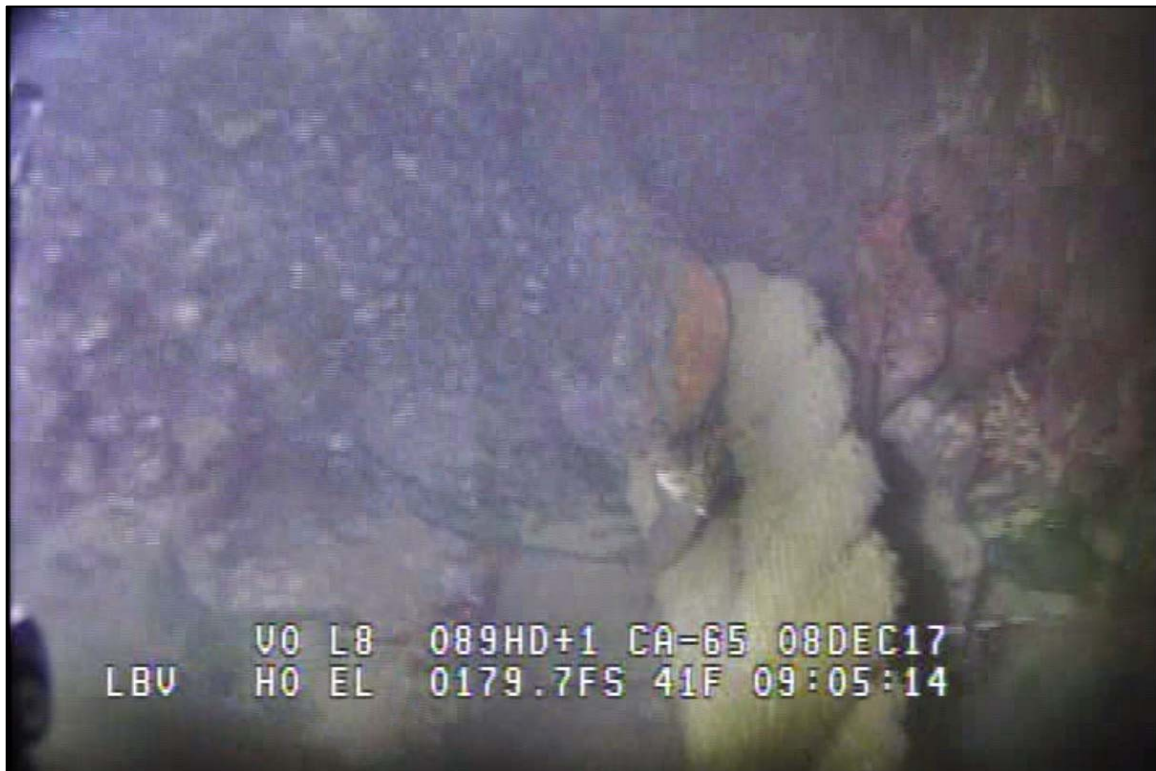
Photograph 44: View of Lower Anchor Chain to Rope Connection (Rope and Shackle) at Primary System Anchor Line 11, Looking South.
