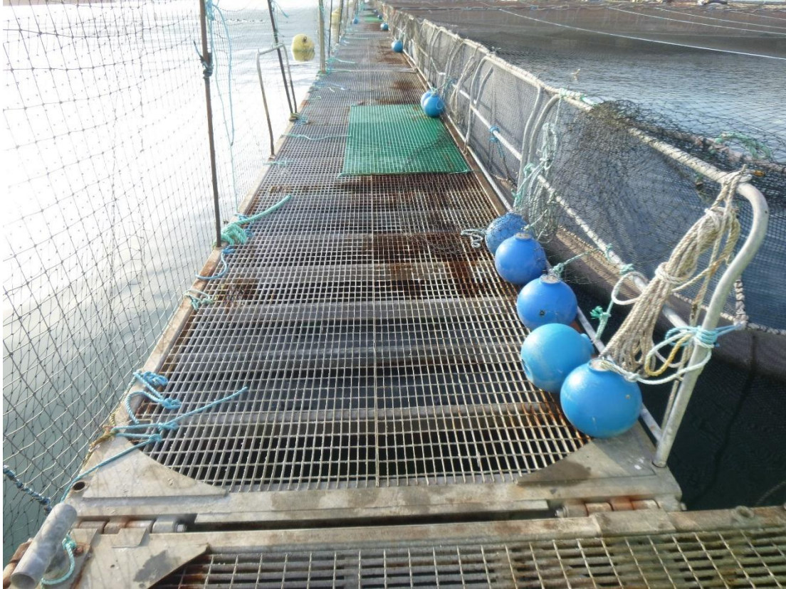
Figure C-4: Floating Docks Between Anchor 1 and 2 (Looking South)
