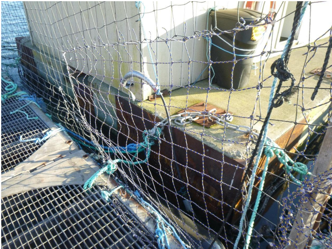
Figure C-87: Northwest Corner of Office and Gen-set Barge – Looking Southeast
