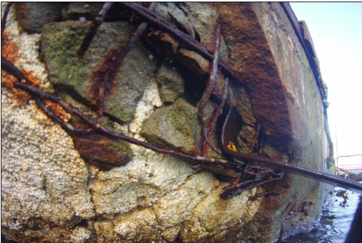
Photograph 22: View of the Area of Section Loss and Exposed Foam Floatation on the Southeast Corner of the Building Barge Float, Looking Northwest.
