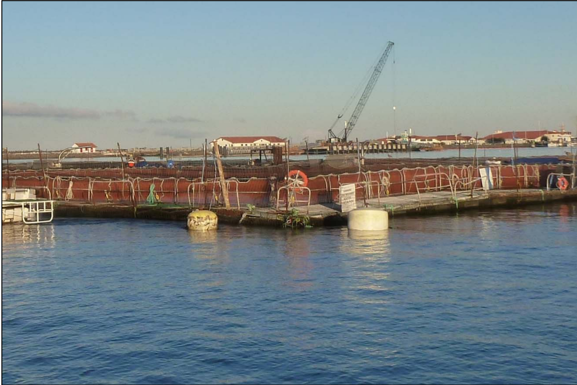
Photograph 7: View of the Typical Anchor Line Buoy Attachment at the Northwest Corner, Looking Southeast.
