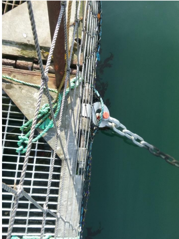
Figure C-46: Anchor 14 Left Shackle and Padeye
