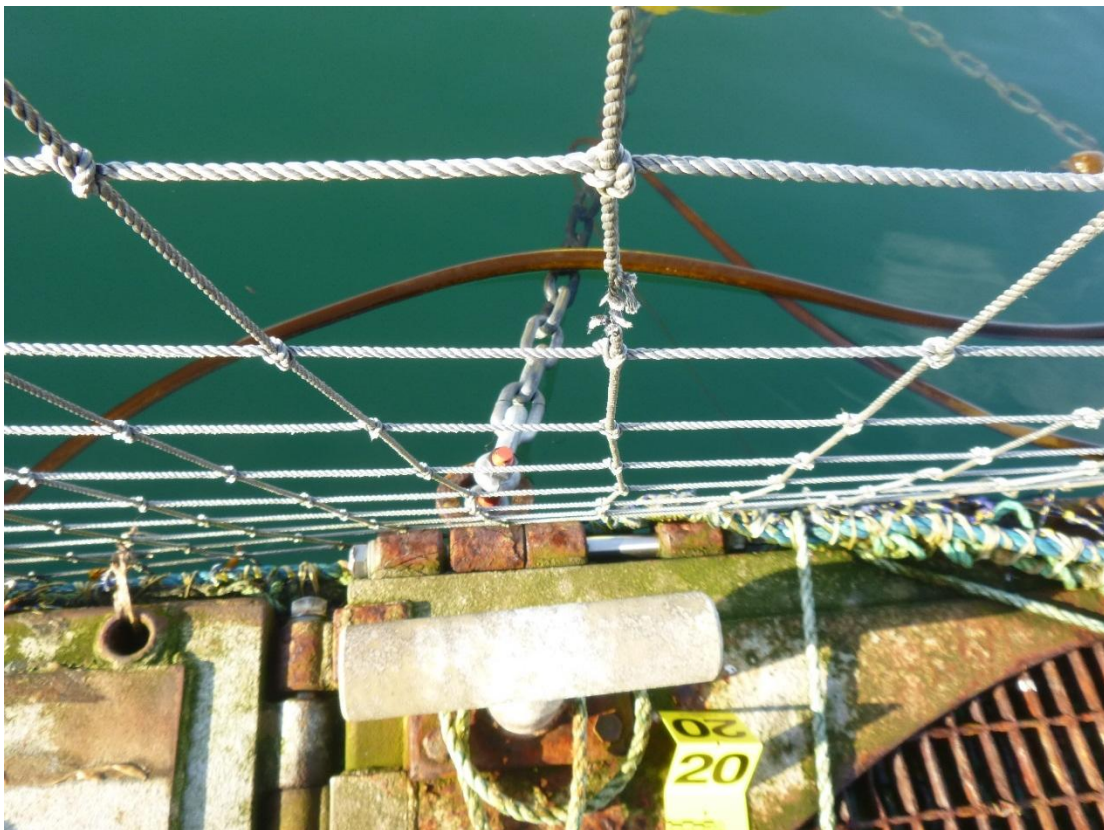
Figure C-67: Anchor 20 Left Padeye, Shackle and Chain
