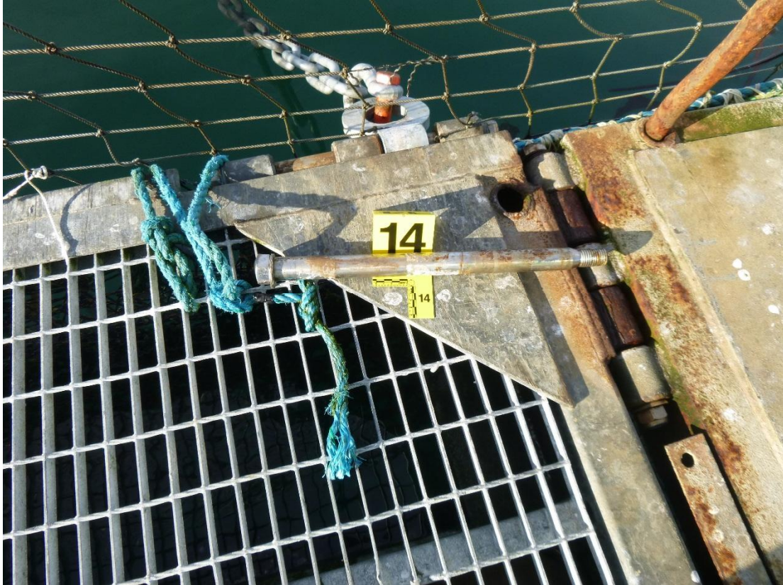
Figure C-44: Anchor 14 Right Shackle, Padeye and Typical S.S. Hinge Pin
