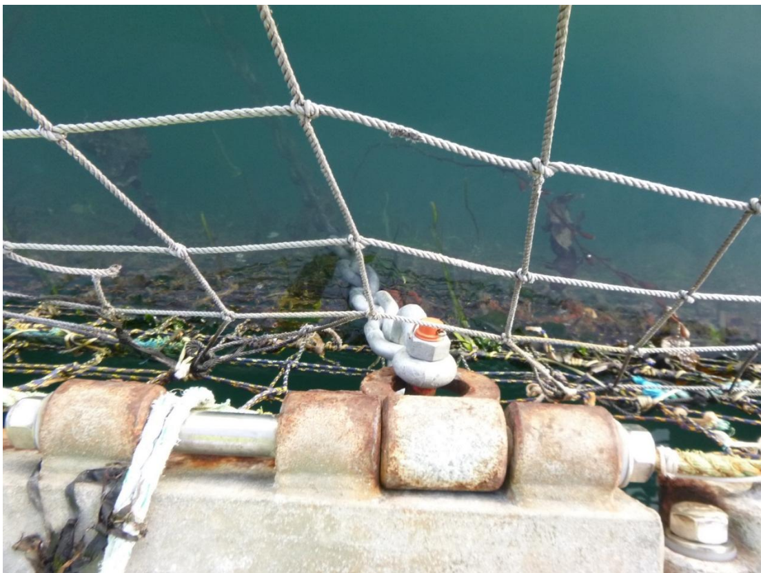
Figure C-7: Anchor 2 Right Bridle Chain
