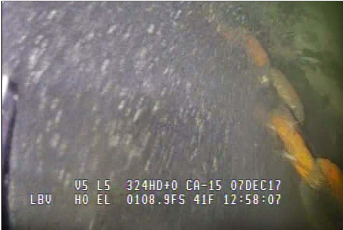
Photograph 64: View of Lower Anchor Chain Condition (Typical) at Primary System Anchor Line 19, Looking West.
