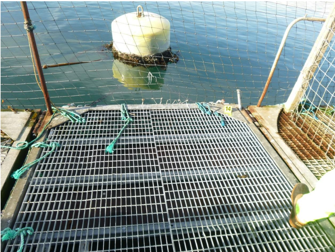
Figure C-43: Anchor 14 (Looking West)
