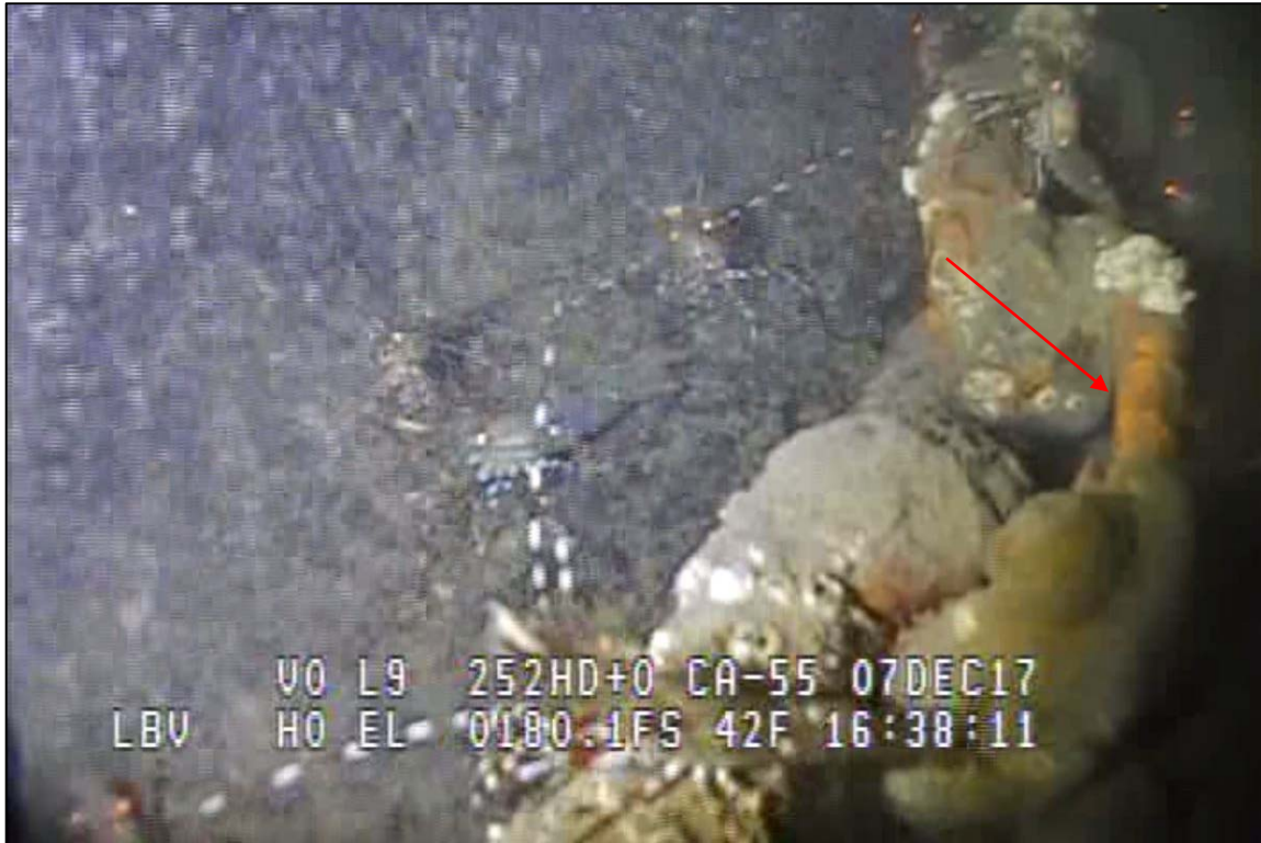
Photograph 51: View of Heavy Section Loss in the Lower Anchor Chain at Primary System Anchor Line 14, Looking West.
