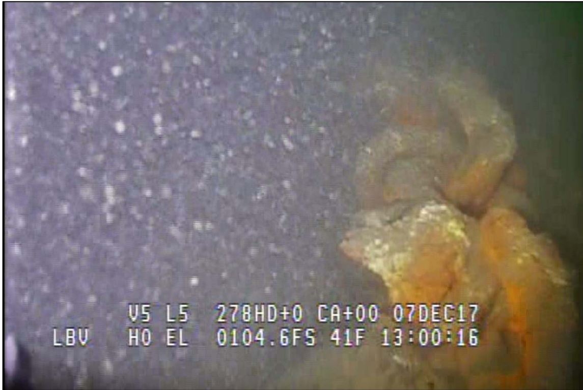
Photograph 66: View of Lower Anchor Chain to Anchor Connection (Shackle) at Primary System Anchor Line 19, Looking West.
