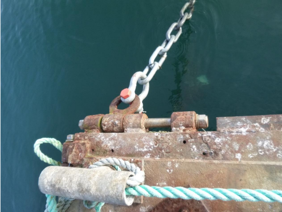
Figure C-16: Anchor 5 Left Padeye, Shackle and Bridle
