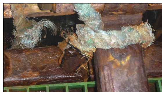
PHOTO 7 TYPICAL CORROSION AND DAMAGE TO PRIMARY FRAME OF BOARDING FLOATS
