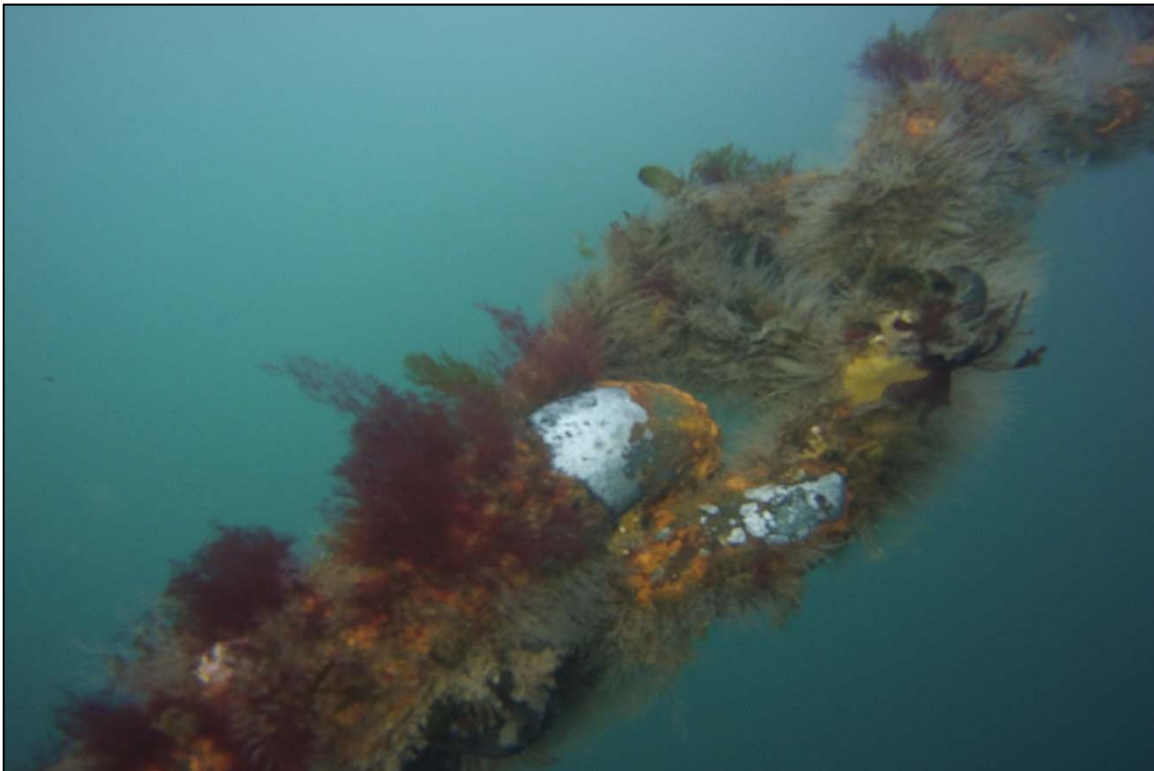
Photograph 30: View of Upper Chain Condition with Heavier Marine Growth at Anchor 8 (Typical), Looking North.
