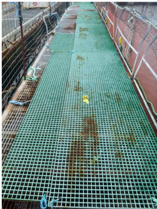
Figure C-77: Location 24 South Edge of Pen 5 (Looking West)
