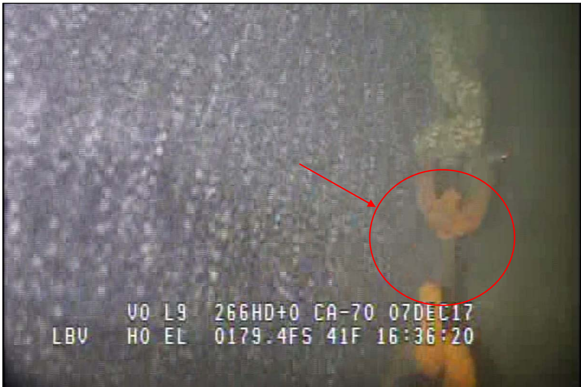
Photograph 50: View of a Broken Chain Link in the Lower Anchor Chain at Primary System Anchor Line 14, Looking West.
