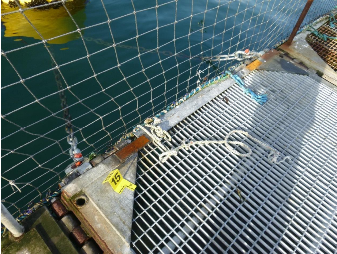
Figure C-48: Anchor 15 Bridle, Shackles and Padeyes
