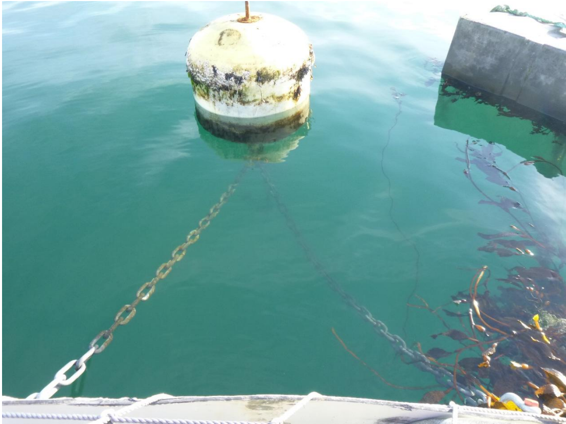
Figure C-28: Anchor 9 Bridle Chain and Buoy
