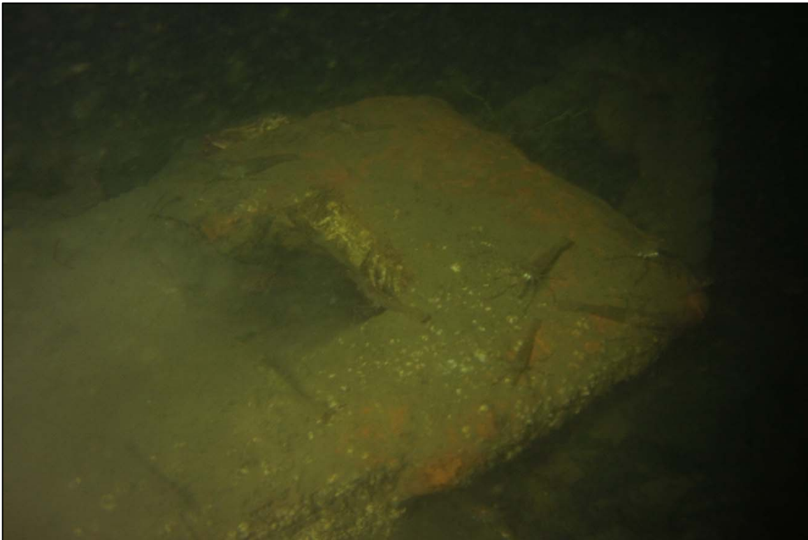
Photograph 36: View of the top of the Anchor at Anchor Line 21 (Typical Observed by Diver), Looking North.
