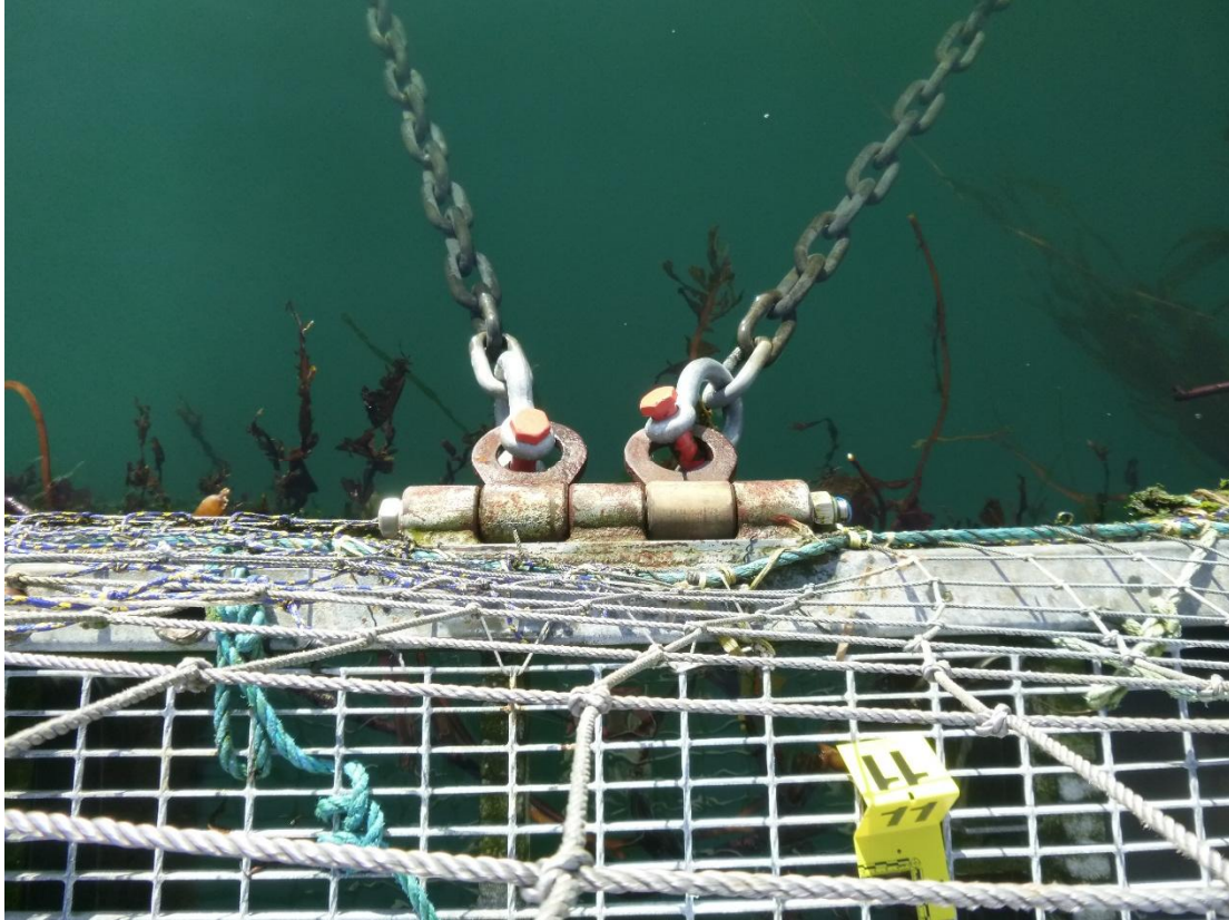
Figure C-36: Anchor 11 Padeye and Bridle on right, Unknown Anchor Chain on left
