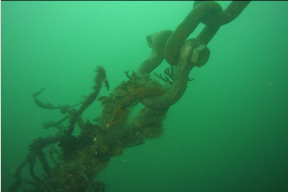
Photograph 31: View of the Upper Rope to Chain Connection at Anchor Line 15 (Typical), Looking South.
