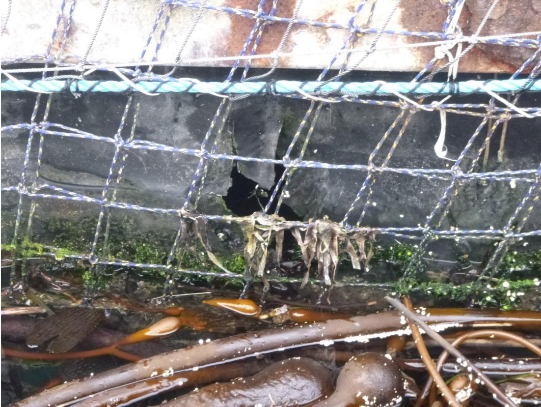
Figure C-76: Location 23 Damaged Pontoon (South Edge of Pen 5)
