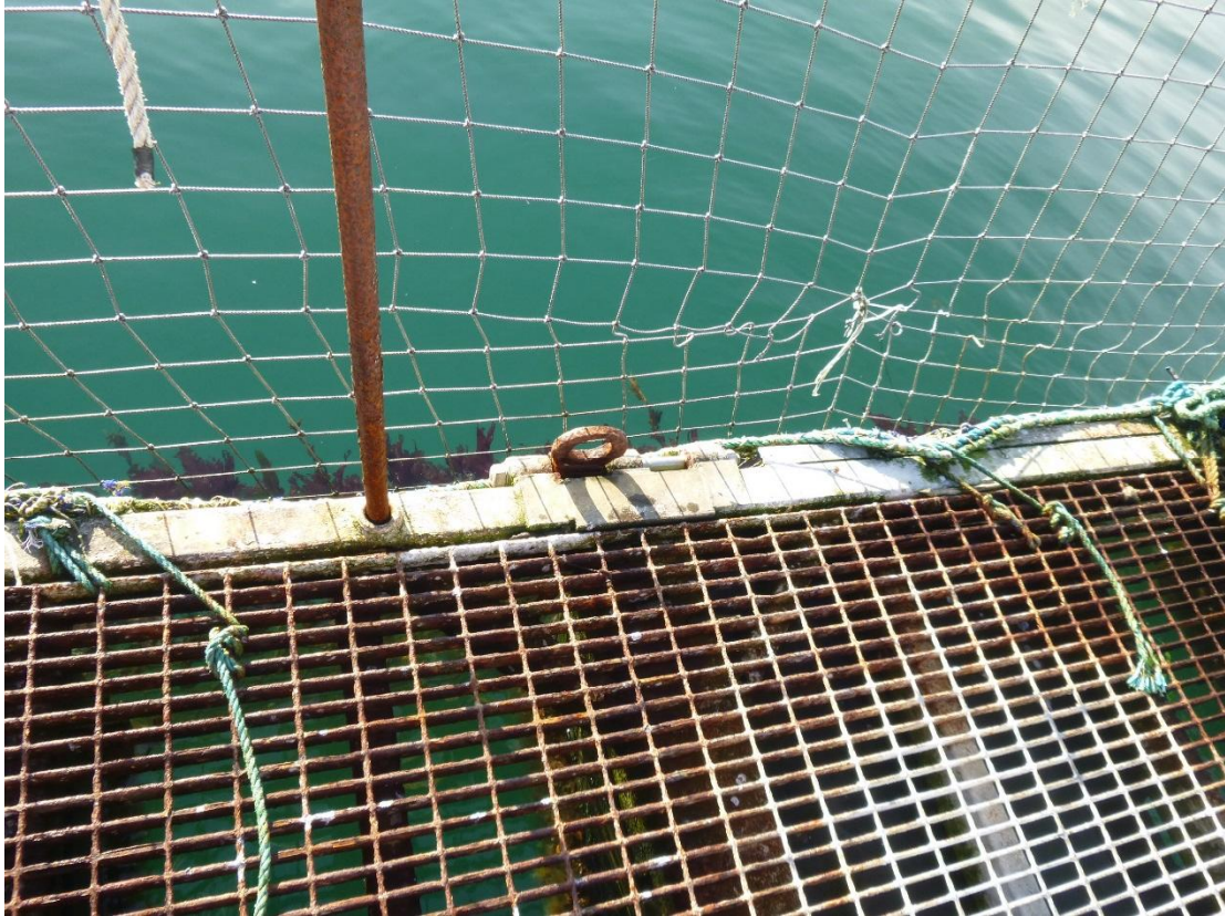
Figure C-34: Padeye Midway Between Anchor 10 and Anchor 11
