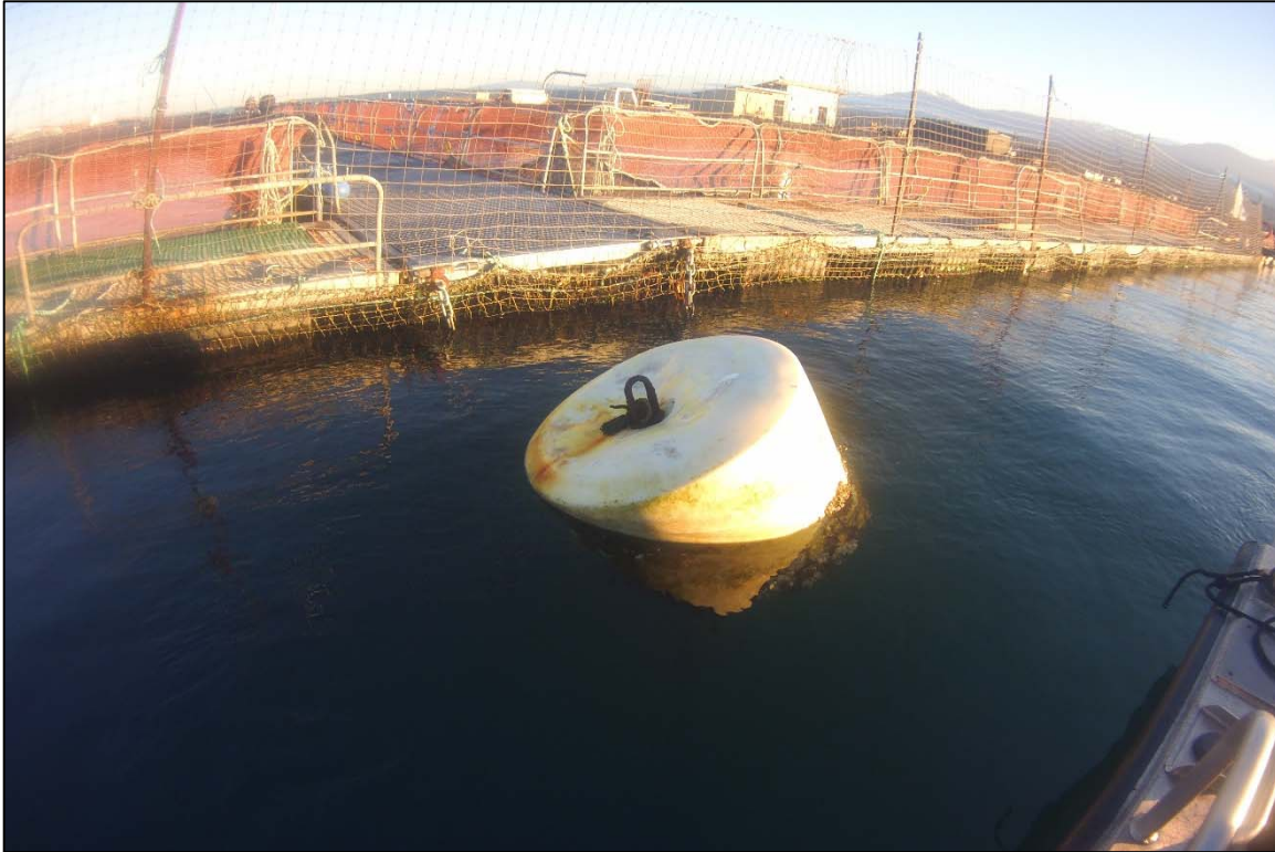
Photograph 13: View of the Depressed Anchor Line Buoy at Anchor Line 20, Looking Southeast.
