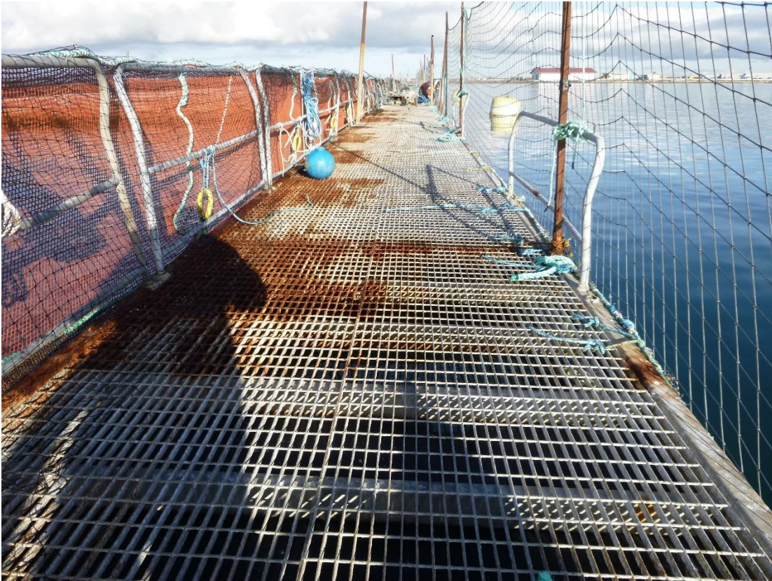
Figure 26: Docks Between Anchor 8 and Anchor 9 (From Anchor 9 looking North)
