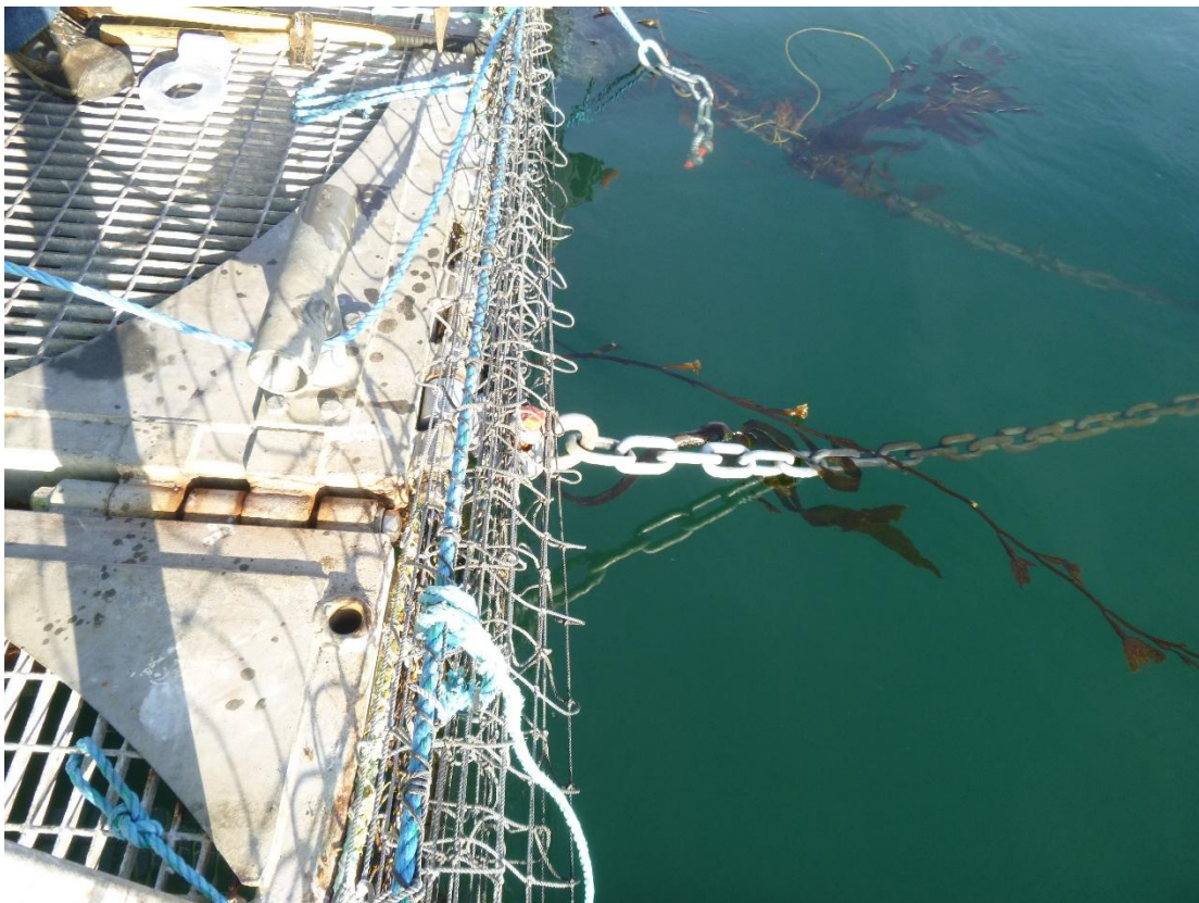
Figure C-25: Anchor 8 Bridle Chain & Shackles
