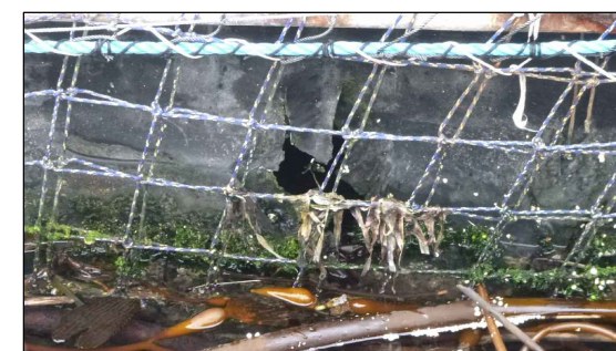
PHOTO 9 DAMAGE TO FLOATING PONTON
