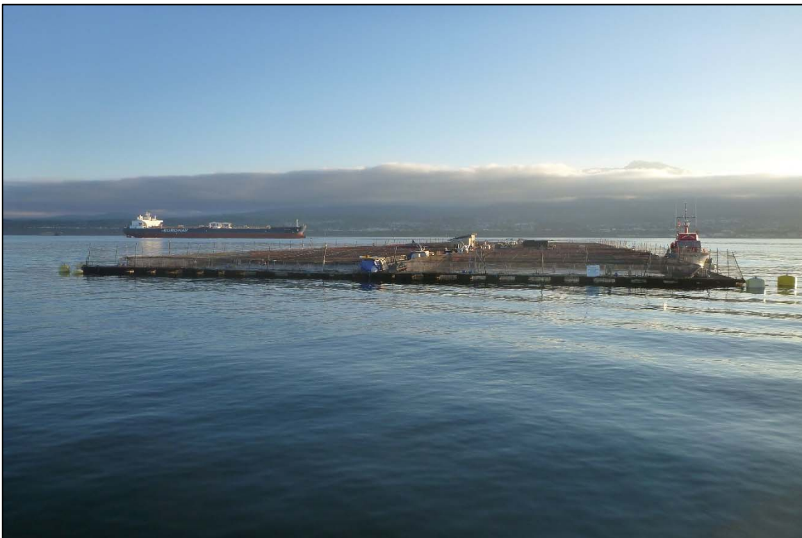
Photograph 2: Overall View of the Primary Fish Net Pens System, Looking South.
