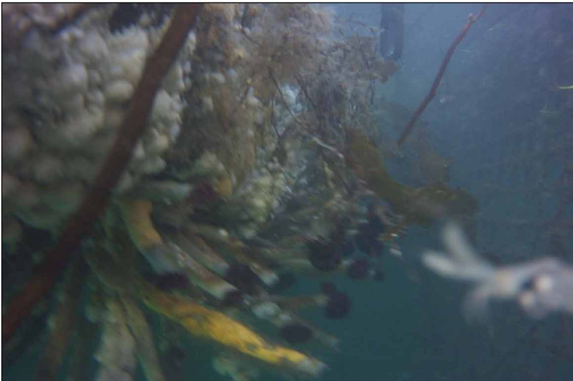
Photograph 26: View of Typical Heavy Marine Growth on the Bottom of the Office Building Barge, Looking West.
