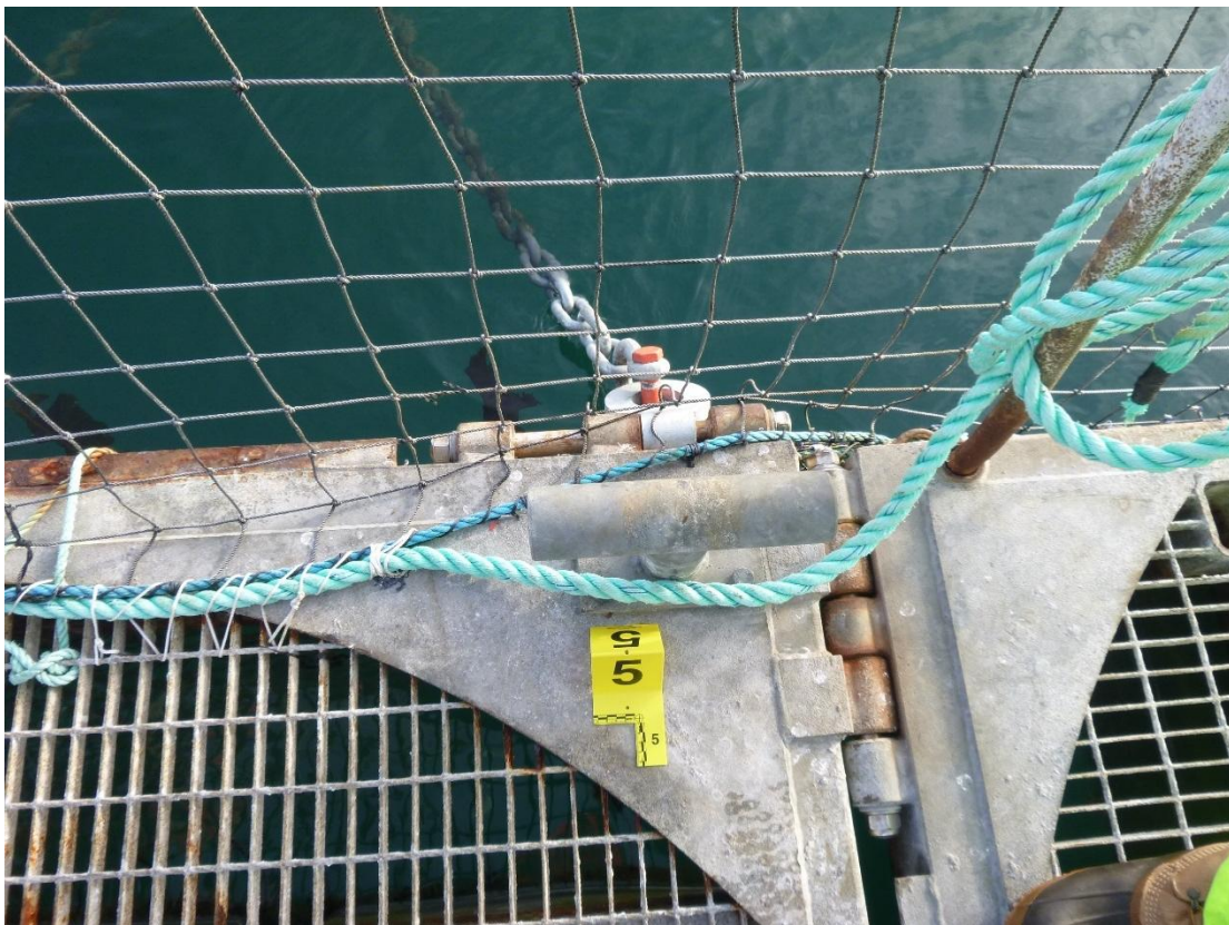
Figure C-15: Anchor 5 New Right Padeye and Shackle
