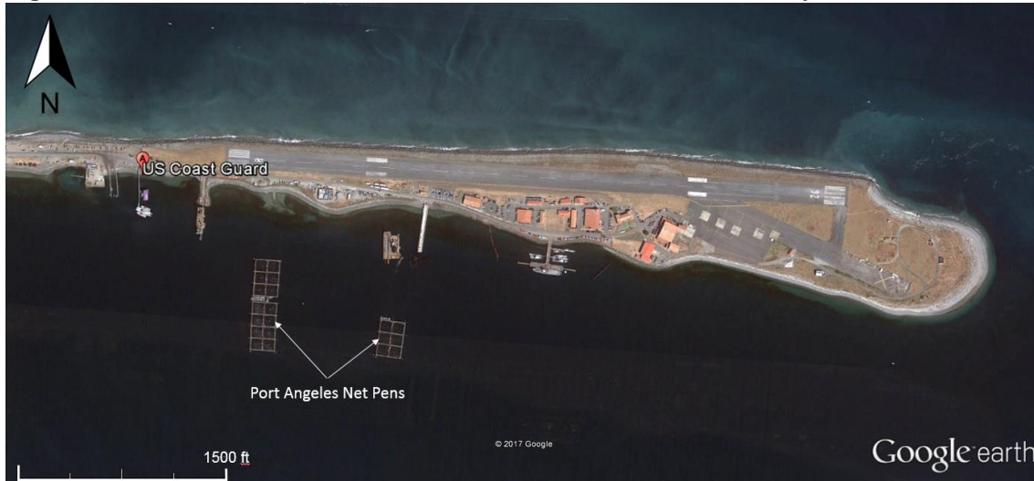
Figure 5: Location of wind observations at the US Coast Guard facility
