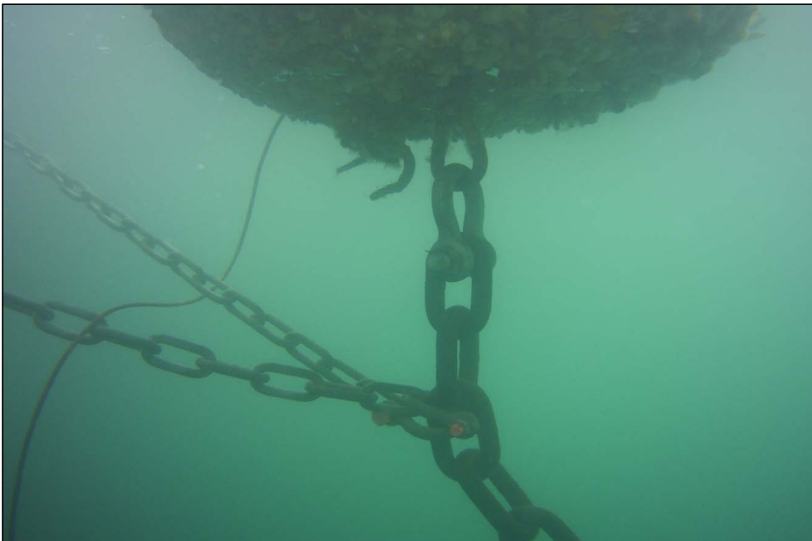
Photograph 16: View of the Typical Buoy, Anchor Chain, and Bridle Chain Connection, Anchor Line 16 Shown.
