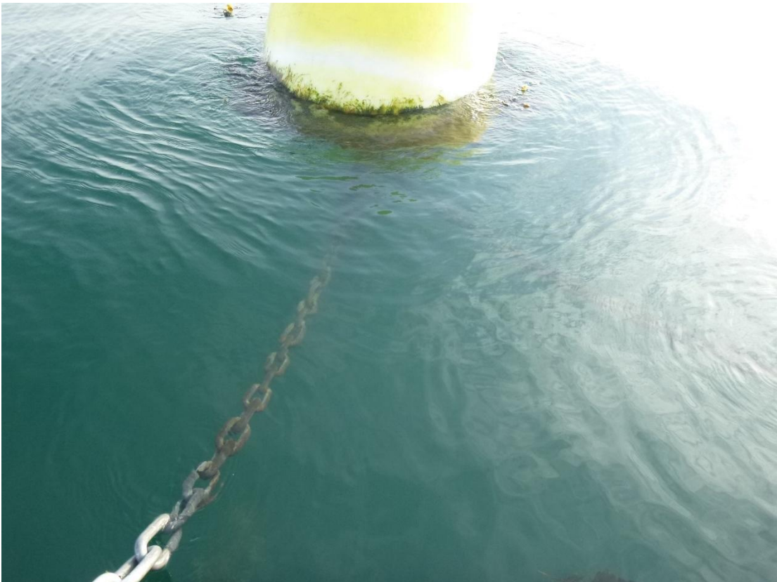
Figure C-17: Anchor 5 Bridle Chain
