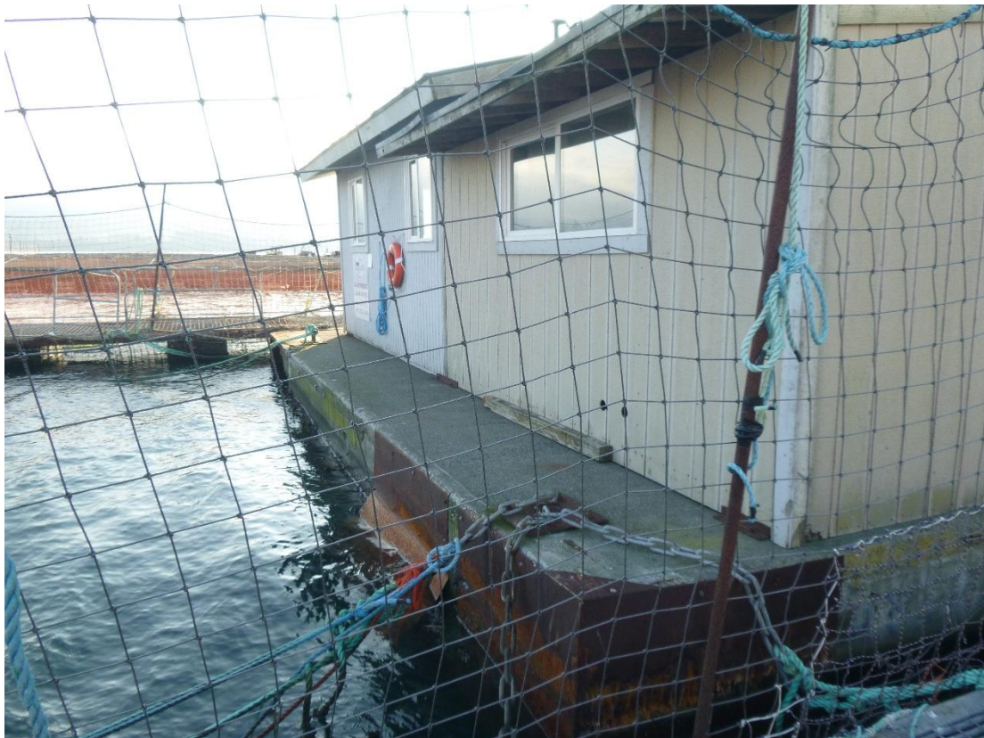
Figure C-85: Northeast Corner of Office and Gen-set Barge – Looking South
