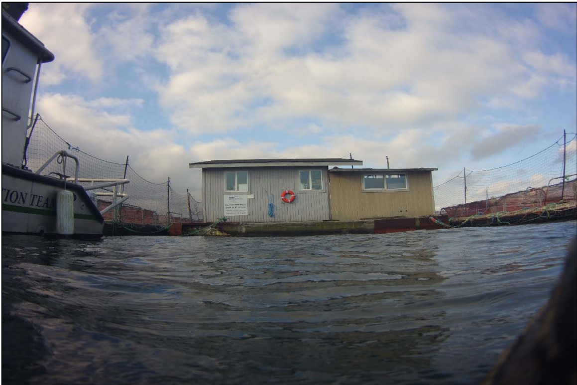
Photograph 20: View of the Storage Buildings Located between Pens 6 and 8, Looking West.
