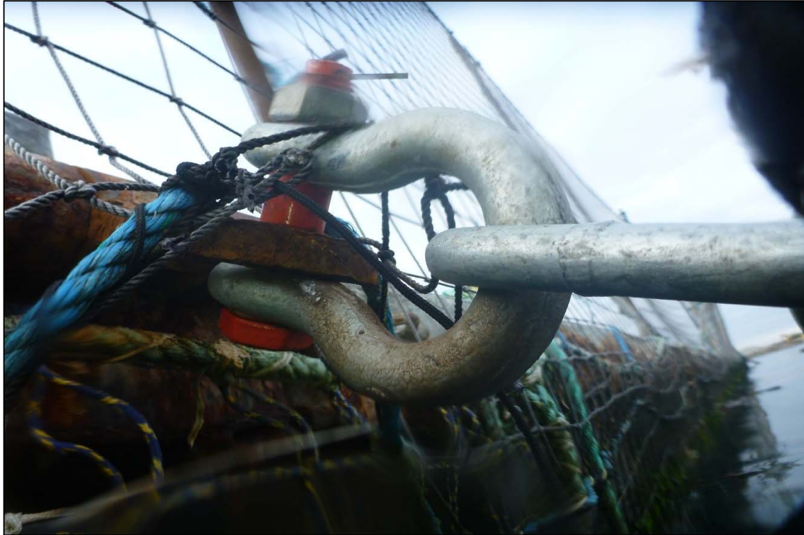
Photograph 27: View of the Upper Pen to Anchor Line Connection (Shackle and Padeye) at Anchor Line 2, Looking West.
