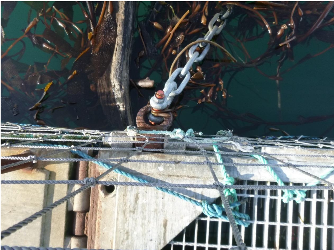
Figure C-65: Anchor 19 Left Padeye and Chain
