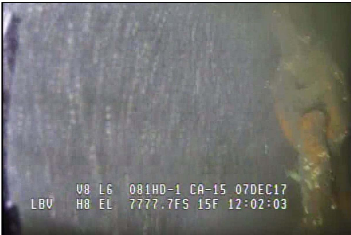
Photograph 40: View of Lower Anchor Chain Condition (Typical) at Primary System Anchor Line 4, Looking East.
