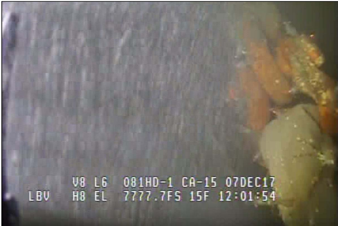
Photograph 39: View of Lower Anchor Chain to Rope Connection at Primary System Anchor Line 4, Looking East.
