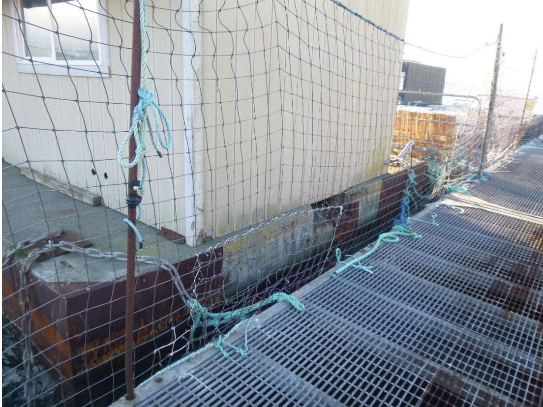
Figure C-86: North Face of Office and Gen-set Barge – Looking Southwest
