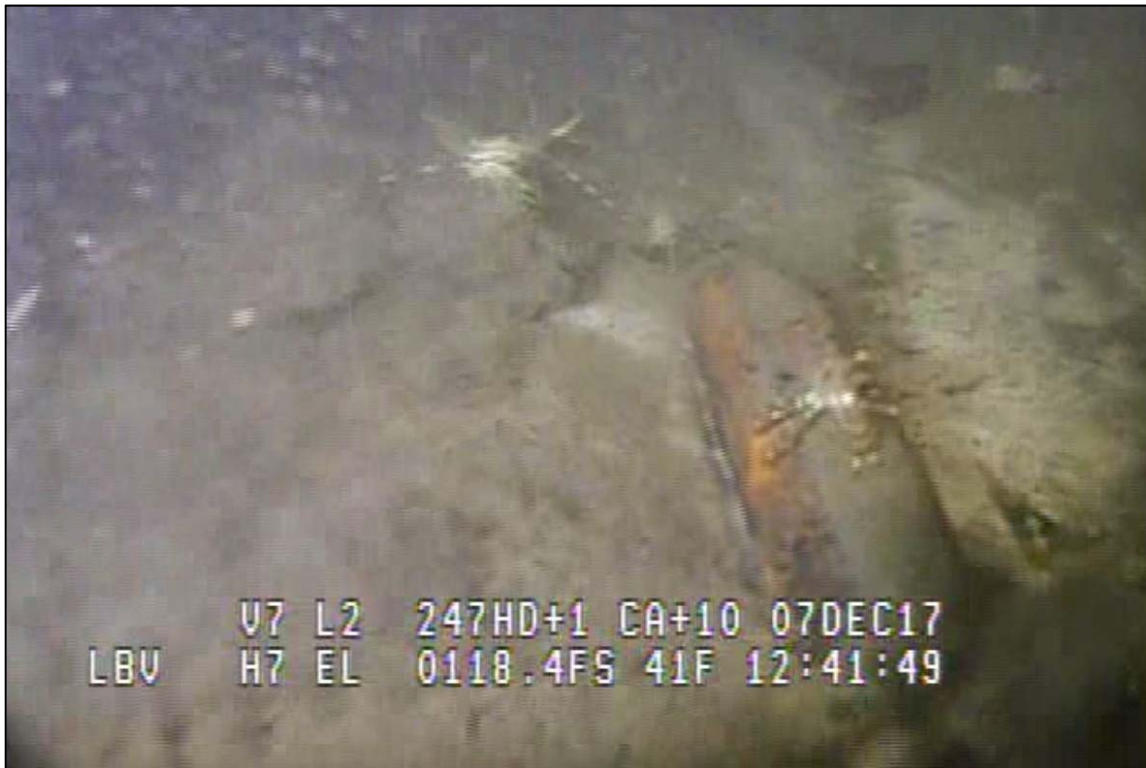
Photograph 71: View of Lower Anchor Chain Embedment in the Channel Bottom at Primary System Anchor 20, Looking Southwest.
