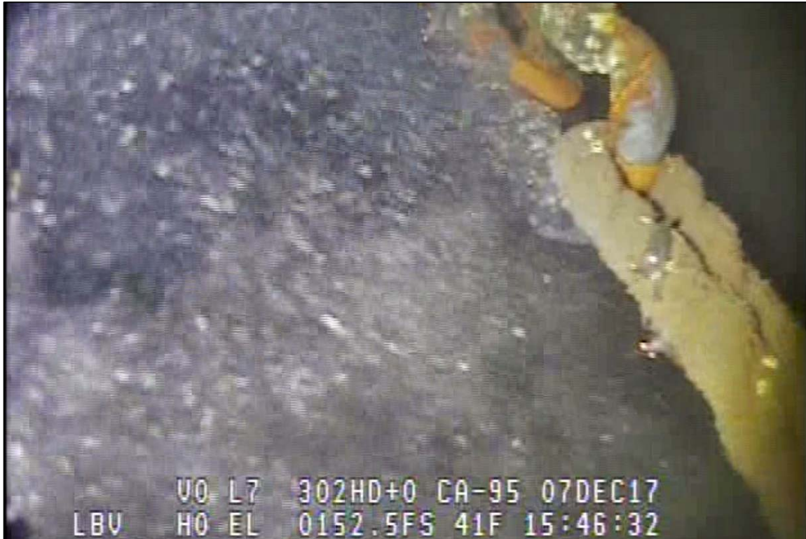
Photograph 55: View of Lower Anchor Chain to Rope Connection (Rope and Shackle) at Primary System Anchor Line 16, Looking West.
