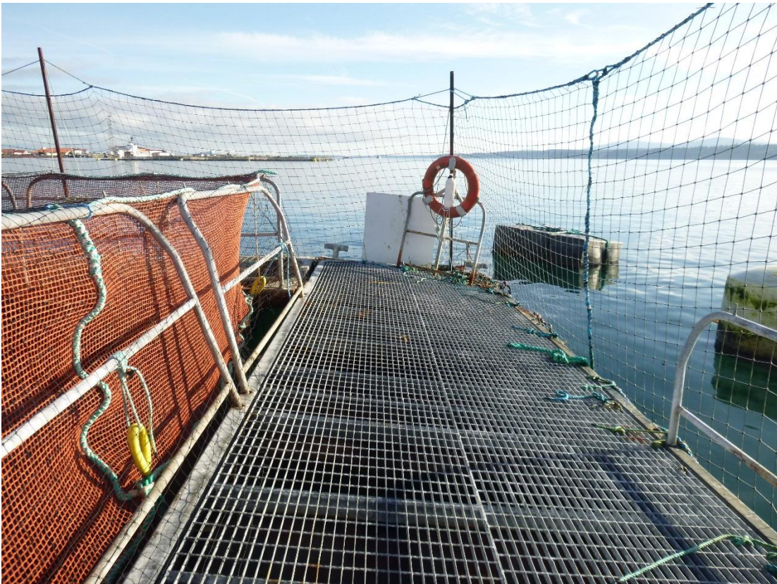
Figure C-31: Showing Sloped Docks Along South Edge of Pen 14 Looking East
