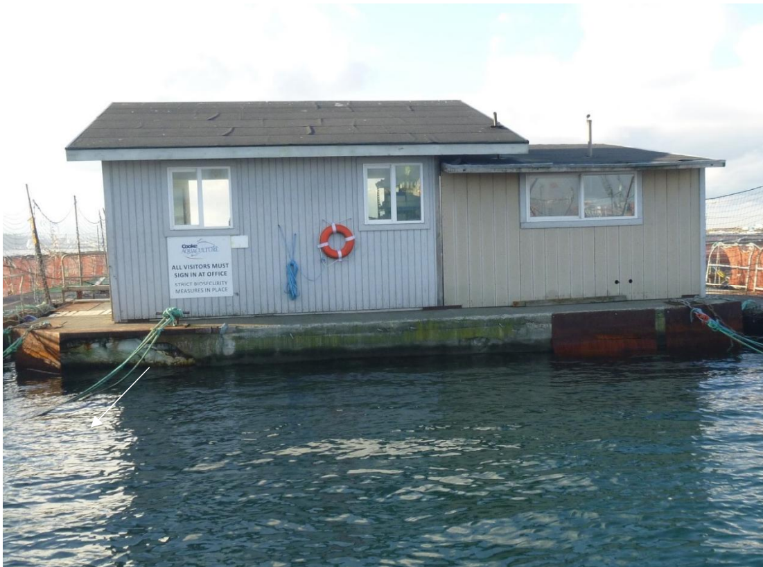
Figure C-84: East face of Office and Gen-set Barge – Looking West
