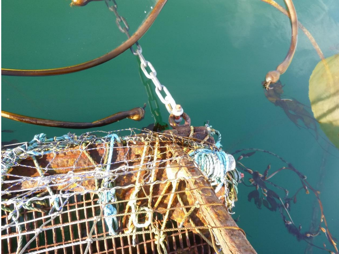
Figure C-68: Anchor 20 Right Padeye, Shackle and Chain
