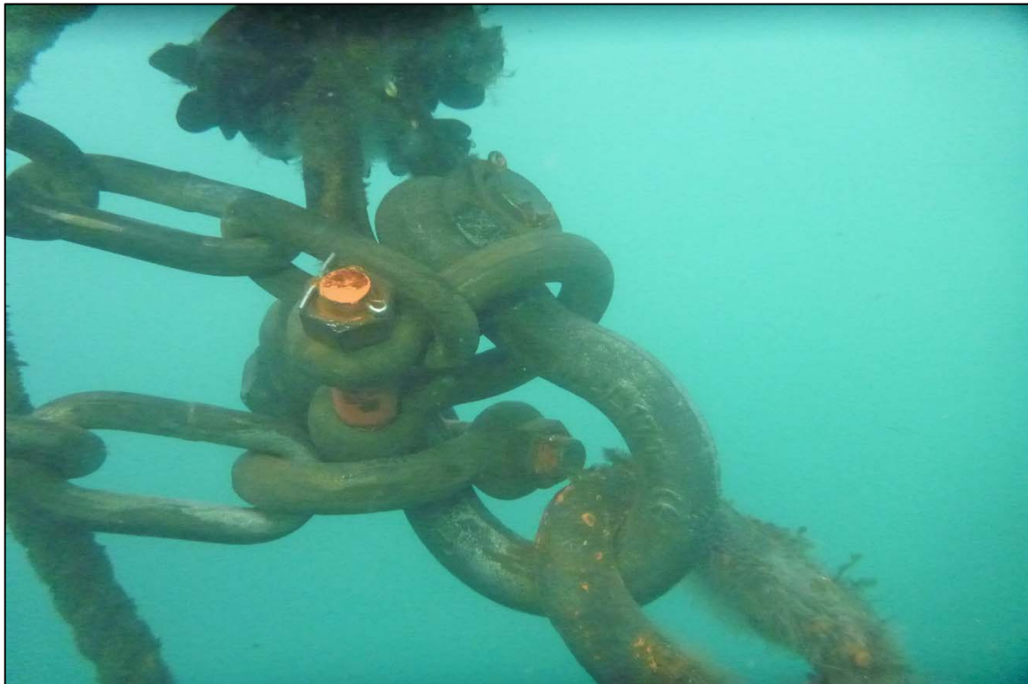
Photograph 28: View of Bridle Chain, Buoy, Anchor Chain Connection (Shackles and Chain) at Anchor 2, Looking South.
