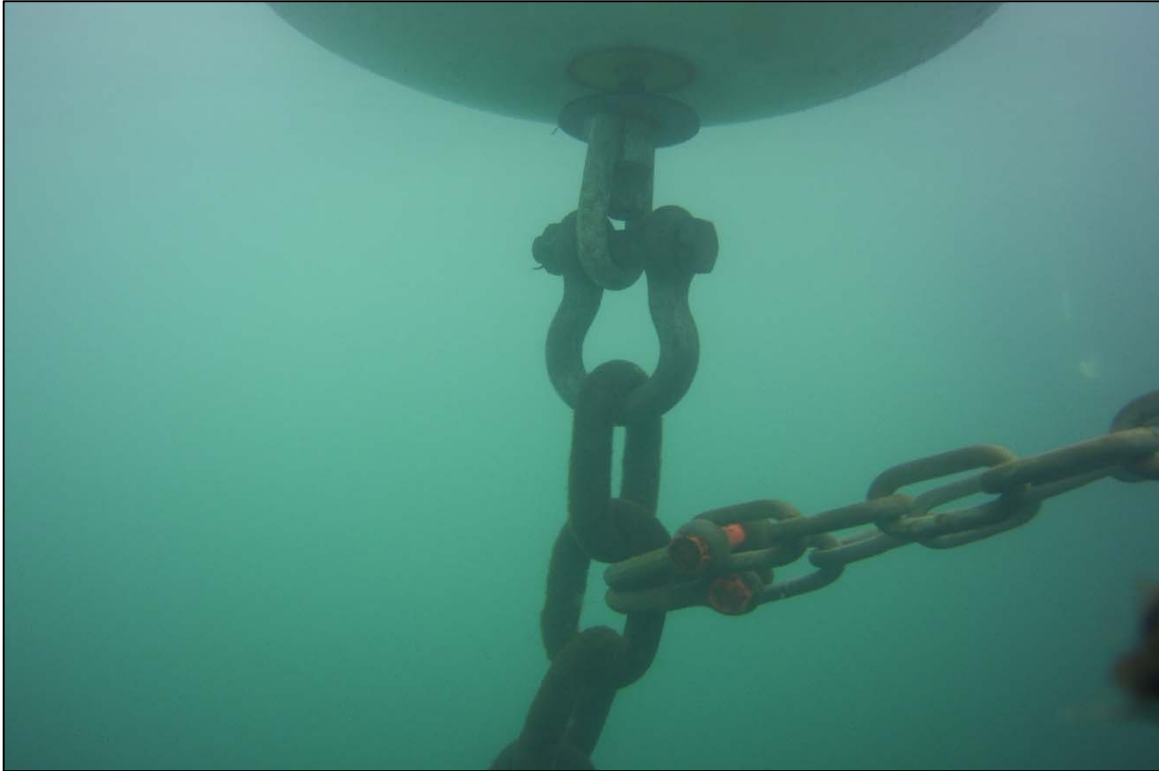
Photograph 15: View of the Typical Buoy, Anchor Chain, and Bridle Chain Connection, Anchor Line 20 Shown.
