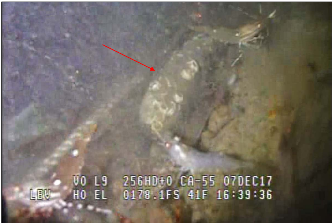
Photograph 52: View of Lower Anchor Chain Embedment in the Channel Bottom at Primary System Anchor Line 14, Looking West.
