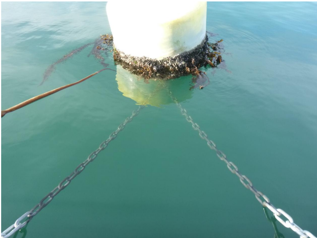
Figure C-45: Anchor 14 Bridle Chains
