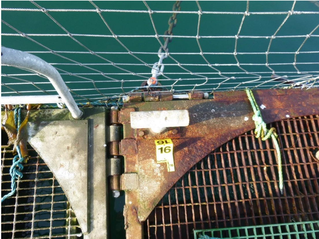
Figure C-50: Anchor 16 Left Shackle and Padeye
