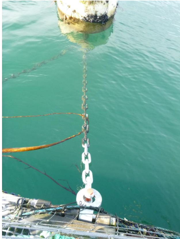
Figure C-40: Anchor 12 Right Bridle Connection
