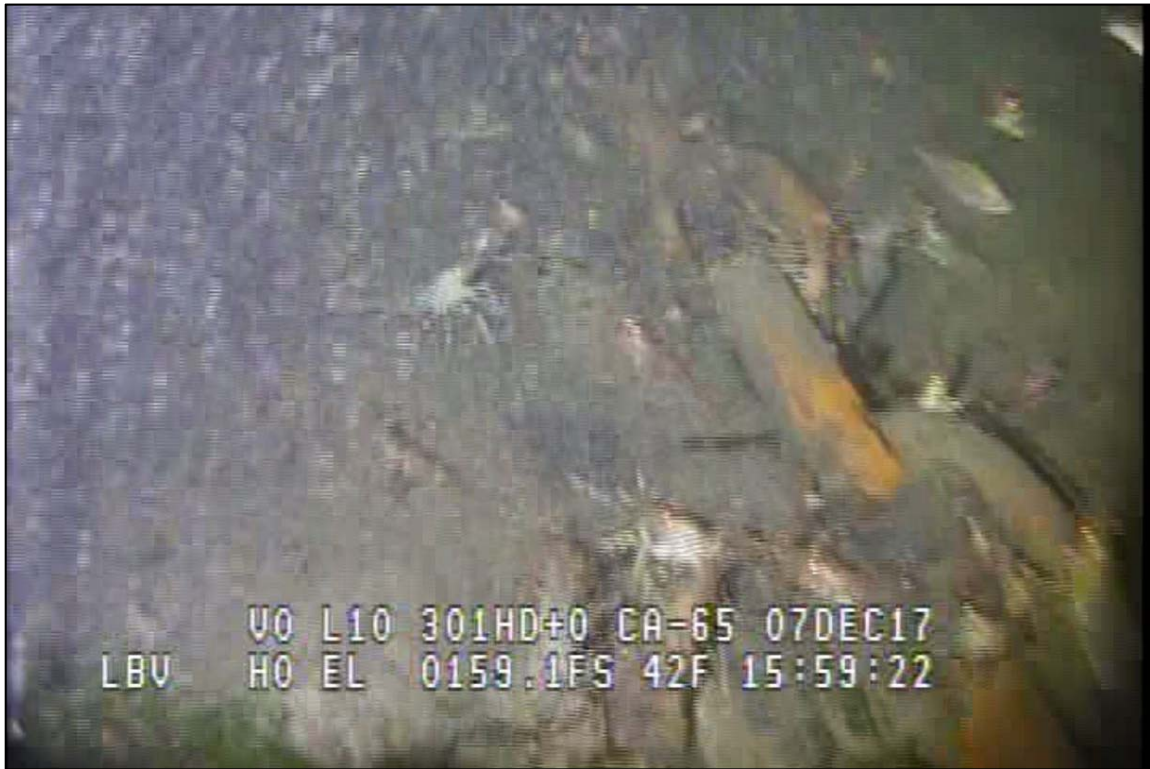
Photograph 59: View of Lower Anchor Chain Embedment in the Channel Bottom at Primary System Anchor Line 16, Looking West.
