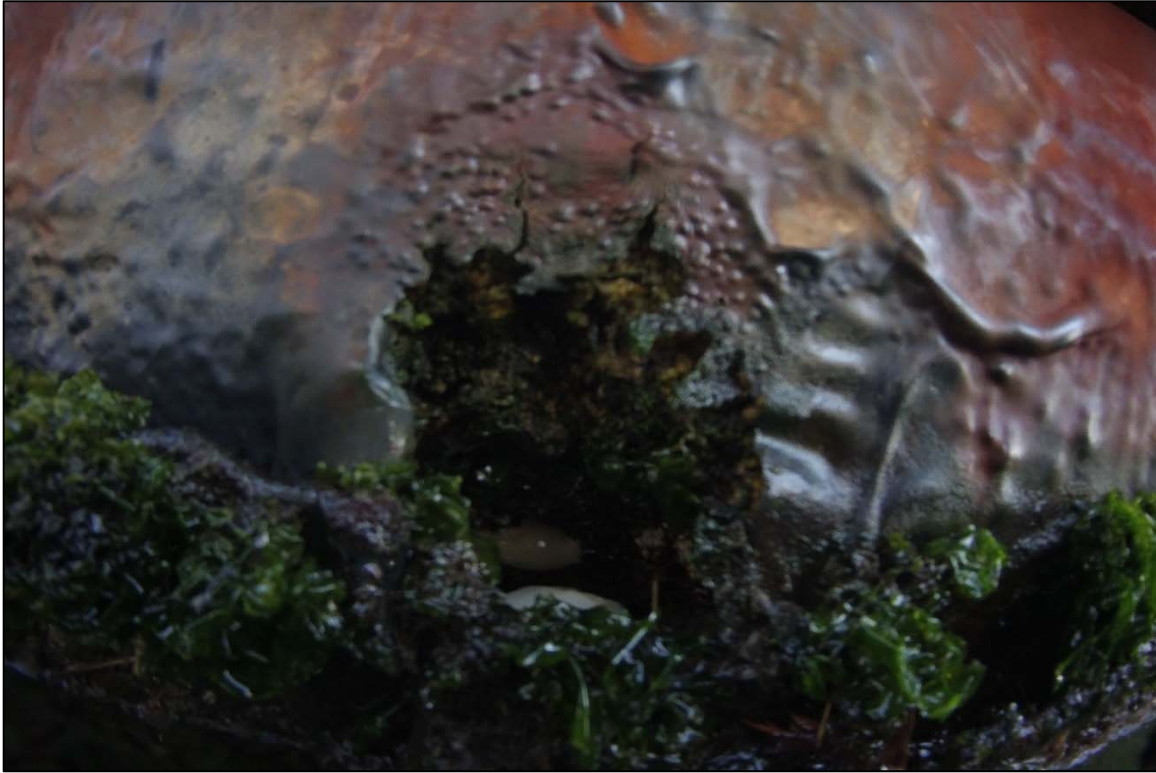
Photograph 17: View of the Heat Damage (Melted Plastic) Float 4 Shown, Looking North.
