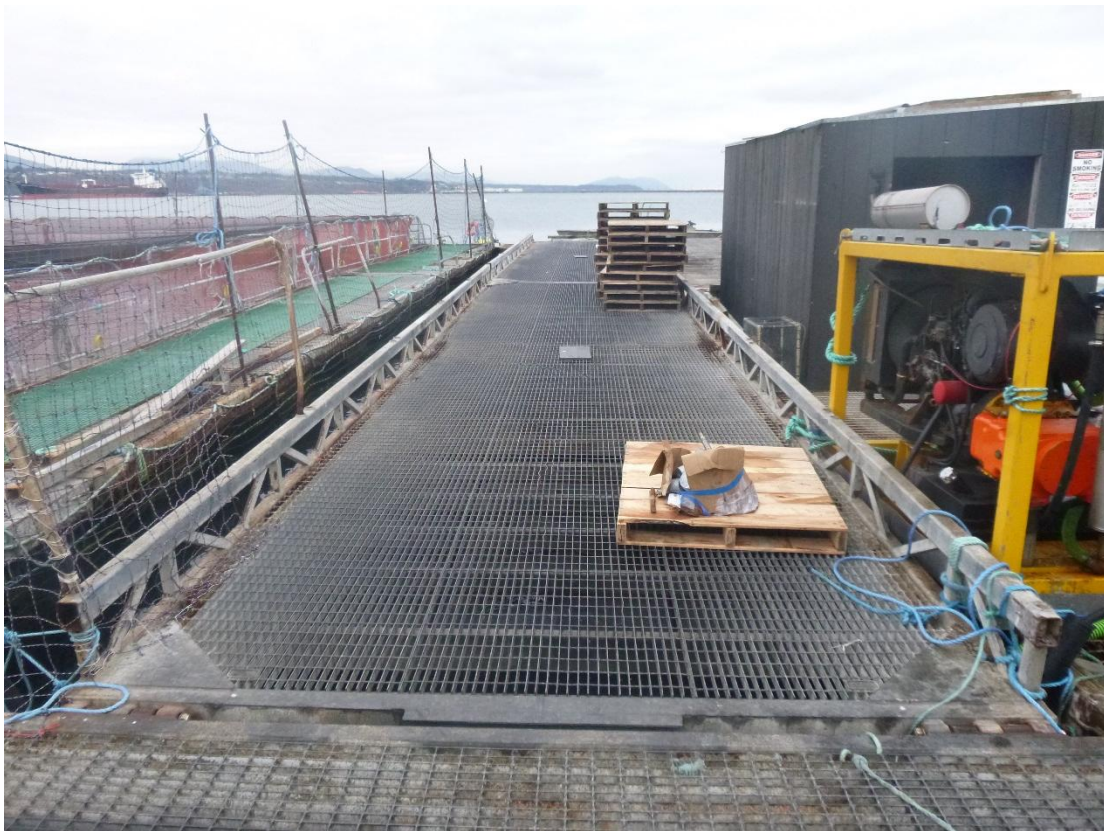
Figure C-80: Boarding Area Between 6 and 8 Pen Sections- South Dock looking west
