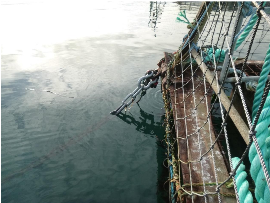
Figure C-13: Anchor 4 Right Bridle Chain, Shackle and Padeye (Looking South)
