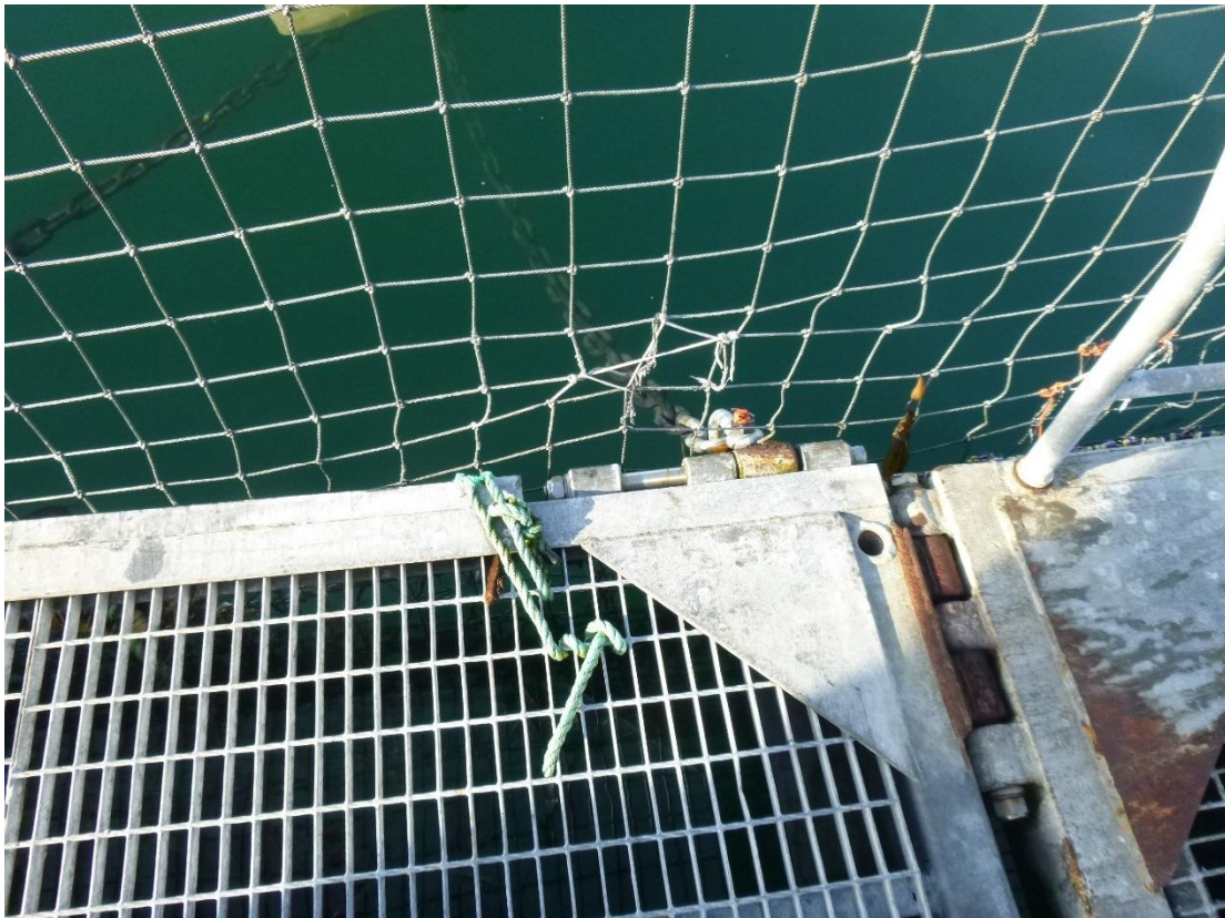
Figure C-61: Anchor 18 Right Padeye Shackle and Chain
