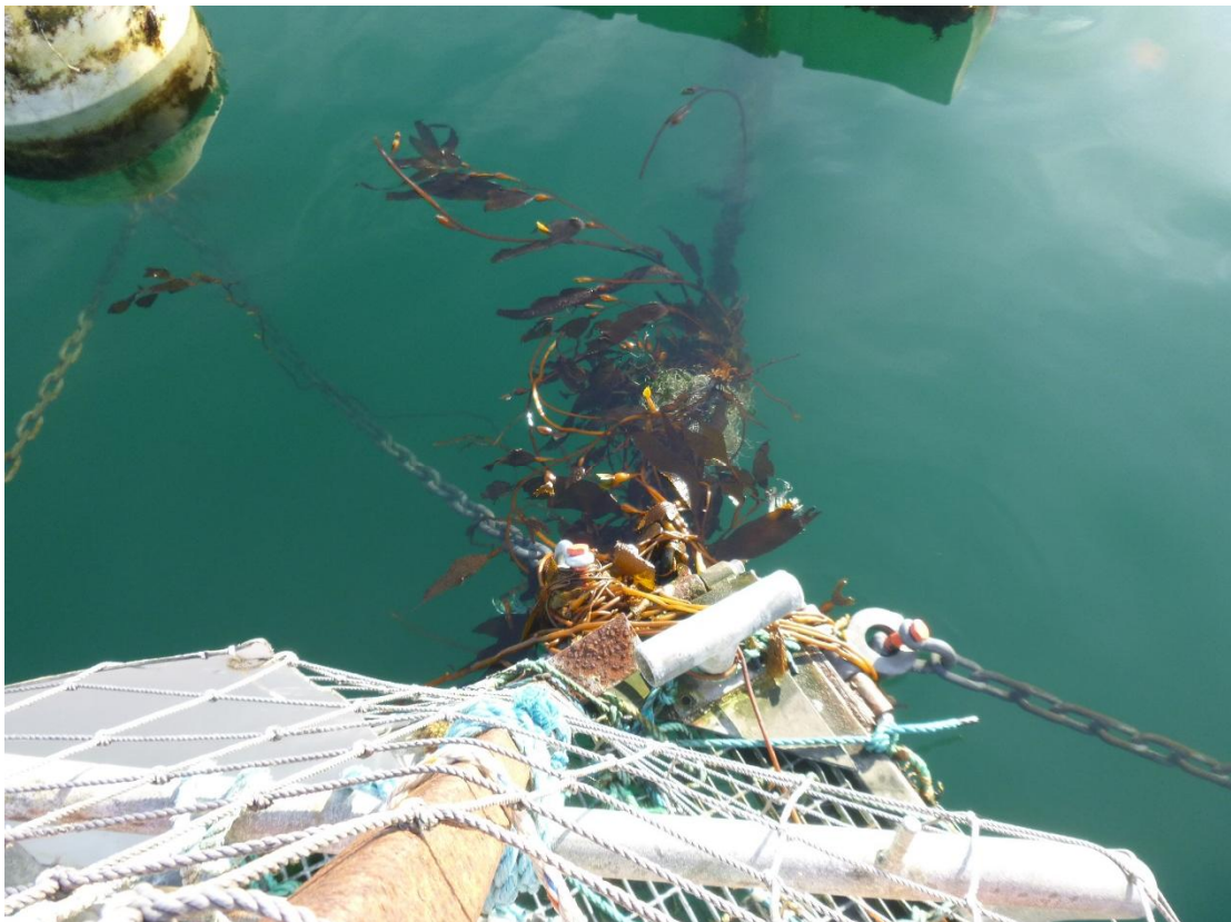
Figure C-29: South East Corner Showing Additional Anchor Pontoon Float and Padeye
