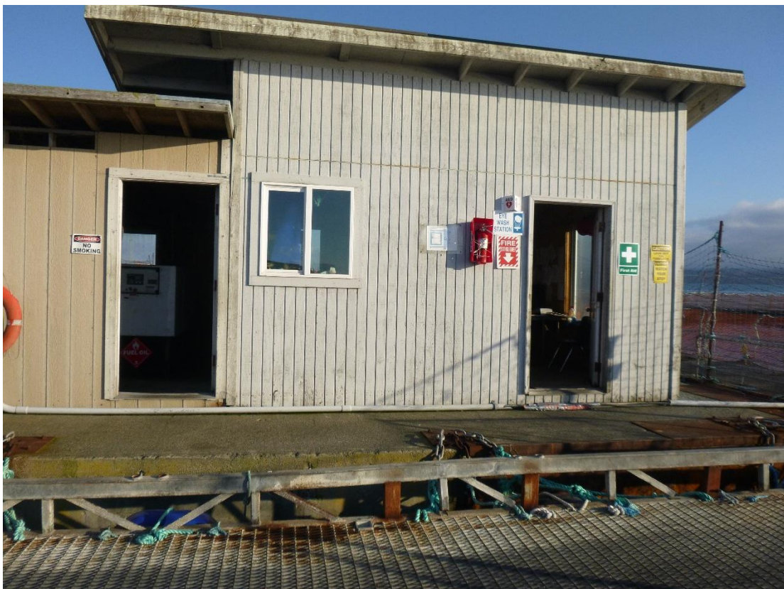
Figure C-89: West Face of Office and Gen-set Barge – Looking East
