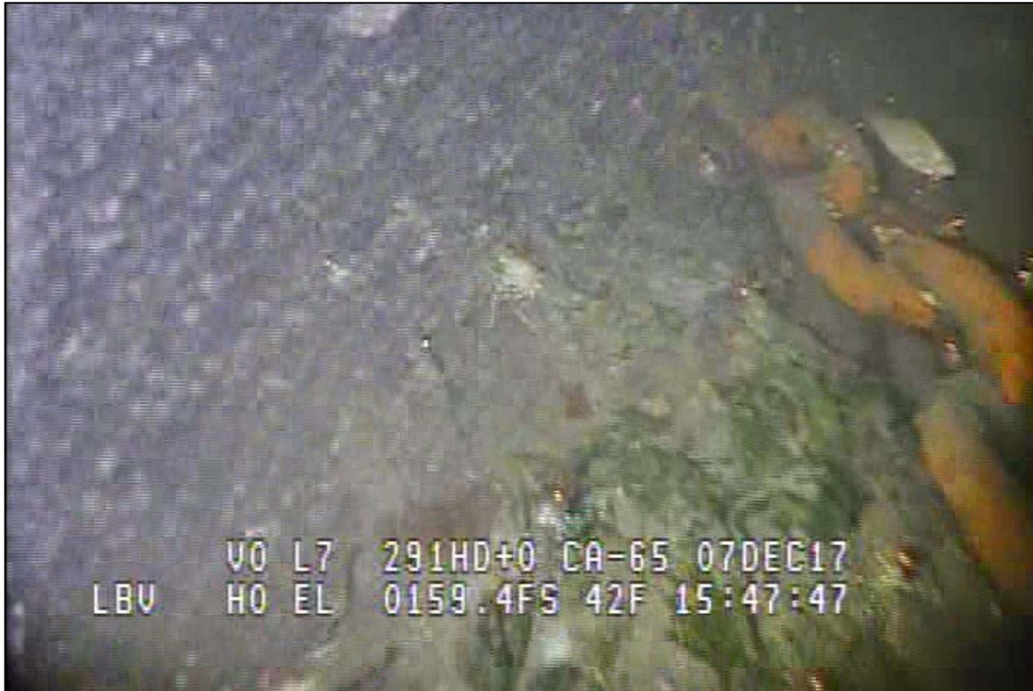
Photograph 57: View of Lower Anchor Chain on Channel Bottom at Primary System Anchor Line 16, Looking West.
