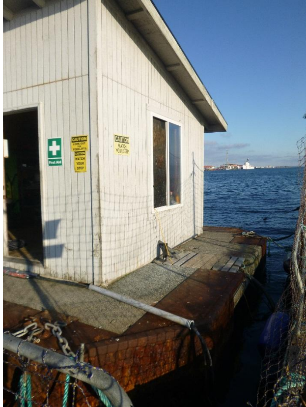
Figure C-90: Southwest Corner of Office and Gen-set Barge – Looking East
