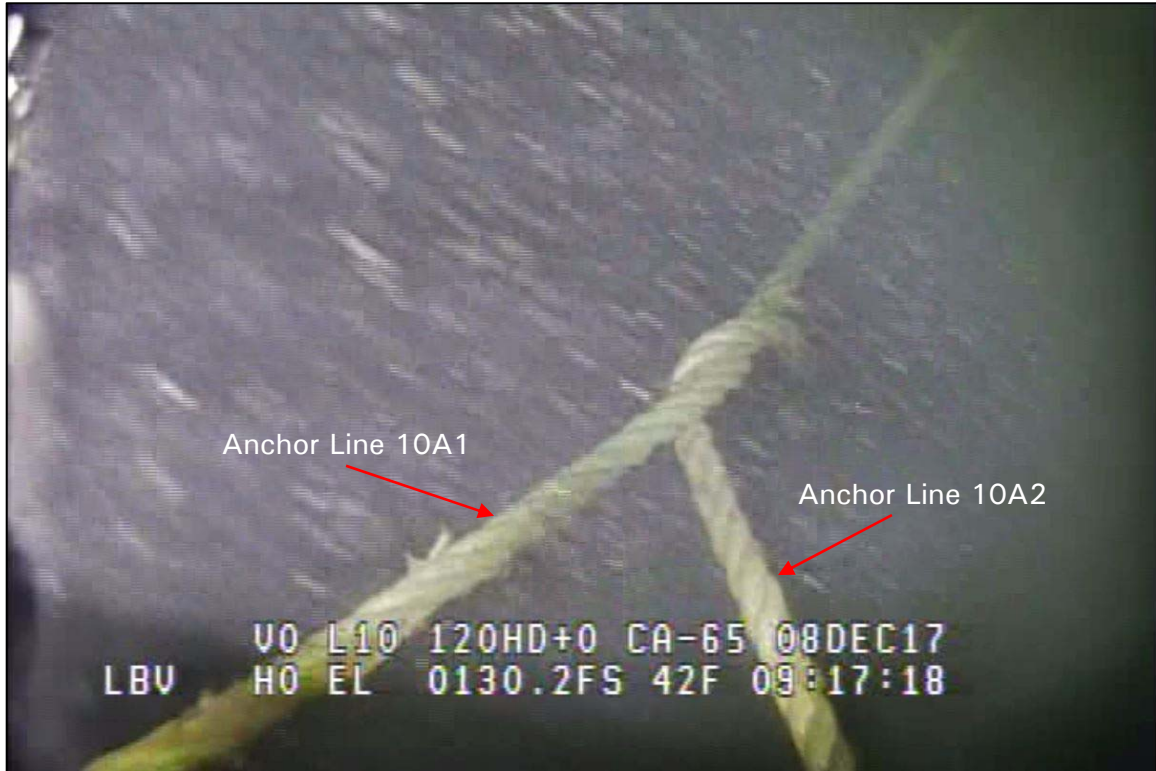
Photograph 43: View of Primary System Anchor Line 10A2 wrapped around Primary System Anchor Line 10A1, Looking South.
