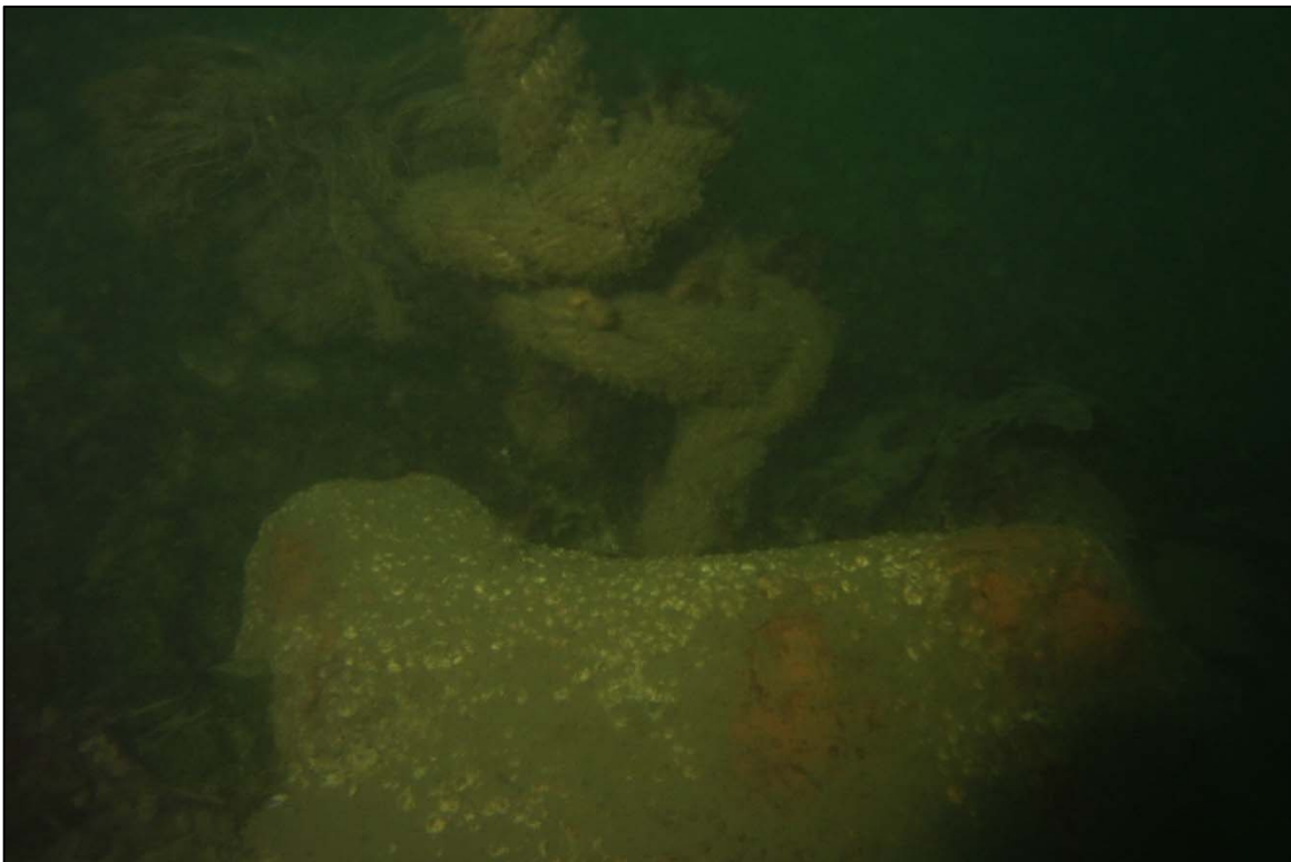
Photograph 38: View of Anchor Head at Anchor 22 (Typical Observed by Diver), Looking South.
