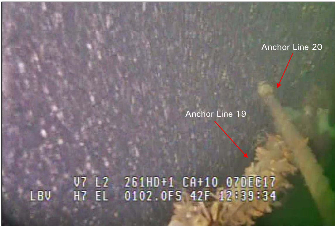
Photograph 69: View of Anchor 20 Crossing Above Anchor Line 19, Looking Southwest.
