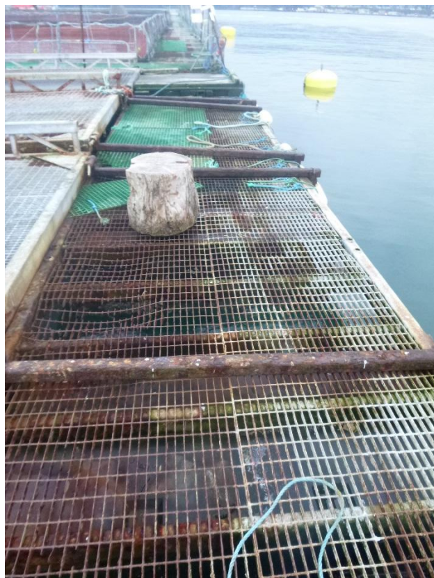
Figure C-53: Floating Dock Boarding Area Looking South
