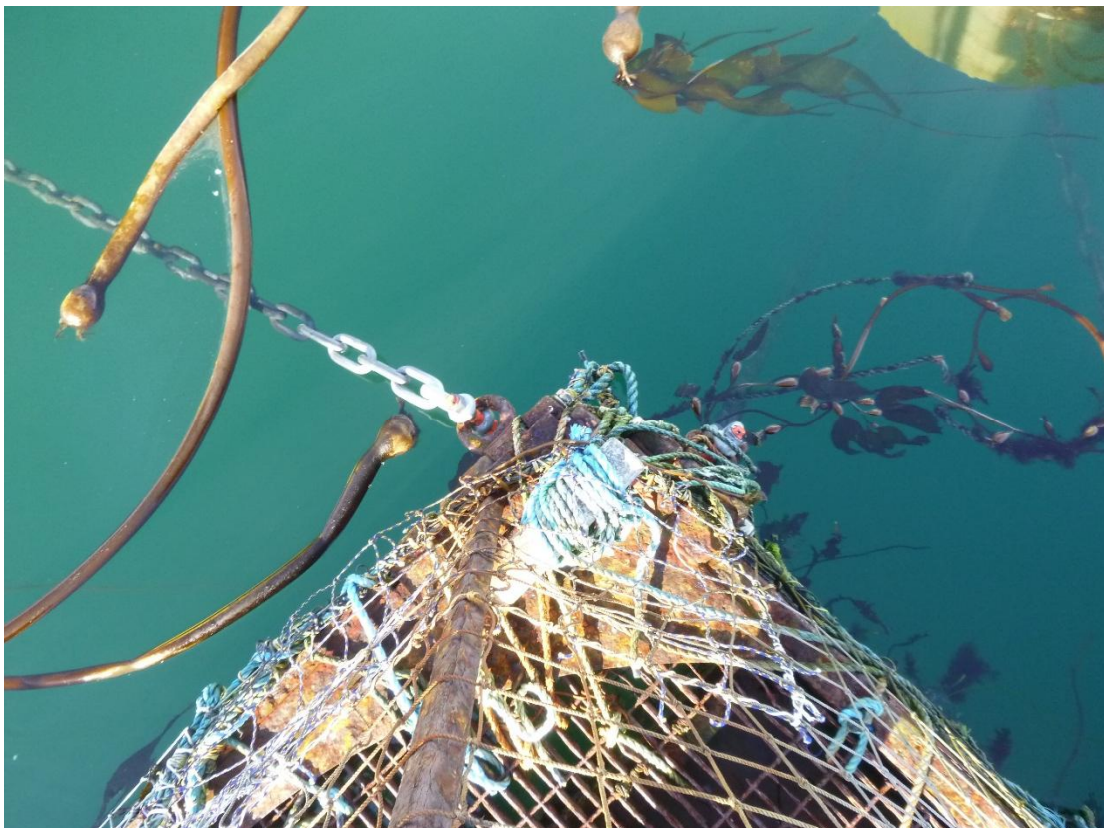
Figure C-71: Anchor 21 Left Padeye, Shackle and Chain (Single Hinge Setup)
