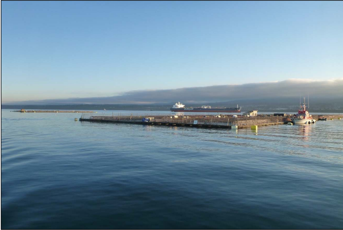
Photograph 5: Overall View of the Primary Fish Net Pens System, Looking Southeast.
