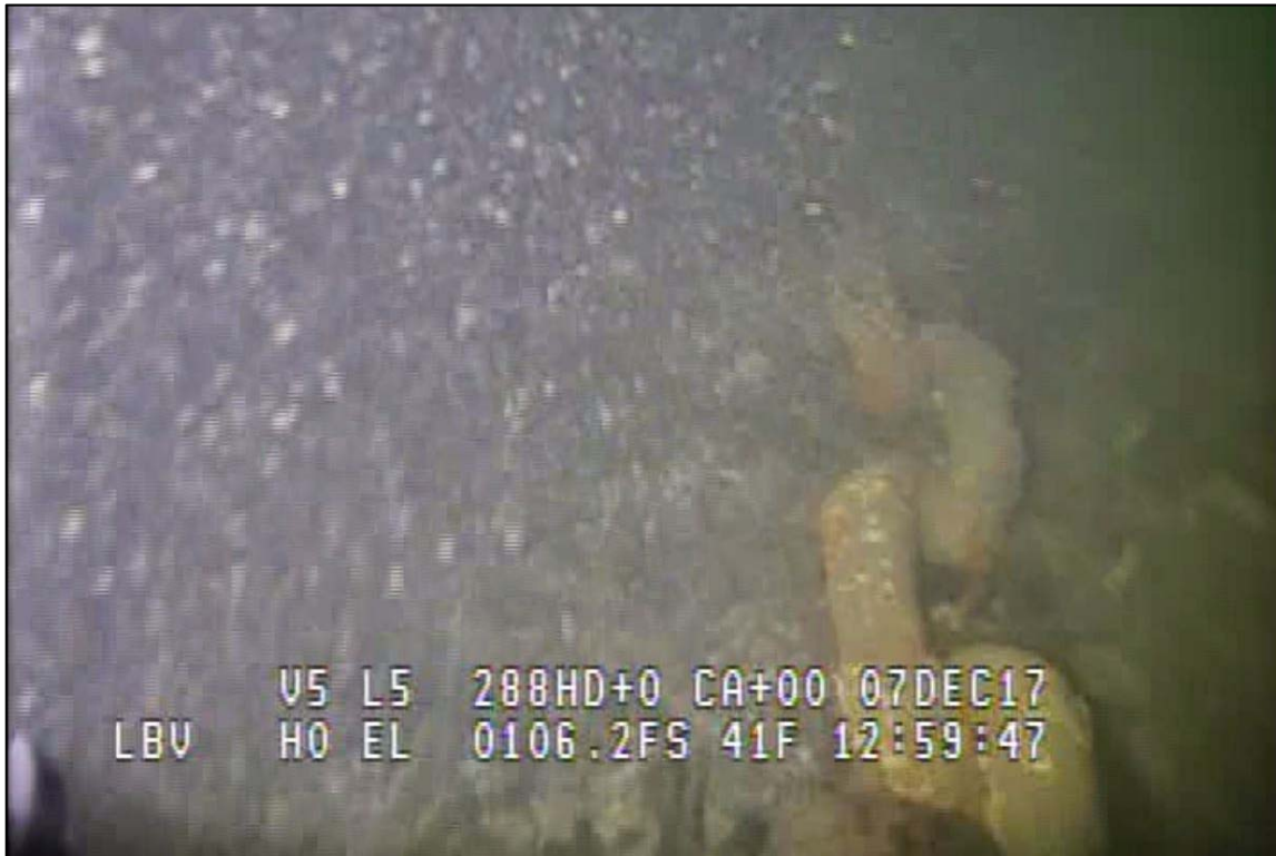
Photograph 65: View of Lower Anchor Chain Embedment in the Channel Bottom at Primary System Anchor Line 19, Looking West.
