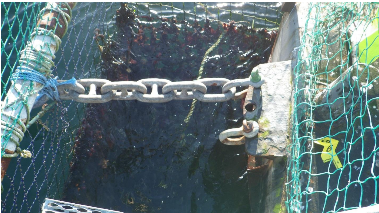
Figure C-15: Anchor #5, East Side of the North Net Pen. Note chain tied to predator support pipe.
