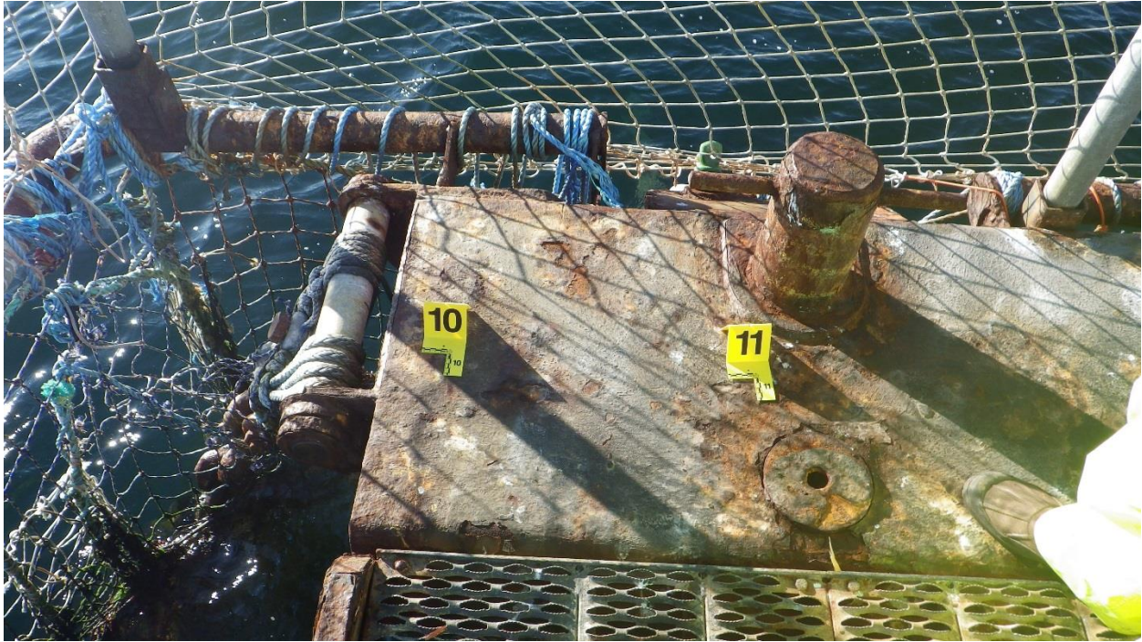
Figure D-25: Anchors #10 and #11, SW Corner of the South Net Pen.
