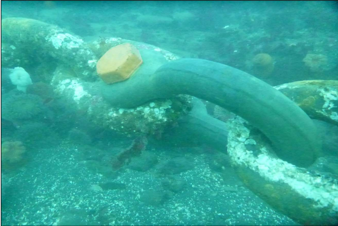
Photograph 43: View of Shackle Connection in the Anchor Chain at Orchard Rocks North Anchor Line 14, Looking Northeast.
