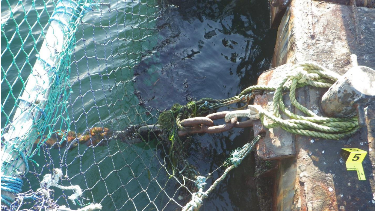
Figure C-14: Anchor #5, East Side of the North Net Pen
