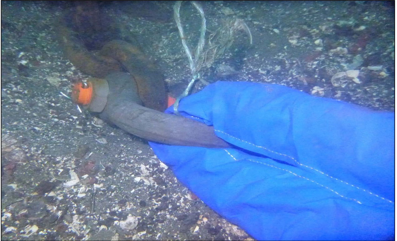
Photograph 97: View of Lower Anchor Chain to Anchor Rope Connection (Shackle and PVC) at Orchard Rocks South Anchor Line 16, Looking North.
