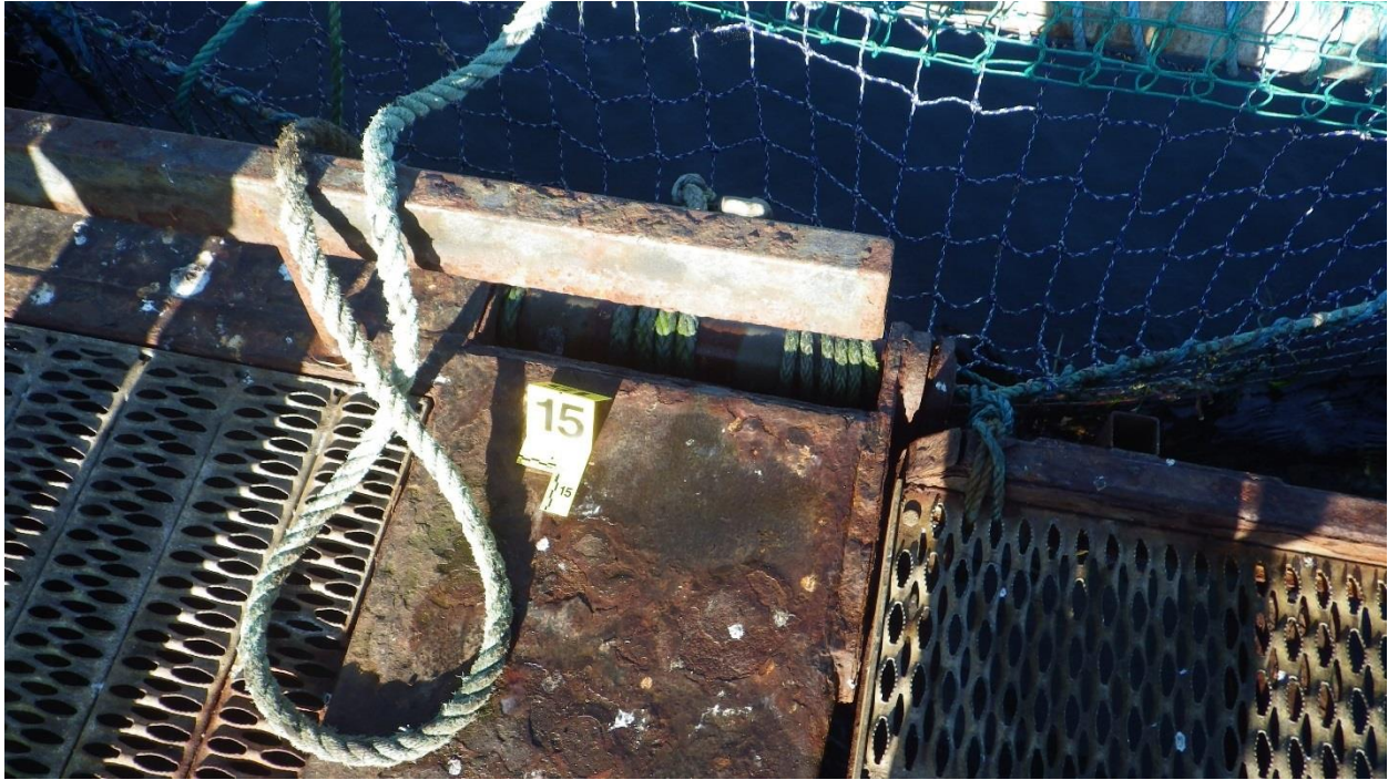
Figure C-32: Anchor #15, North Side of the North Net Pen
