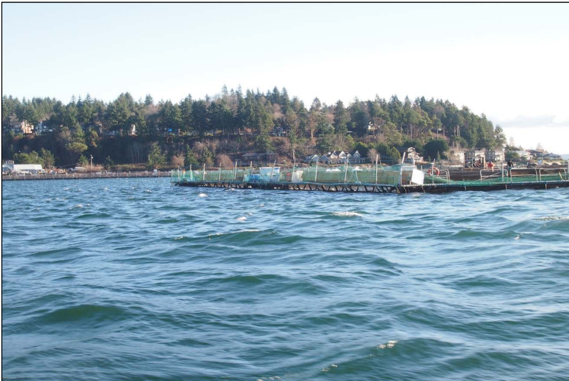
Photograph 2: Overall View of the Orchard Rocks North Fish Net Pens System, Looking East.
