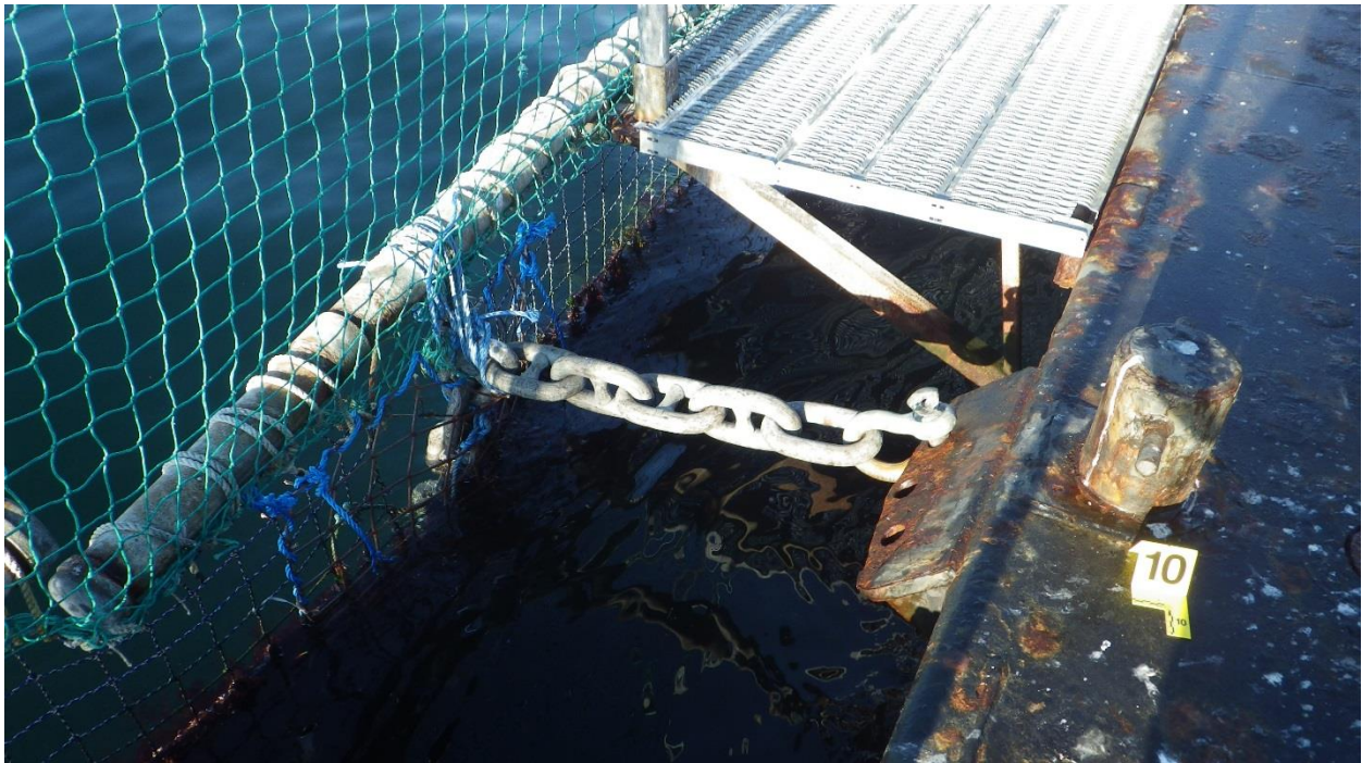
Figure C-23: Anchor #10, West Side of the North Net Pen.
