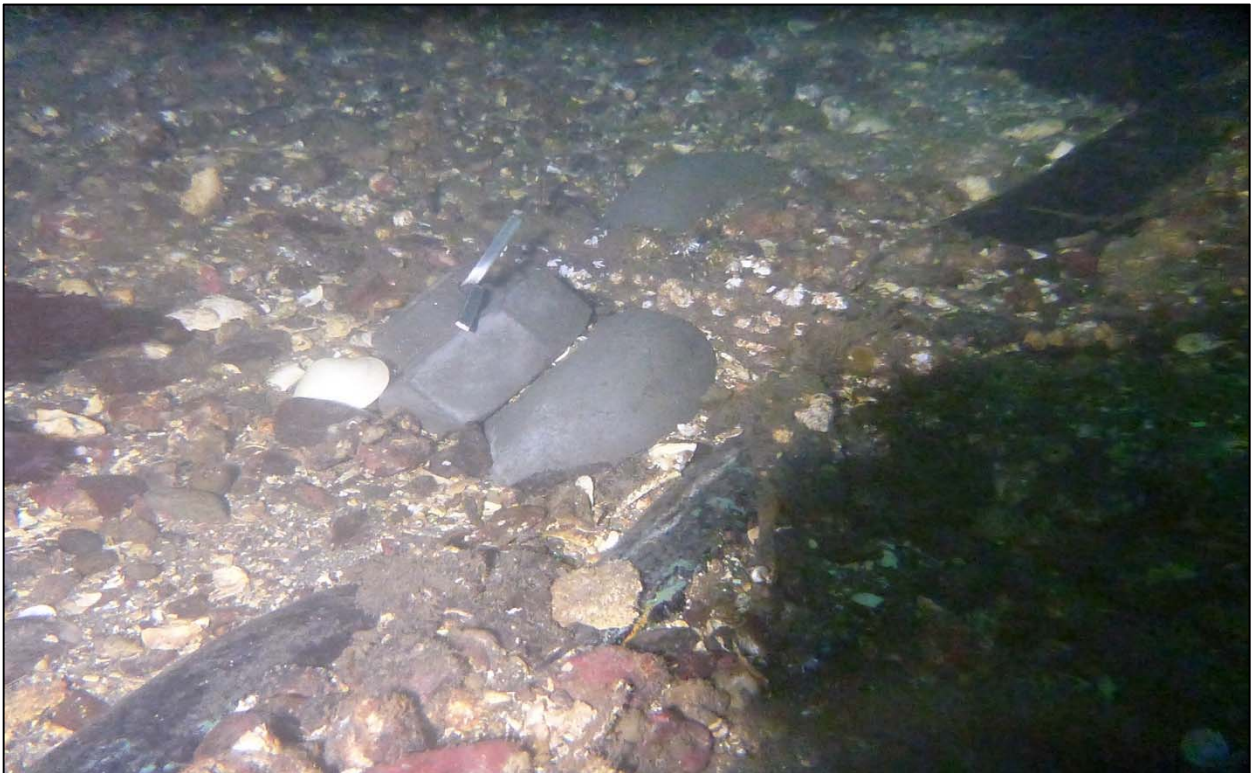
Photograph 92: View of Lower Anchor Chain to Anchor Connection (Shackle) at Orchard Rocks South Anchor Line 14, Looking West.
