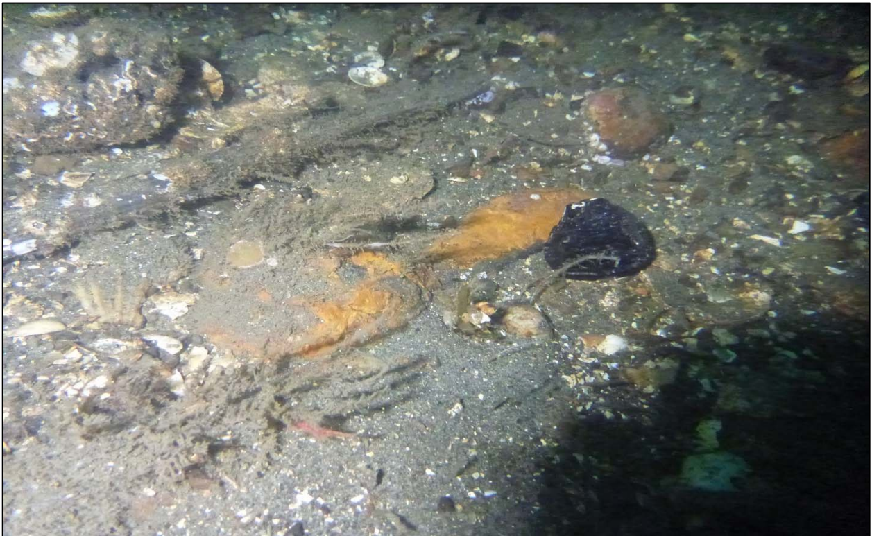
Photograph 94: View of Lower Anchor Chain 90% Buried at Orchard Rocks South Anchor Line 15, Looking South.
