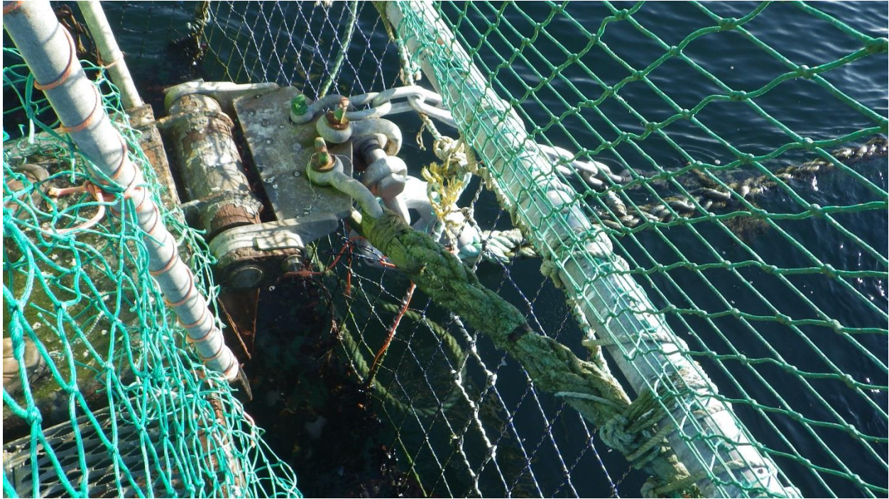
Figure C-40: North East Hinge – Connection of North and South Net Pens. Hinge with moderate corrosion.
