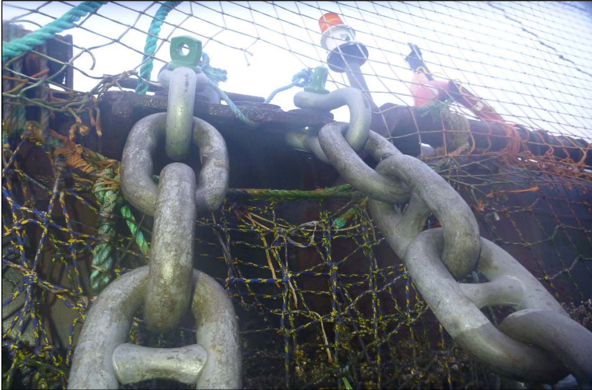
Photograph 69: View of Upper Anchor Chain to Float Connection for Anchor 6 and 6A at Orchard Rocks South Anchor Line 4, Looking West.
