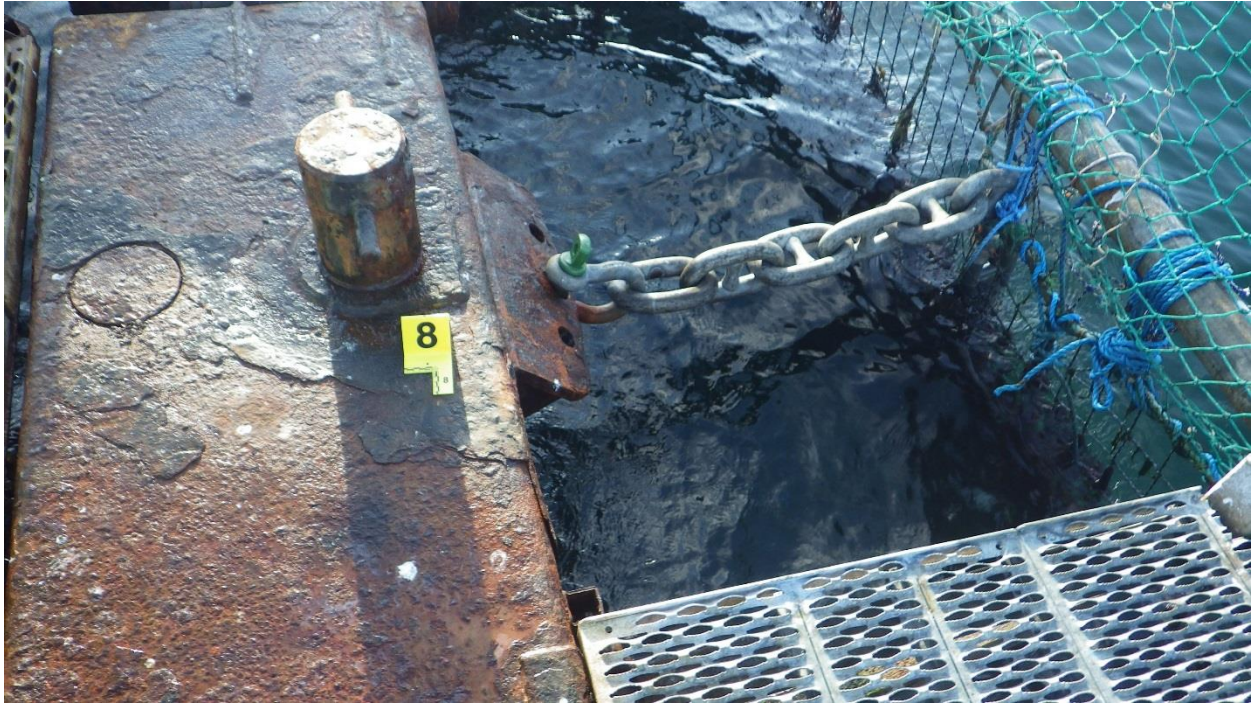
Figure C-18: Anchor #8, West Side of the North Net Pen. New shackle and chain. Chain tied to predator support pipe.
