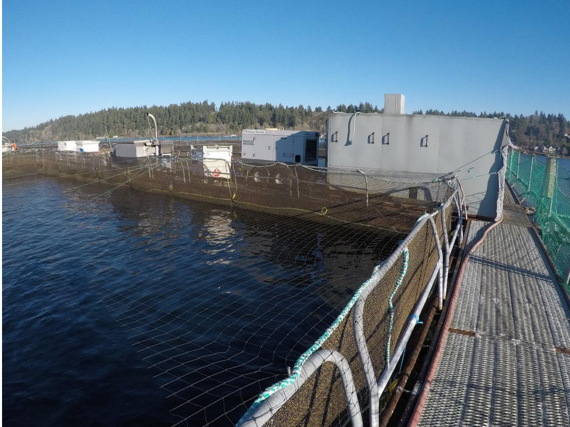
Figure C-4: Center Bridge and staff shed
