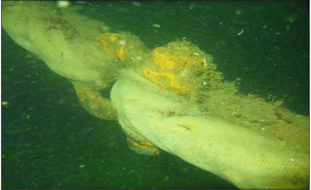
Photograph 95: View of Lower Anchor Rope to Anchor Rope Connection (Shackle) at Orchard Rocks South Anchor Line 15, Looking South.
