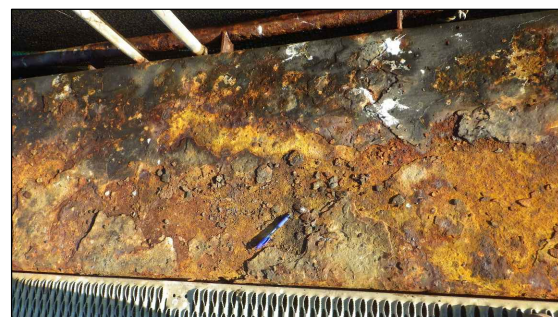
PHOTO 7 MAJOR CORROSION ON WALKWAY
