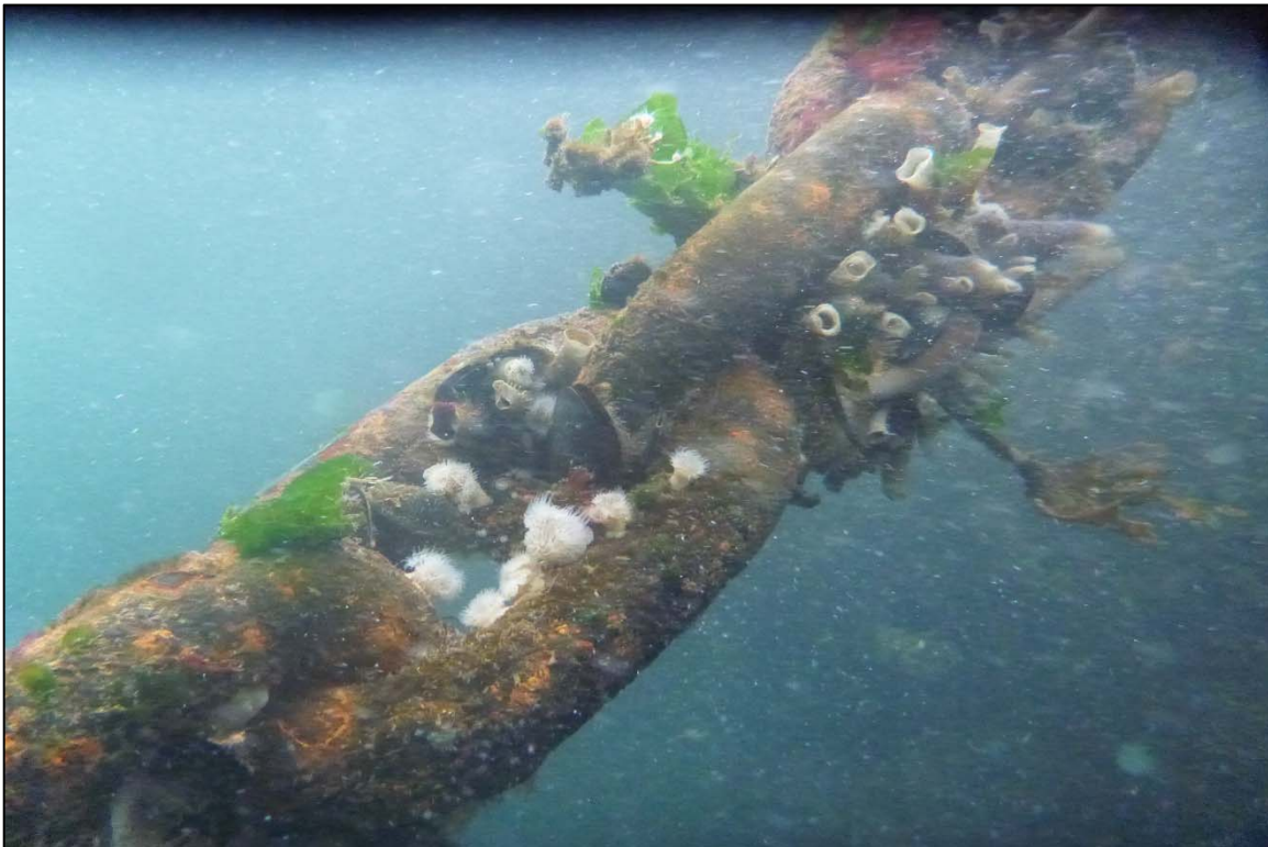
Photograph 56: View of Upper Chain Condition at Orchard Rocks South Anchor Line 2, Looking East.
