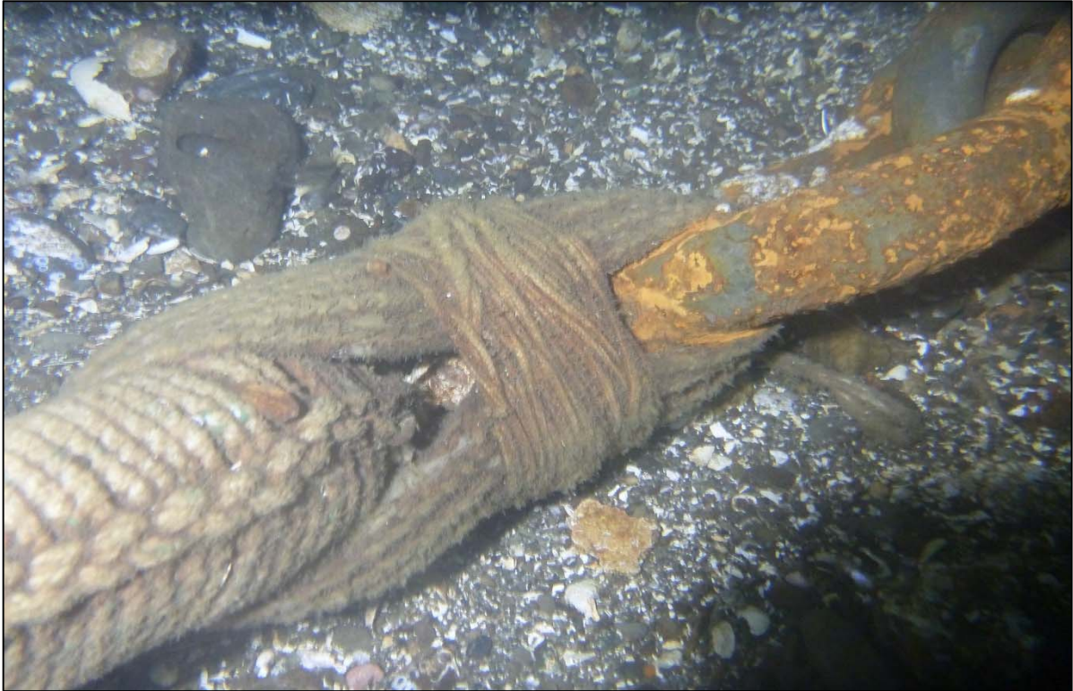
Photograph 77: View of Lower Anchor Chain to Anchor Rope Connection with Lashing at Orchard Rocks South Anchor Line 7, Looking South.
