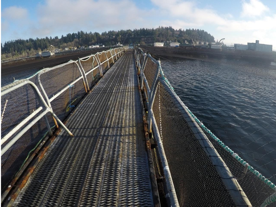
Figure D-47: Grating Walkway between net pens.
