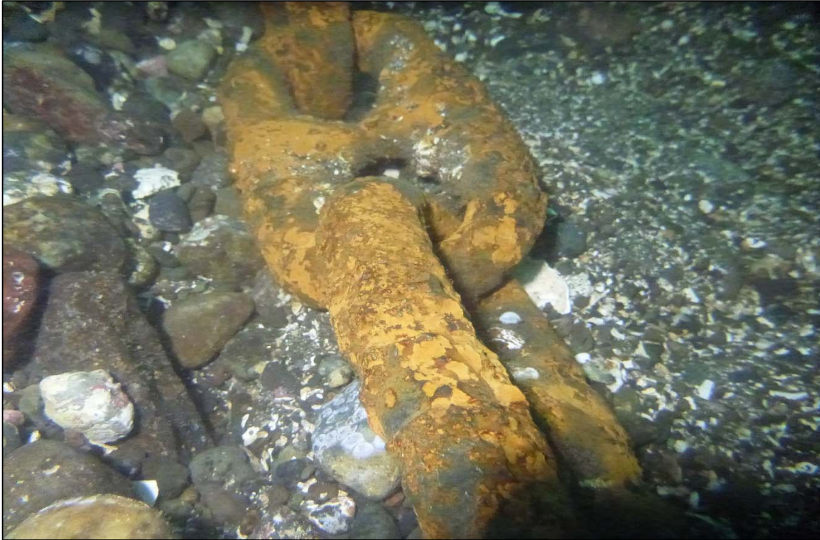
Photograph 67: View of Lower Anchor Chain Moderate Corrosion at Orchard Rocks South Anchor Line 5, Looking East.
