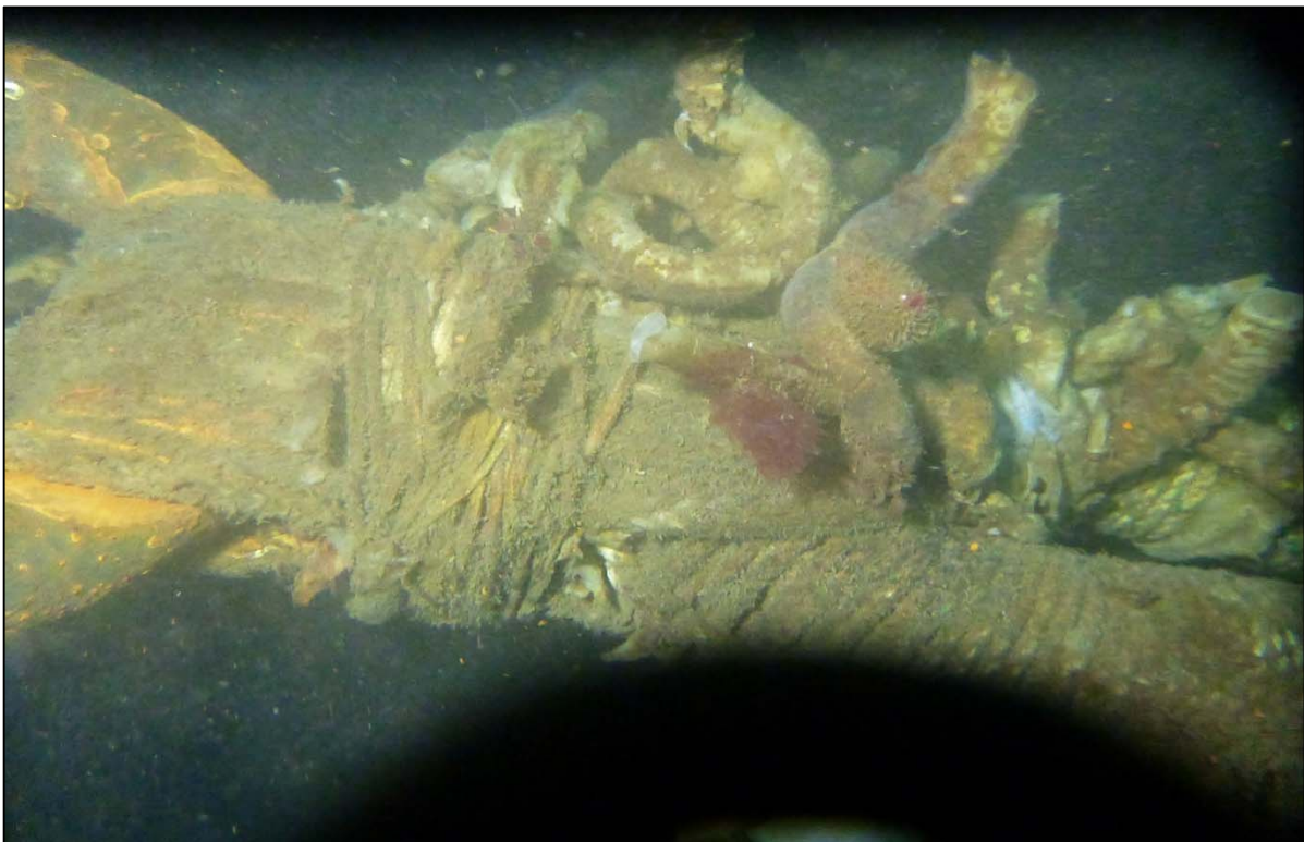
Photograph 78: View of Lower Anchor Chain to Anchor Rope Connection (Lashing) at Orchard Rocks South Anchor Line 8, Looking South.
