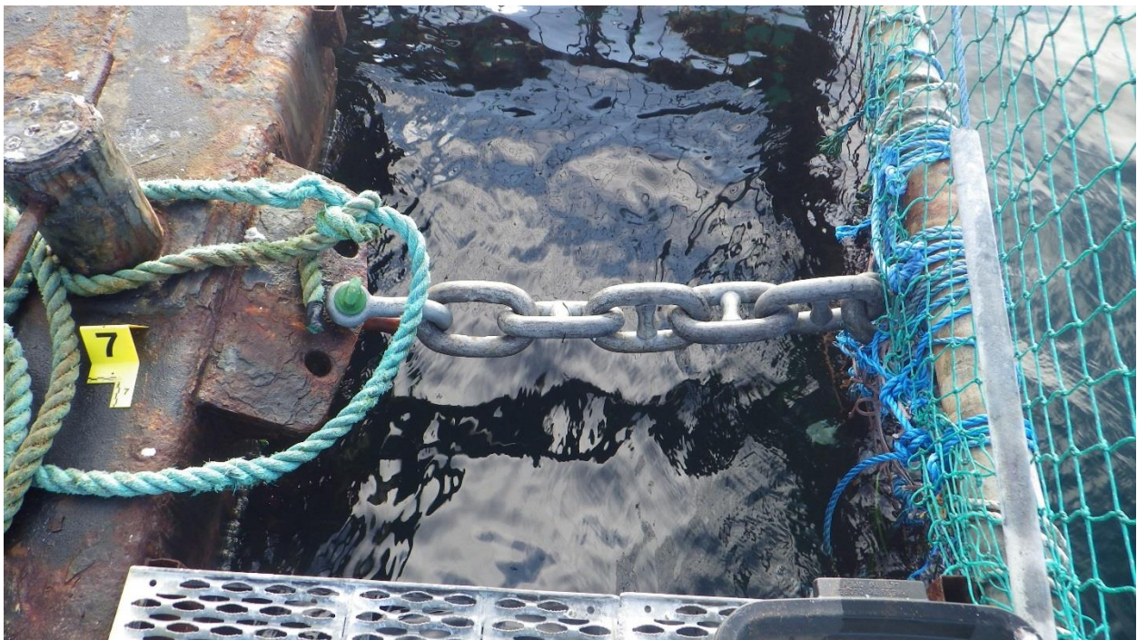
Figure C-17: Anchor #7, SW Corner of the North Net Pen. New shackle and chain. Chain tied to predator support pipe.
