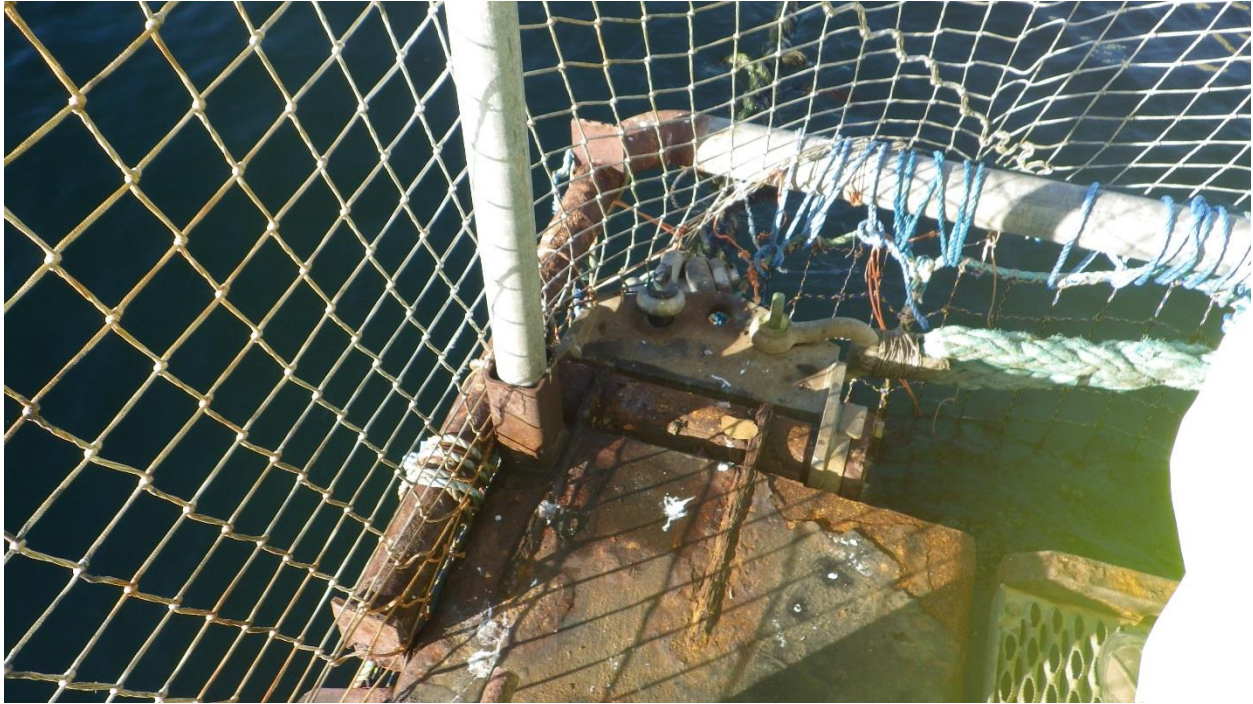
Figure D-43: South West Hinge connected to North pen.
