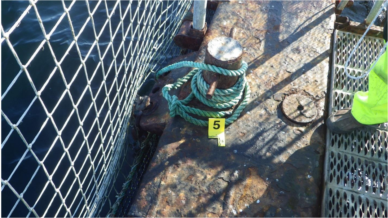
Figure D-13: Anchor #5, East Side of the South Net Pen
