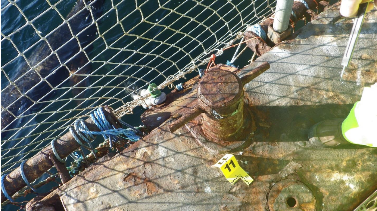
Figure D-27: Anchor #11, SW Corner of the South Net Pen. New shackle and chain.
