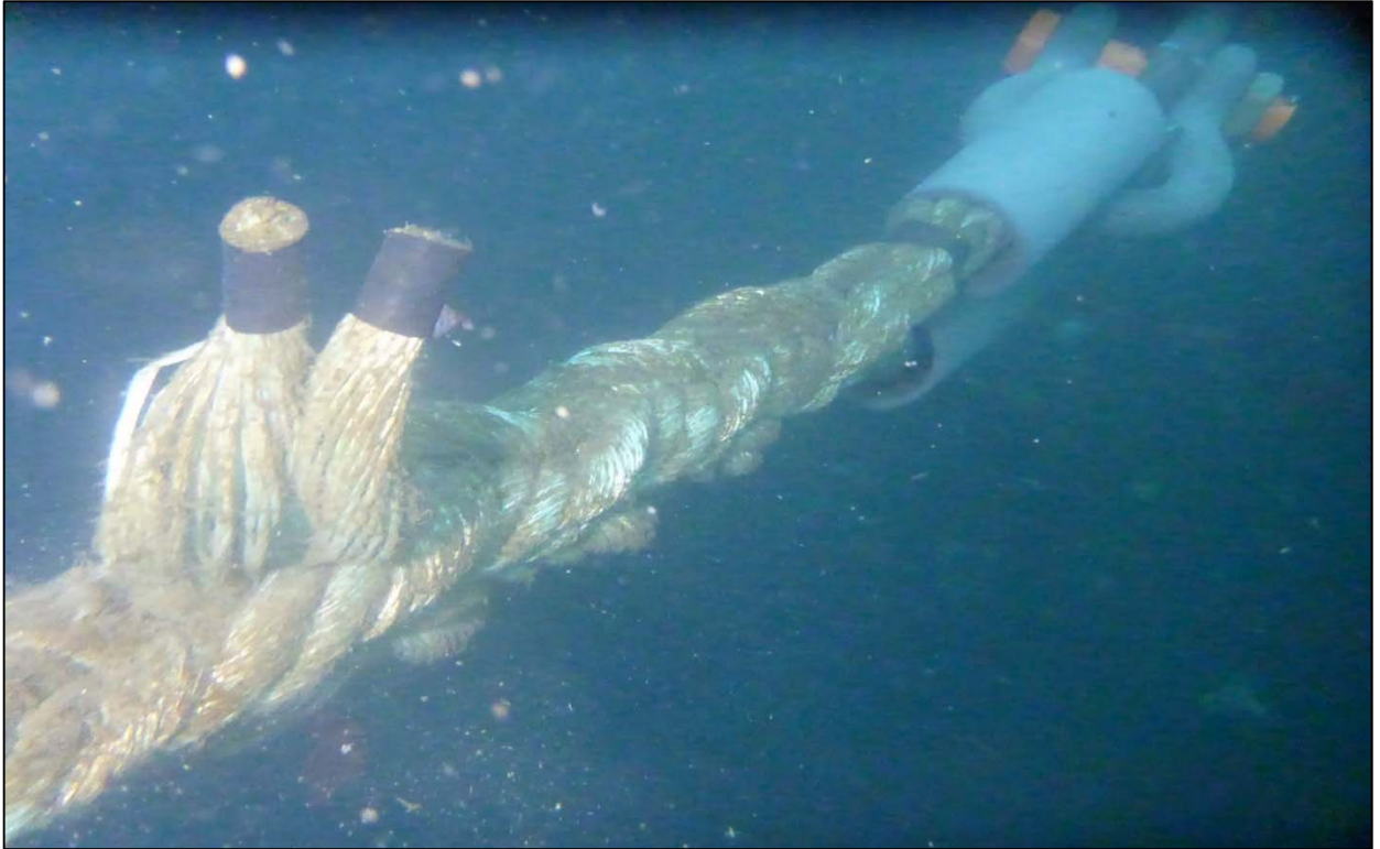
Photograph 91: View of Lower Anchor Chain to Anchor Rope Connection (Shackle and Thimble) at Orchard Rocks South Anchor Line 14, Looking West.
