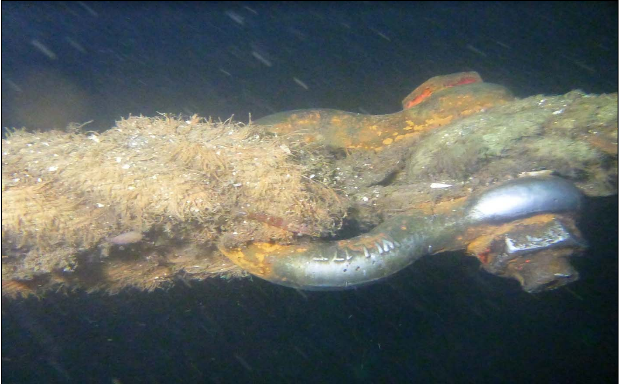
Photograph 89: View of Lower Anchor Rope to Anchor Rope Connection (Shackle) at Orchard Rocks South Anchor Line 13, Looking South.
