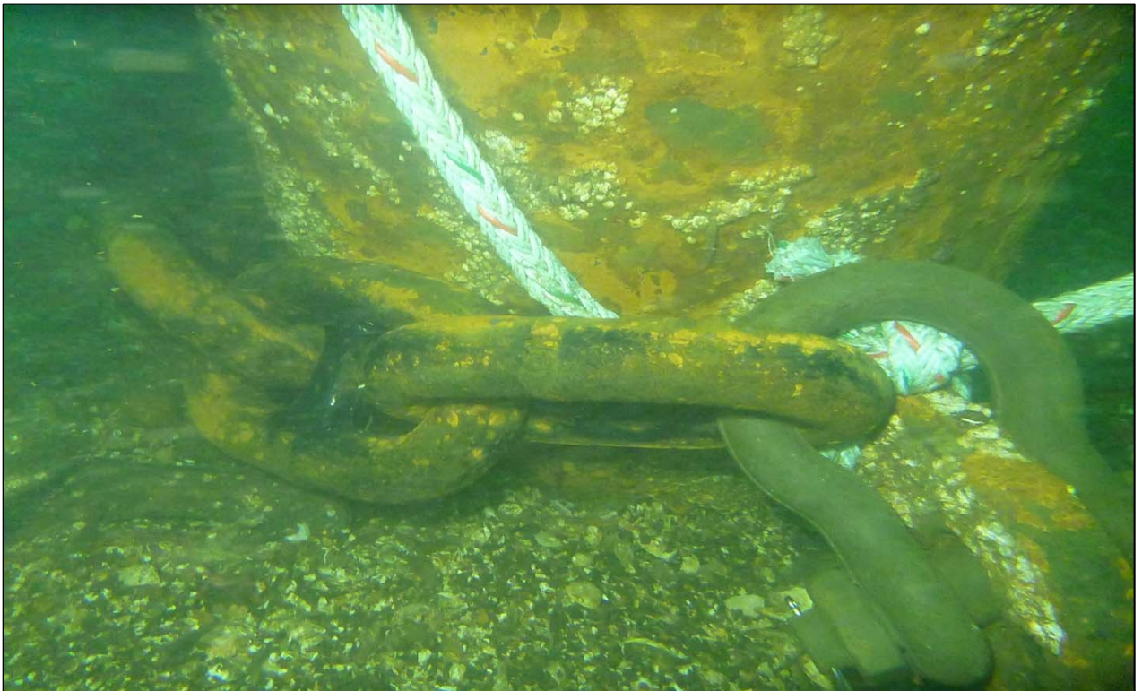
Photograph 98: View of Lower Anchor Rope to Pipe Anchor Connection (Shackle) at Orchard Rocks South Anchor Line 16, Looking South.
