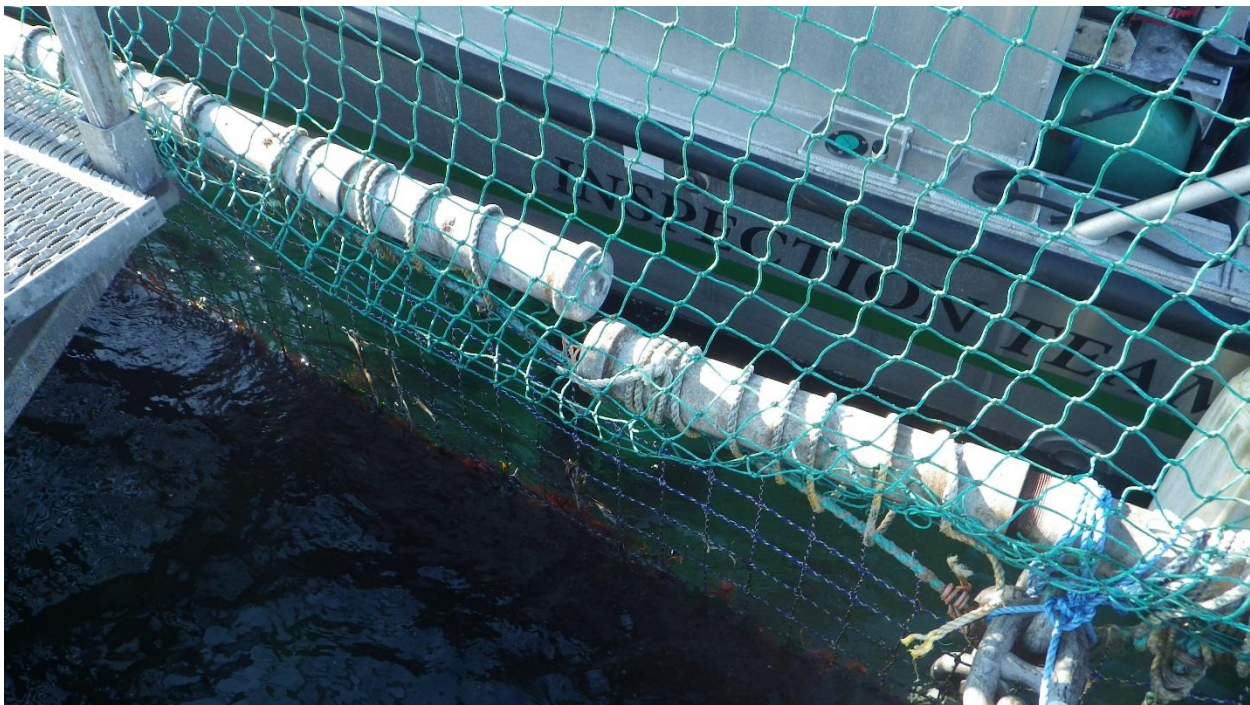
Figure C-55: Near Anchor 10, Discontinuous Predator Net Railing – Bent due chain connection load.
