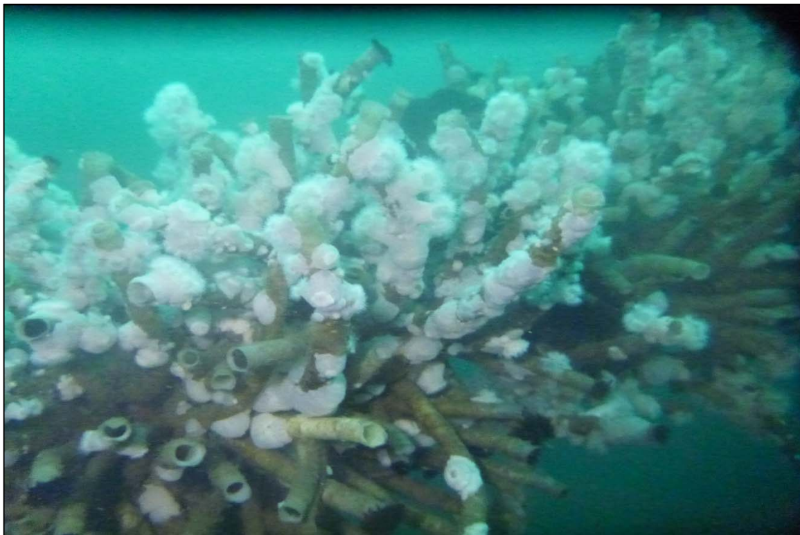
Photograph 26: View of Rope Condition with Heavy Marine Growth at Orchard Rocks North Anchor Line 4, Looking Northeast.
