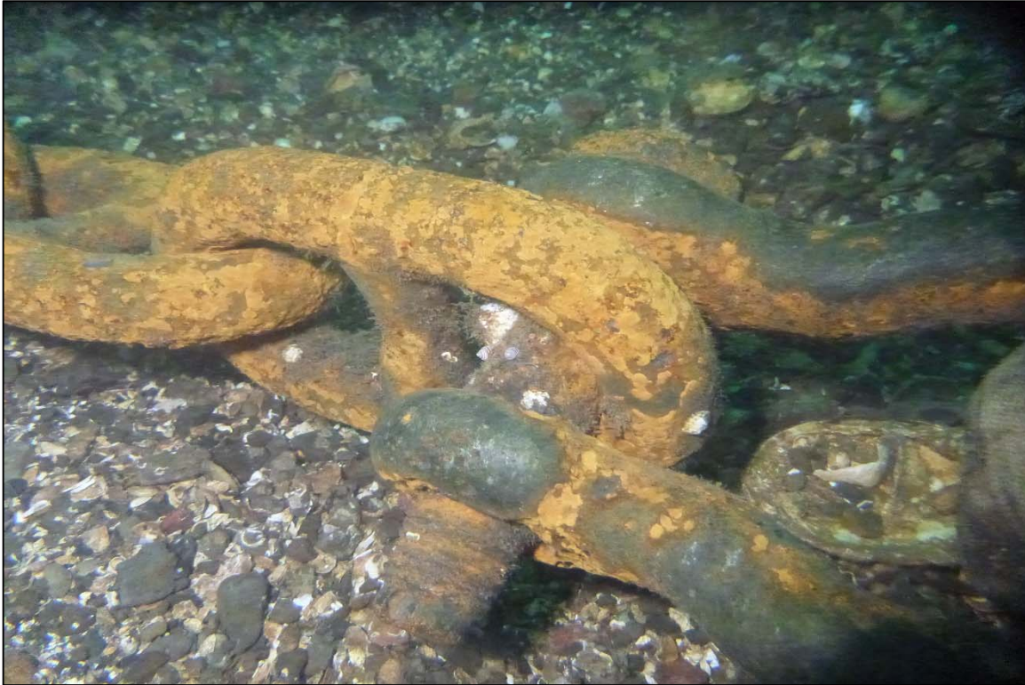
Photograph 59: View of Rope to Lower Anchor Chain Connection (Shackle and Sleeve) with Missing Nut and Cotter Pin at Orchard Rocks South Anchor Line 2, Looking South.
