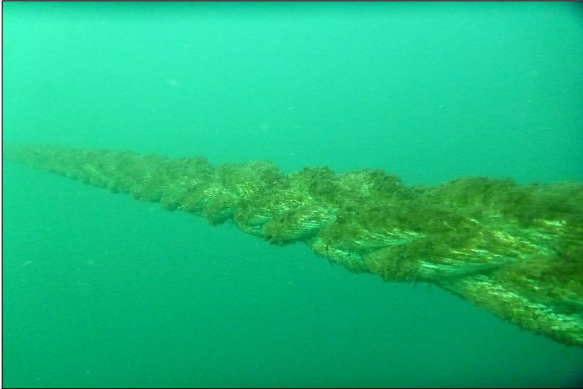
Photograph 33: View of Rope Condition with Light Marine Growth at Orchard Rocks North Anchor Line 10, Looking Northwest.
