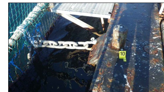
PHOTO 5 ANCHOR 10/MOORING CHAIN CONNECTED TO PREDATOR PIPE
