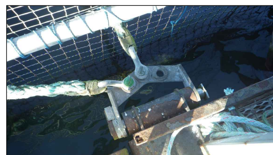
PHOTO 8 HINGE CONNECTION AND LINE TO NORTH NET PEN
