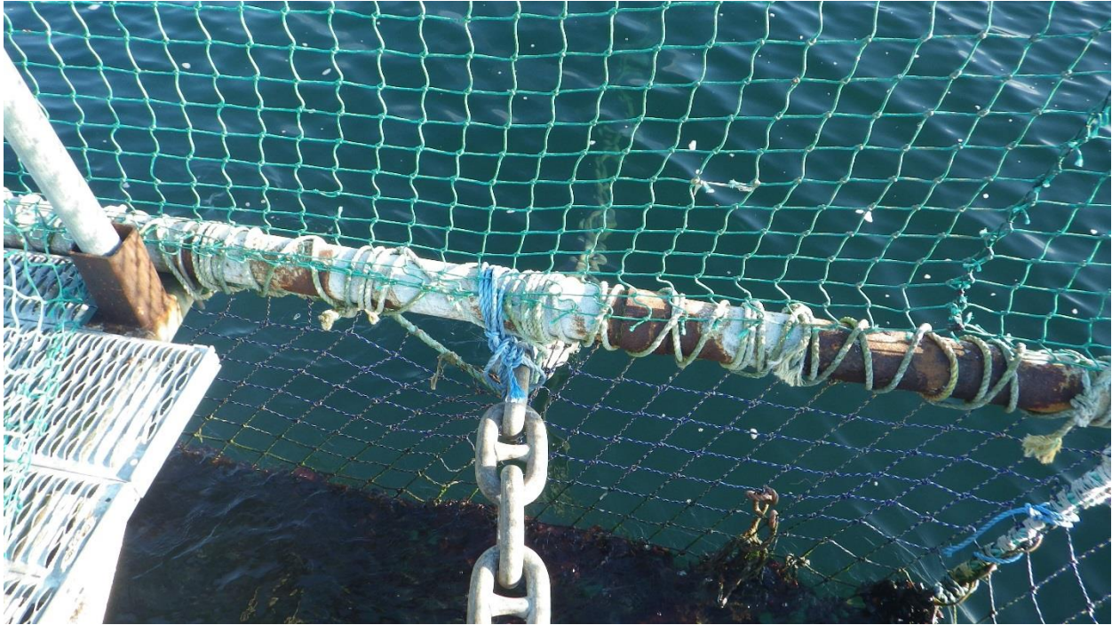
Figure C-16: Anchor #6, SE Corner of the North Net Pen. Chain attached to predator support pipe.
