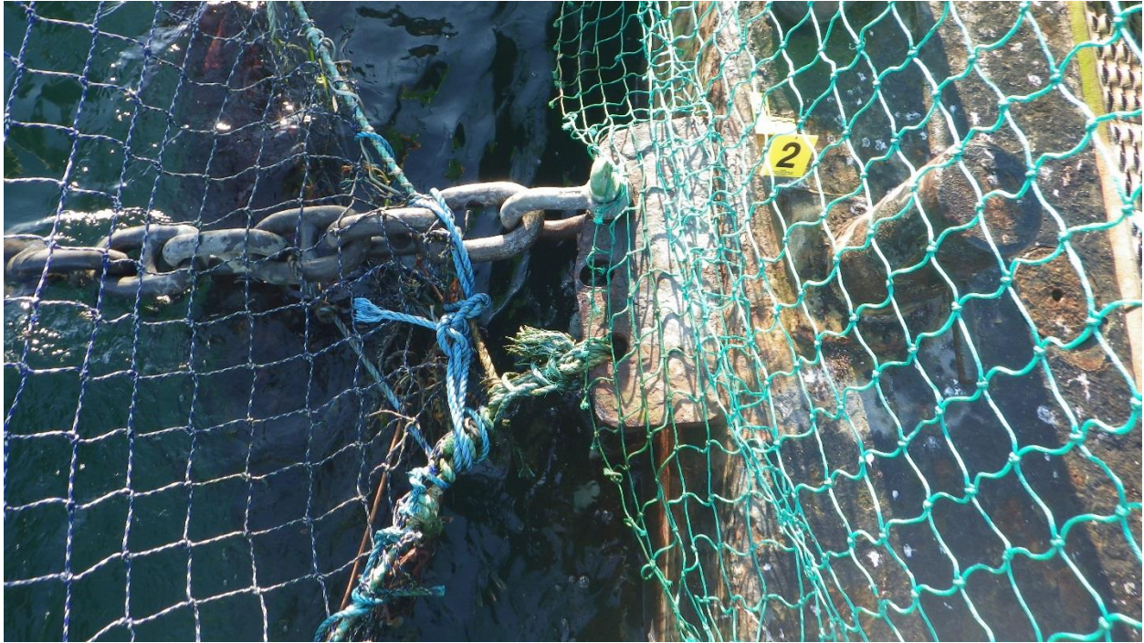
Figure C-8: Anchor #2, East Side of the North Net Pen. New shackle and chain.
