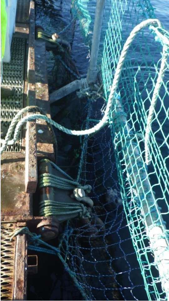
Figure C-34: Anchor #15, North Side of the North Net Pen. Hinge at different angle than chain.
