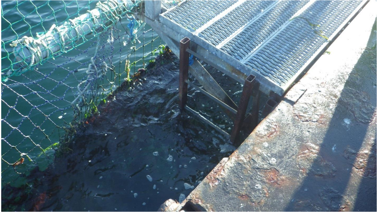
Figure C-44: Typical Fixed Ladder Connection on East side, Used for Divers
