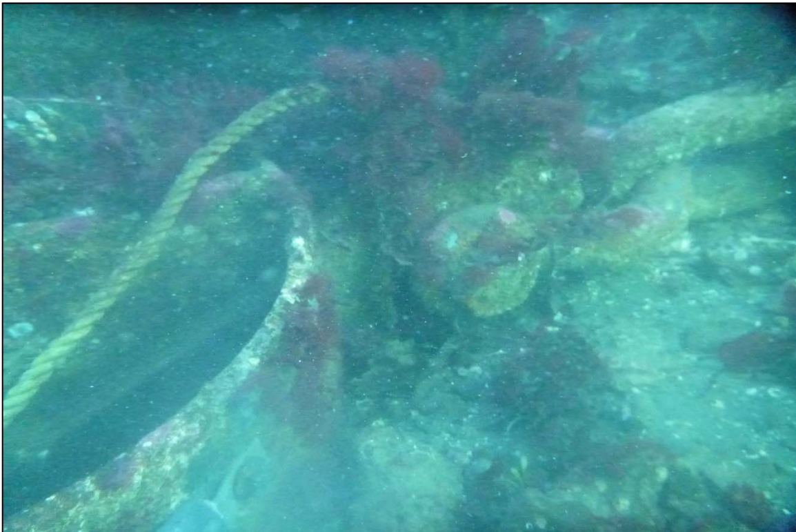
Photograph 46: View of the Anchor Chain to Pipe Anchor Connection at Orchard Rocks North Anchor Line 15, Looking East.
