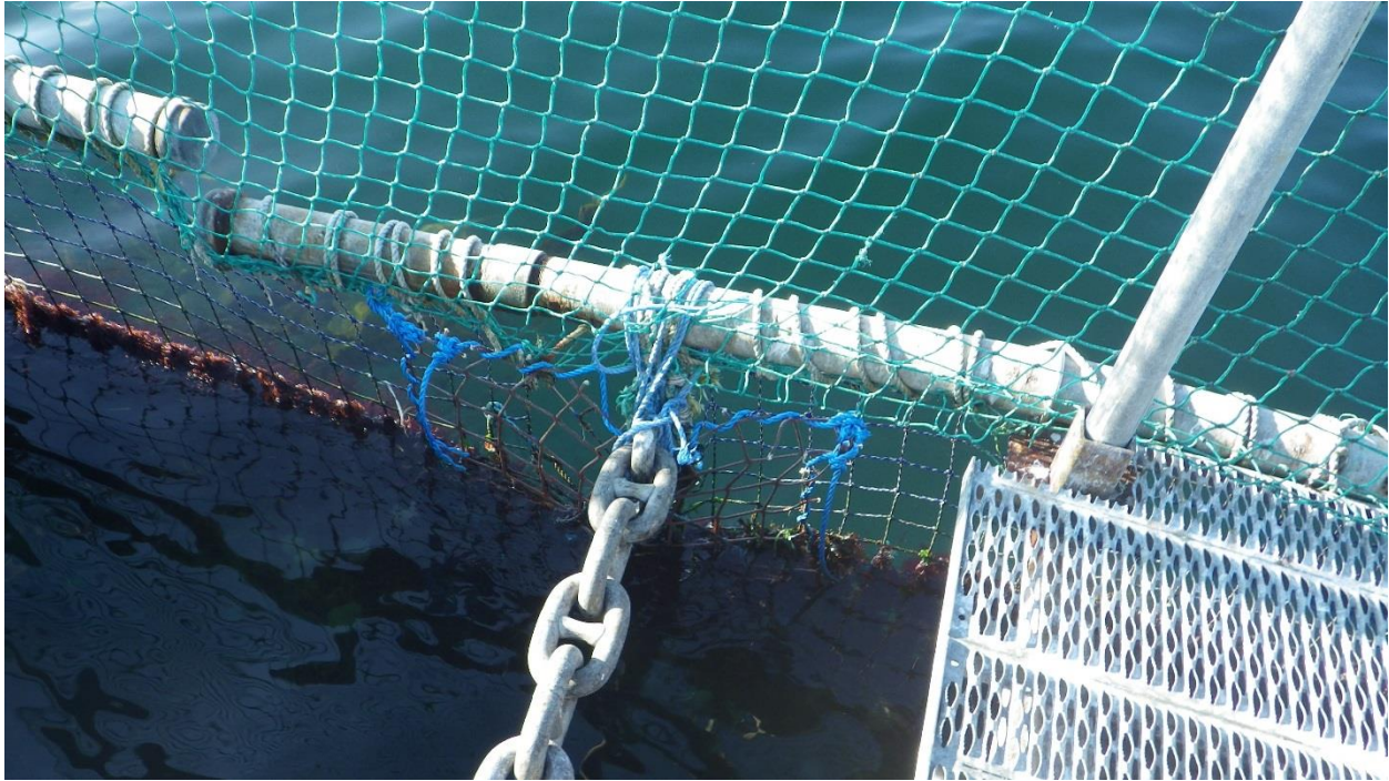
Figure C-56: Near Anchor 10, Discontinuous Predator Net Railing – Bent due chain connection load.
