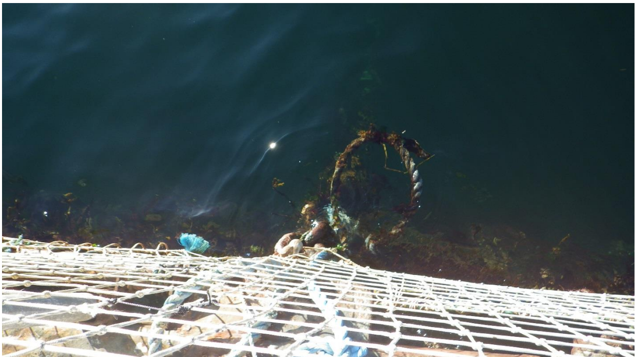
Figure D-36: Anchor #15, West Side of the South Net Pen. New shackle, with minor corrosion on chain.
