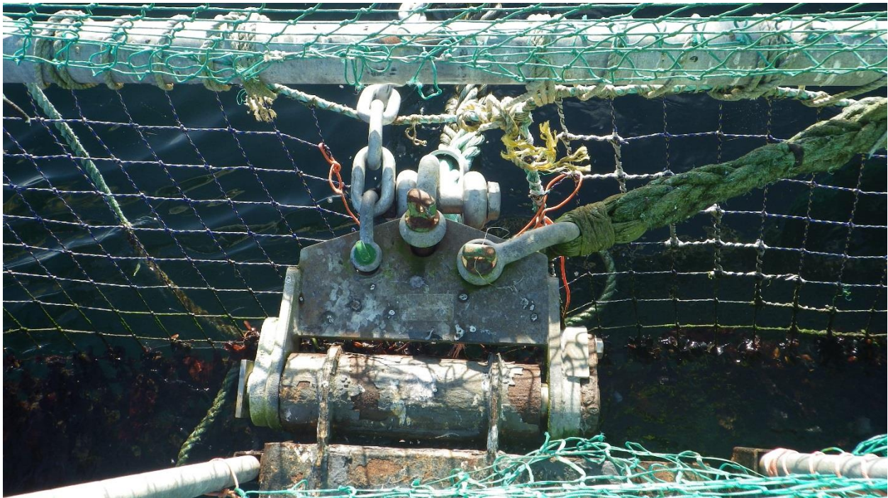
Figure C-39: North East Hinge – Connection of North and South Net Pens. Hinge with moderate corrosion.
