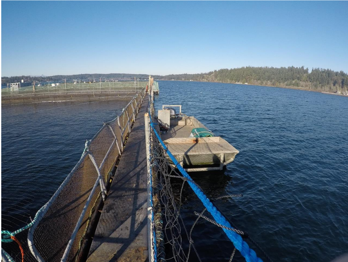
Figure D-3: View from East Side of South Net Pens, Looking North
