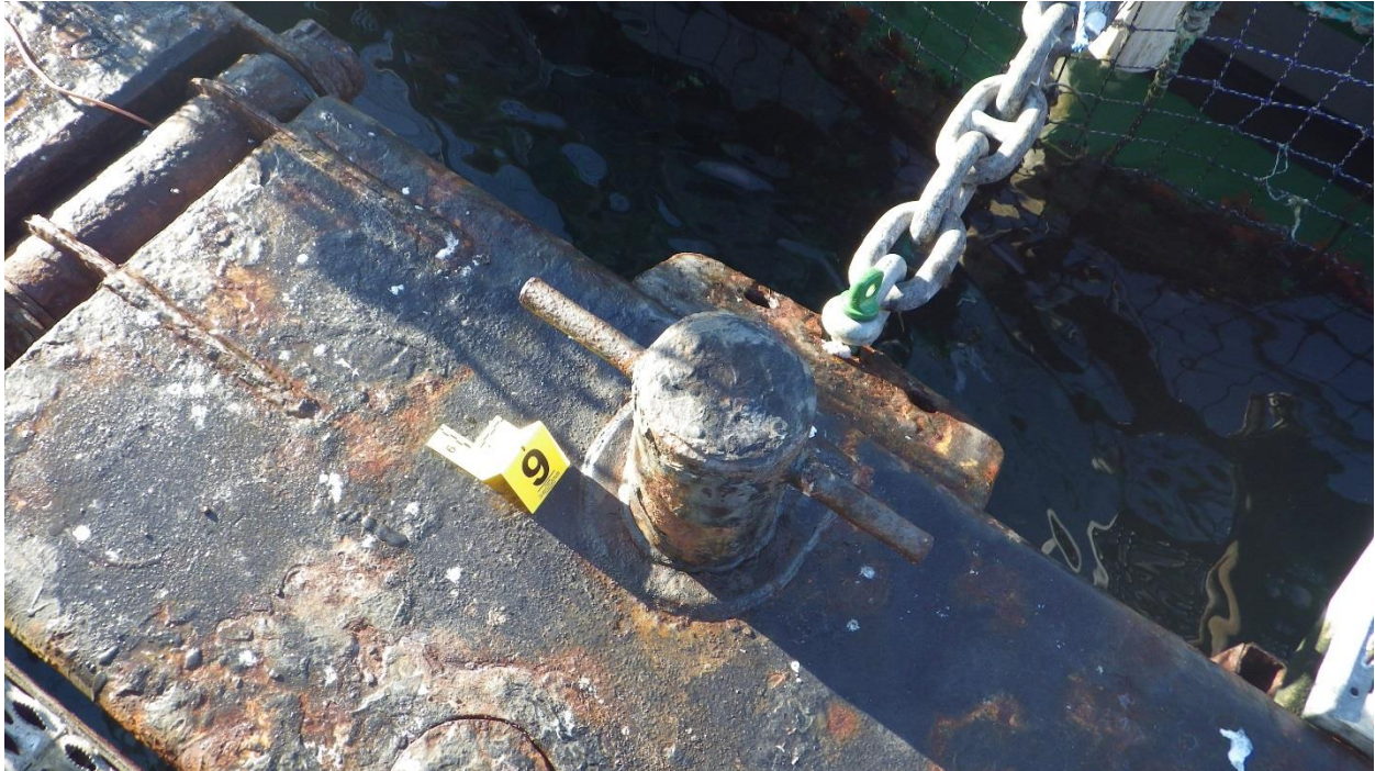
Figure C-20: Anchor #9, West Side of the North Net Pen. New shackle and chain.
