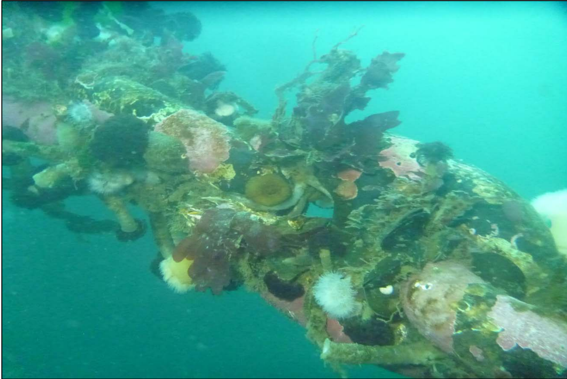
Photograph 21: View of Upper Anchor Chain Condition with Heavy Marine Growth at Orchard Rocks North Anchor Line 3, Looking North.
