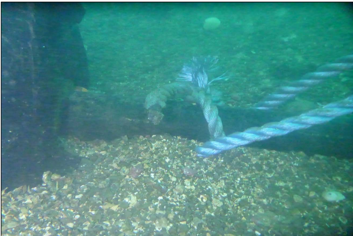
Photograph 16: View of Anchor Fluke Embedment at Orchard Rocks North Anchor Line 1, Looking East.
