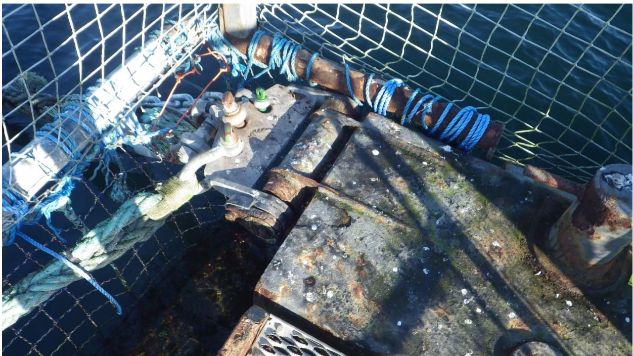
Figure D-40: South East Hinge connected to North pen.
