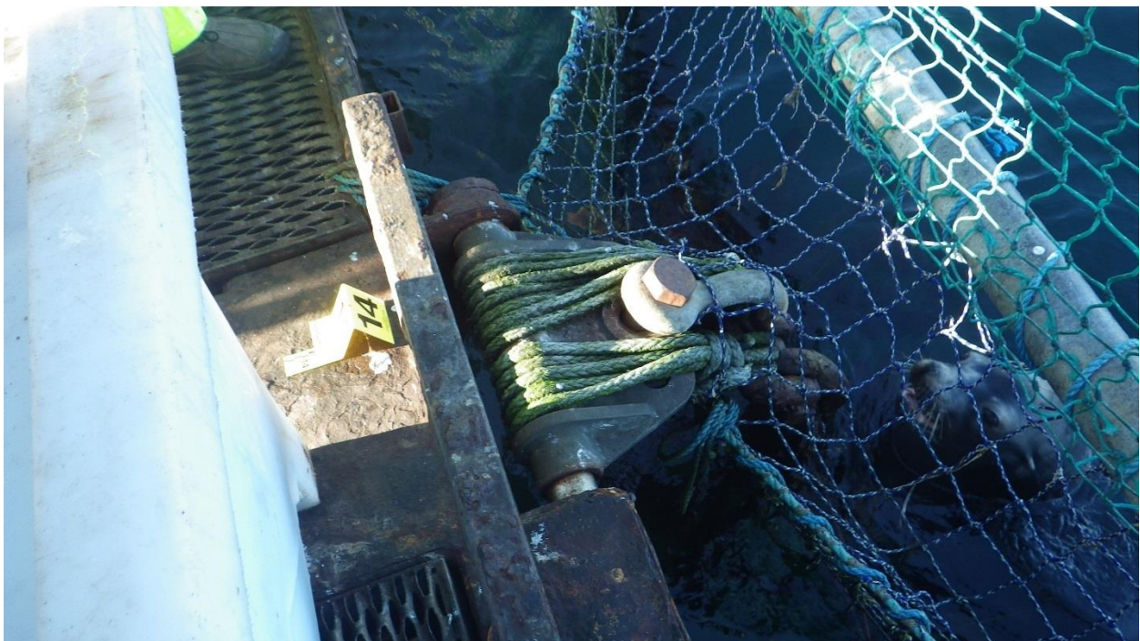
Figure C-31: Anchor #14, North Side of the North Net Pen. Hinge at different angle than chain.
