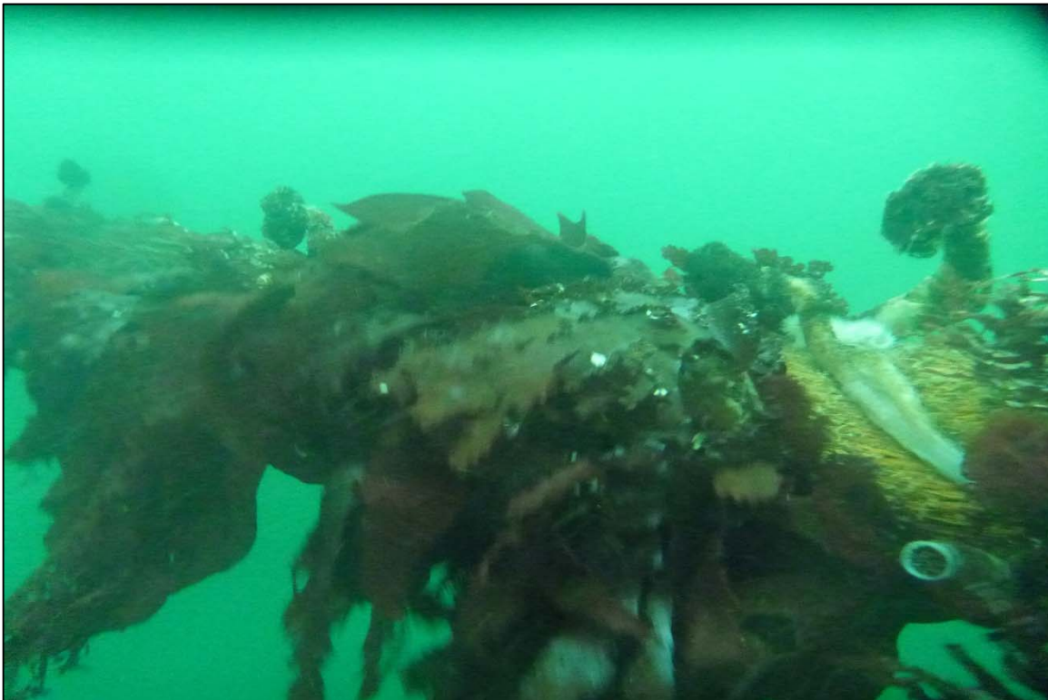
Photograph 58: View of Heavy Marine Growth on the Rope at Orchard Rocks South Anchor Line 2, Looking Southeast.
