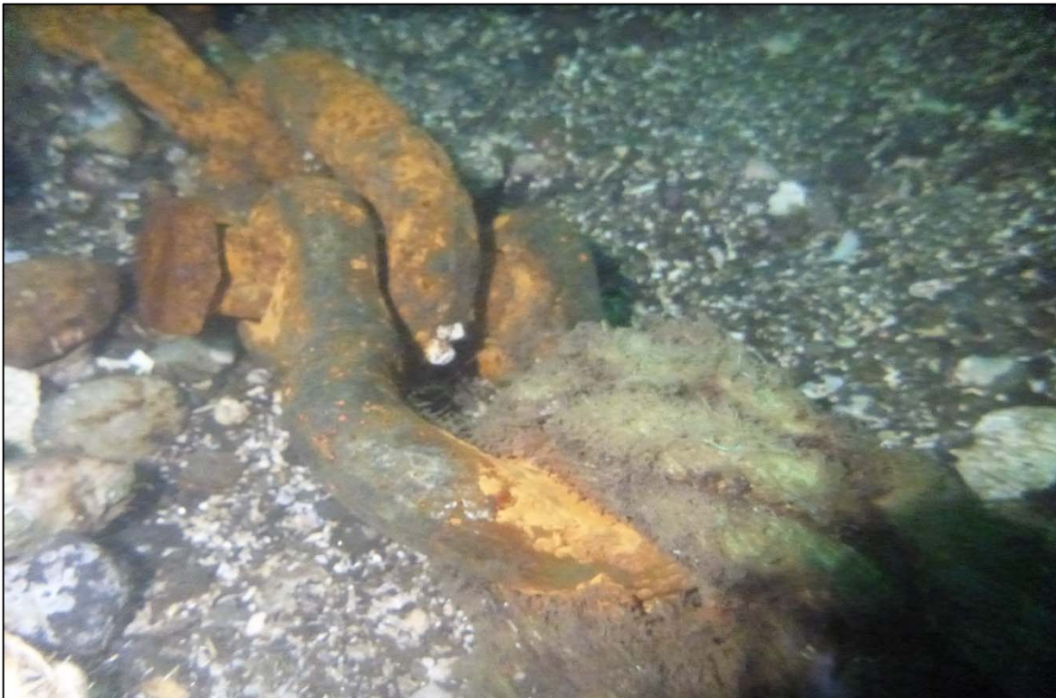
Photograph 68: View of Lower Anchor Chain to Anchor Rope Connection at Orchard Rocks South Anchor Line 5, Looking East. Bolt Head is Not Flush with Shackle indicating the bolt is likely loose.
