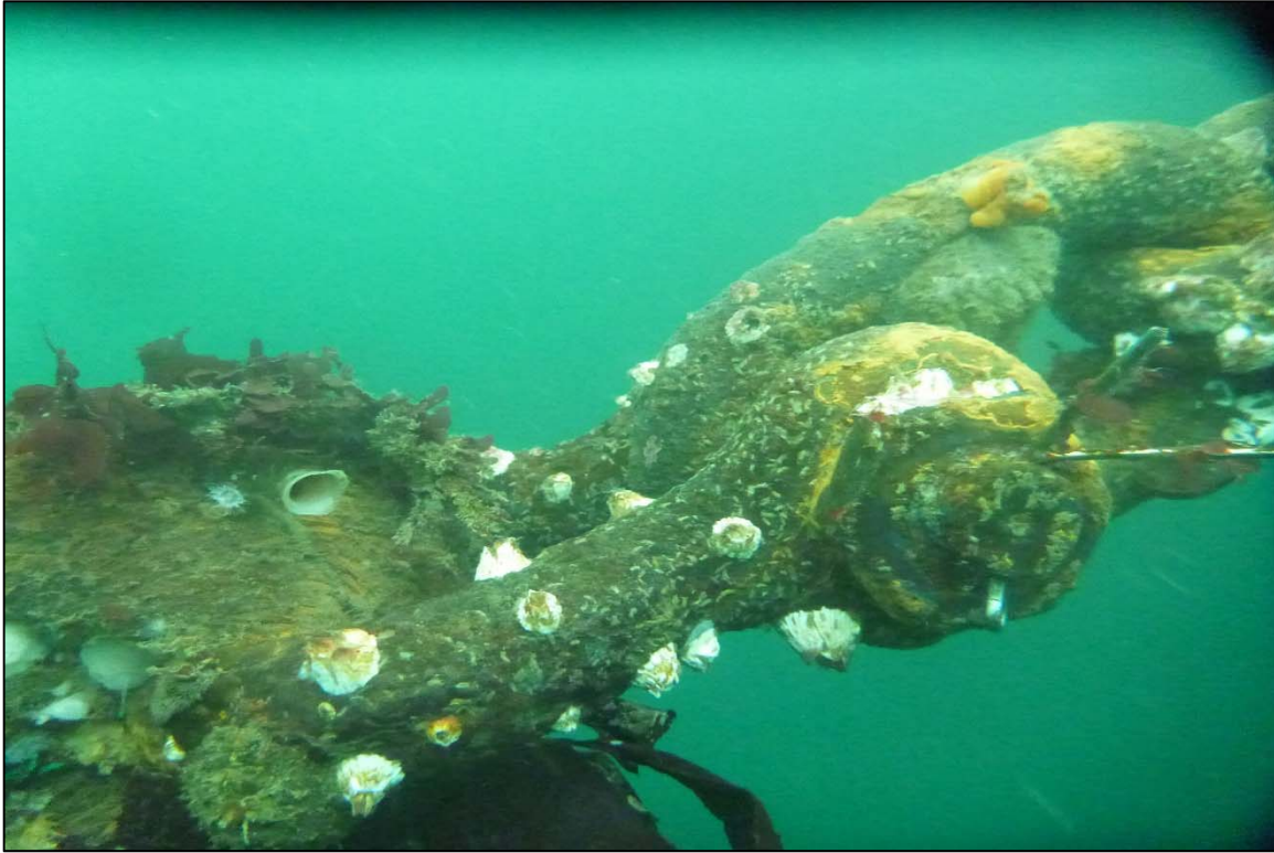
Photograph 57: View of Upper Chain to Rope Connection (Shackle) at Orchard Rocks South Anchor Line 2, Looking South.
