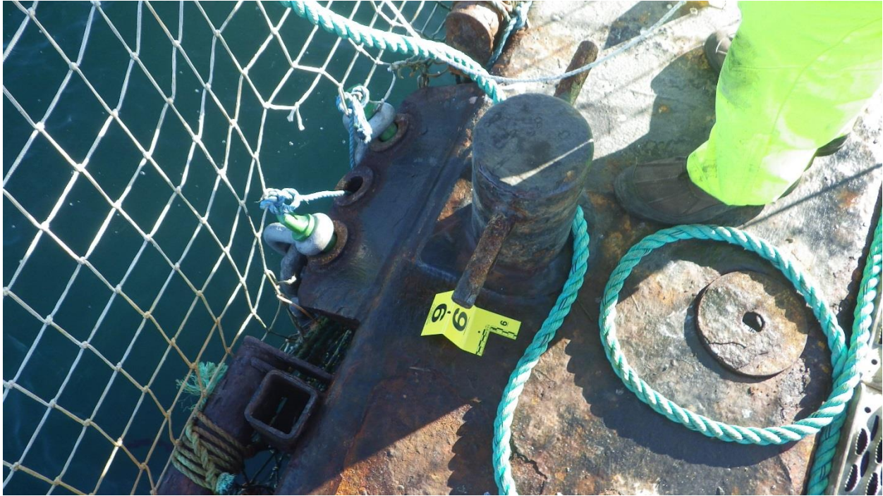
Figure D-15: Anchor #6, SE Corner of the South Net Pen
