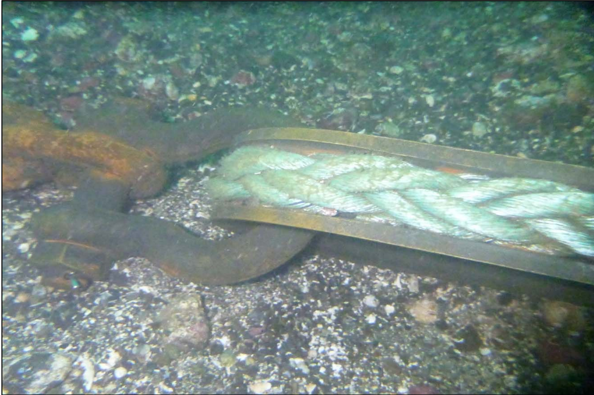
Photograph 65: View of Secure Lower Anchor Chain to Float Connection at Orchard Rocks South Anchor Line 4, Looking West.
