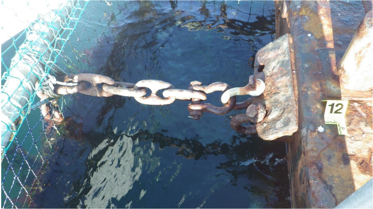
Figure C-26: Anchor #12, NW Corner of the North Net Pen. Chain tied to predator support pipe.
