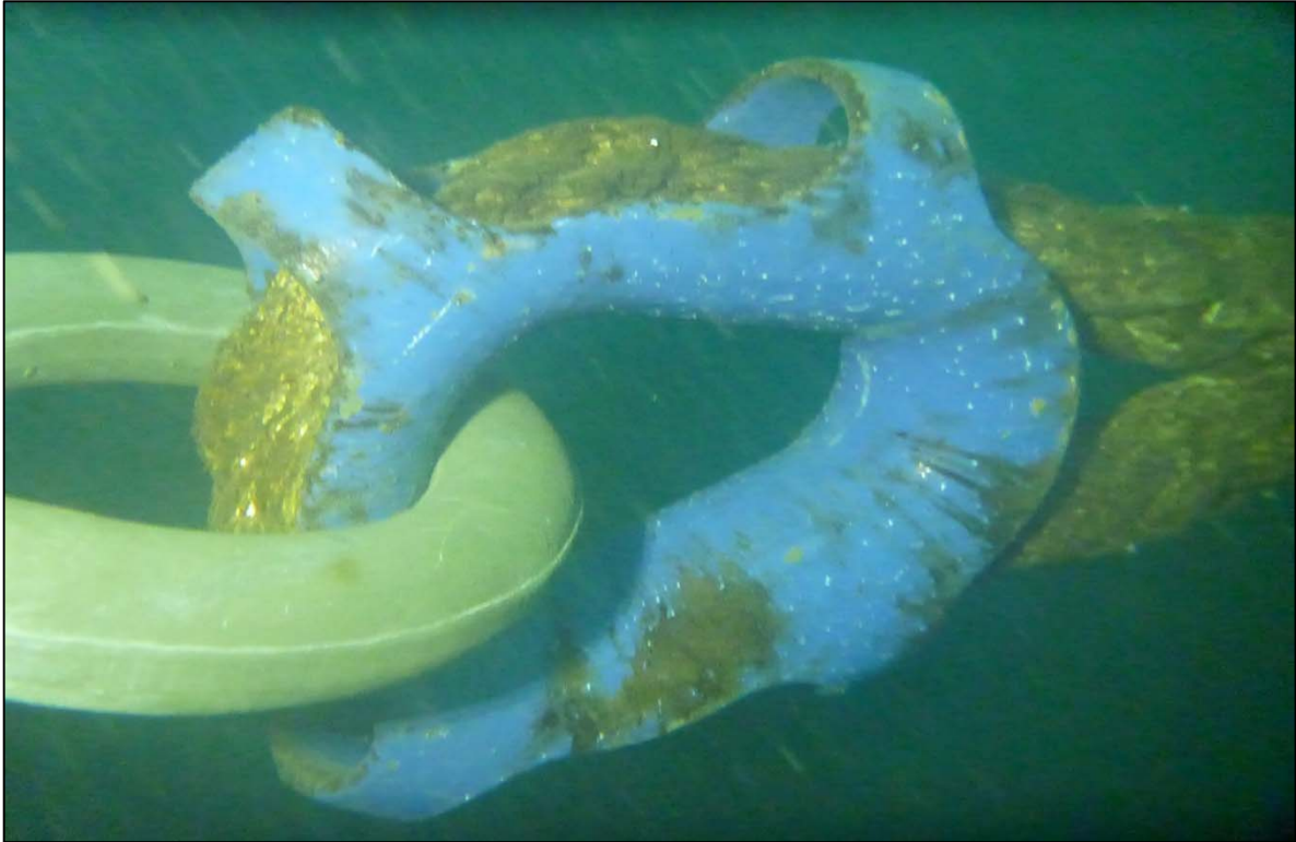
Photograph 73: View of Upper Anchor Chain to Anchor Rope Connection (Thimble and Shackle) at Orchard Rocks South Anchor Line 6A, Looking West.
