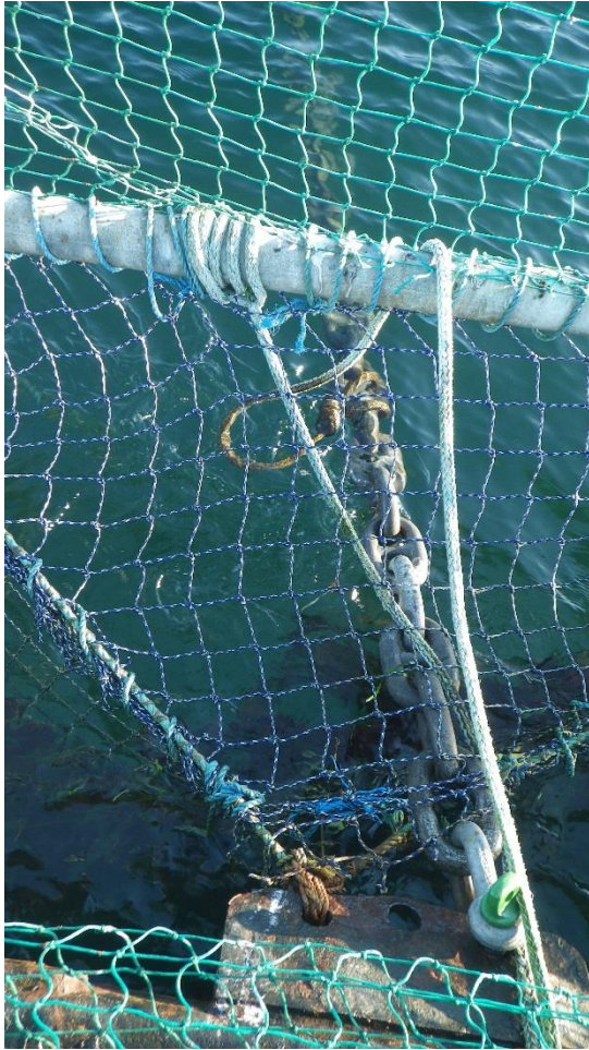
Figure C-6: Anchor #1, NE Corner of the North Net Pen. New shackle and chain.
