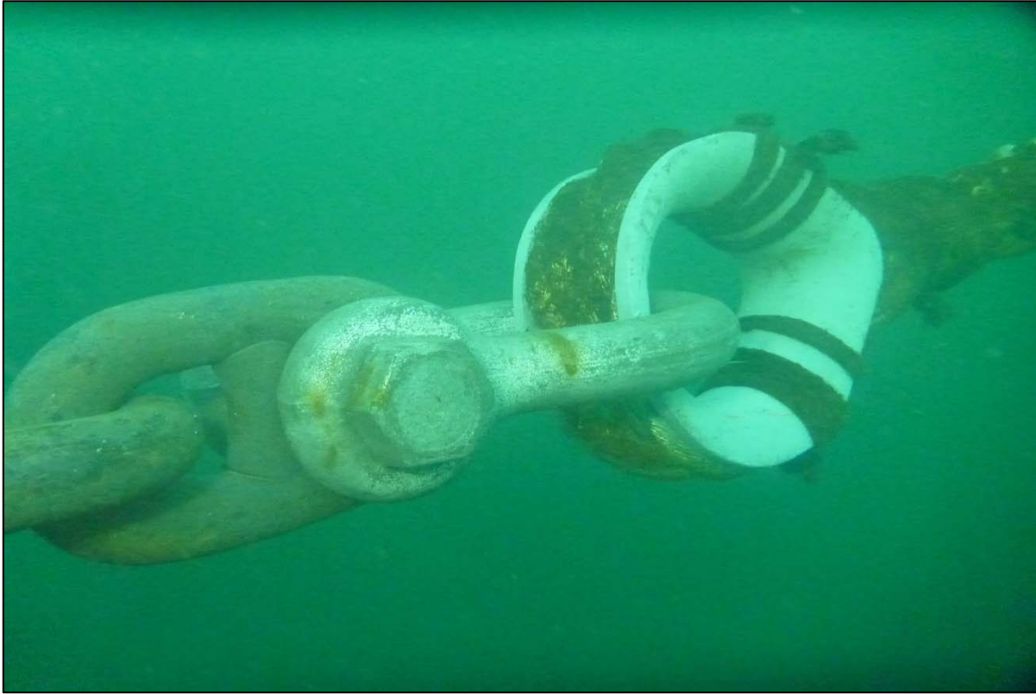
Photograph 13: View of Upper Anchor Chain to Rope Connection (Shackle and Thimble) Orchard Rocks North Anchor Line 1, Looking Northeast.
