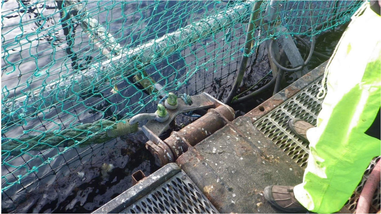
Figure C-36: North East Mid – Interconnection of North and South Net Pens
