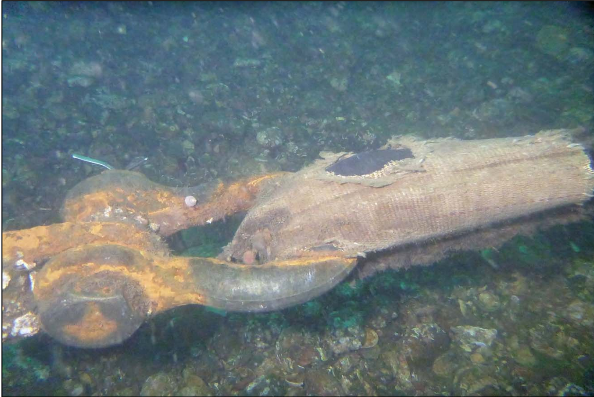
Photograph 61: View of Rope to Lower Anchor Chain (Shackle and Sleeve) at Orchard Rocks South Anchor Line 3, Looking South.
