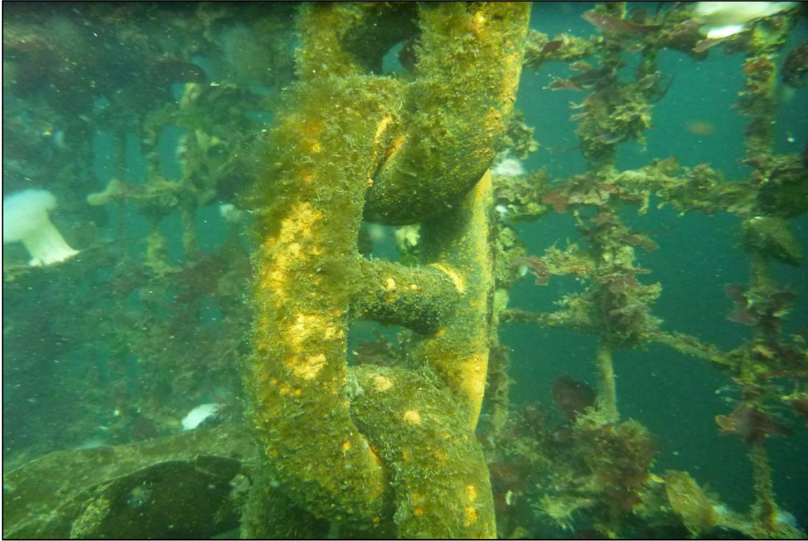
Photograph 35: View of Light Marine Growth on the Upper Anchor Chain at Orchard Rocks North Anchor Line 11, Looking North.
