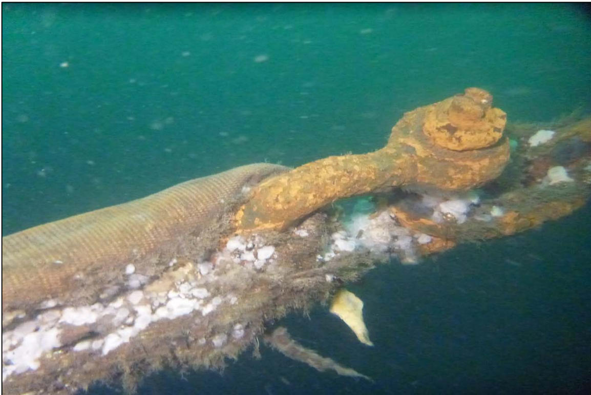
Photograph 60: View of Upper Anchor Chain to Rope Connection (Shackle and Sleeve) with Missing Cotter Pin at Orchard Rocks South Anchor Line 3, Looking South.
