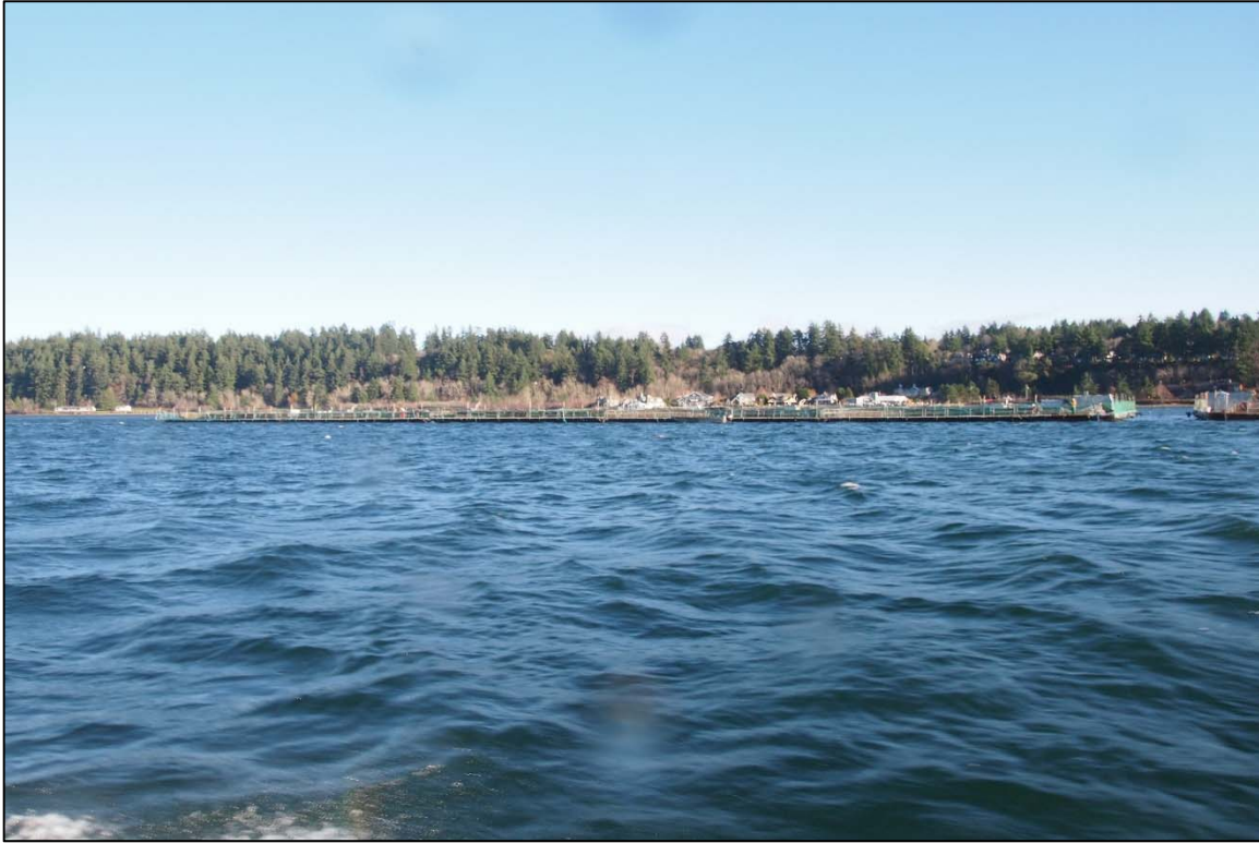
Photograph 3: Overall View of the Orchard Rocks North Fish Net Pens System, Looking East.
