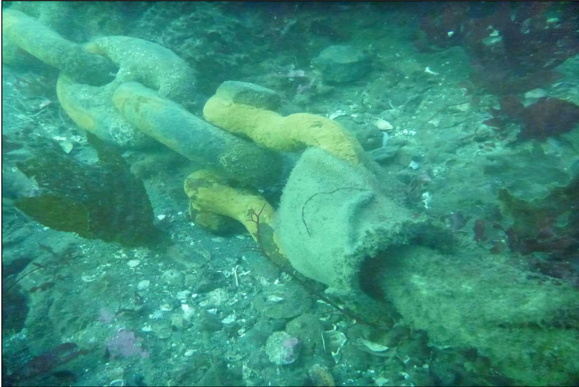
Photograph 39: View of the Rope to Lower Anchor Chain (Shackle and Sleeve) at Orchard Rocks North Anchor Line 12, Looking Northeast.
