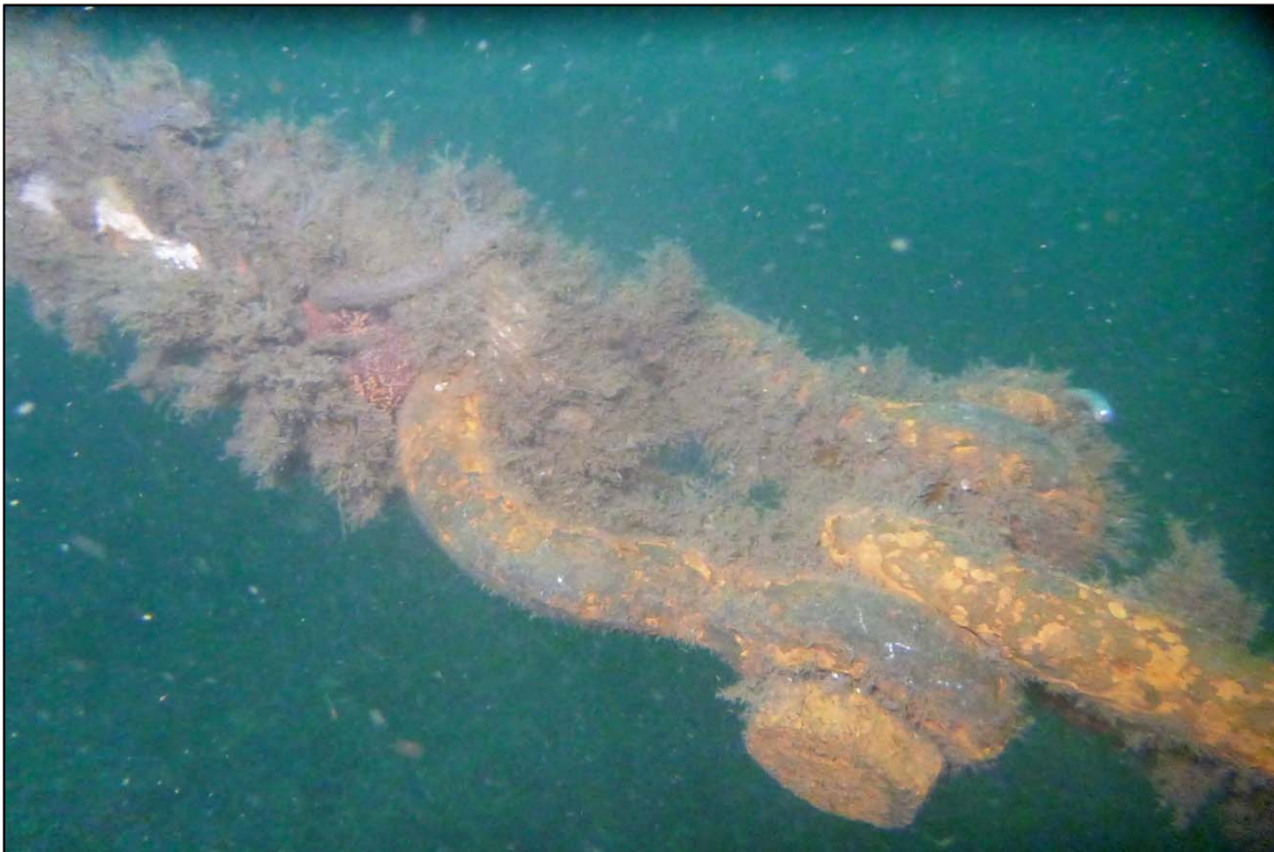
Photograph 22: View of Rope to Lower Anchor Chain Connection (Shackle) with Severe Corrosion and Thread Loss on the Bolt at Orchard Rocks North Anchor Line 3, Looking North.
