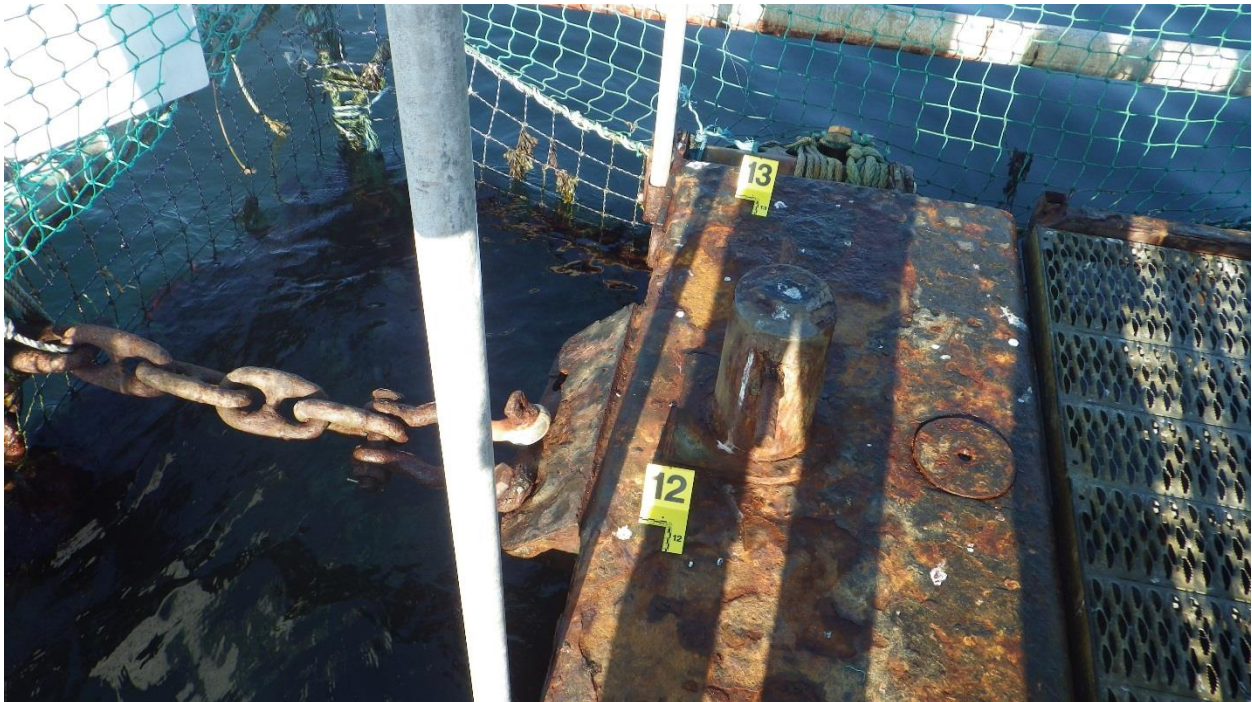
Figure C-25: Anchor #12, NW Corner of the North Net Pen. Moderate corrosion on chain.
