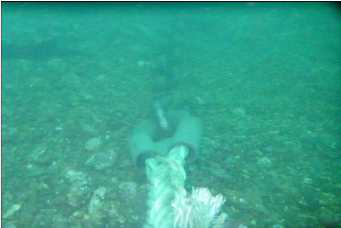
Photograph 18: View of Rope to Lower Anchor Chain Connection (Shackle and Thimble) at Orchard Rocks North Anchor Line 2, Looking East.
