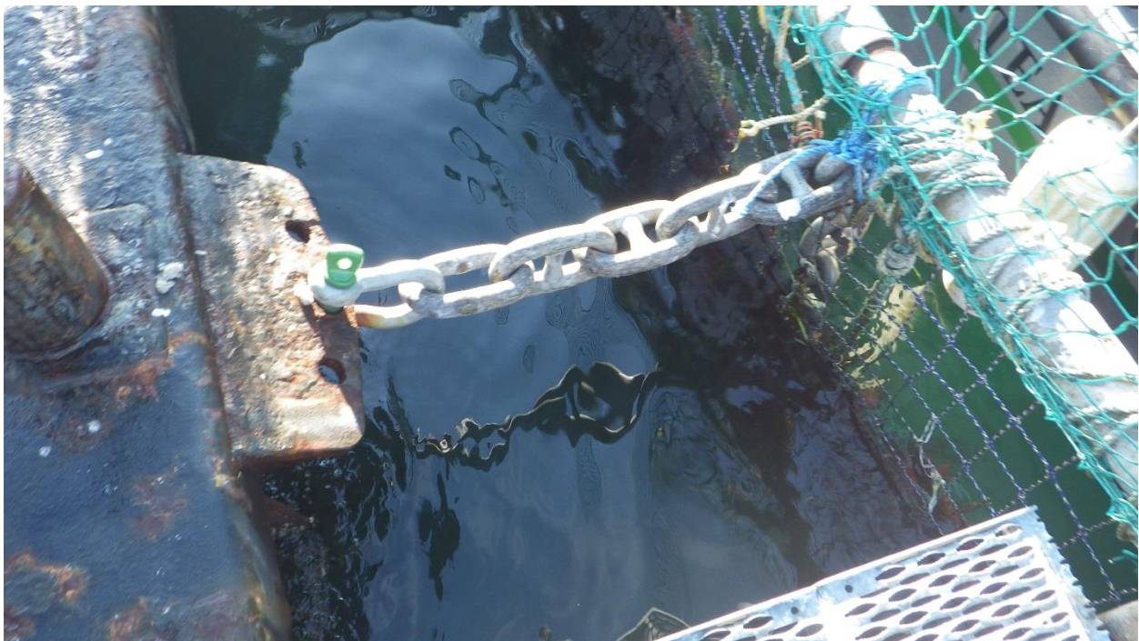
Figure C-21: Anchor #9, West Side of the North Net Pen. Chain tied to predator support pipe.
