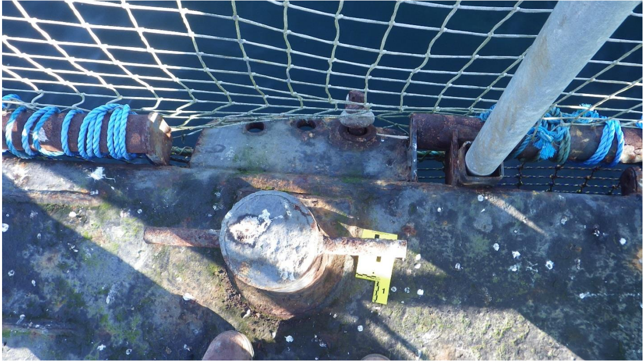
Figure D-5: Anchor #1, NE Corner of the South Net Pen
