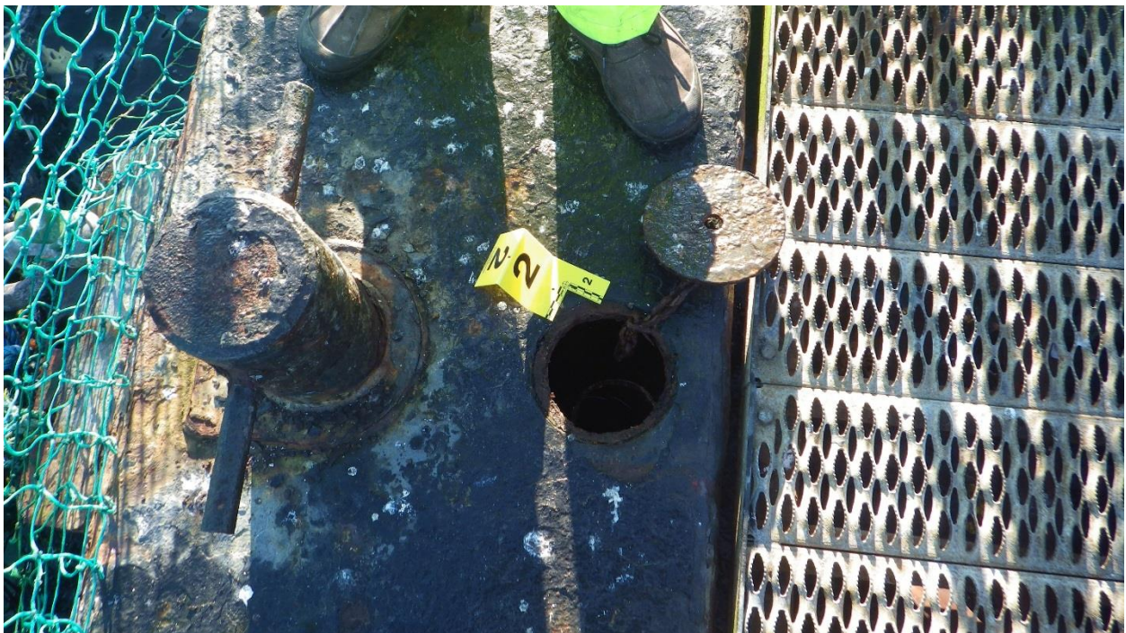
Figure C-9: Anchor #2, East Side of the North Net Pen. Old anchor access port.
