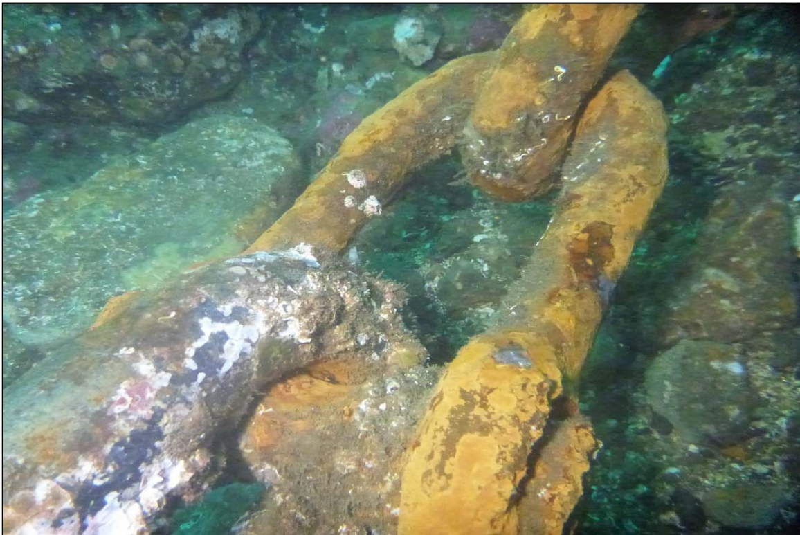
Photograph 48: View of Lower Anchor Shackle with Heavy Corrosion and Section Loss at Orchard Rocks North Anchor Line 16, Looking North.
