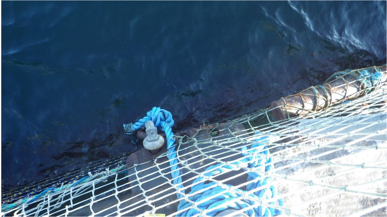
Figure D-7: Anchor #2, East Side of the South Net Pen. Newer shackle, old chain.
