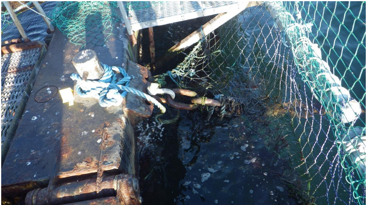
Figure C-11: Anchor #3, East Side of the North Net Pen
