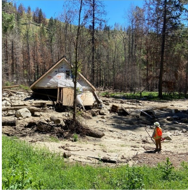
House impacted by a 2022 post-fire debris flow in Conconully, Okanogan County following a storm event after the 2021 Muckamuck Fire
