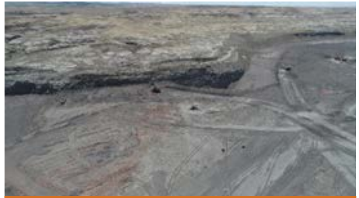
The Yazzie Wildlife Bluff – Backfilling process
