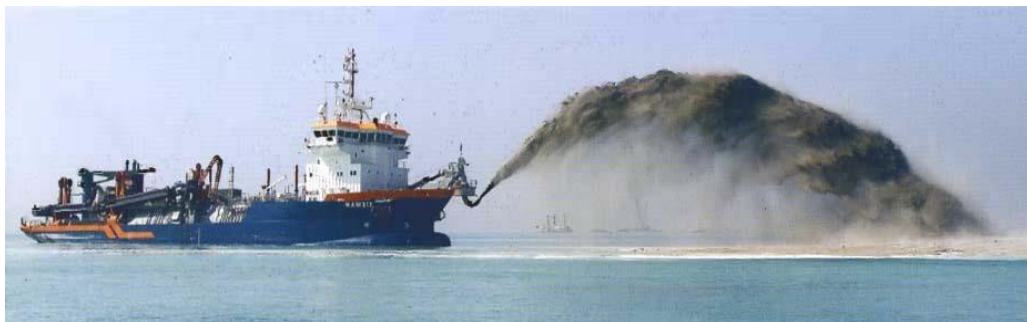
Figure 4.7: Trailing Suction Hopper Dredger Rainbowing (Van Oord Australia)
