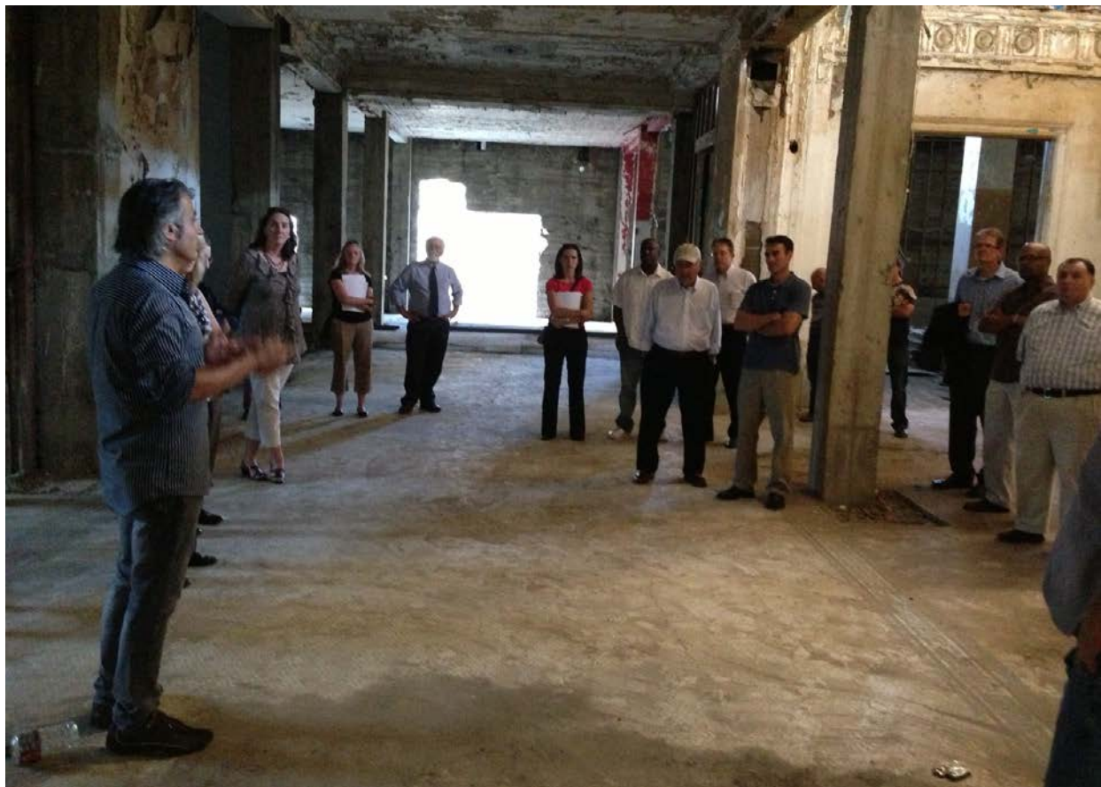
Figure 7: Hotel Rehabilitation, Fresno, California. Developers often encounter challenges in converting a historic building to a new use. Photo source: Renaissance Planning Group
