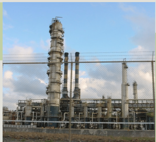
Oil refinery on St. Croix, U.S. Virgin Islands.
