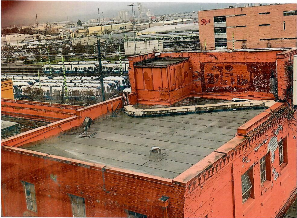
Building 10 Roof View (Facing Southwest)
