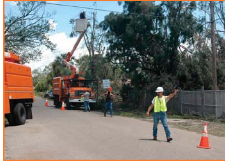
Appoint a flagger or use barricades and warning signs to control traffic or onlookers.
