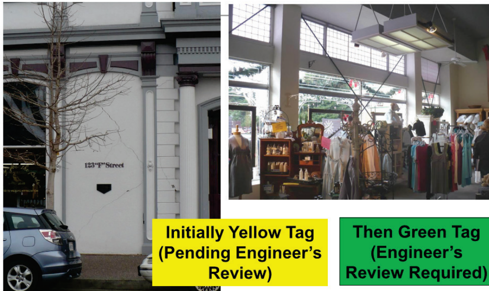
Figure 6-2 Placard posting approach in commercial building in 2010 Eureka, California earthquake. The initial placard was a yellow RESTRICTED USE tag with the recommendation for an engineering review. The placard was subsequently changed to a green INSPECTED tag, but still said an engineer review is required.
