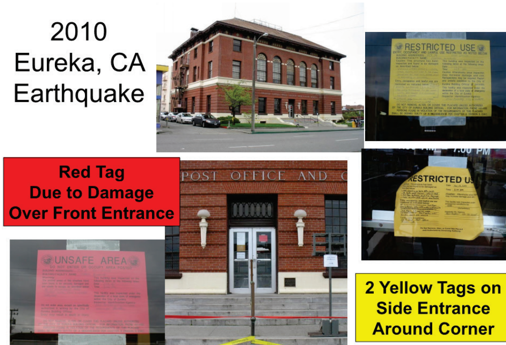
Figure 6-3 Placards posted on a government building in 2010 Eureka, California earthquake. Both yellow RESTRICTED USE and red UNSAFE placards were observed. Placards should be consistent on each side of the building.
