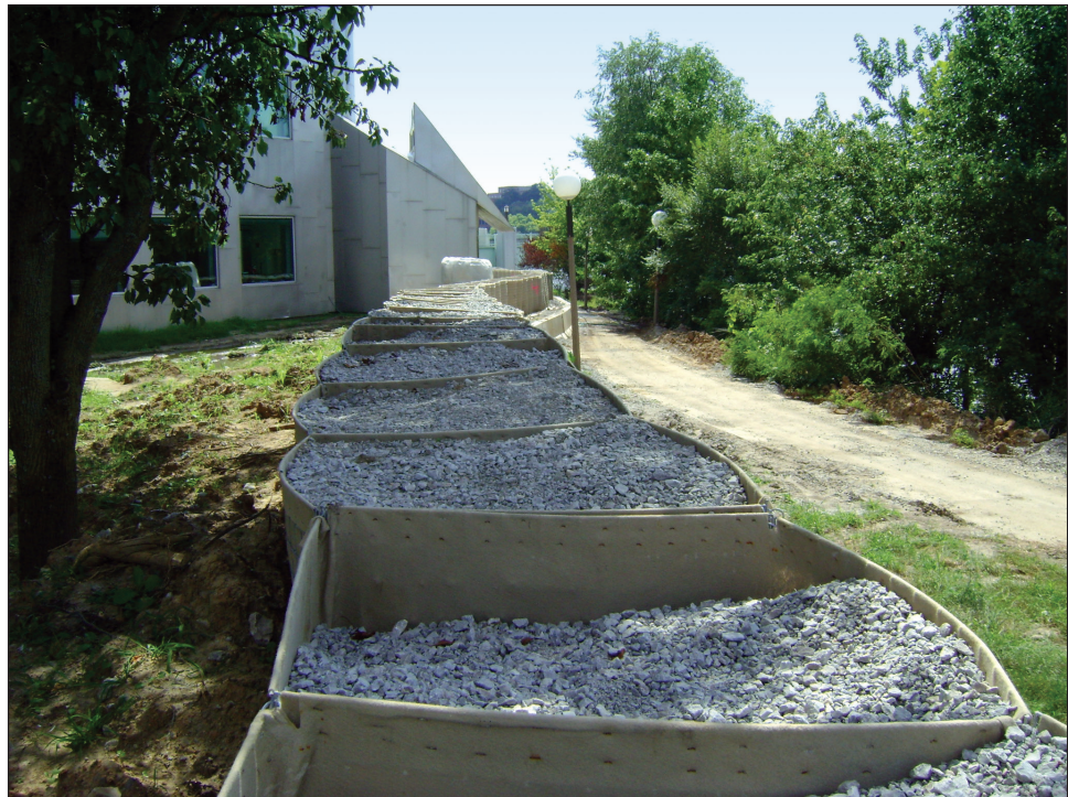
Figure 4-24. Gravel-filled containers that formed a barrier to protect the University of Iowa (2008)
