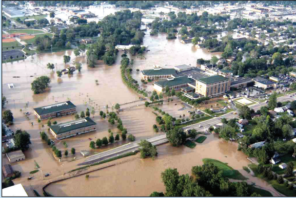
Figure 4-7. Floodwaters surround Columbus Regional Hospital in 2008
