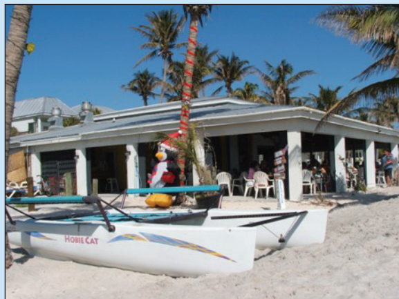
Figure 4-12. The Duval Beach Club after wet floodproofing retrofits
