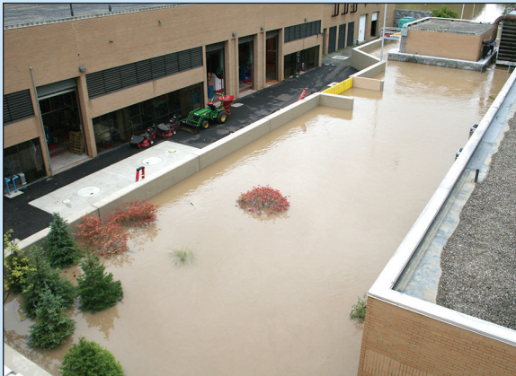
Figure 4-5. Floodwall successfully safeguards Lourdes Hospital from Tropical Storm Lee flooding (source: FloodBreak)
