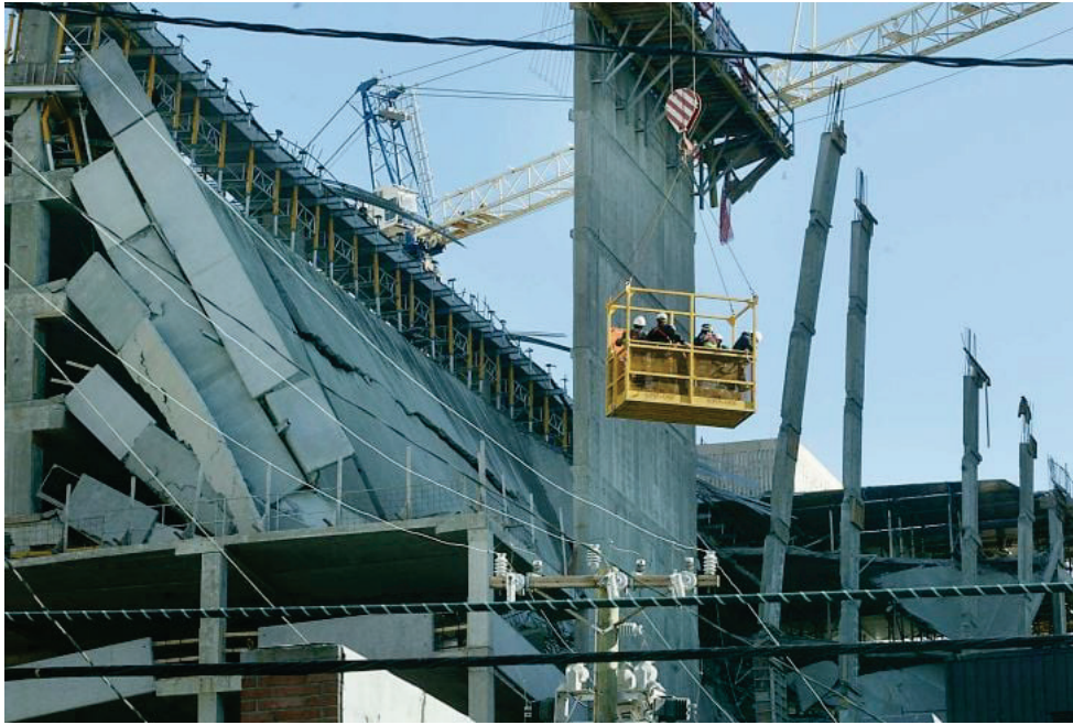
Figure 3-10 Laterally unsupported columns and shear wall following partial collapse of Tropicana Casino parking garage during construction in Atlantic City, New Jersey, 2003.
