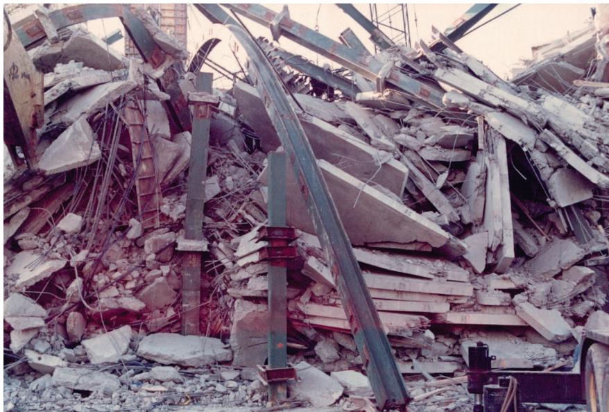
Figure 3-27 L'Ambiance Plaza collapse during construction, Bridgeport, Connecticut, 1987 (Exponent/Peraza).
