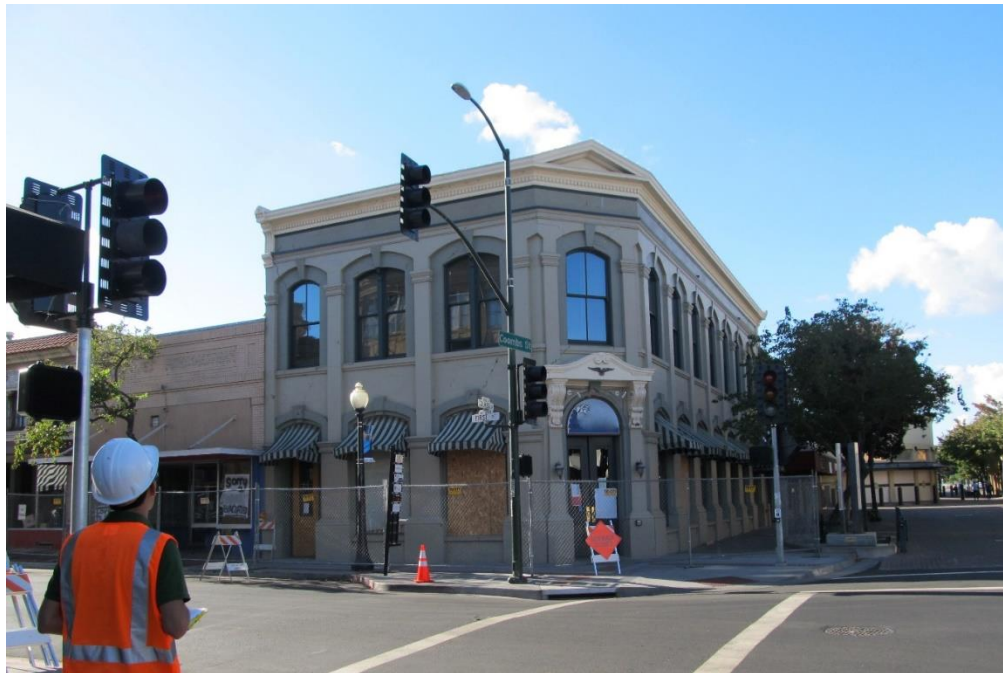
Figure 2-3 A URM building with in UNSAFE placard with a very narrow cordon around it. (FEMA P-1024 Figure 12-1).
