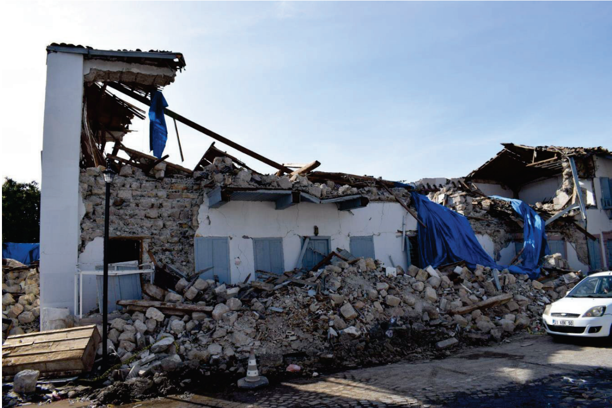
Figure 3-39 Adobe dwelling in Arsuz after the 2023 Kahramanmaraş Earthquake (Türkiye) (Photo Credit: Thornton Tomasetti/Galvis).
