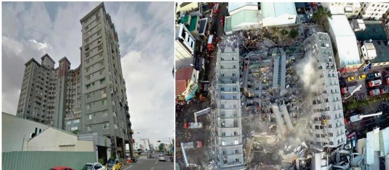
Figure 4: Pre-Collapse photo West Side (Source: google maps)
