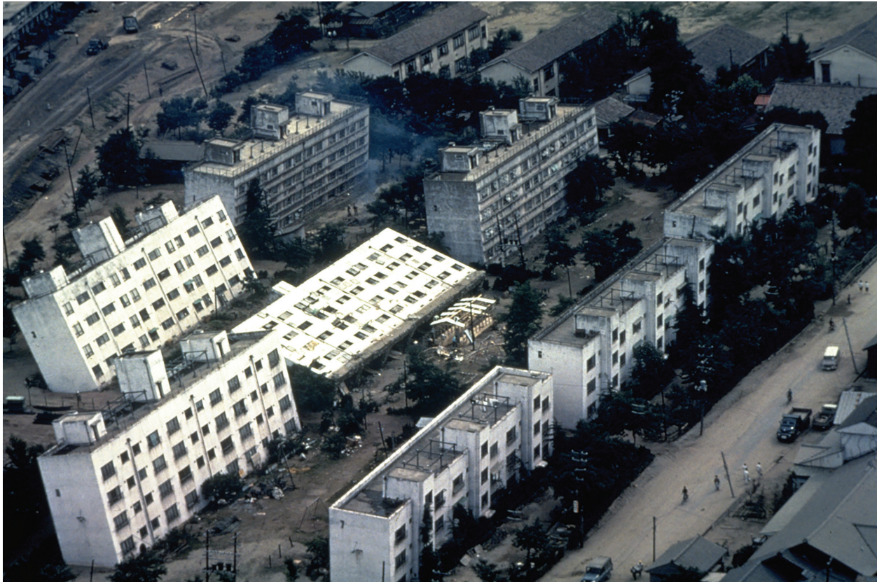
Figure 3-5 Tilting of apartment buildings due to liquefaction in 1964 Niigata Japan earthquake (Photo Credit: NISEE).
