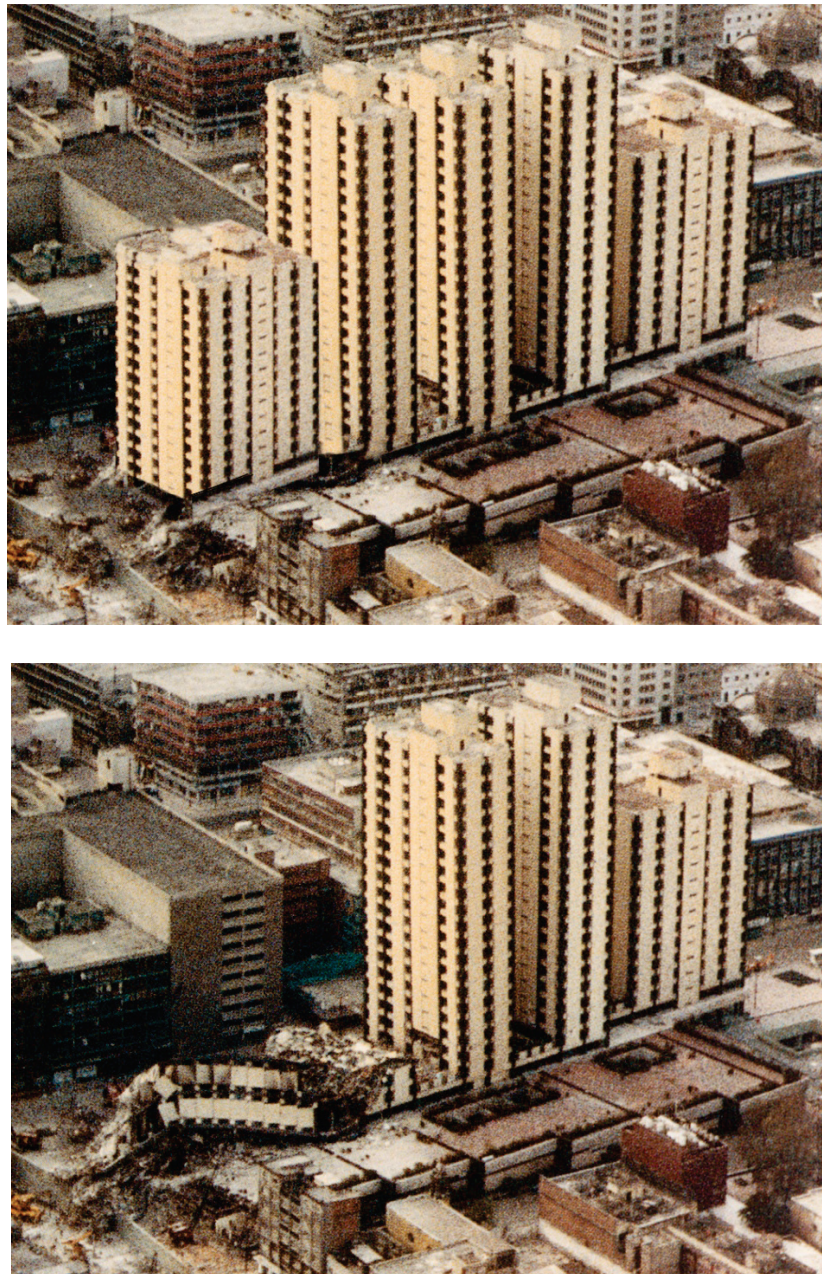
Figure 3-6 Piño Suarez towers before and after the 1985 Mexico City Earthquake (from Reports on the Damage Investigation of the 1985 Mexico Earthquake , Architectural Institute of Japan, 1987; upper image photoshopped by Exponent to include all five original towers).
