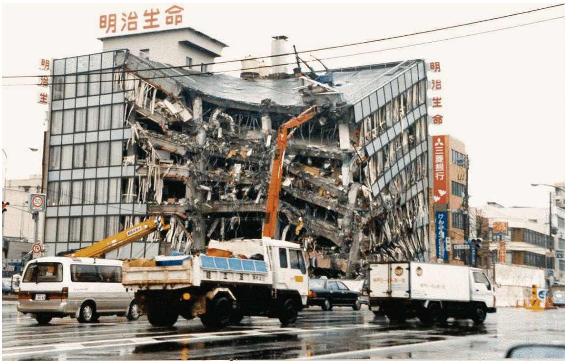
Figure 3-22 Corner building collapse in 1995 Kobe Earthquake in Japan (Exponent/Osteraas).
