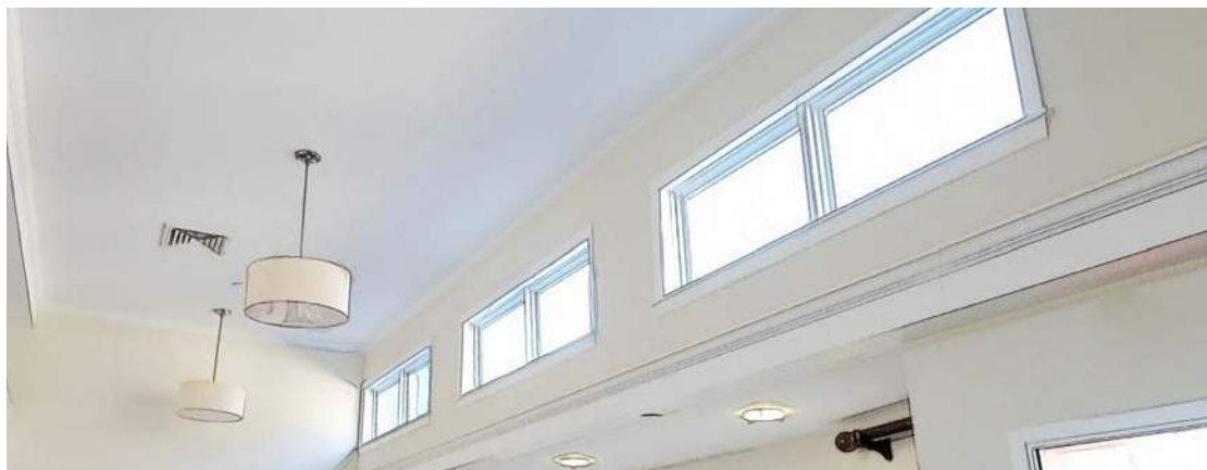
Figure 32: Clerestory lighting at White Oak Cottages. Photo Credit R.Wrublowsky, 2016. Westwood, MA. EGA Architects.
