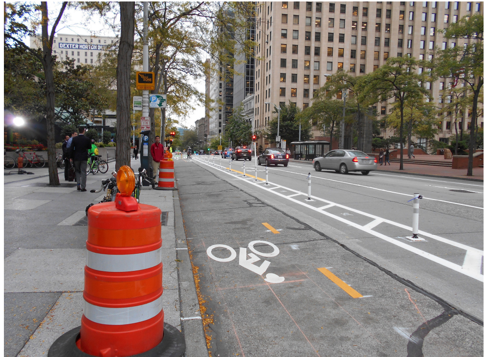
Seattle's 2nd Avenue two-way separated bike lane provides adequate width and access for street sweeping vehicles. (Source: Seattle Department of Transportation)
