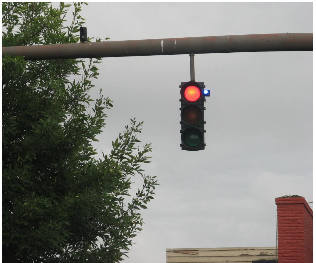
A blue light detector feedback device along NE Multnomah Street in Portland, OR. (Source: Jesse Boudart)
