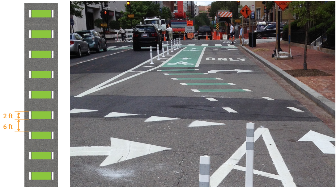
Green paint across a mixing zone opening on M Street NW in Washington, DC (Source: Jason Broehm)
