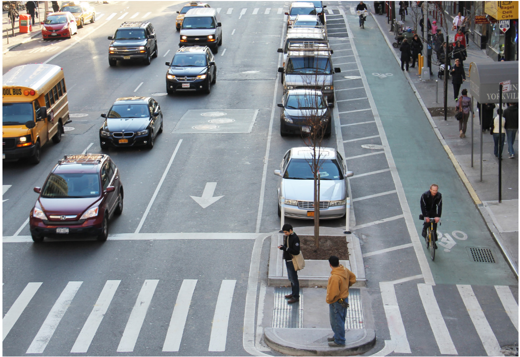
Pedestrians wait to cross 1st Avenue in New York City on a median island refuge. (Source: NYCDOT)
