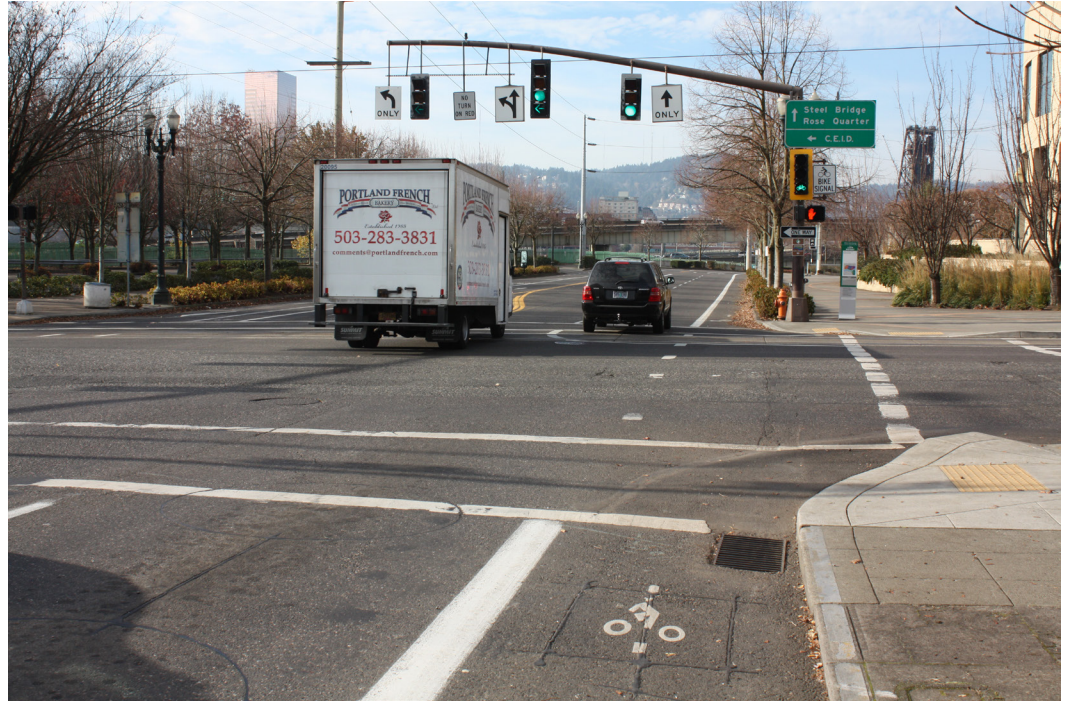
A bicycle detector pavement marking (MUTCD Figure 9C-7) communicates to bicyclists where to position themselves for signal detection in Portland, Oregon (Source: Jesse Boudart)
