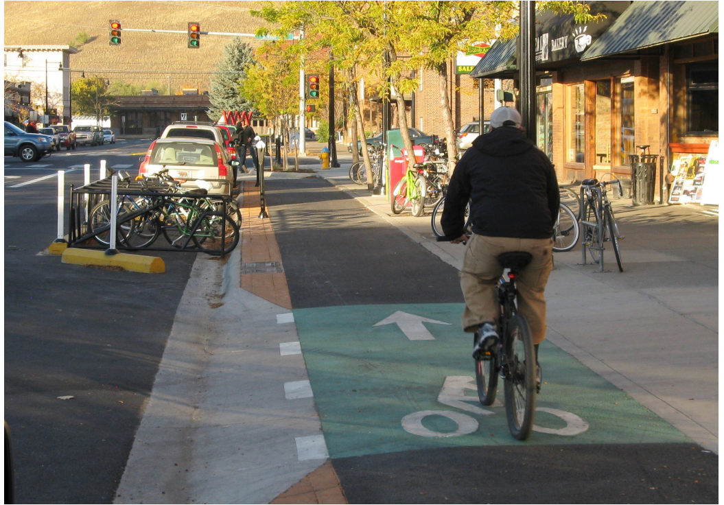
A raised lane combined with curbside bicycle and car parking provide vertical and horizontal separation from vehicular traffic on Higgins Street in Missoula, MT. (Source: City of Missoula)
