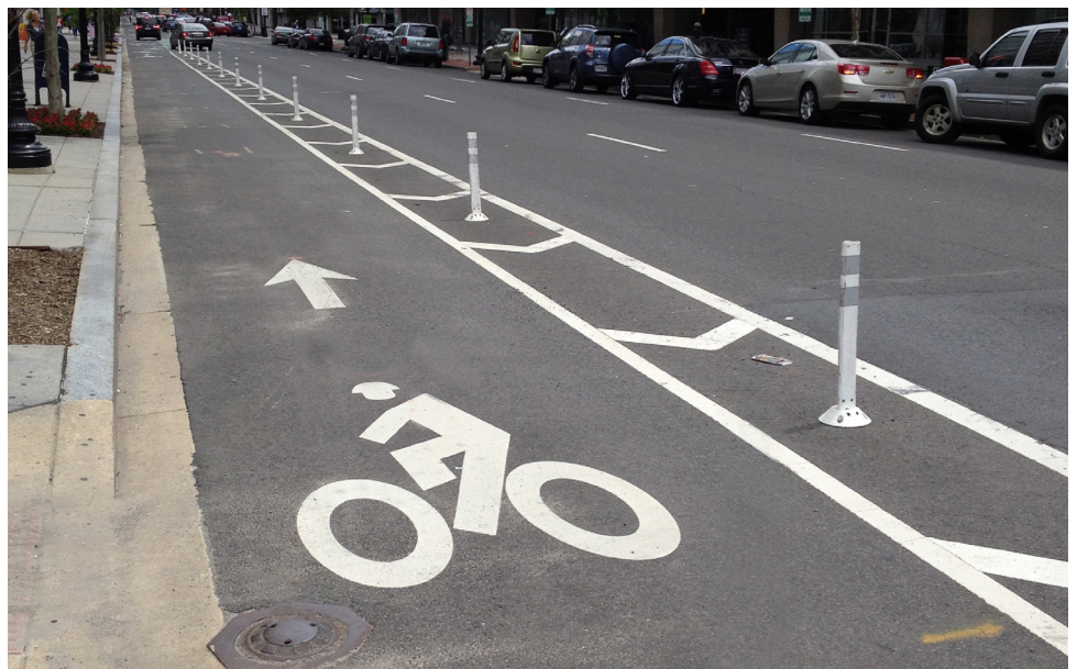
Inexpensive treatment with flexible delineator posts on L Street, Washington DC (Source: DDOT)
