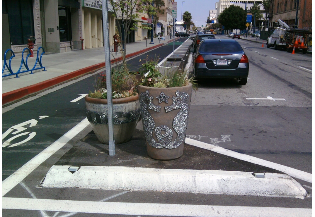
Long Beach, CA, has installed left-side, one-way separated bike lanes along a pair of one-way streets downtown. (Source: City of Long Beach)
