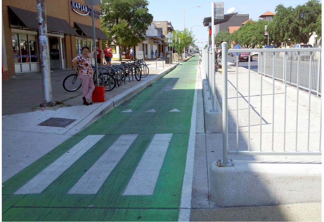
Island bus platform adjacent to a separated bike lane in Austin, TX. (Source: Kelly Blume)
