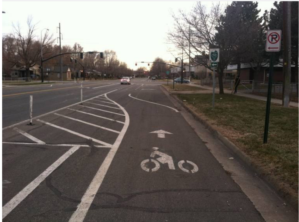
300 East Corridor separated bike lane. (Source: City of Salt Lake City)
