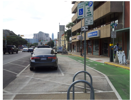
A reserved parking sign is placed alongside a floating parking lane in Austin, Texas (Source: Kelly Blume)
