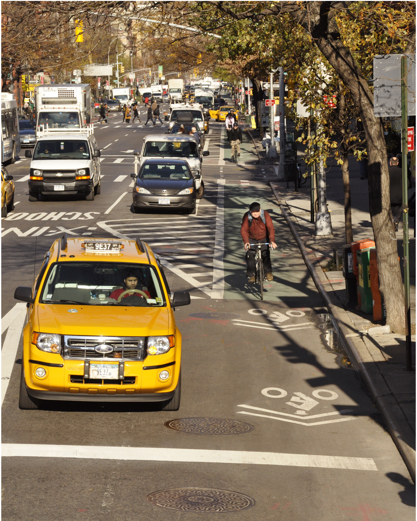
A mixing zone along New York City's 2nd Avenue separated bike lane. (Source: NYC DOT)
