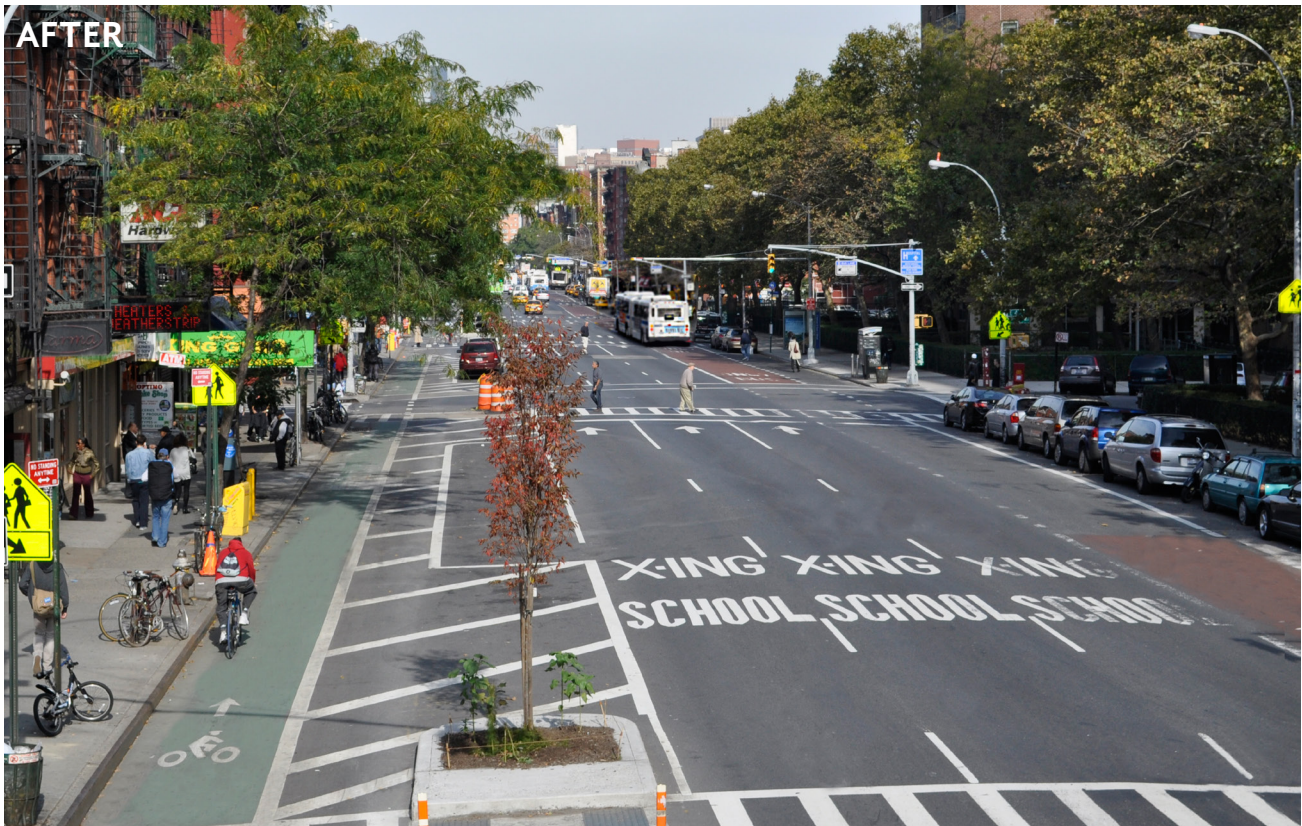
A Complete Streets retrofit has improved safety outcomes along 1st Avenue in New York City (Source: NYCDOT)
