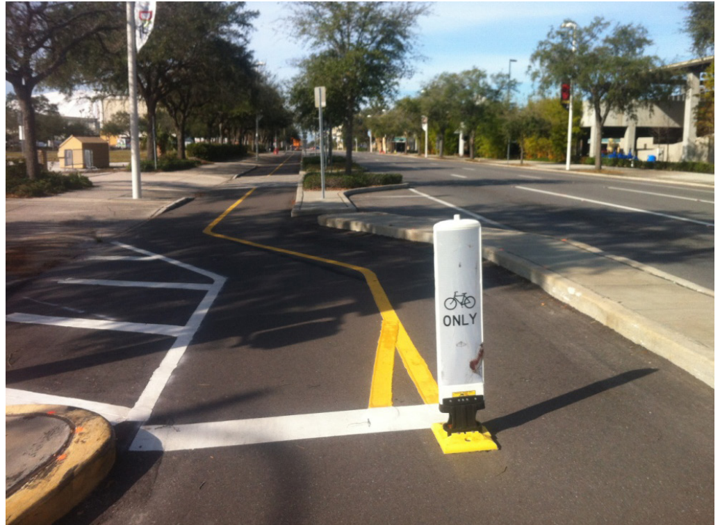
A bend-in design approaching an intersection in St. Petersburg, FL. (Source: Rory Rowan)
