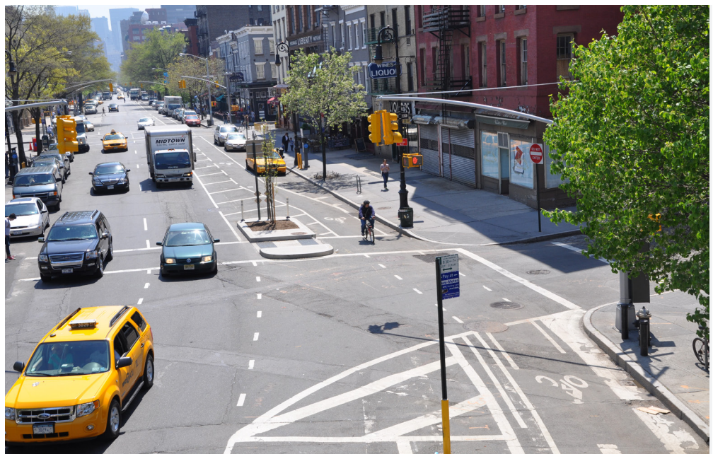
Transition from a buffered bike lane to separated bike lane on 8th Avenue in New York City, NY. (Source: NYC DOT)
