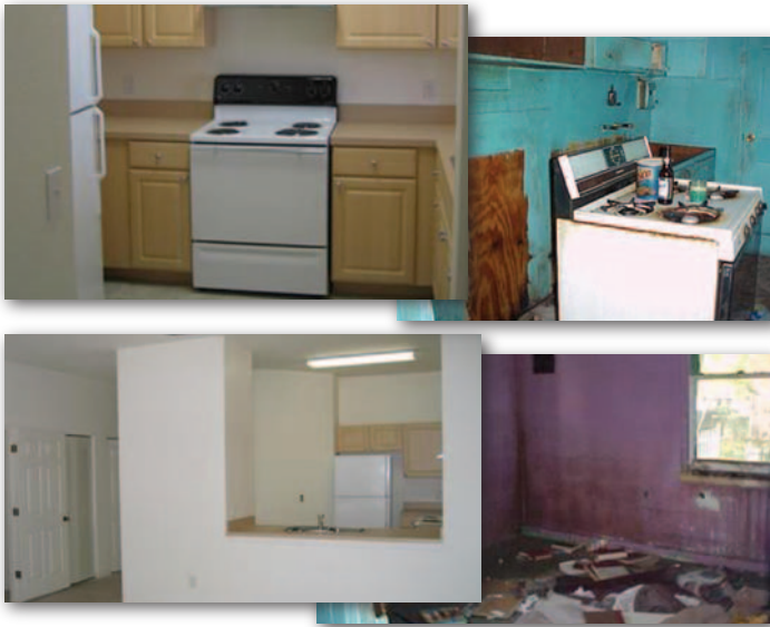
▲ Interior views of the Railroad Avenue Apartments before and after its restoration.
