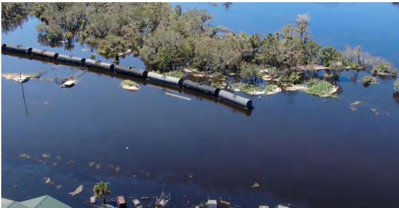
Figure 18: Railway flooding and damage in DeSoto County along the Peace River 90
