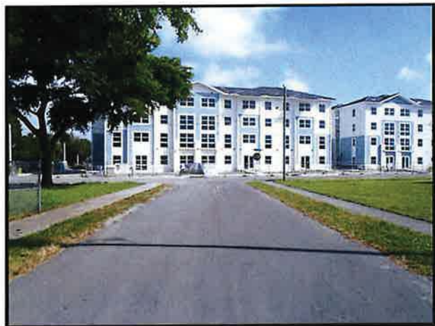
STREET SCENE OF SW 8TH AVENUE FACING NORTH
