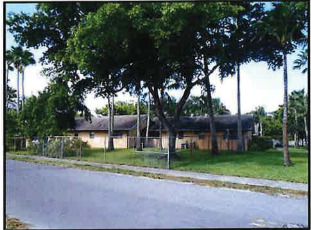
VIEW OF SUBJECT FACING SOUTHWEST
