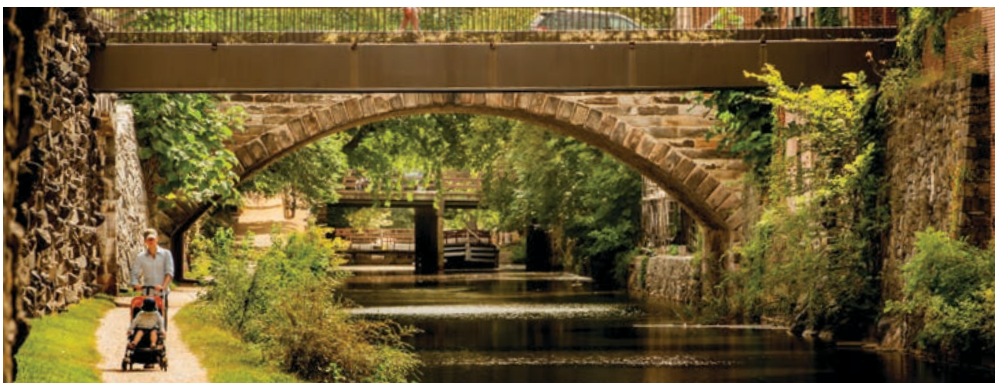
The revitalization of Georgetown’s one mile span of the 185-mile C&O Canal National Historic Park is a big focus of Georgetown 2028.
