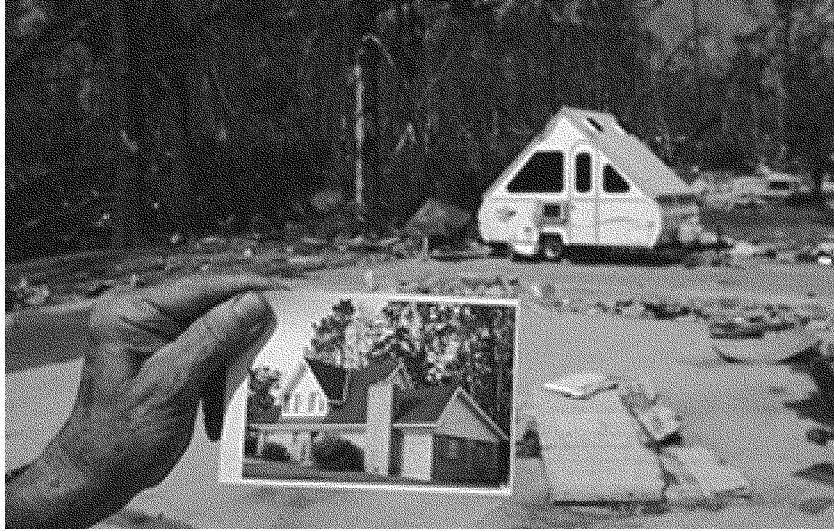
Figure 1. Only the foundation remains of a home in Waveland, Mississippi, after Hurricane Katrina. 9
