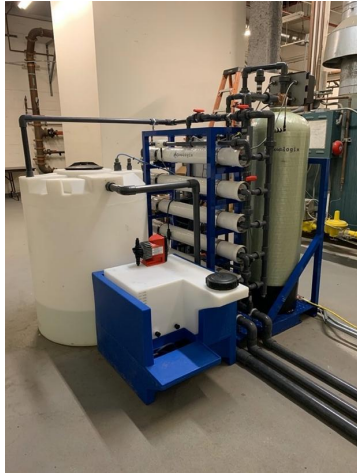
Blowdown recovery system Lloyd D. George U.S. Courthouse
