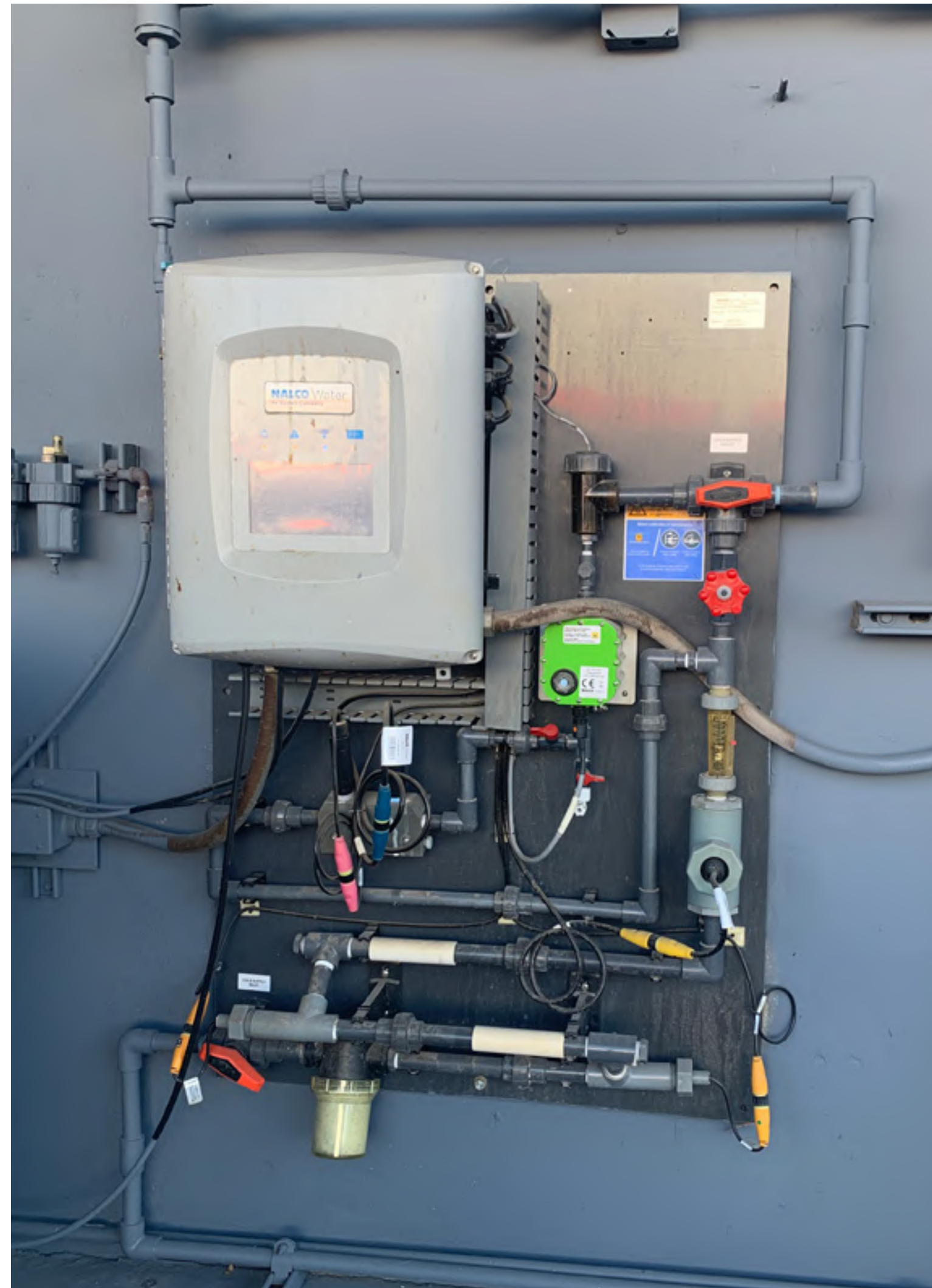
Cooling Tower Tempe, Ariz
