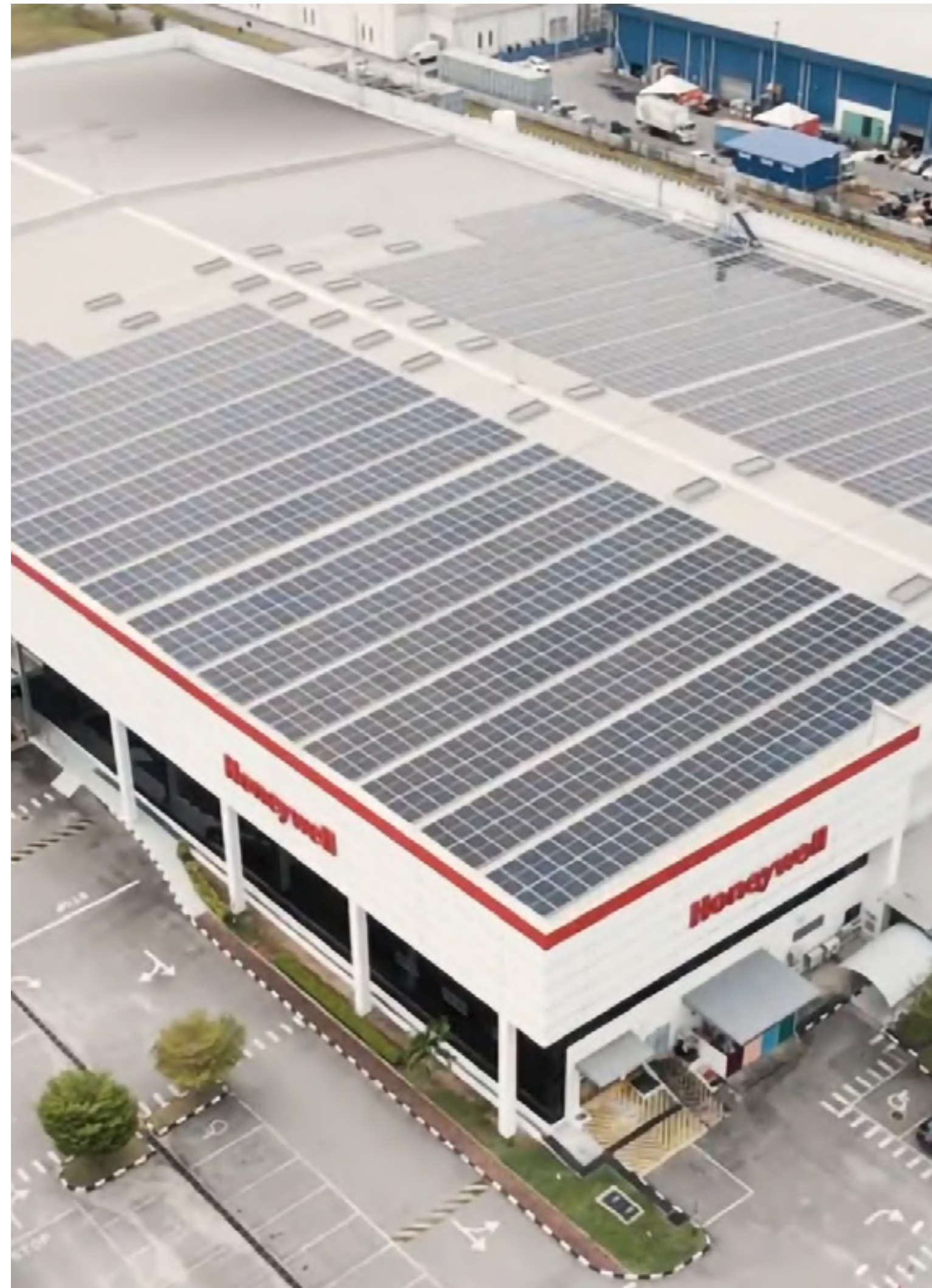
Solar panels in Penang, Malaysia
