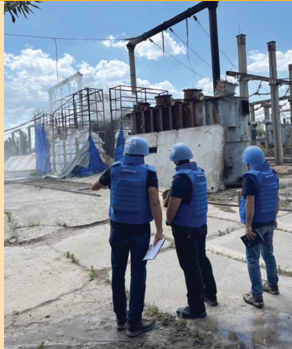
IAEA team observes the damage at the Raduga electrical substation (Photo: ZNPP)
