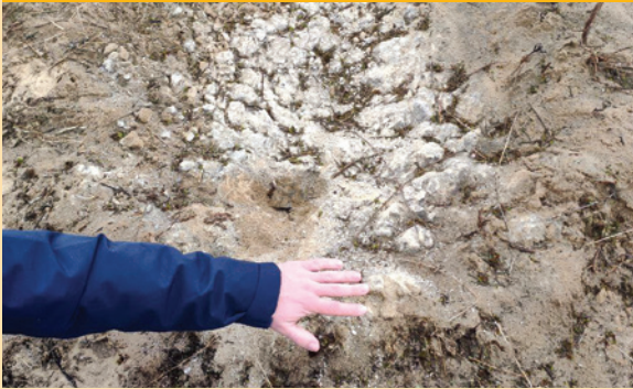
Small crater observed in the ground outside the wall surrounding the diesel fuel storage tanks (Photo: ZNPP)
