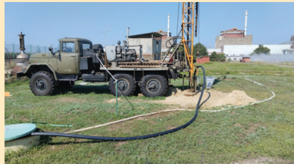
IAEA team observes the drilling of additional wells (Photo: ZNPP)
