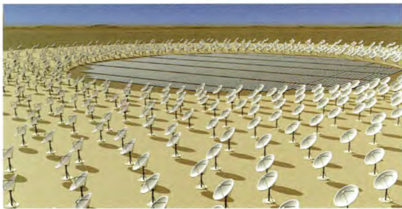
An artist's view of the central segment of the Square Kilometre Array (SKA), a next generation radio astronomy facility that will provide two orders of magnitude increase in the sensitivity over any existing radio telescope. The SKA reference design involves phased-array antennas for lower frequencies (the central part of the picture) and a large number of parabolic antennas for higher frequencies. Further details are available at www.skatelescope.org .
