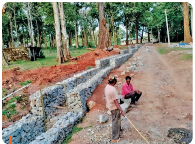
A gabion structure constructed at Nagarhole Tiger Reserve in Karnataka
