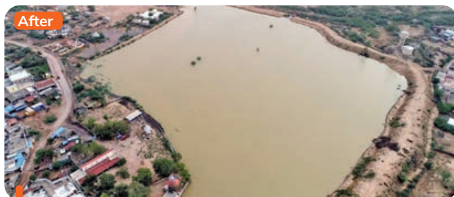
Desilting of a pond at Lodai village in Kachchh, Gujarat
