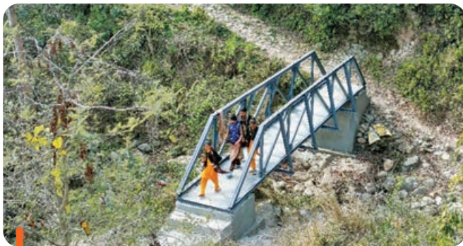
A pedestrian footbridge in Jammu and Kashmir
