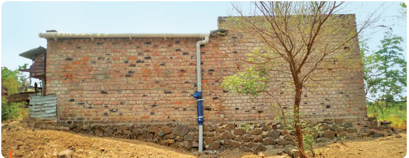
Rainwater harvesting pipe installed at Babhalgaon village in Dharashiv district, Maharashtra
