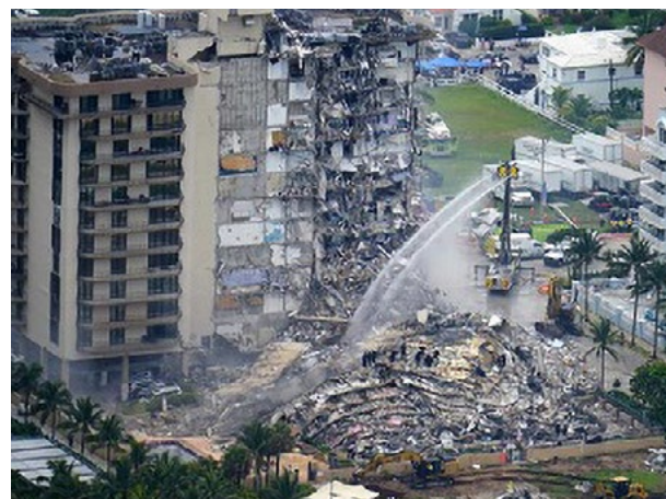
MIAMI FIELD OFFICE: The Homeland Security Investigations (HSI) manager overseeing the Champlain Towers investigation recognized Miami FO Group 40 for its support in helping track missing people from the building collapse in Surfside, Florida. Group 40's efforts resulted in them being able to quickly locate all 40 people and/or their family members.
