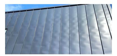
Oil canning is a cosmetic phenomenon that has no impact on the structural integrity of the roof and often diminishes over time as metal settles and adapts. However, when metal roofing resurged in popularity in the 1980s, some homeowners were not prepared for this effect and complained, causing roofing manufacturers to develop ribbed panels as an alternative that would be less likely to flex.
