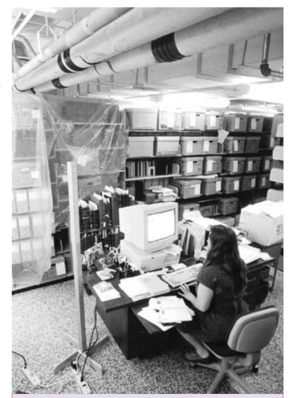
The Special Collections Department is one of the library areas suffering from deterioration and insufficient storage facilities. Overhead pipes are taped to stop leaks, and plastic sheets cover areas of collection storage to protect the materials from damage.
