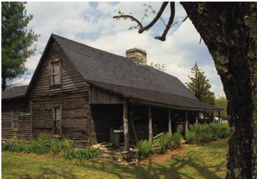
Gragg House, Watauga County, North Carolina. The house was constructed in the mid-nineteenth century and provides one of the state's finest examples of dovetailed plank construction. It is listed on the National Register of Historic Places. Photograph by Tim Buchman, 1988. Reproduction and use of this material requires permission from Preservation North Carolina.
