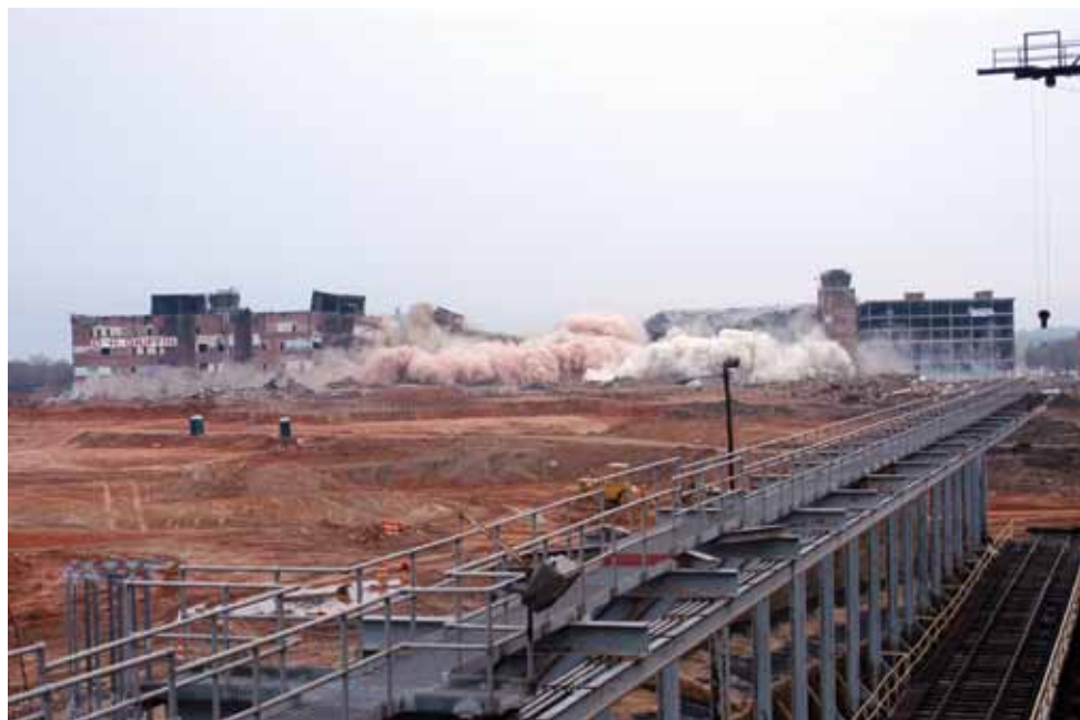
The Towel Distribution Center implosion, March 24, 2008.
