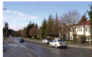
Figure 30. Most side streets lack sidewalks on at least one side.
