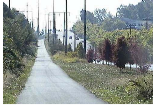
Figure 34. Existing conditions on the Interurban Trail.
