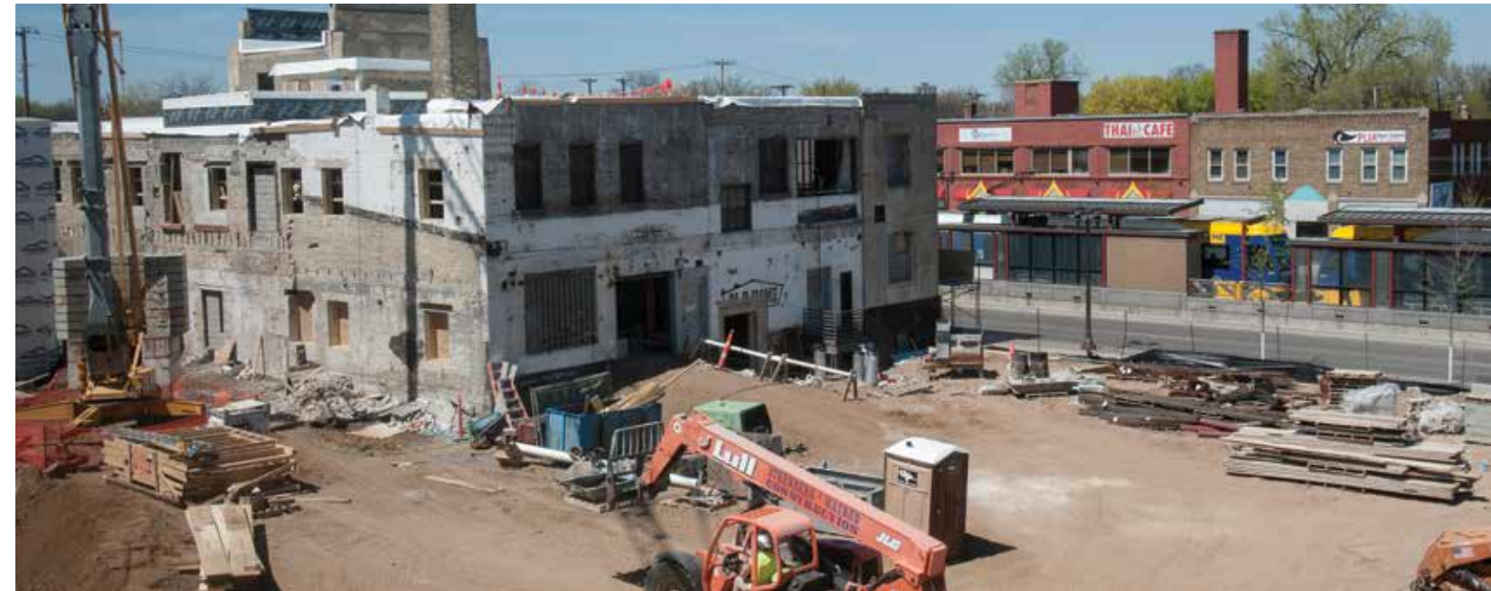
Construction of Western U Plaza in 2015.
