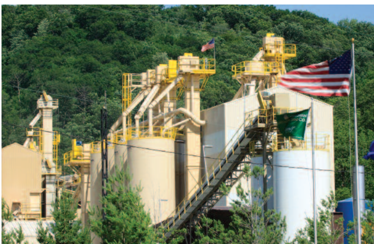
Wisconsin Industrial Sand recently expanded its facility in Maiden Rock.
