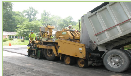
Typical hot mix asphalt paving operation
