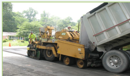
Typical hot mix asphalt paving operation
