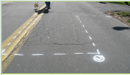
Typical survey paint markings
