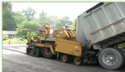
Typical hot mix asphalt paving operation
