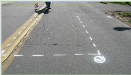
Typical survey paint markings
