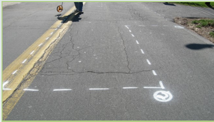
Typical survey paint markings
