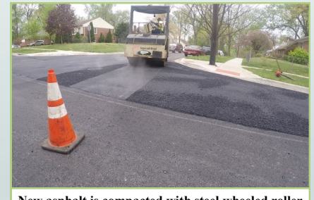
New asphalt is compacted with steel wheeled roller
