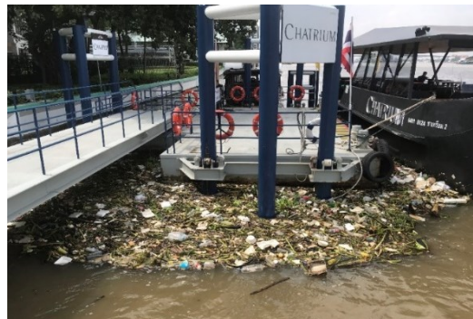
Figure 4.2 Example of structure that allows constant accumulation
