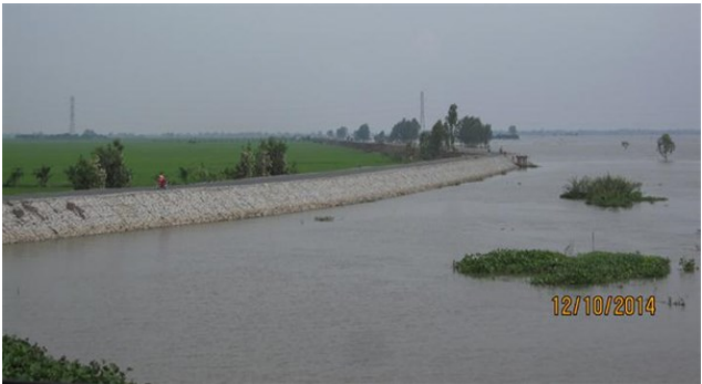
Figure 3.7. Example of a disconnected floodplain
