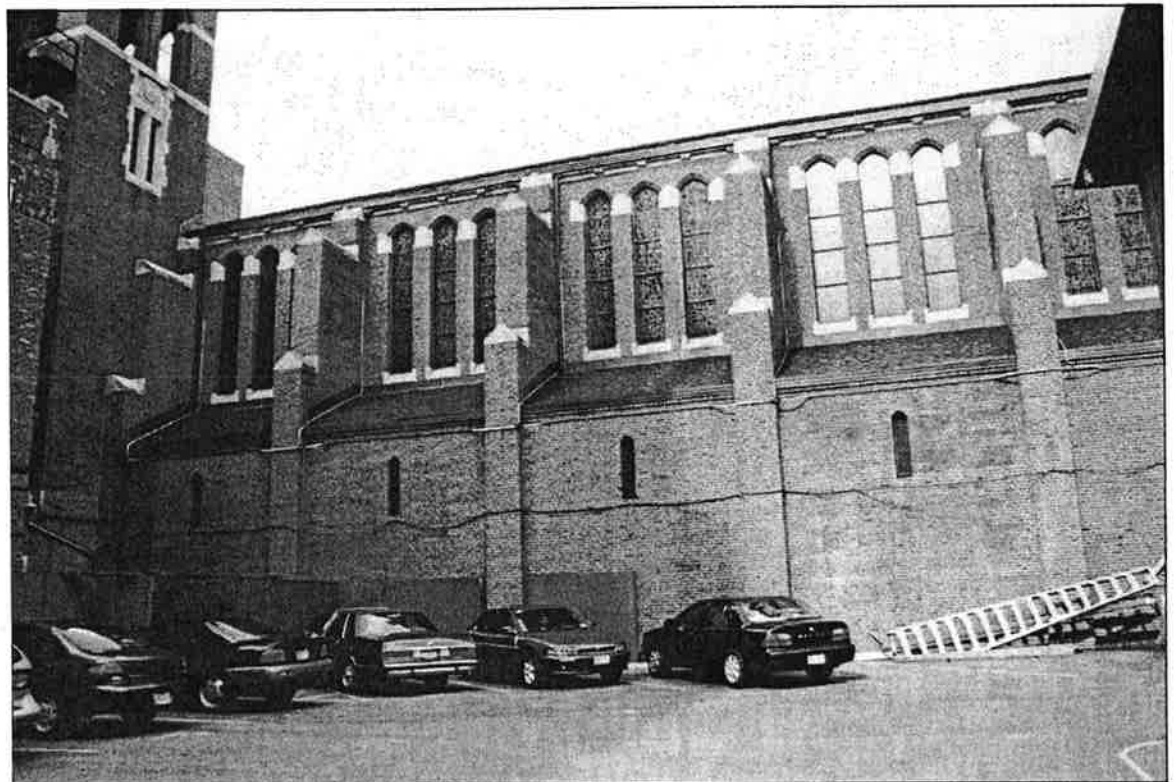
Existing shadows on east facade of St. Catherine of Siena. 10:15 am
