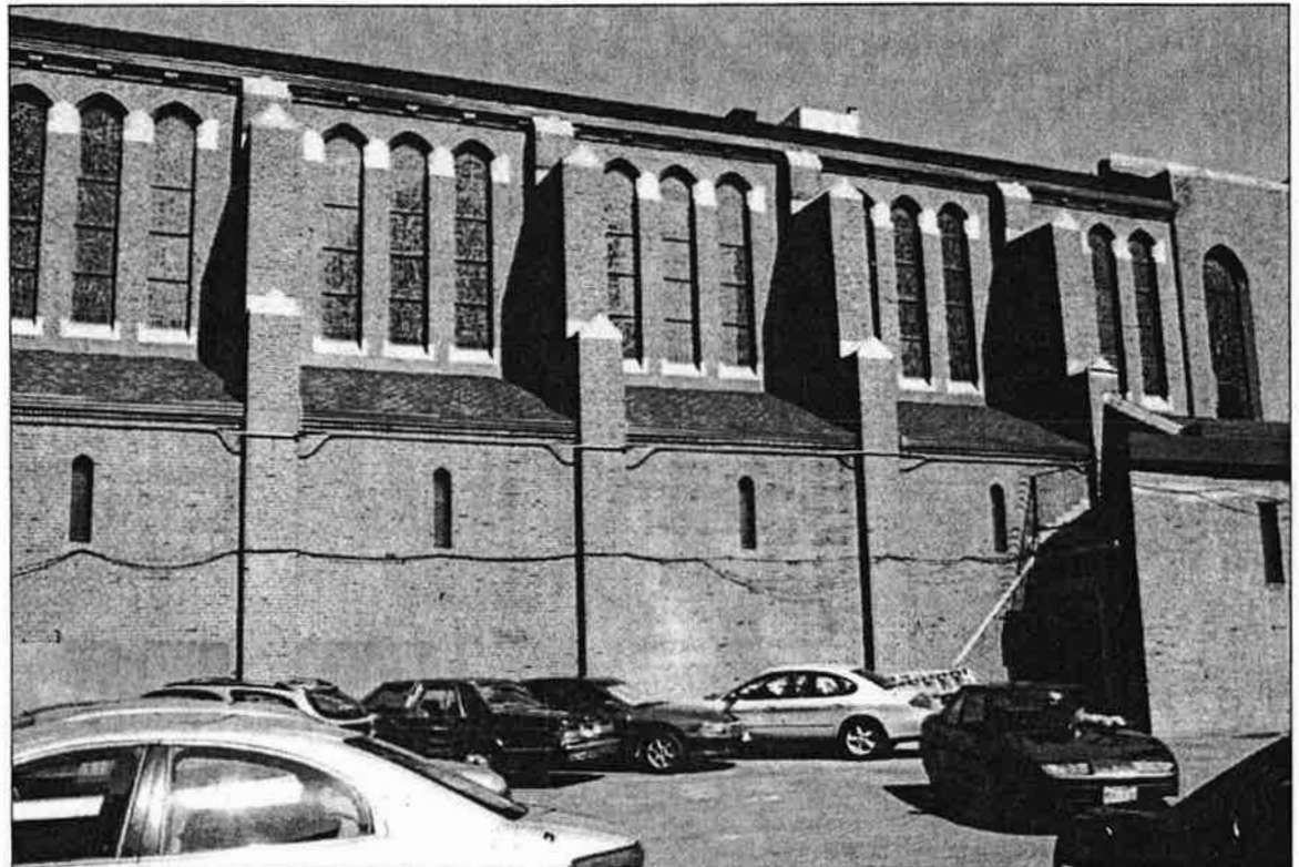
Existing shadows on east facade of St. Catherine of Siena. 10:00 am
