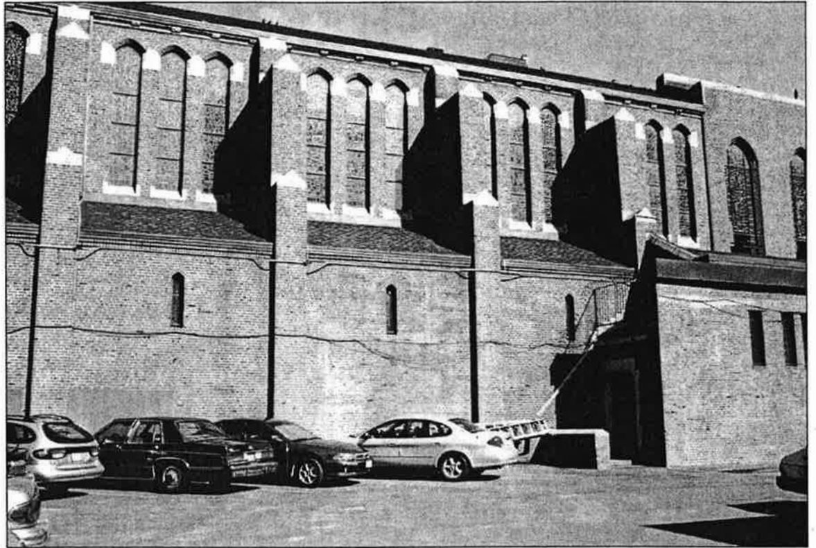
Existing shadows on east facade of St. Catherine of Siena. 9:00 am
