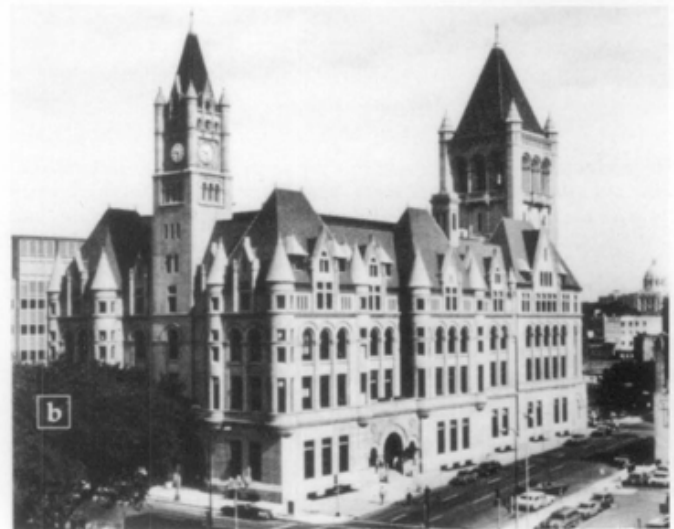
Figure 5. (a) Clay tile was a popular roofing material during the Romanesque Revival period, not only for residential structures including these rowhouses in the Dupont Circle Historic District in Washington, D.C., and designed and built by Thomas F. Schneider between 1889-1892, but also for large-scale public buildings such as (b) the Old Federal Courts Building (1894-1901) in St. Paul, Minnesota, designed by Willoughby J. Edbrooke. Photo: (a) Anne Grimmer, and (b) Winsor/Farcy Architects.
