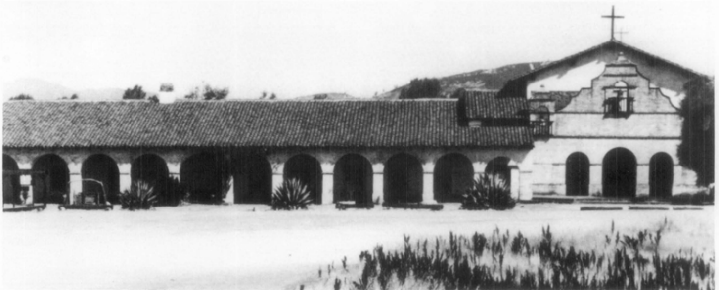
Fig. 3. Clay tiles were first produced on the west coast in 1780 at Mission San Antonio de Padua in Monterey County, California. The present church shown here dates from 1810. Photo: Gene Falk.
