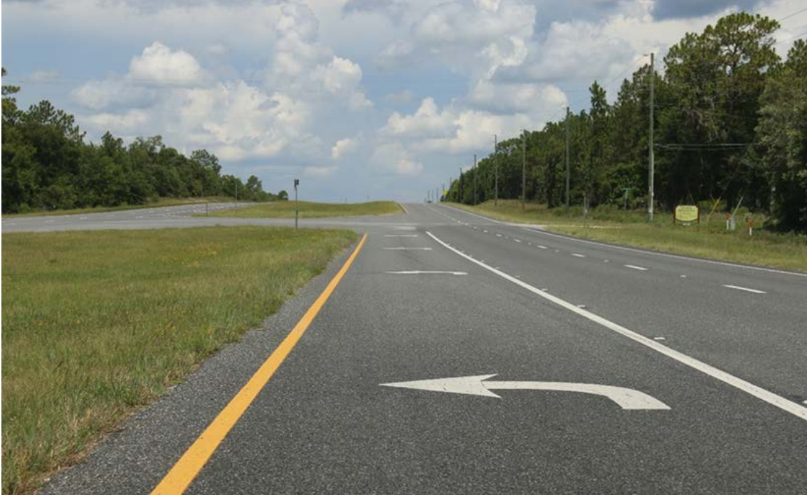
Figure 3. Approach to the crash scene from the US-27A westbound left turn lane, looking west as viewed from the truck's route of travel.
